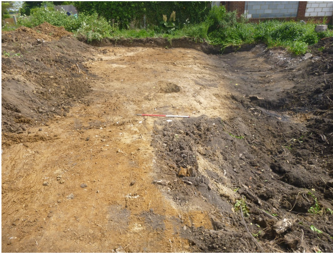
Photograph 5 Completed east plot, with pit F1 seen in the centre, and pipe trench F2 seen in background to the right, view east.
