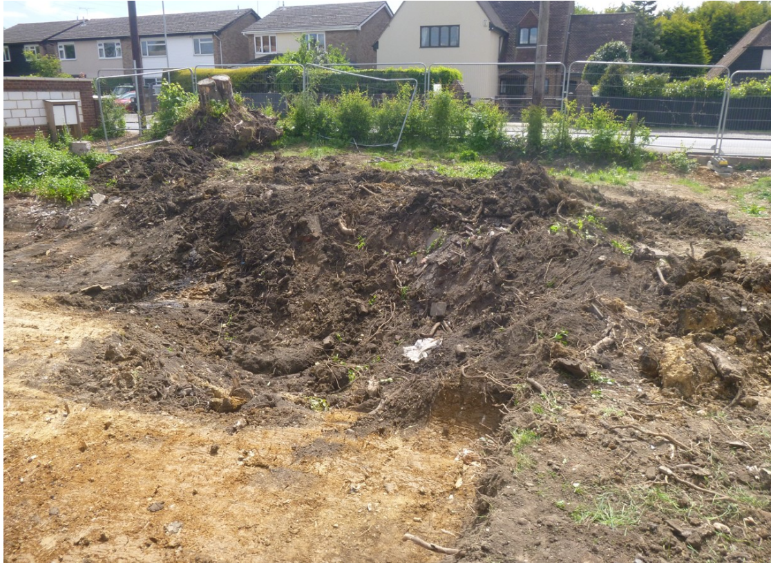
Photograph 4 Area of disturbance caused by tree removal in east plot, view south.
