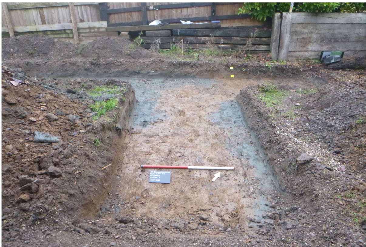
Photograph 5 The trench, looking north-west.
