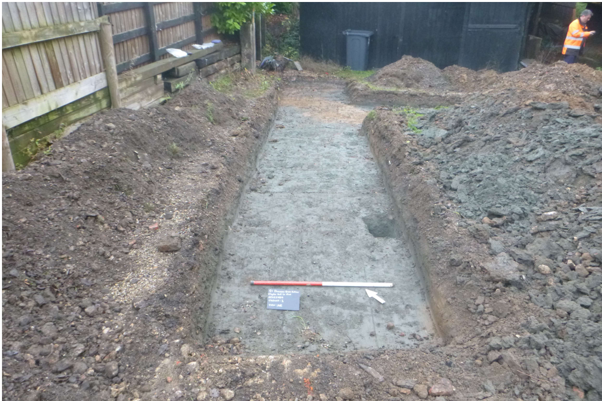
Photograph 3 The trench, with hand excavated slot through staining in L2, looking north-east.
