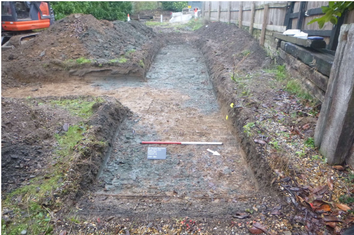
Photograph 1 The trench, looking south-west.
