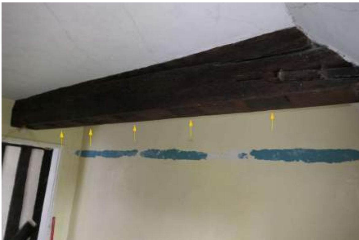
Photograph 47 Detail of reused tie-beam in ceiling of bedroom 5, yellow arrows highlight shallow mortices. Photograph taken facing south.
