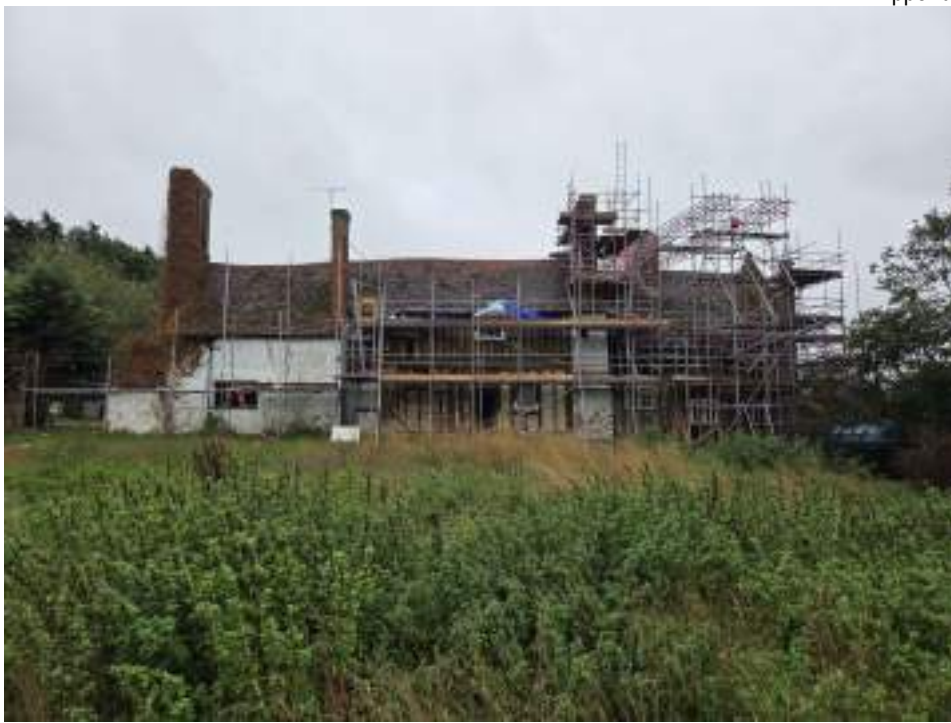
EEX62136_PhotoGraph_041 North-western elevation (ranges 1, 2, 5 and 6). Photograph taken facing south-east.
