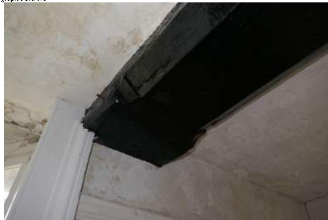
EEX62136_Photograph_138 Detail of curved stepped stop on chamfered binding beam in ceiling of living room. Photograph taken facing south.
