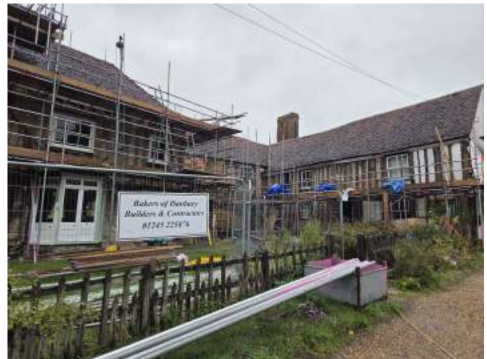
EEX62136_Photograph_020 South-eastern and south-western elevation (ranges 4, 5 and 7). Photograph taken facing north.
