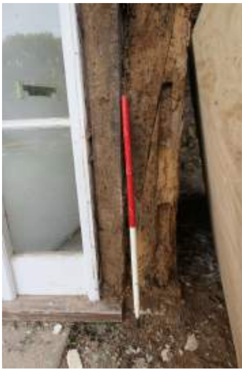
EEX62136_Photograph_049 Detail of reused post visible on south-eastern elevation (range 4). Photograph taken facing north-west.
