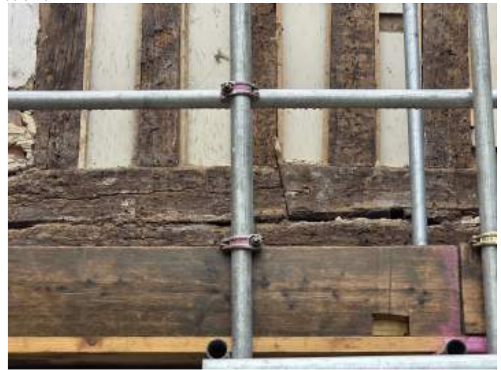
EEX62136_Photograph_026 Detail of scarf-joint in girding beam and possible carpenters marks on studs in south-eastern elevation (range 5). Photograph taken facing north-west.
