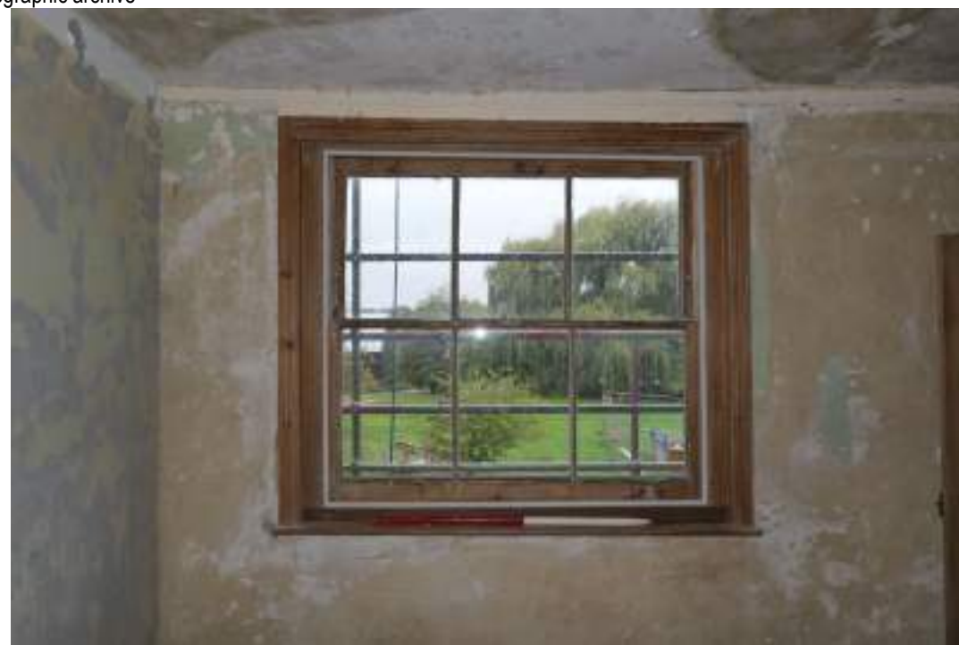
EEX62136_Photograph_190 Detail of window in south-eastern wall of bedroom 2. Photograph taken facing south-east.
