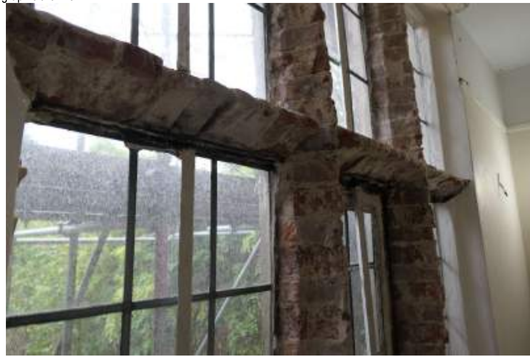
EEX62136_PhotoGraph_154 Detail of brick mullions and transoms in window in south-western wall of dining room. Photograph taken facing west.
