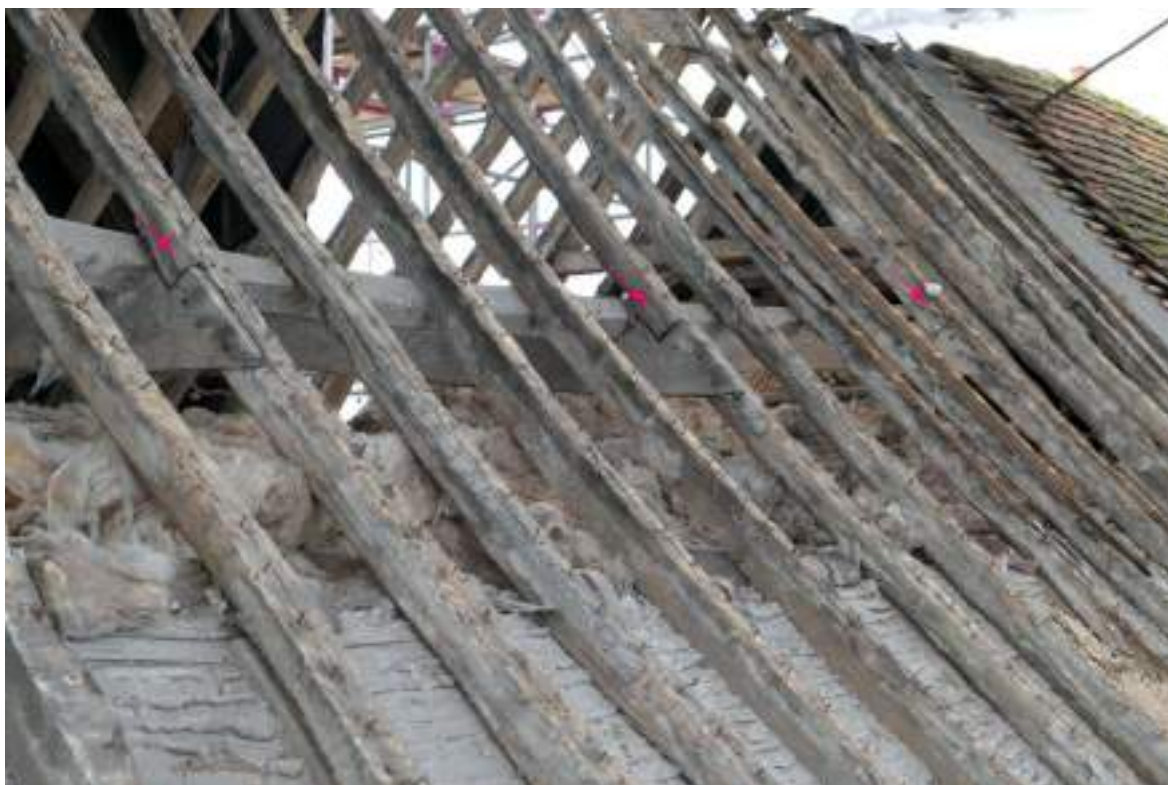
Photograph 21 Roof timbers covering range 6. Pink arrows pointing to lap-dovetail joints securing the collars. Photograph taken facing south.
