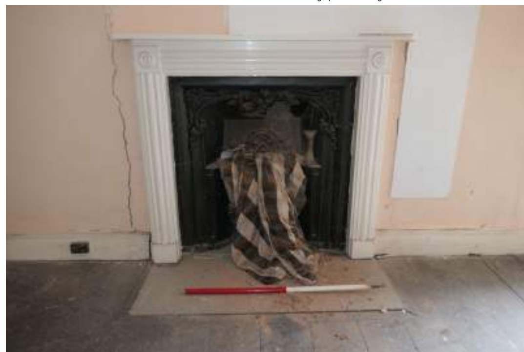
EEX62136_Photograph_216 Detail of fireplace in north-eastern wall of bedroom 6. Photograph taken facing north-east.
