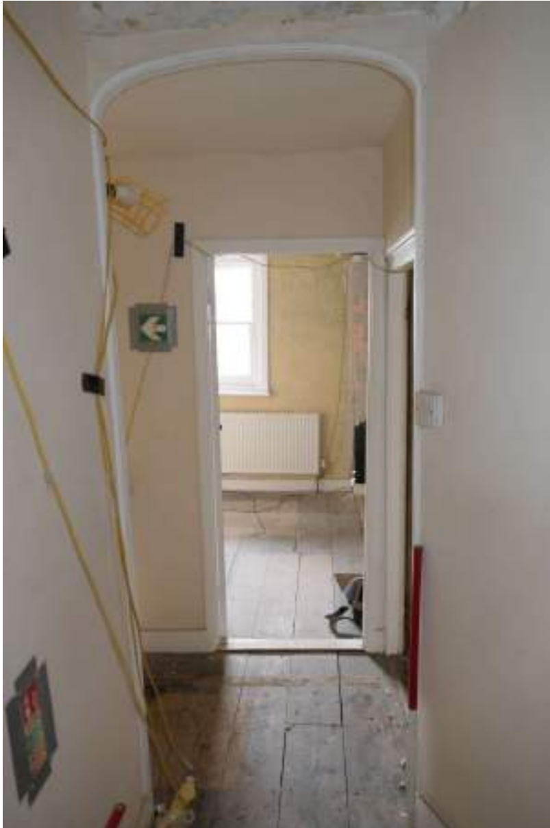
Photograph 40 Detail of arched doorway in corridor 3. Photograph taken facing south-east.
