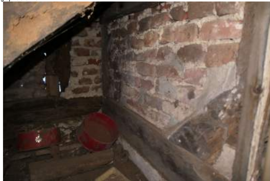
EEX62136_Photograph_090 Detail of brickwork beneath rear stairs. Photograph taken facing north.
