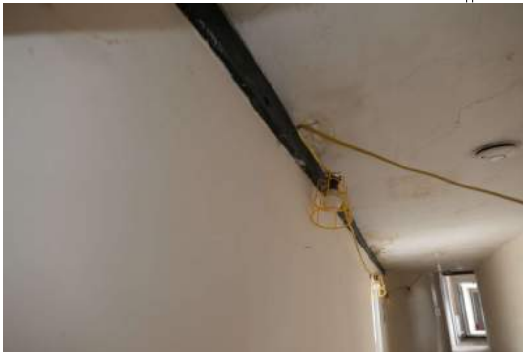
EEX62136_Photograph_169 Detail of exposed wall-plate in corridor 3. Photograph taken facing north.
