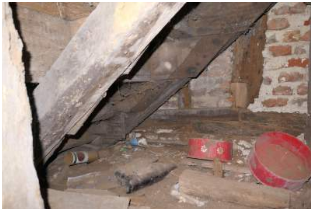
EEX62136_Photograph_091 Detail of rear stairs from beneath. Photograph taken facing west north-west.
