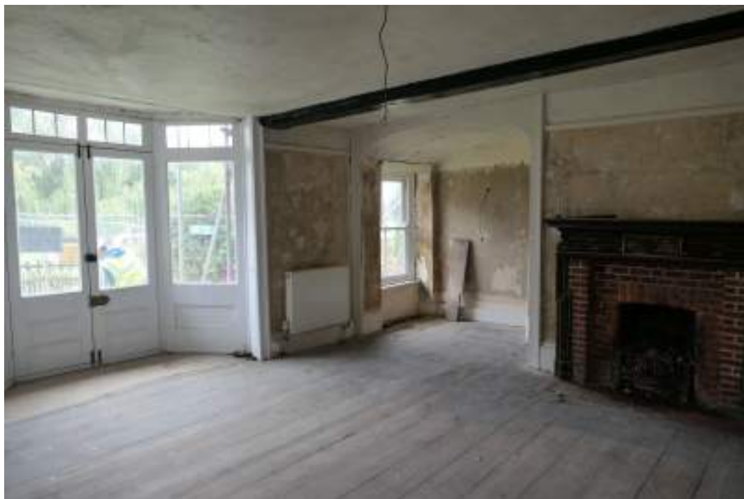
EEX62136_Photograph_131 Interior of living room. Photograph taken facing west.
