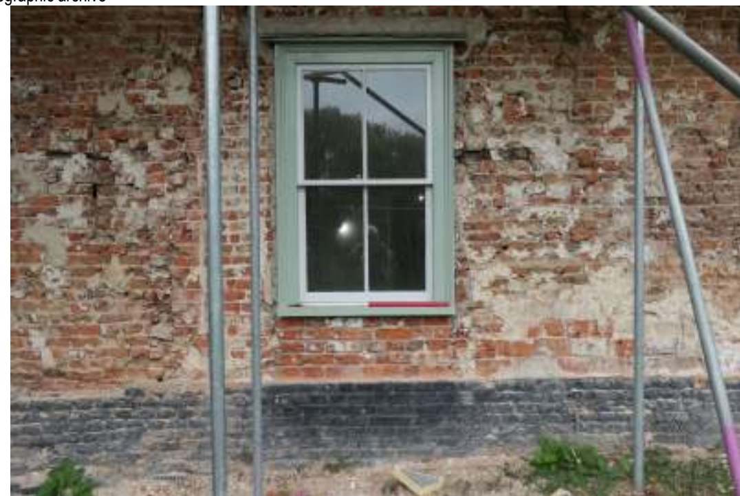
EEX62136_PhotoGraph_014 Detail of brickwork and window in south-eastern elevation (range 3). Photograph taken facing north-west.
