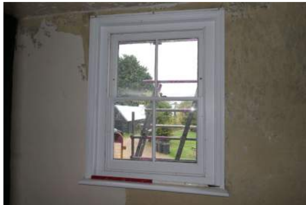
EEX62136_Photograph_196 Detail of window in south-eastern wall of bedroom 3. Photograph taken facing east south-east.
