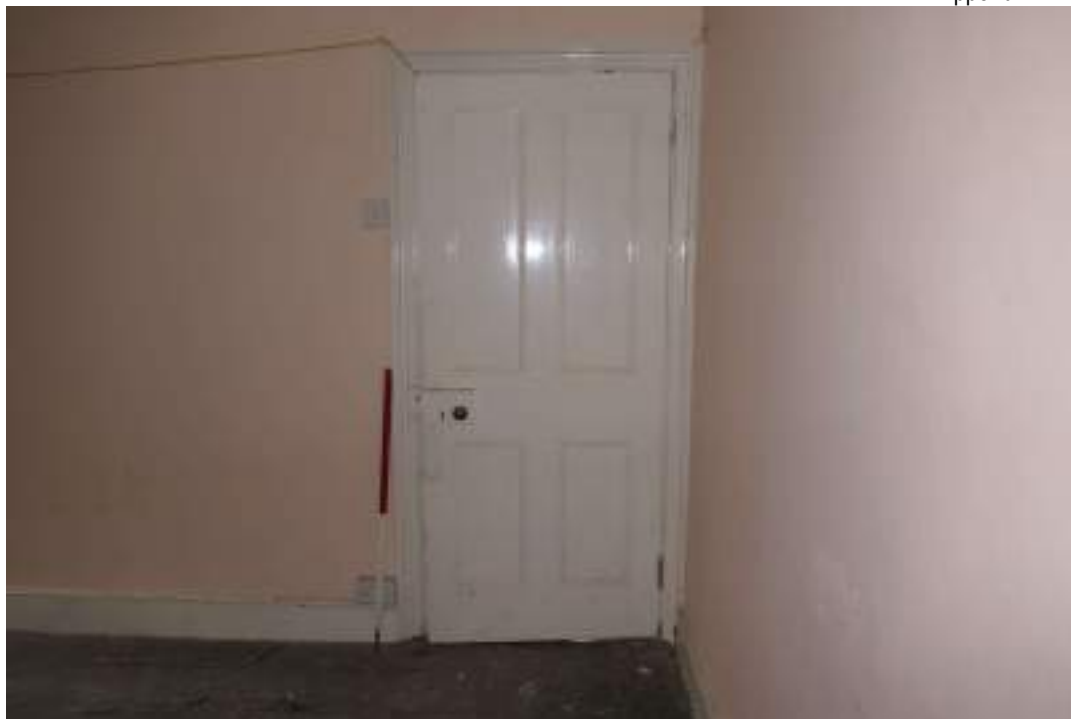
EEX62136_Photograph_217 Detail of door in south-eastern wall of bedroom 6. Photograph taken facing south-east.
