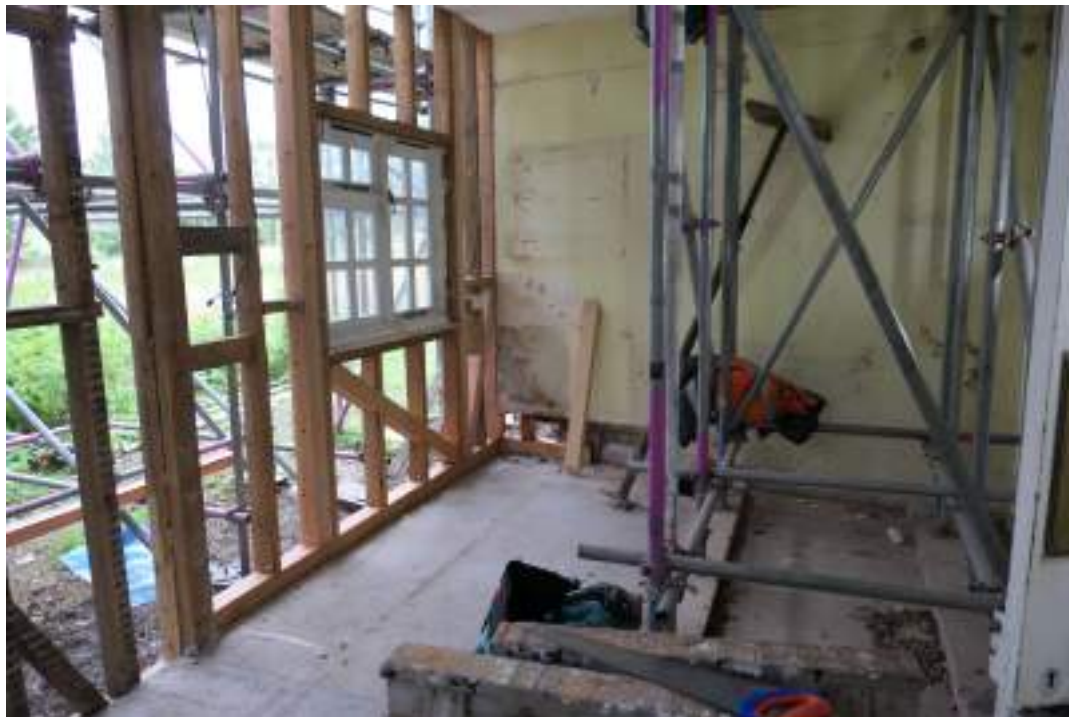
EEX62136_PhotoGraph_155 Interior of kitchen. Photograph taken facing north.
