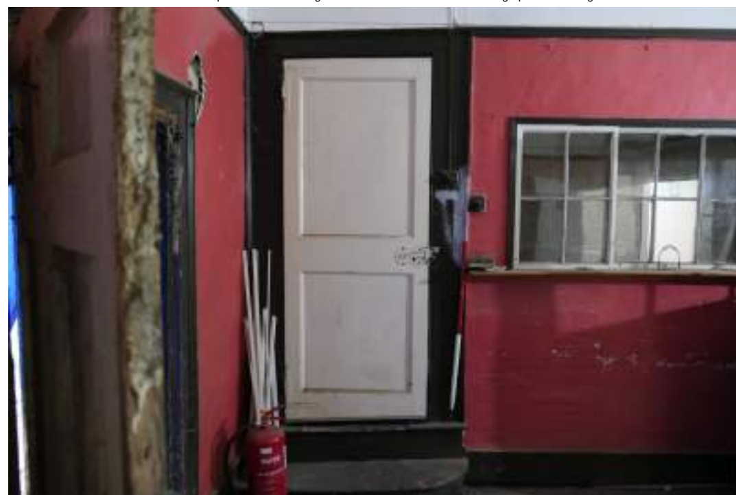
EEX62136_Photograph_100 Detail of door in north-eastern wall of office. Photograph taken facing north-east.
