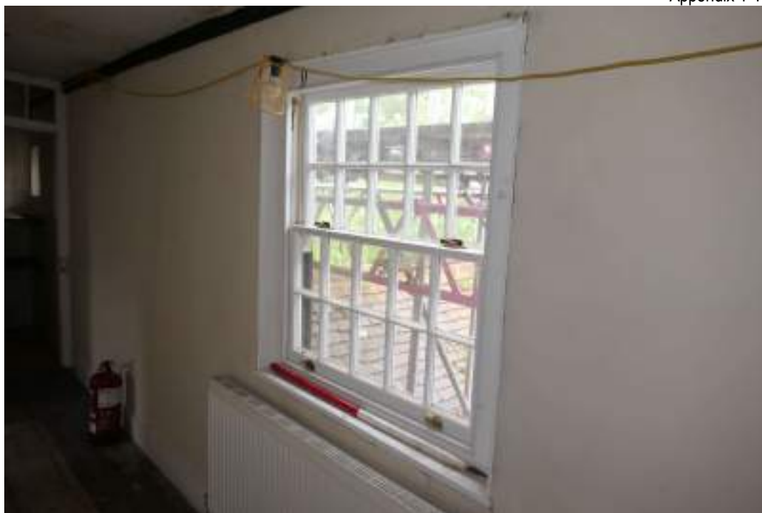
EEX62136_Photograph_165 Detail of window in north-western wall of corridor 3. Photograph taken facing west.
