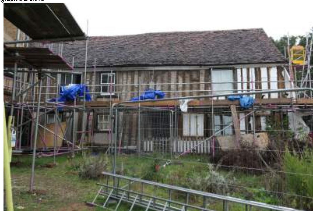
EEX62136_Photograph_054 South-western elevation (range 7). Photograph taken facing north-east.
