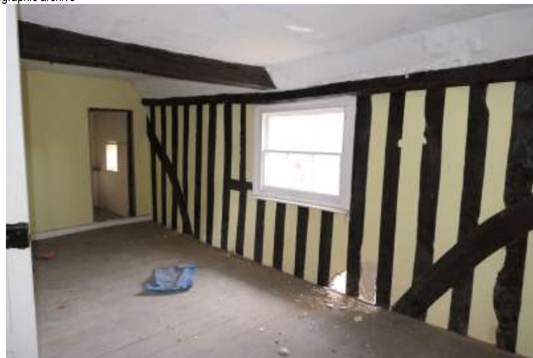
EEX62136_Photograph_226 Interior of bedroom 4. Photograph taken facing west.
