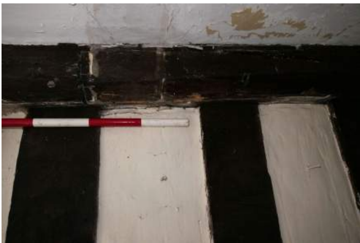
Photograph 42 Detail of scarf-joint in wall-plate in south-eastern wall of corridor 4. Photograph taken facing south-east.
