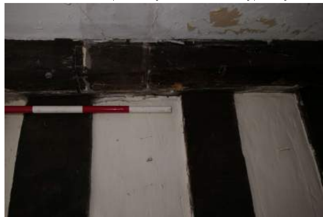
EEX62136_Photograph_204 Detail of scarf-joint in wall-plate in south-eastern wall of corridor 4. Photograph taken facing south-east.
