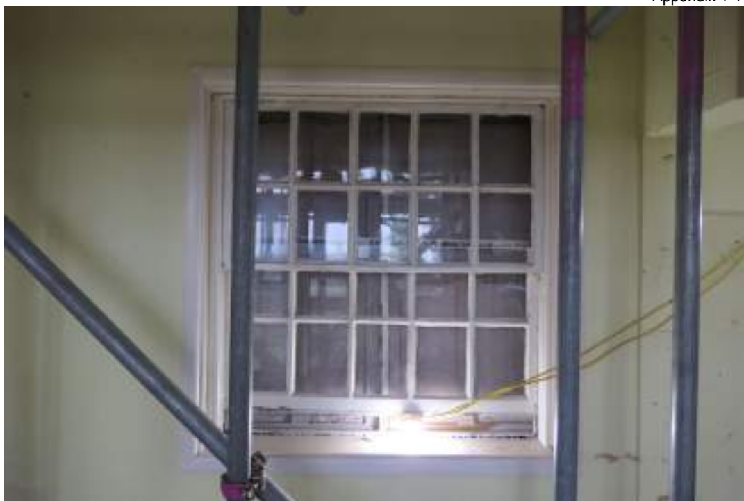
EEX62136_Photograph_157 Detail of window in south-eastern wall of kitchen. Photograph taken facing south-east.
