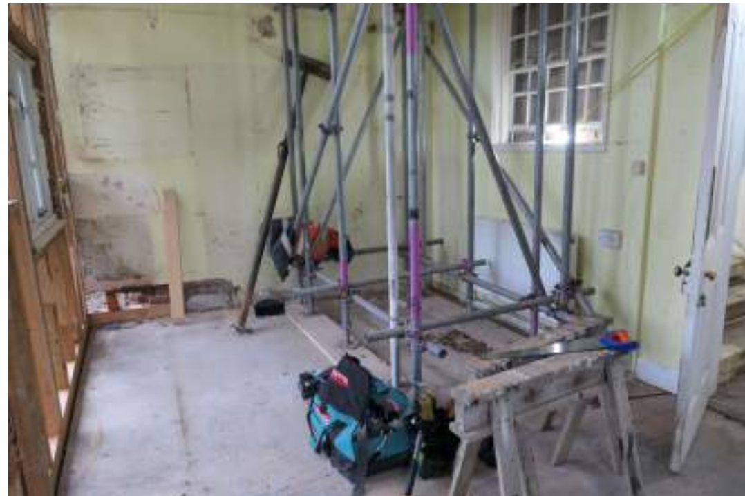
EEX62136_PhotoGraph_156 Interior of kitchen. Photograph taken facing south-east.
