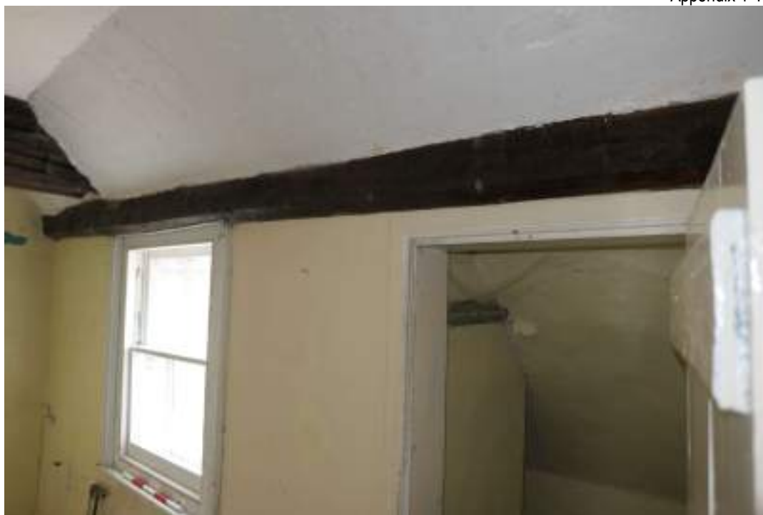
EEX62136_Photograph_225 Detail of exposed wall-plate in north-western wall of bedroom 5. Photograph taken facing west north-west.
