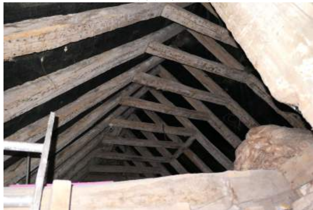
EEX62136_Photograph_056 Detail of roof construction above bedroom 1. Photograph taken facing west.
