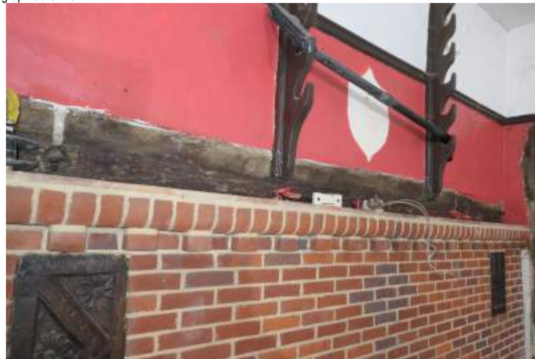
EEX62136_Photograph_106 Detail of exposed timber mantle in south-western wall of office. Photograph taken facing west.
