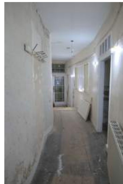
EEX62136_Photograph_110 Interior of corridor 1. Photograph taken facing south-west.
