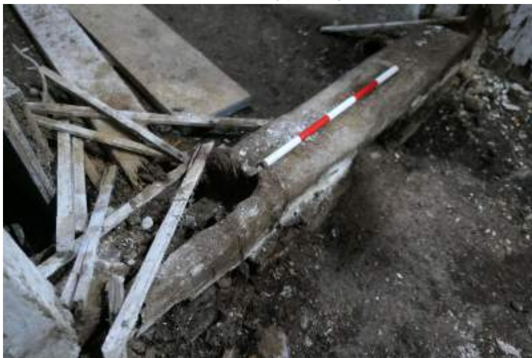
EEX62136_PhotoGraph_243 Detail of reused sill-beam in basement. Photograph taken facing south.
