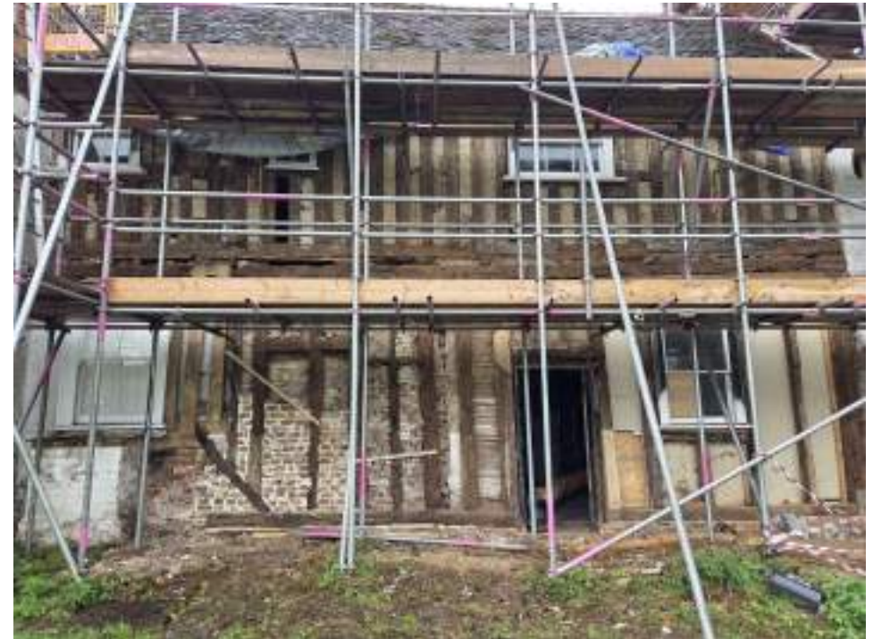
EEX62136_Photograph_028 Detail of exposed timber-framing of north-western elevation (range 5). Photograph taken facing south-east.
