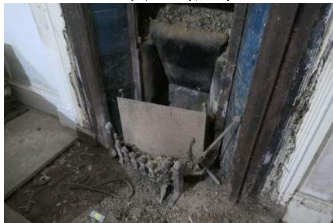
EEX62136_Photograph_084 Detail of fire grate in fireplace in north-western wall of spare room 2. Photograph taken facing west north-west.
