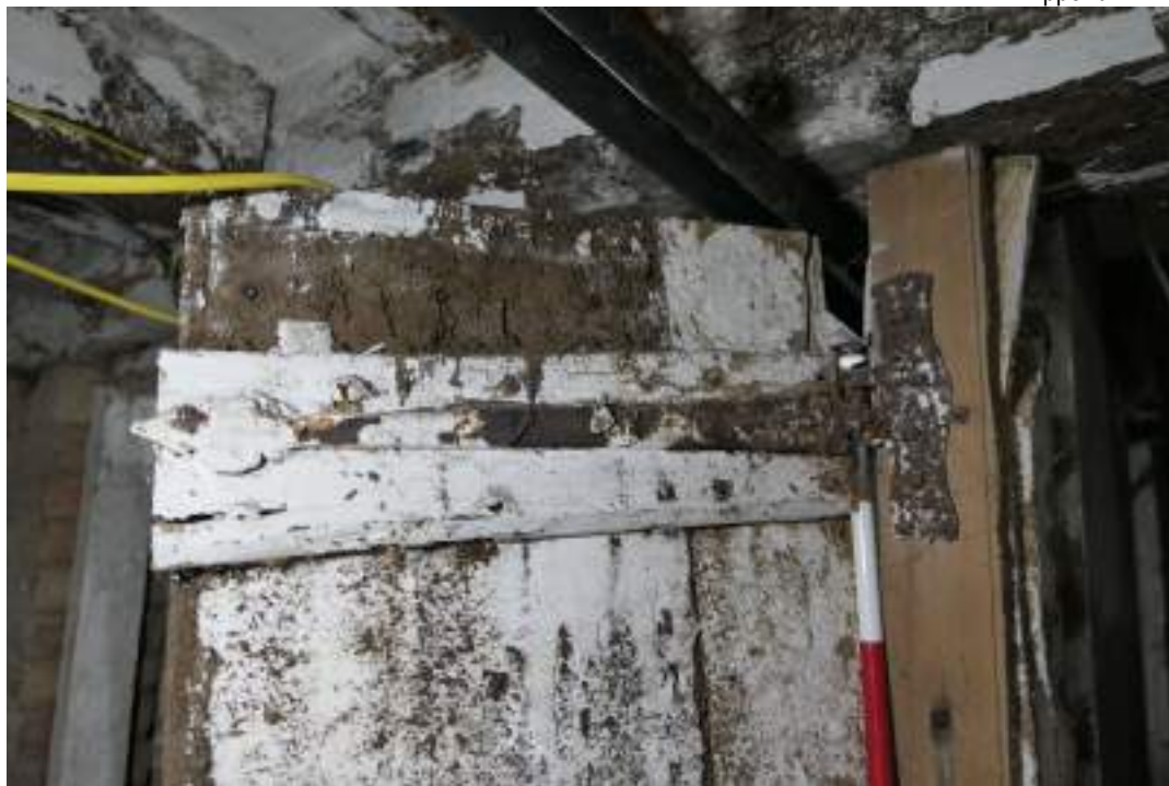
EEX62136_Photograph_245 Detail of strap hinge on door in basement. Photograph taken facing north.
