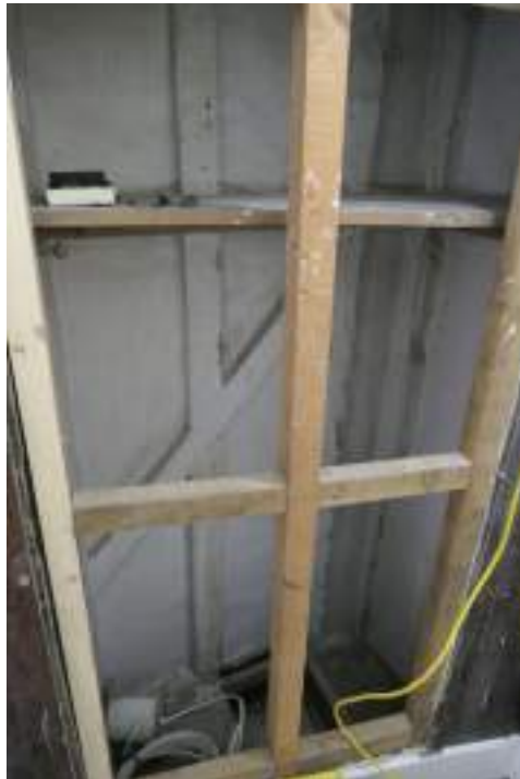
EEX62136_Photograph_255 Detail of hidden alcove in south-eastern wall of corridor 4. Photograph taken facing south-east.
