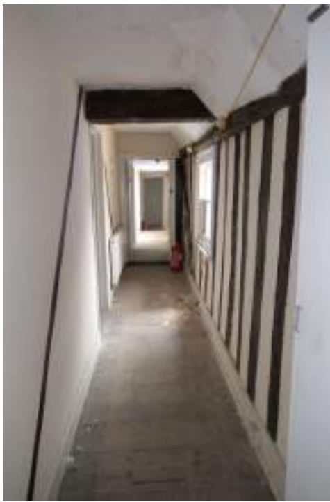
EEX62136_PhotoGraph_197 Interior of corridor 4. Photograph taken facing north-east.
