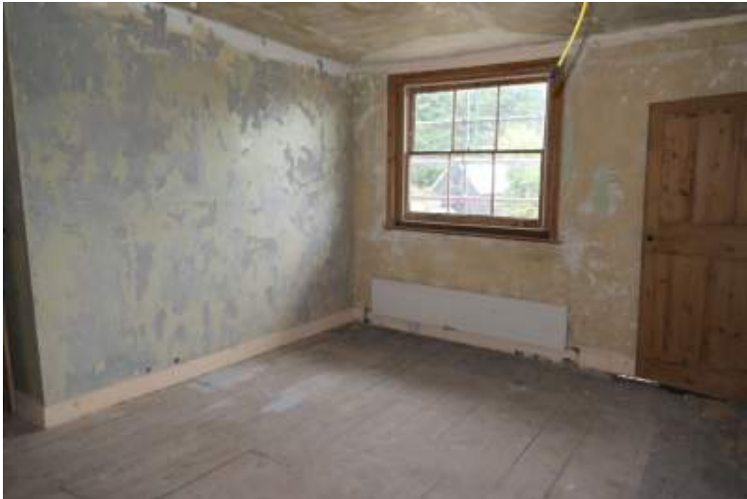
EEX62136_Photograph_183 Interior of bedroom 2. Photograph taken facing east.
