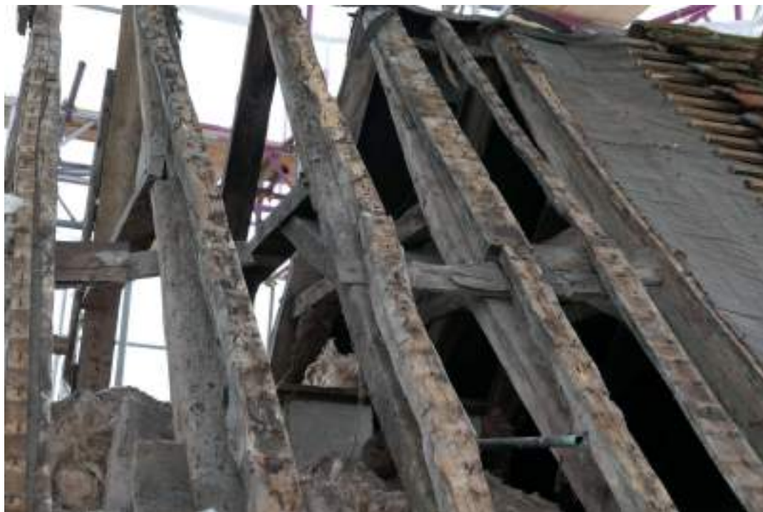
EEX62136_Photograph_063 Detail of roof construction above range 5. Photograph taken facing south south-east.
