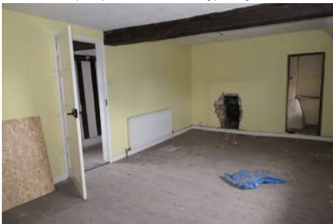
EEX62136_Photograph_227 Interior of bedroom 4. Photograph taken facing south.
