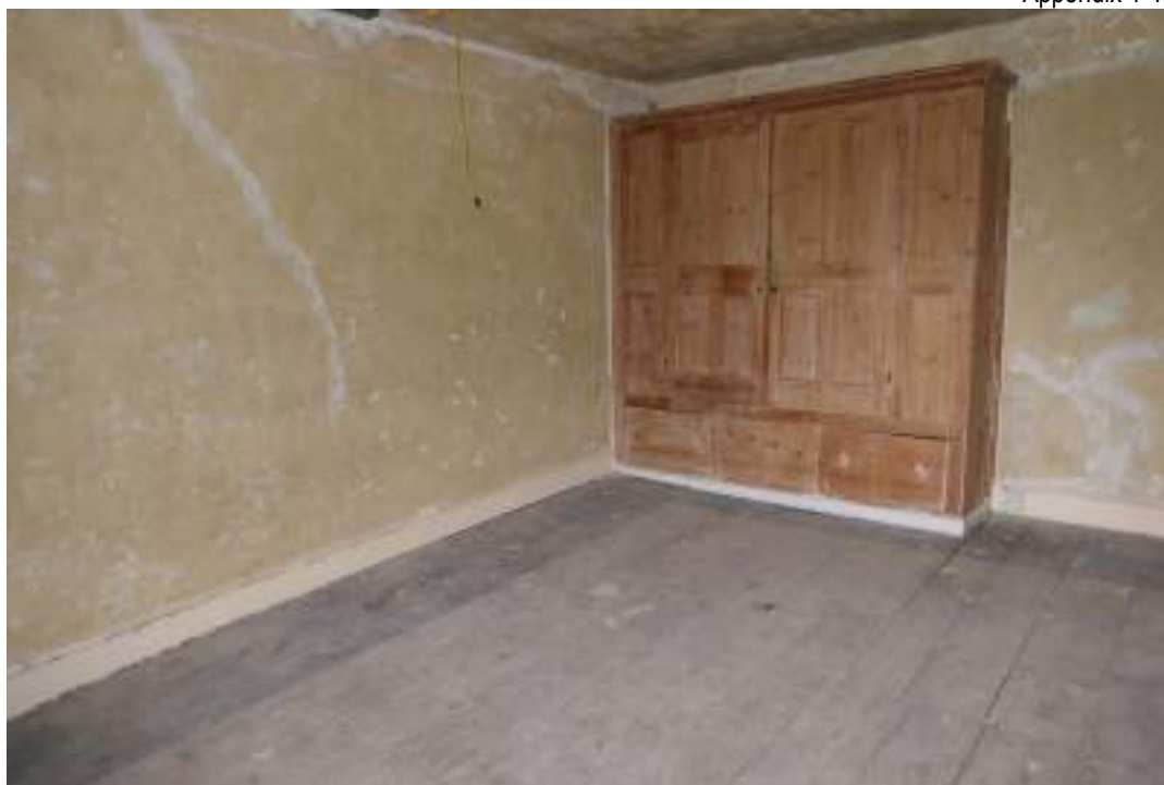
EEX62136_Photograph_185 Interior of bedroom 2. Photograph taken facing west.
