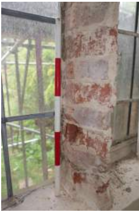
EEX62136_PhotoGraph_153 Detail of brick mullion in window in south-western wall of dining room. Photograph taken facing west.
