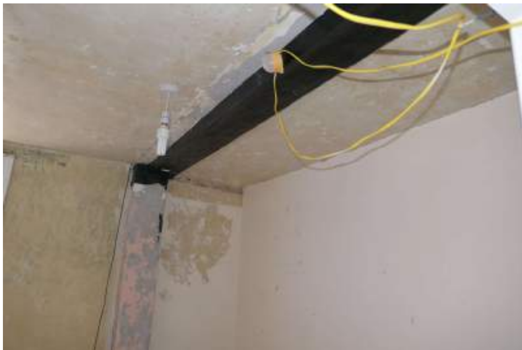
EEX62136_Photograph_195 Detail of exposed square beam in ceiling of bedroom 3. Photograph taken facing south.
