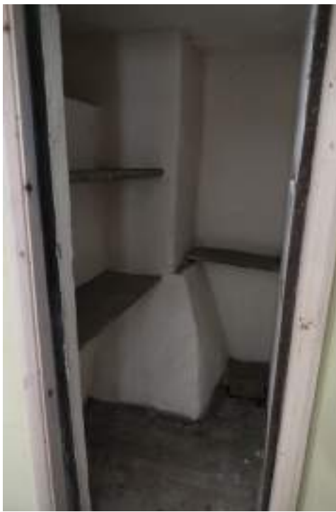
EEX62136_Photograph_257 Detail of hidden alcove in bedroom 4. Photograph taken facing south-west.
