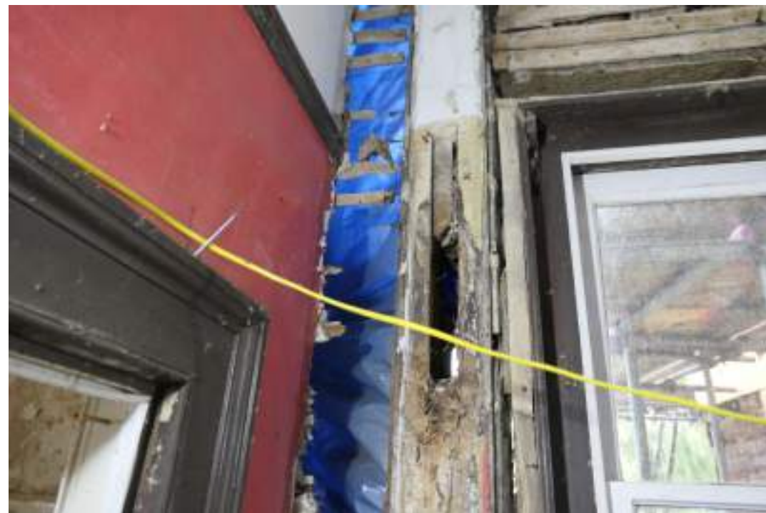
EEX62136_Photograph_108 Detail of empty mortice on post in south-eastern wall of office. Photograph taken facing south south-west.
