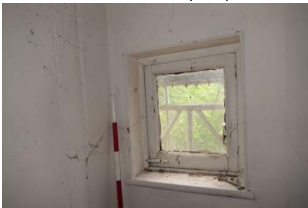
EEX62136_Photograph_167 Detail of window in north-western wall of cupboard in corridor 3. Photograph taken facing west north-west.
