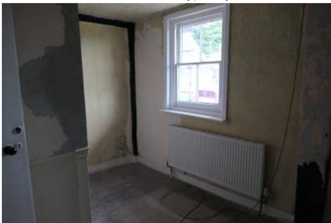
EEX62136_Photograph_191 Interior of bedroom 3. Photograph taken facing east.
