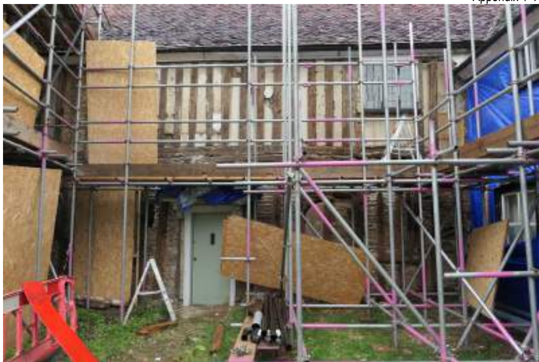
EEX62136_PhotoGraph_021 South-eastern elevation (range 5). Photograph taken facing north-west.
