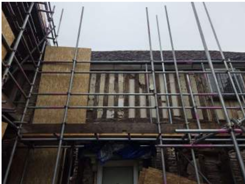
EEX62136_PhotoGraph_023 Detail of timber-framing of south-eastern elevation (range 5). Photograph taken facing north-west.
