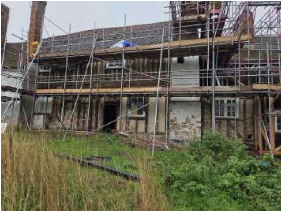
EEX62136_Photograph_027 North-western elevation (range 5). Photograph taken facing south-east.
