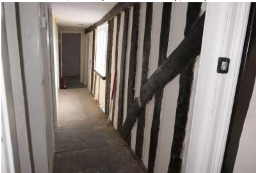
EEX62136_Photograph_203 Detail of exposed timber-framing in south-eastern wall of corridor 4. Photograph taken facing east south-east.
