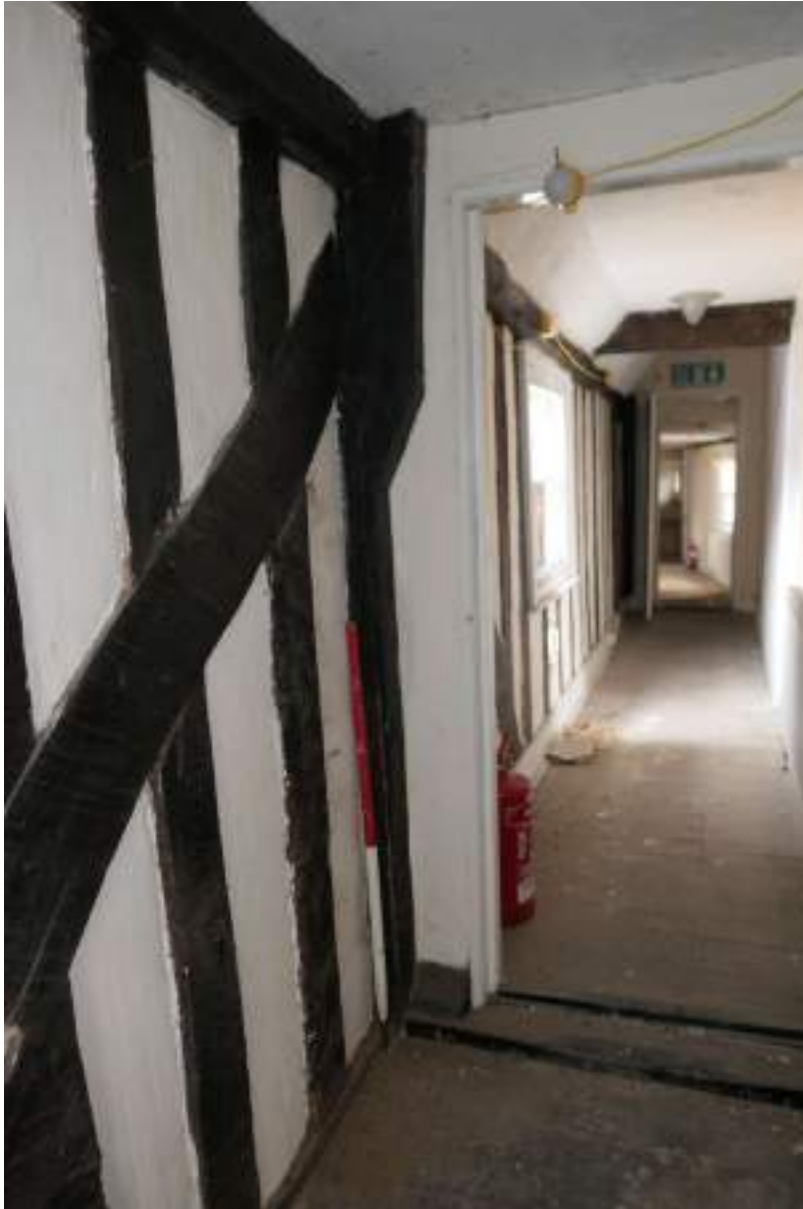
Photograph 43 Detail of jowled post in south-eastern wall of corridor 4. Photograph taken facing south.
