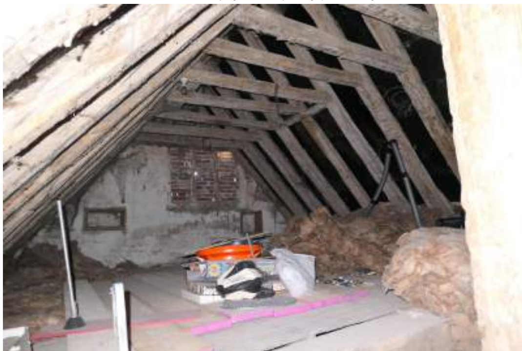
EEX62136_Photograph_055 Detail of roof construction above range 3. Photograph taken facing west.
