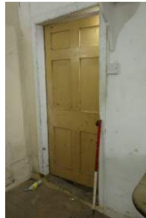
EEX62136_Photograph_070 Detail of door in south-western wall of spare room 1. Photograph taken facing south-west.
