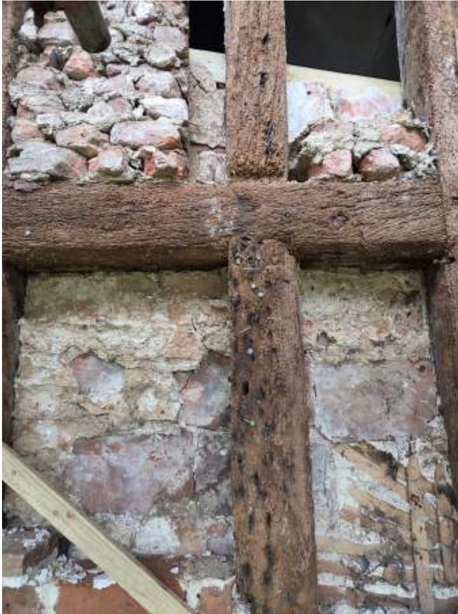
Photograph 17 Detail of peg-tiles used for noggin in north-western elevation (range 5). Photograph taken facing south-east.
