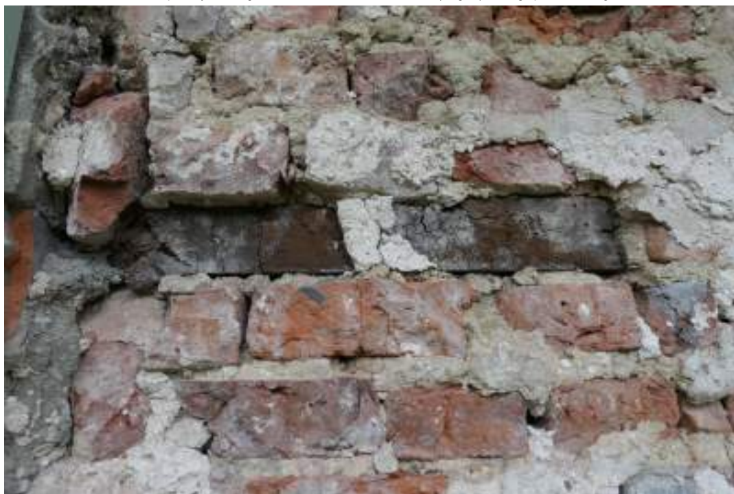
EEX62136_PhotoGraph_015 Detail of exposed timber in brickwork of south-eastern elevation (range 3). Photograph taken facing north-west.
