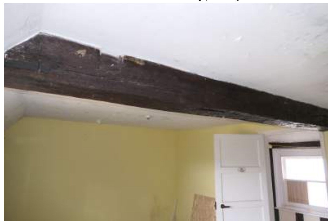
EEX62136_Photograph_232 Detail of exposed tie-beam in ceiling of bedroom 4. Photograph taken facing east.
