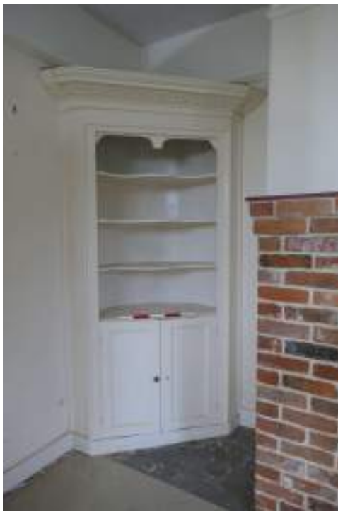
EEX62136_Photograph_149 Detail of in-built cuboard in dining room. Photograph taken facing north.
