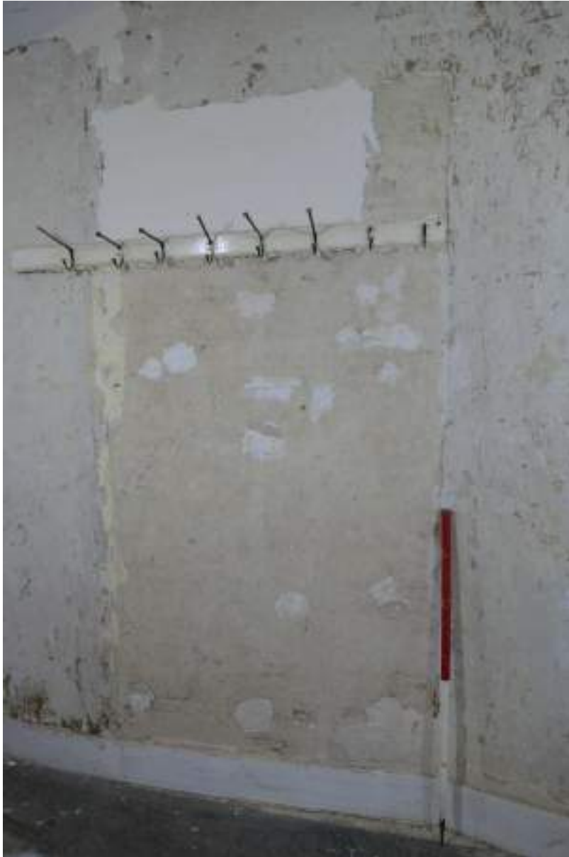
Photograph 30 Detail of blocked doorway in south-eastern wall of corridor 1. Photograph taken facing east south-east.
