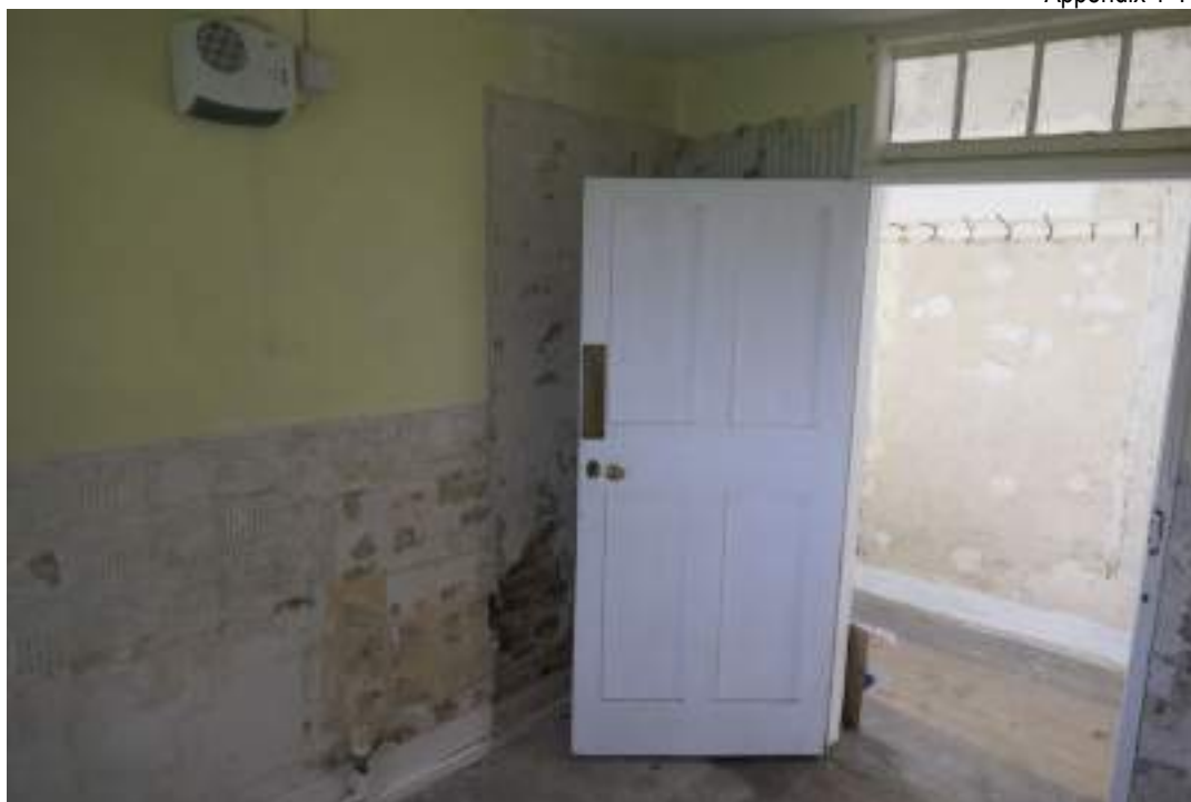
EEX62136_Photograph_141 Interior of bathroom. Photograph taken facing east.
