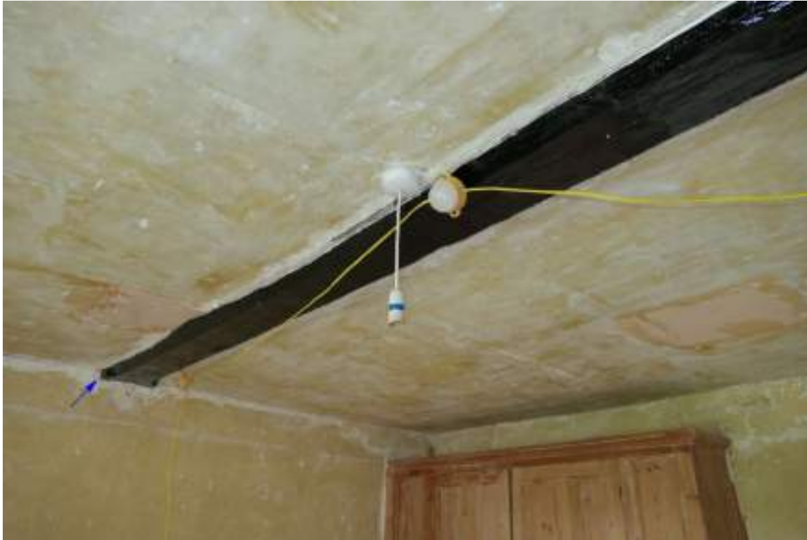
Photograph 38 Detail of chamfered bridging joist, with curved stepped stops (blue arrow). Photograph taken facing west.
