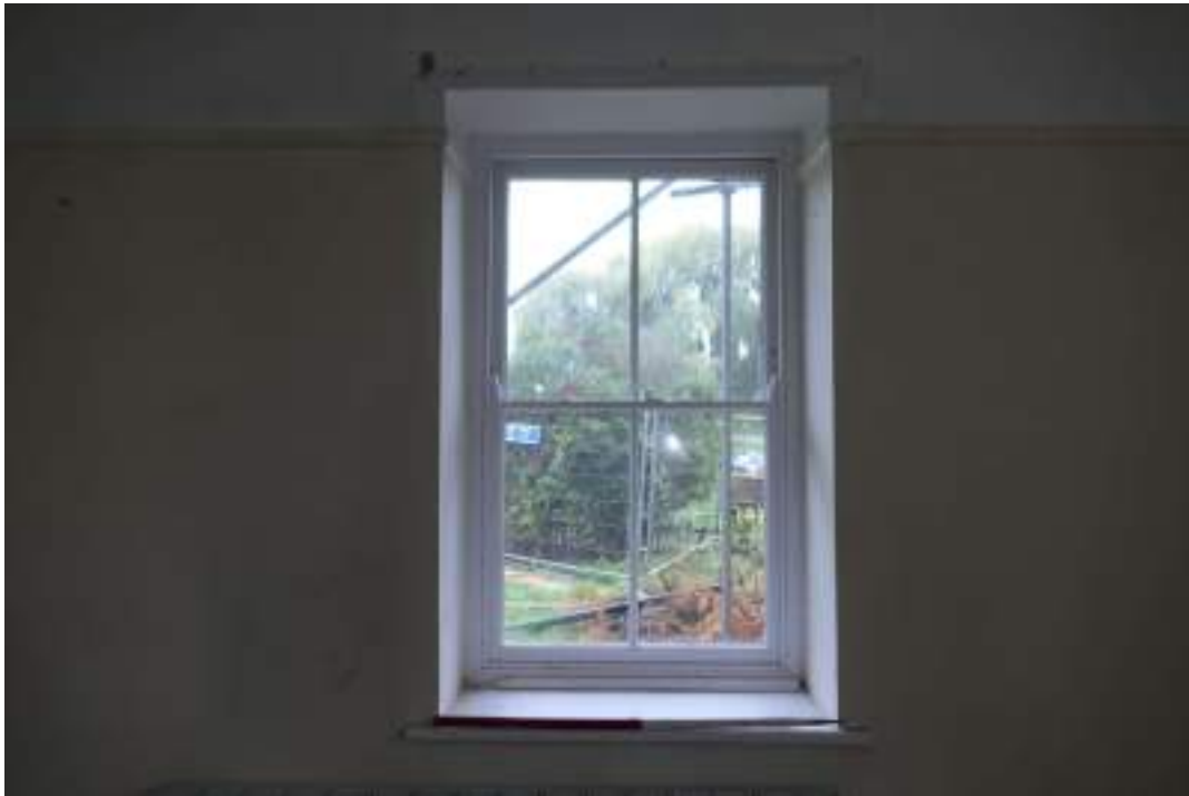
EEX62136_Photograph_151 Detail of window in south-eastern wall of dining room. Photograph taken facing south-east.
