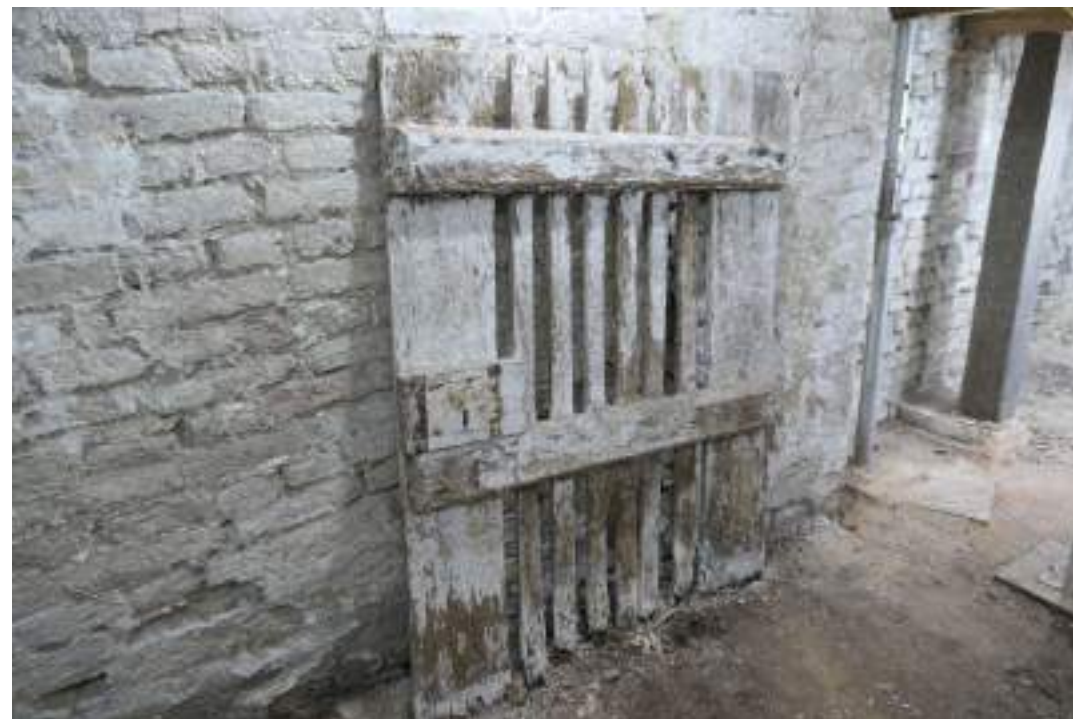
EEX62136_Photograph_248 Detail of off-hinged door in basement. Photograph taken facing south-east.
