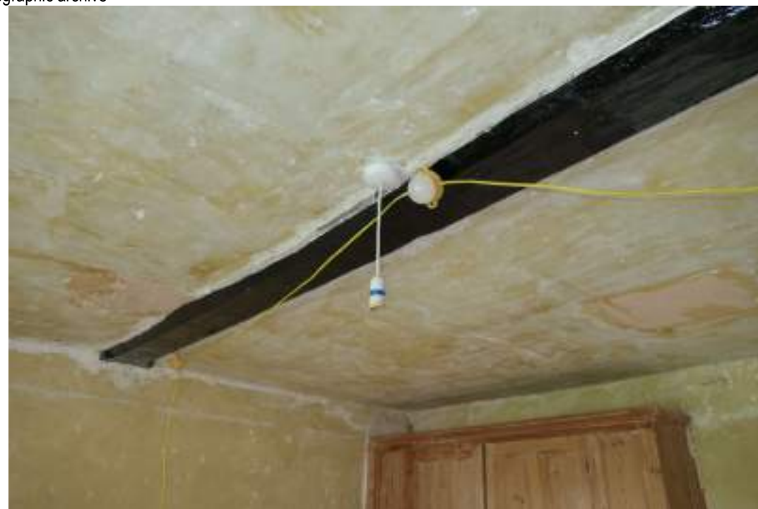
EEX62136_Photograph_186 Detail of chamfered bridging joist, with curved stepped stops. Photograph taken facing west.
