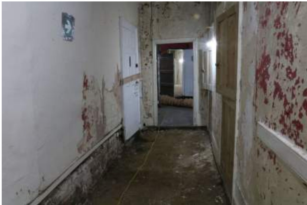
EEX62136_Photograph_071 Interior of corridor 2. Photograph taken facing south-west.
