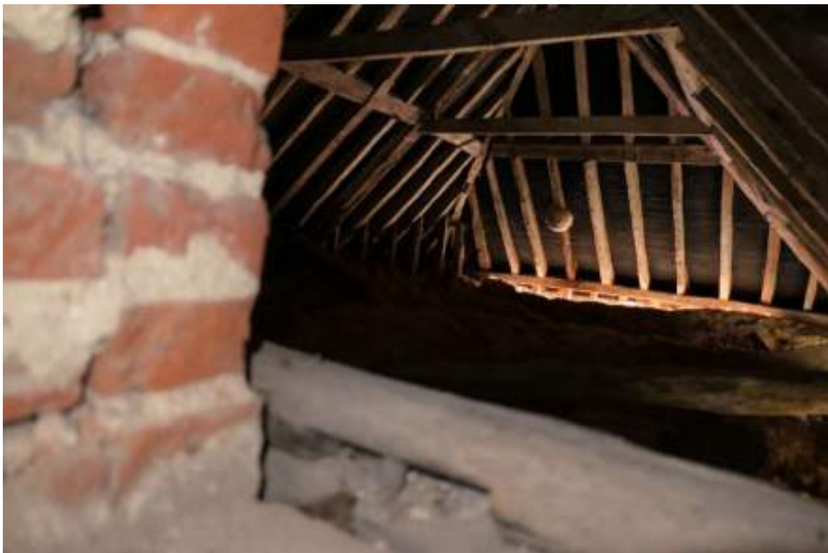
Photograph 19 Detail of roof construction above range 4. Photograph taken facing north.
