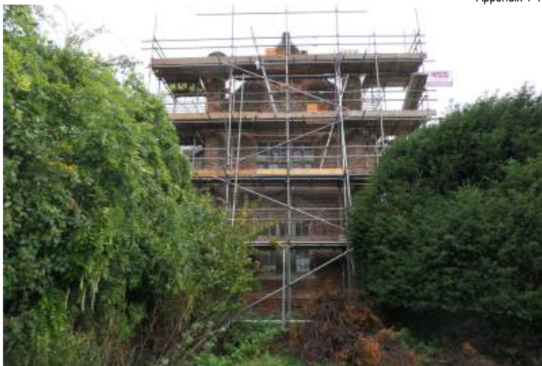
EEX62136_Photograph_001 South-western elevation (range 3). Photograph taken facing north-east.
