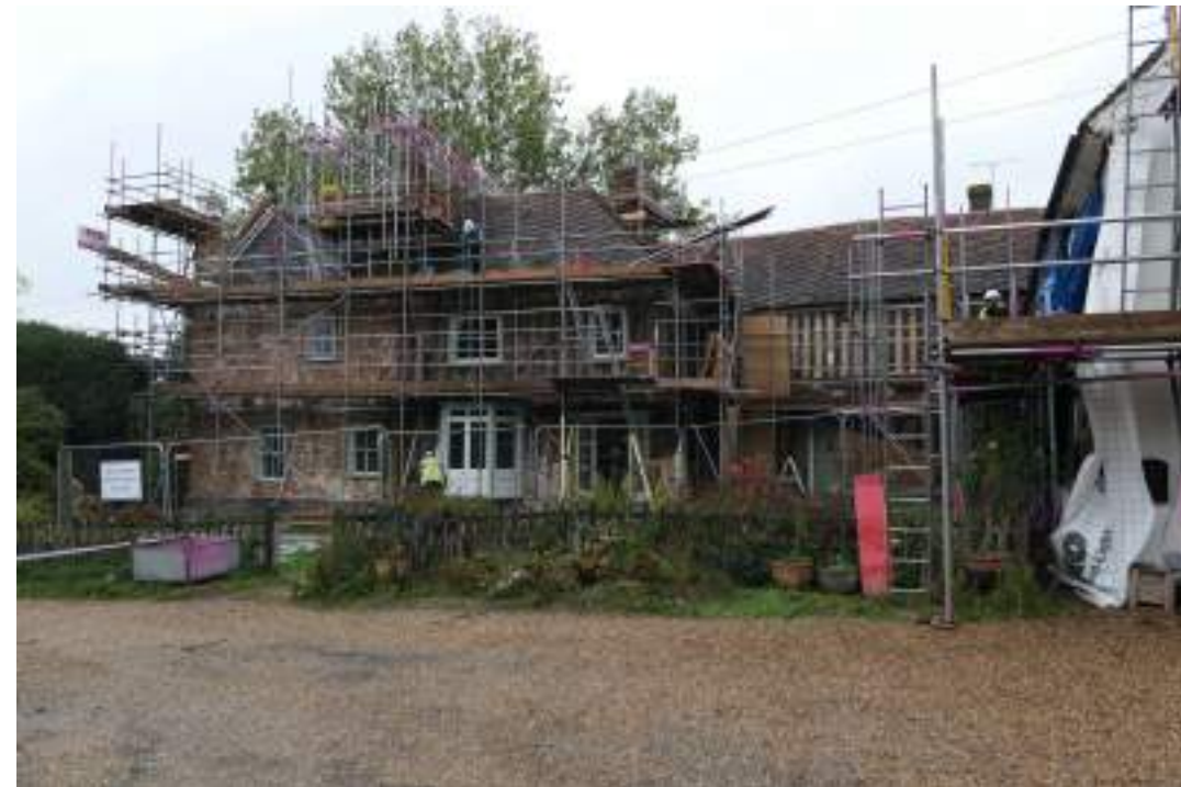
EEX62136_Photograph_052 South-eastern elevation (ranges 3, 4 and 5). Photograph taken facing west north-west.
