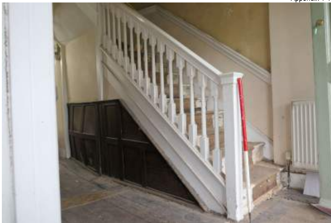
EEX62136_PhotoGraph_113 Detail of staircase in entrance hall. Photograph taken facing north.
