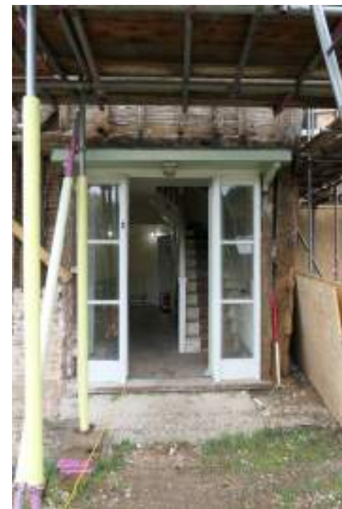
EEX62136_Photograph_048 Detail of door in south-eastern elevation (range 4). Photograph taken facing north-west.
