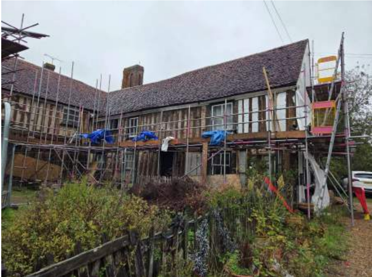
Photograph 13 South-western elevation (range 7). Photograph taken facing north.
