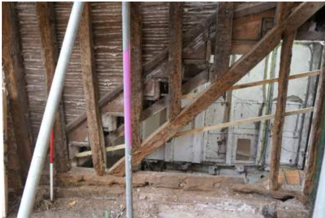
EEX62136_Photograph_051 Detail of exposed timber-framing in north-eastern elevation (range 4). Photograph taken facing south-west.
