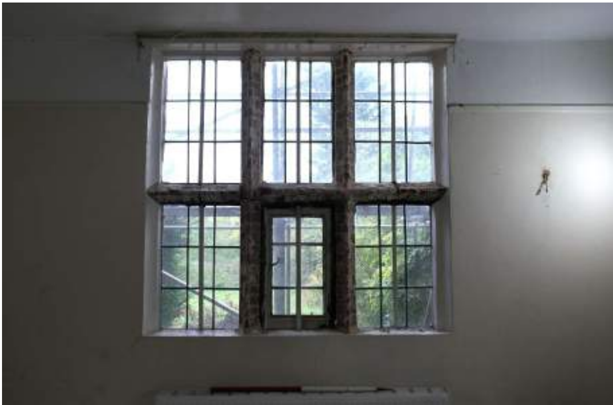
Photograph 26 Detail of window in south-western wall of dining room. Photograph taken facing south-west.
