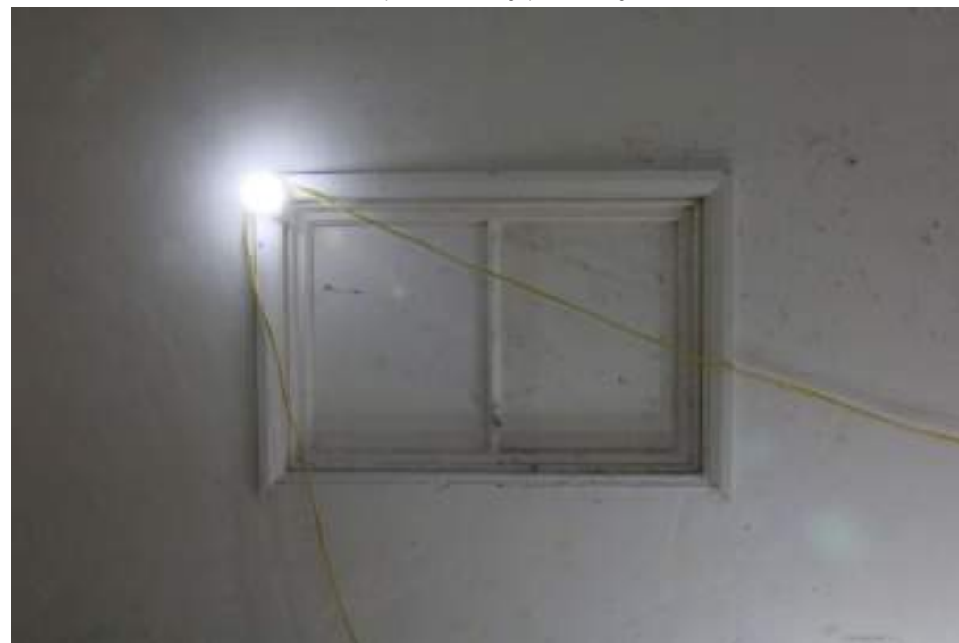
EEX62136_PhotoGraph_068 Detail of serving hatch in south-eastern wall of spare room 1. Photograph taken facing south-east.
