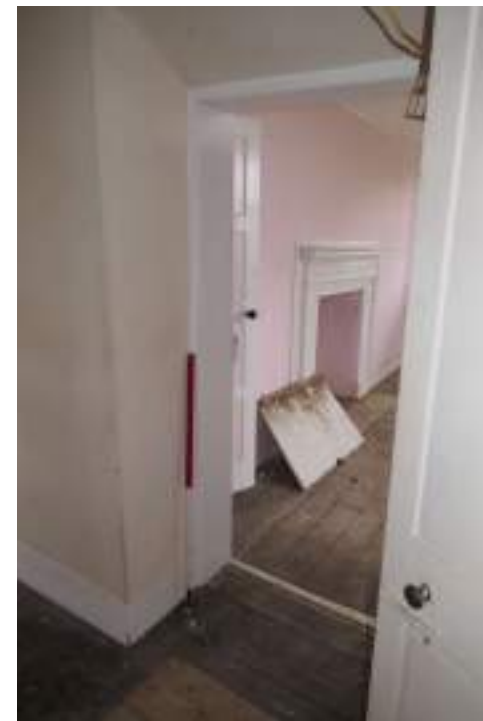
EEX62136_Photograph_170 Detail of doorway in south-eastern wall of corridor 3. Photograph taken facing east.
