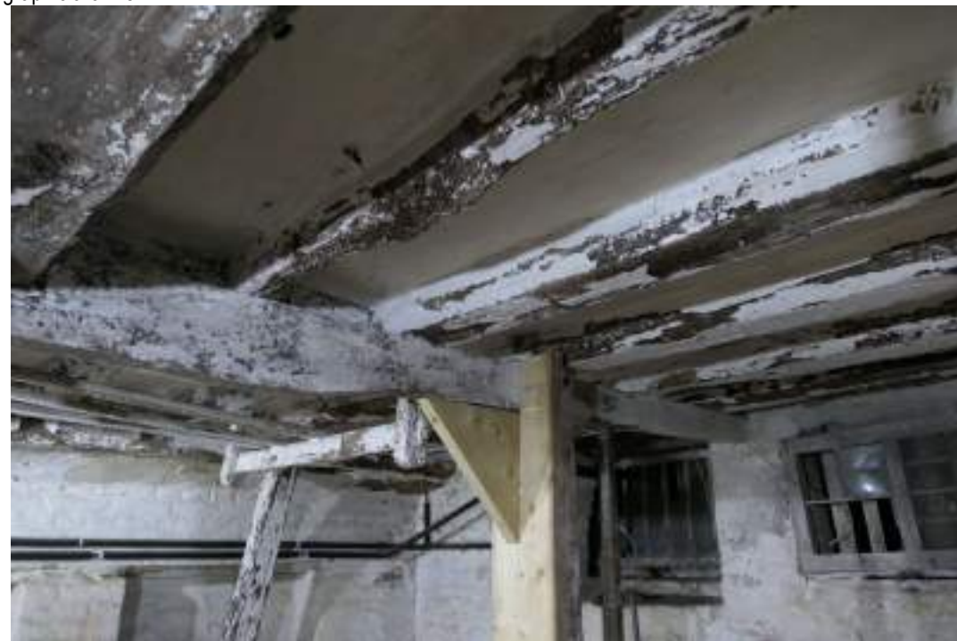
EEX62136_Photograph_246 Detail of binding-beams and joists in ceiling in basement. Photograph taken facing west.
