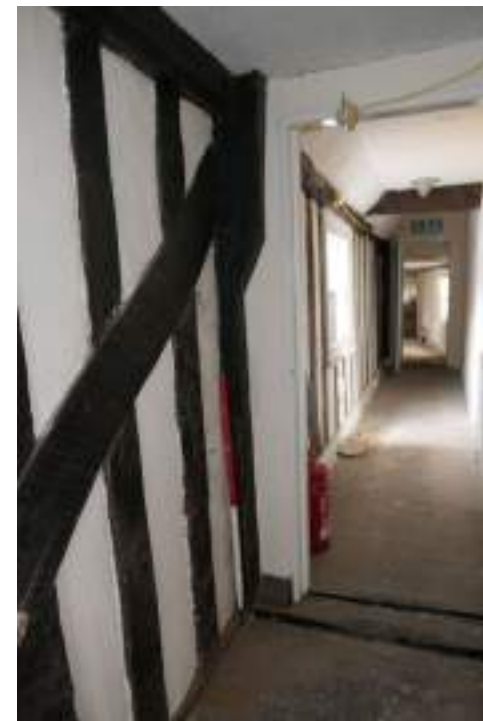
EEX62136_PhotoGraph_238 Detail of jowled post in south-eastern wall of corridor 4. Photograph taken facing south.
