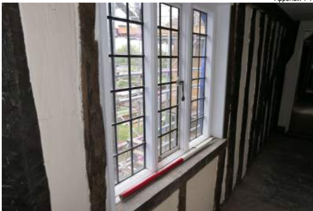
EEX62136_Photograph_205 Detail of window in south-eastern wall of corridor 4. Photograph taken facing south.
