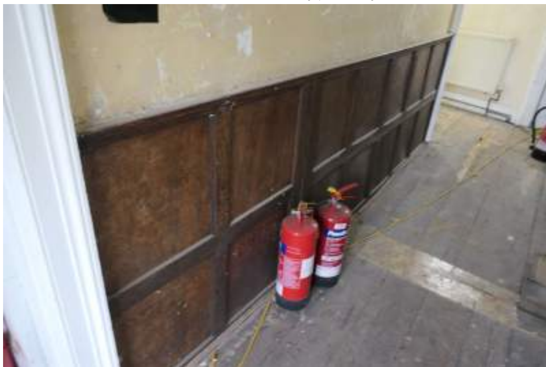
EEX62136_PhotoGraph_115 Detail of paneling on south-western wall of entrance hall. Photograph taken facing north-west.
