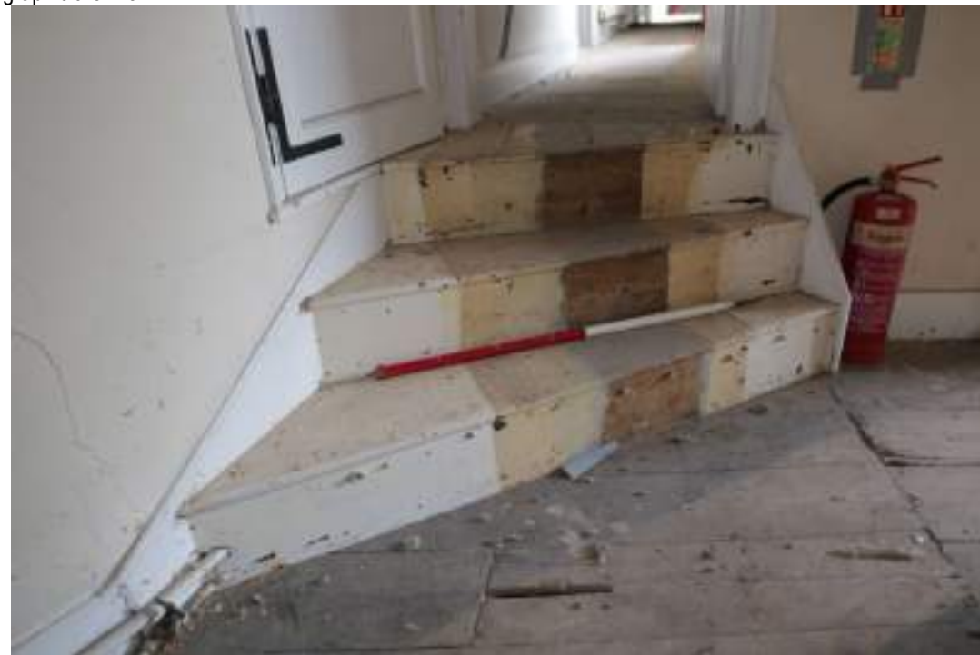
EEX62136_Photograph_162 Detail of stairs in corridor 3. Photograph taken facing north-east.
