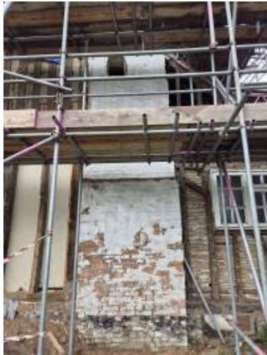
EEX62136_PhotoGraph_043 Detail of brickwork of chimney in north-western elevation (range 2). Photograph taken facing south-east.
