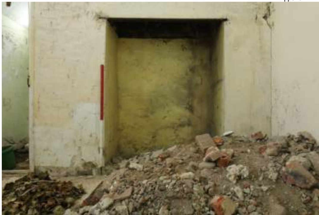
EEX62136_Photograph_069 Detail of fireplace in north-eastern wall of spare room 1. Photograph taken facing north-east.
