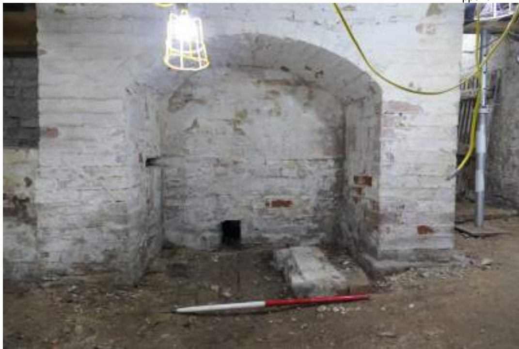
EEX62136_Photograph_253 Detail of brick arch in basement. Photograph taken facing north-east.
