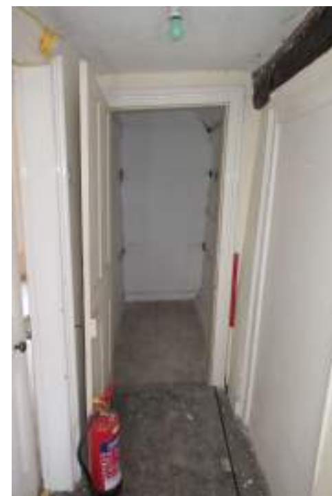
EEX62136_Photograph_206 Detail of door to cupboard in north-eastern wall of corridor 4. Photograph taken facing north-east.
