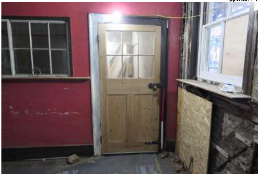
EEX62136_Photograph_097 Detail of door in north-eastern wall of office. Photograph taken facing north-east.
