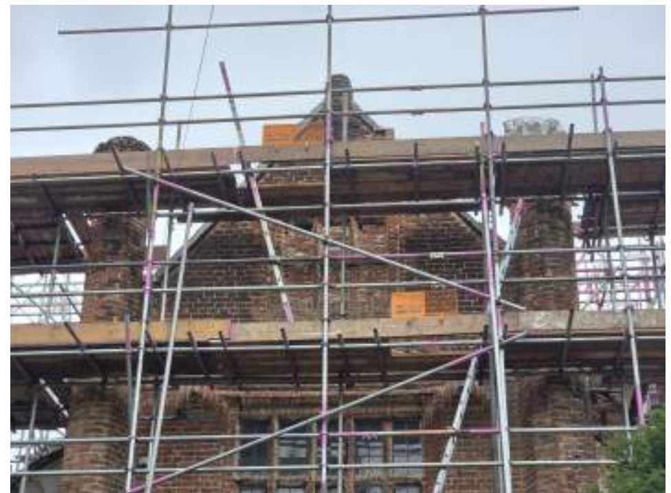
EEX62136_Photograph_004 Detail of blocked window in south-western gable (range 3). Photograph taken facing north-east.
