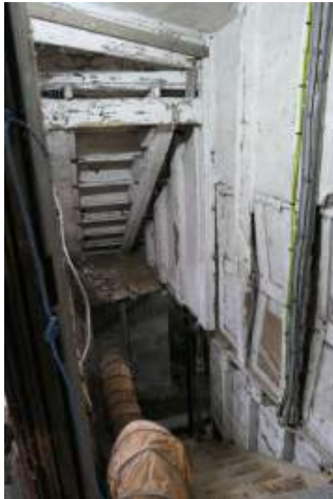
EEX62136_PhotoGraph_239 Detail of entrance to basement. Photograph taken facing south.
