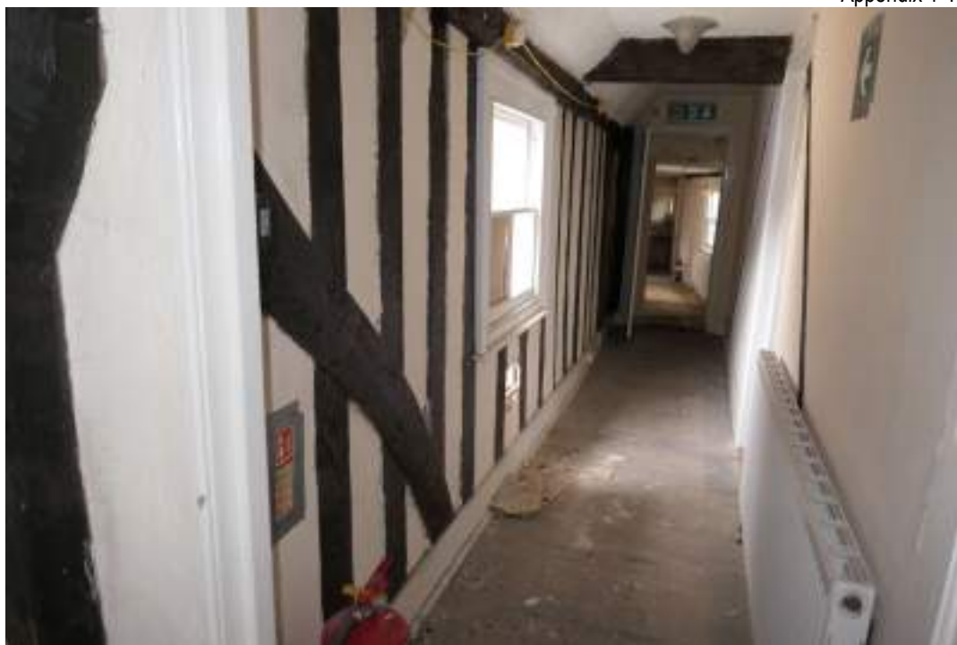
EEX62136_Photograph_201 Detail of the exposed timber-framing in south-eastern wall of corridor 4. Photograph taken facing south.
