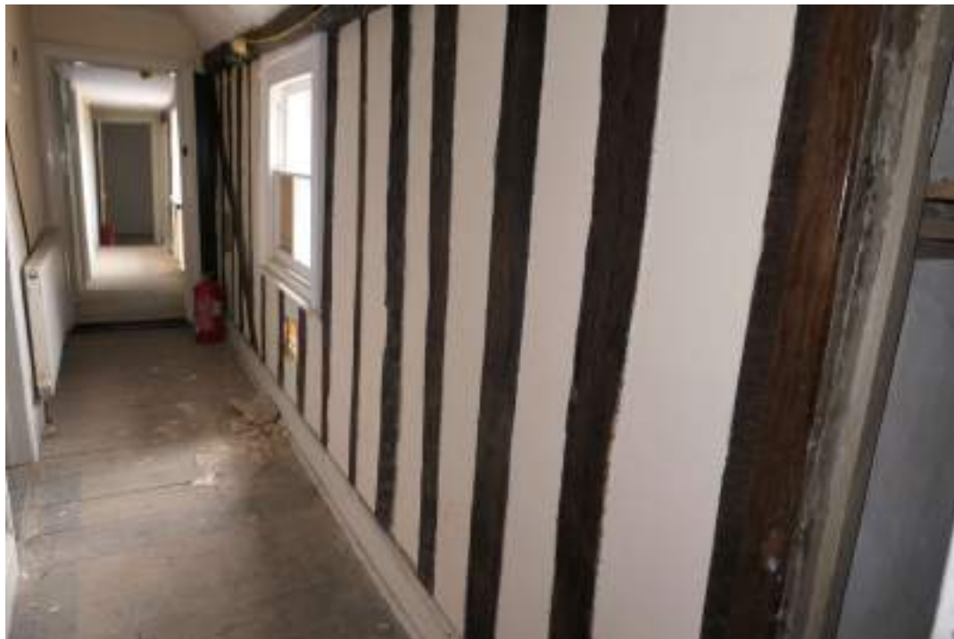
EEX62136_PhotoGraph_199 Detail of exposed timber-framing in south-eastern wall of corridor 4. Photograph taken facing east.
