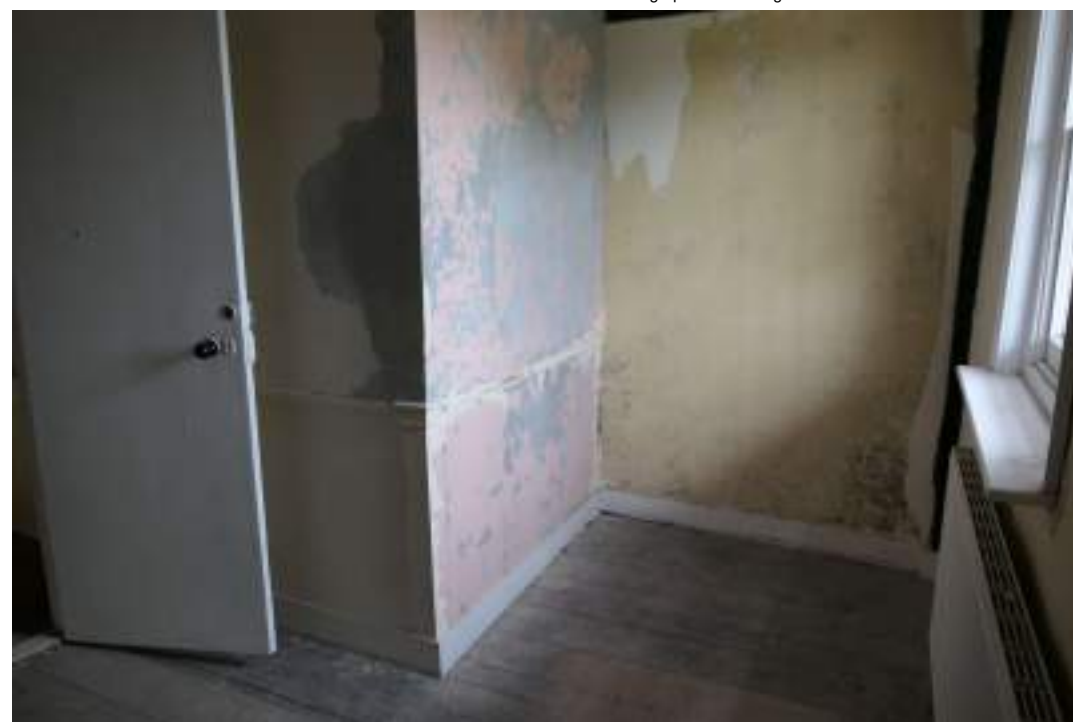
EEX62136_Photograph_192 Interior of bedroom 3. Photograph taken facing north.
