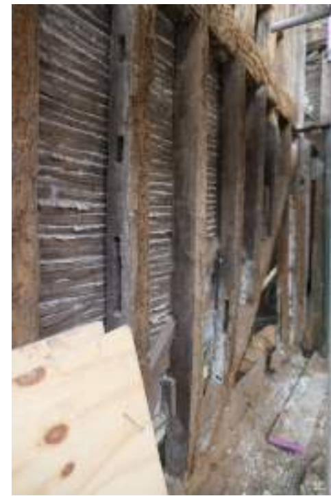
EEX62136_Photograph_050 Detail of exposed timber-framing, with reused stud, in north-eastern elevation (range 4). Photograph taken facing west.
