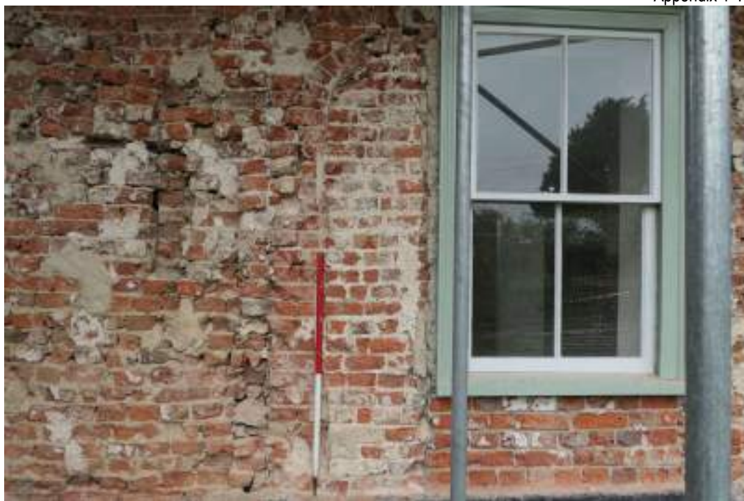
EEX62136_PhotoGraph_013 Detail of blocked, partially surviving brick arch in south-eastern elevation (range 3). Photograph taken facing north-west.
