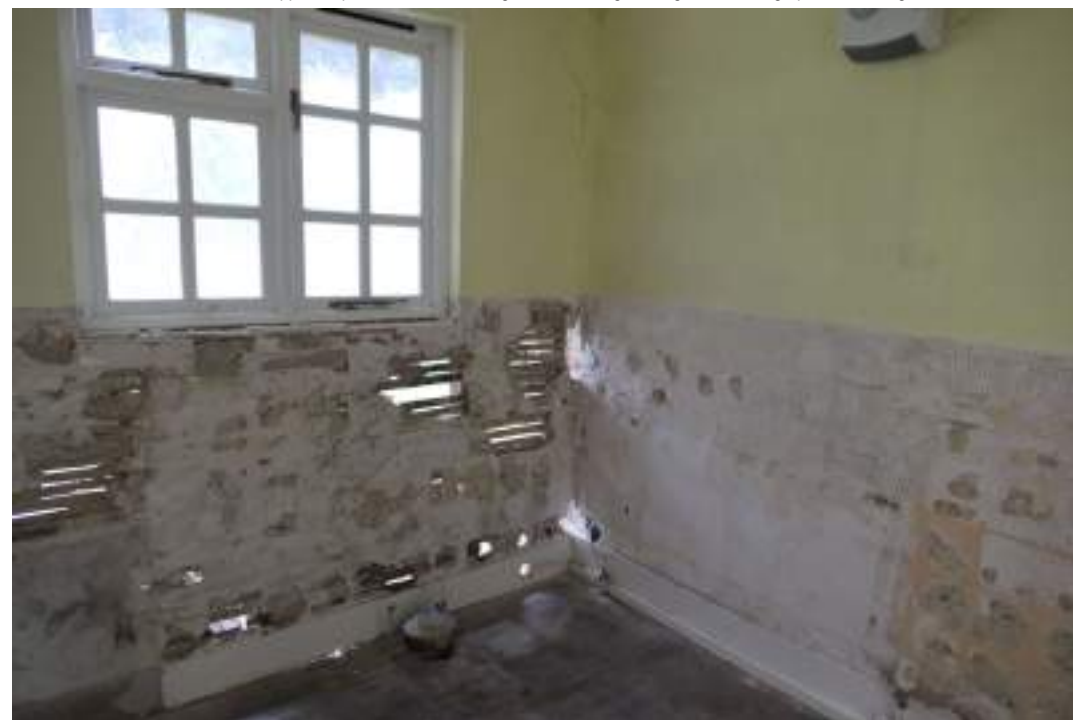
EEX62136_Photograph_140 Interior of bathroom. Photograph taken facing north.
