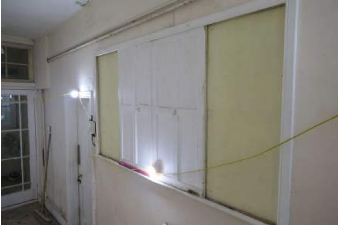
Photograph 31 Detail of window shutters in north-western wall of corridor 1. Photograph taken facing west.
