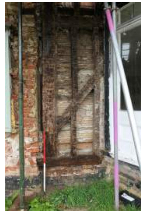
EEX62136_Photograph_046 Detail of exposed timber-framing in south-eastern elevation (range 4). Photograph taken facing north-west.
