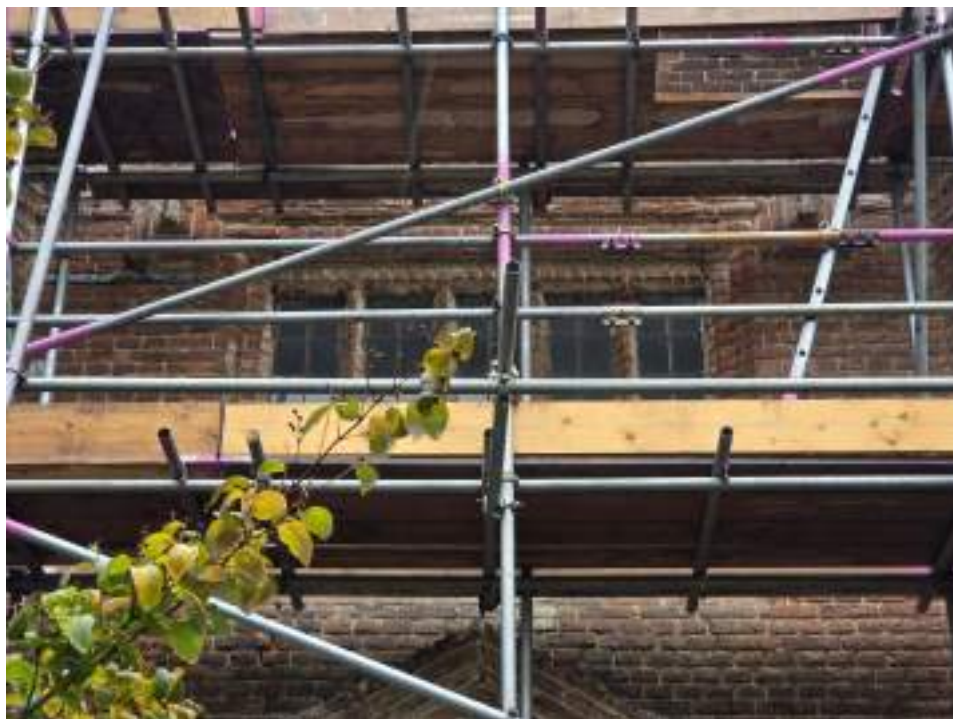
EEX62136_Photograph_003 Detail of window in south-western elevation (range 3). Photograph taken facing north-east.
