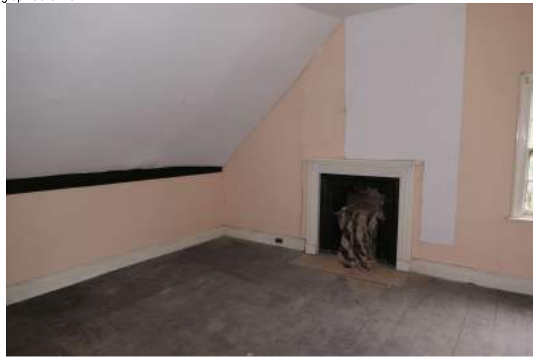
EEX62136_Photograph_210 Interior of bedroom 6. Photograph taken facing north.
