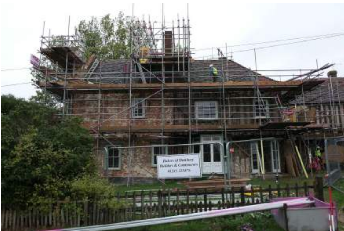
Photograph 2 South-eastern elevation (range 3 and 4). Photograph taken facing north-west.
