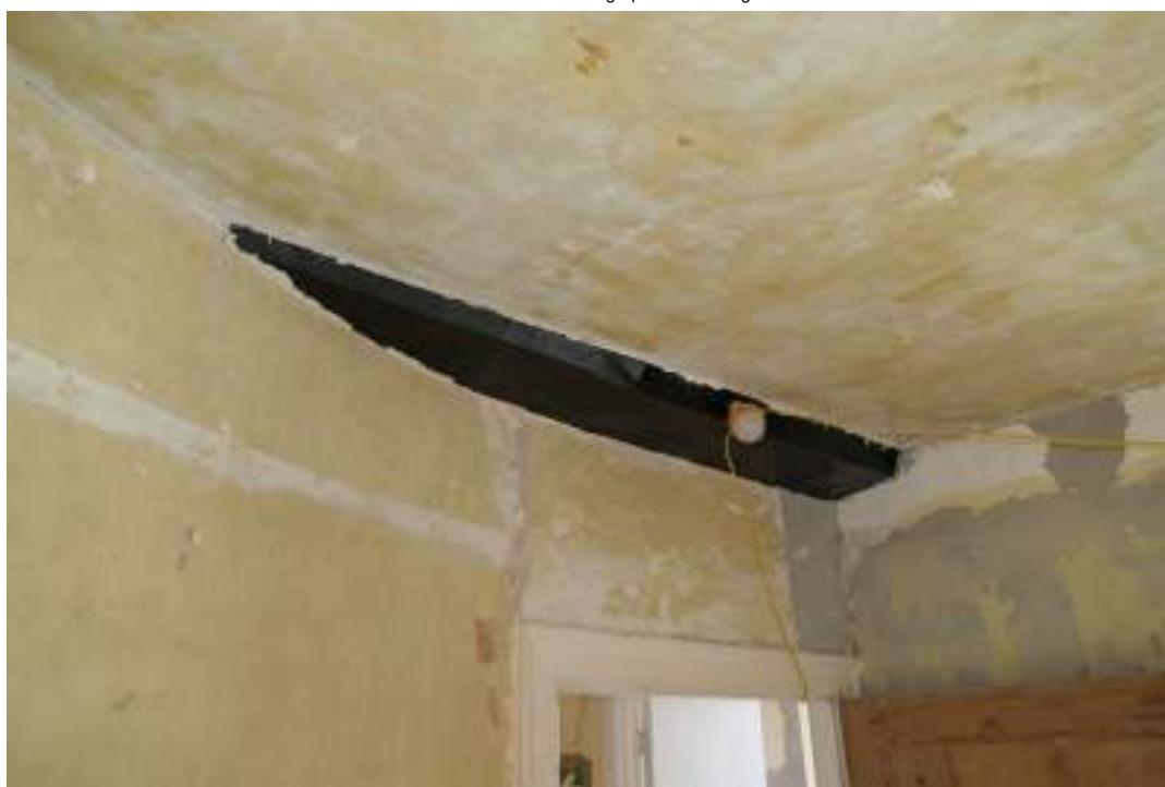
EEX62136_Photograph_187 Detail of exposed chamfered binding in ceiling of bedroom 2. Photograph taken facing south-east.
