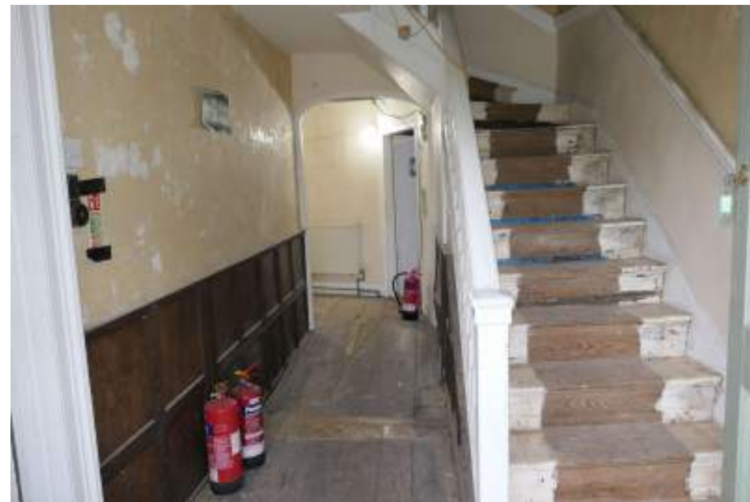
EEX62136_Photograph_112 Interior of entrance hall. Photograph taken facing north-west.
