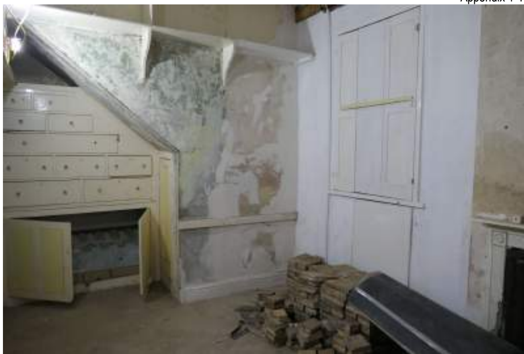
EEX62136_Photograph_081 Interior of spare room 2. Photograph taken facing west.
