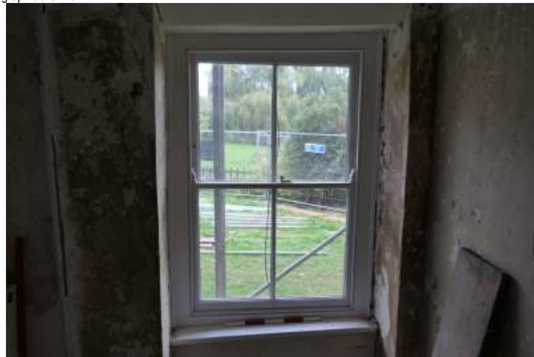
EEX62136_Photograph_134 Detail of window in south-eastern wall of living room. Photograph taken facing south-east.
