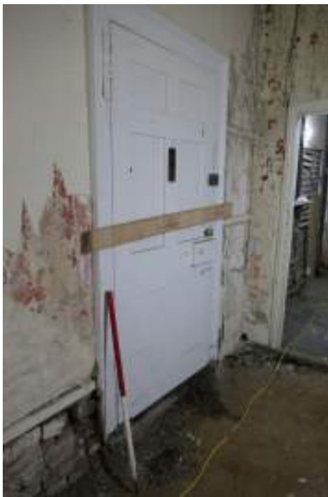
EEX62136_Photograph_077 Detail of door in south-eastern wall of corridor 2. Photograph taken facing south.
