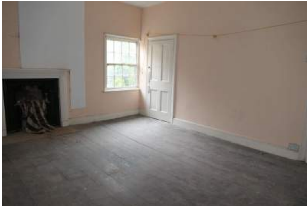
EEX62136_Photograph_211 Interior of bedroom 6. Photograph taken facing east.
