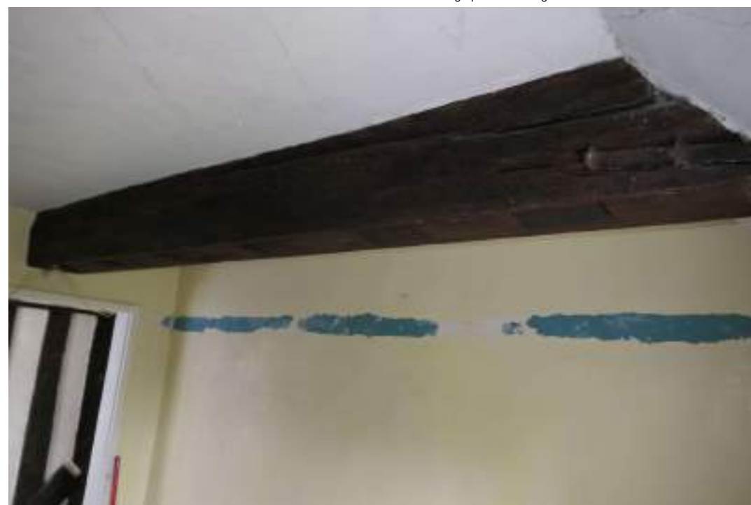
EEX62136_Photograph_224 Detail of reused tie-beam in ceiling of bedroom 5. Photograph taken facing south.
