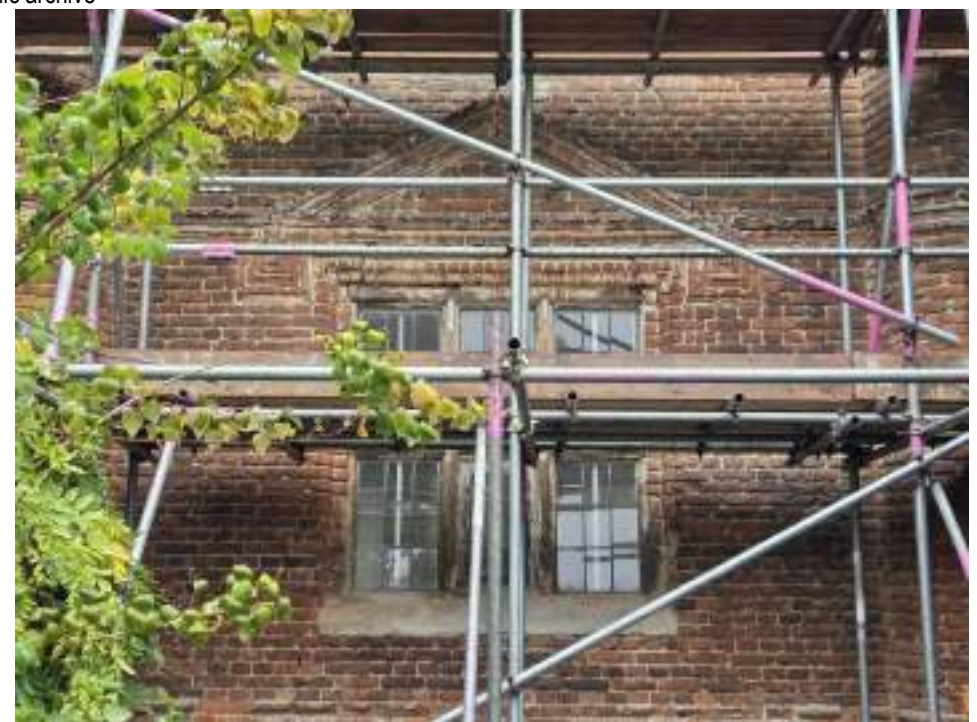
EEX62136_Photograph_002 Detail of window in south-western elevation (range 3). Photograph taken facing north-east.
