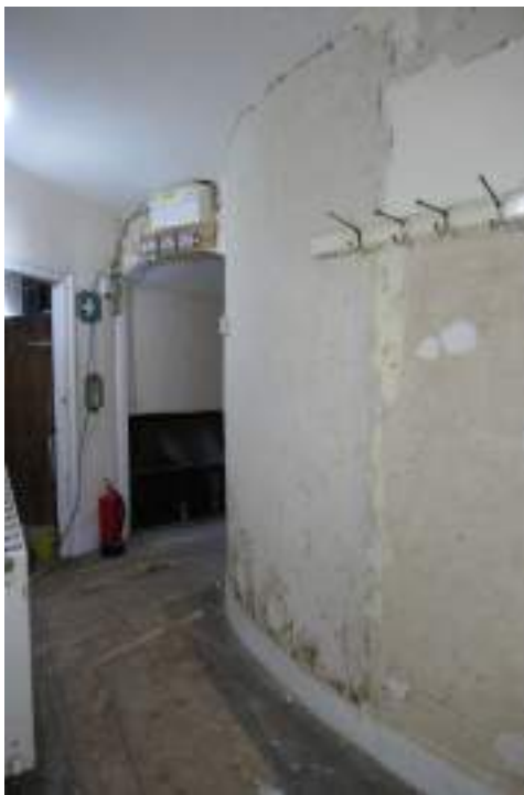
EEX62136_Photograph_117 Detail of curved wall in corridor 1. Photograph taken facing east.
