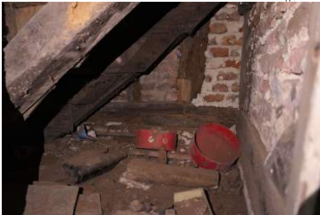
EEX62136_Photograph_089 Detail of rear stairs from beneath. Photograph taken facing north-west.
