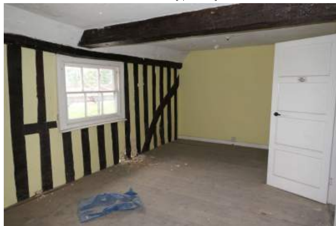
EEX62136_Photograph_228 Interior of bedroom 4. Photograph taken facing north.
