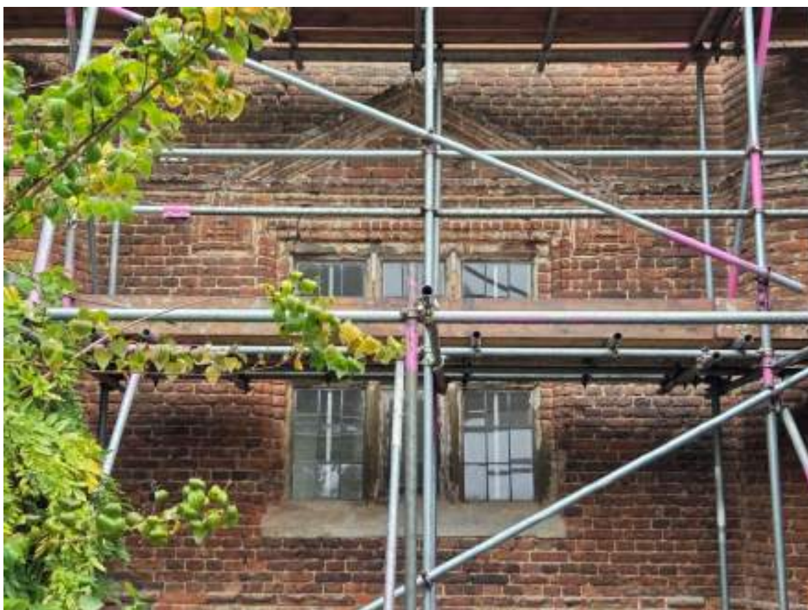
Photograph 11 Detail of window in south-western elevation (range 3). Photograph taken facing north-east.
