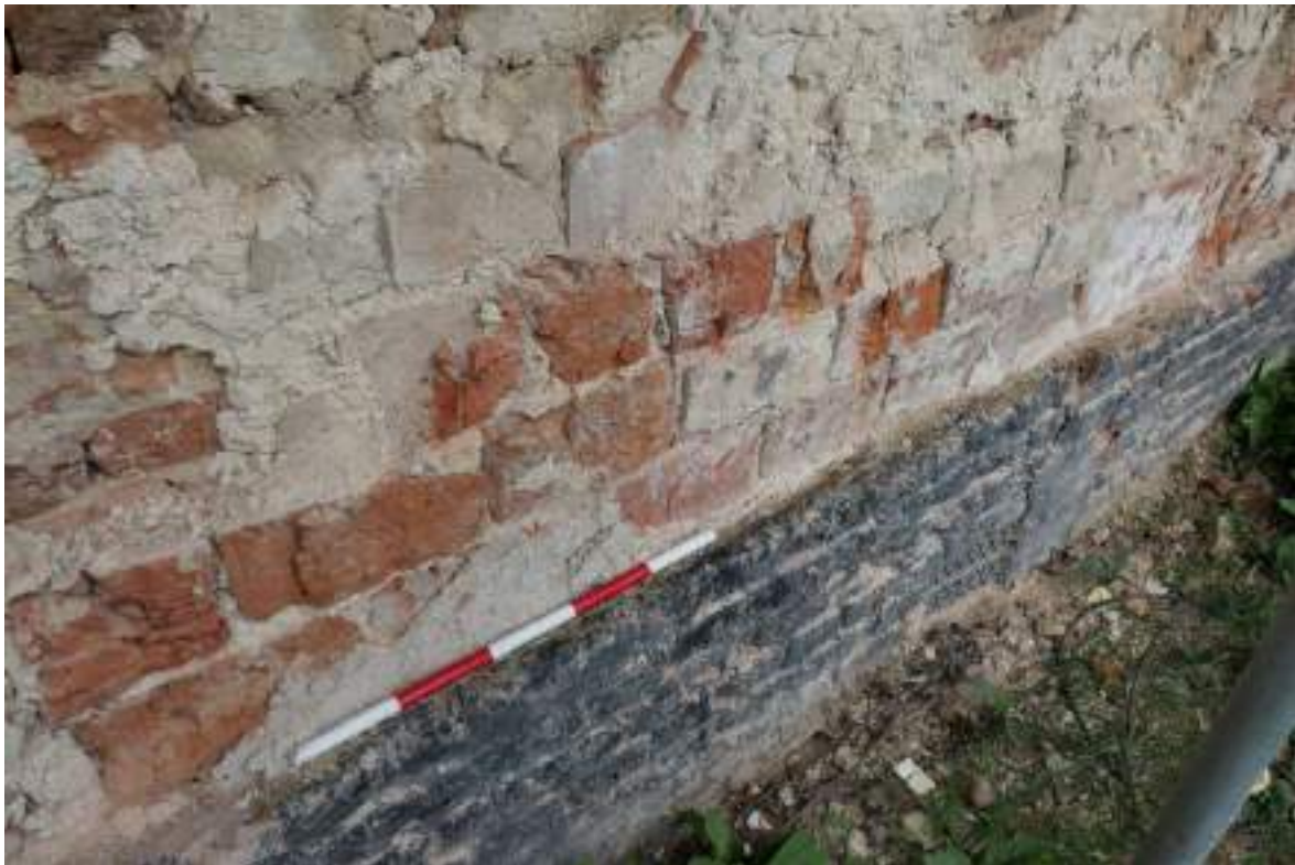
Photograph 3 Detail of bricks laid on-edge in brickwork and plinth of south-eastern elevation (range 3). Photograph taken facing north.
