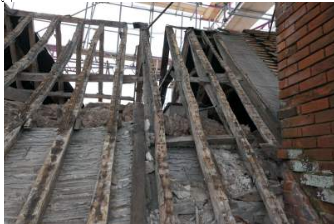
EEX62136_Photograph_062 Detail of roof construction above range 5. Photograph taken facing south south-east.
