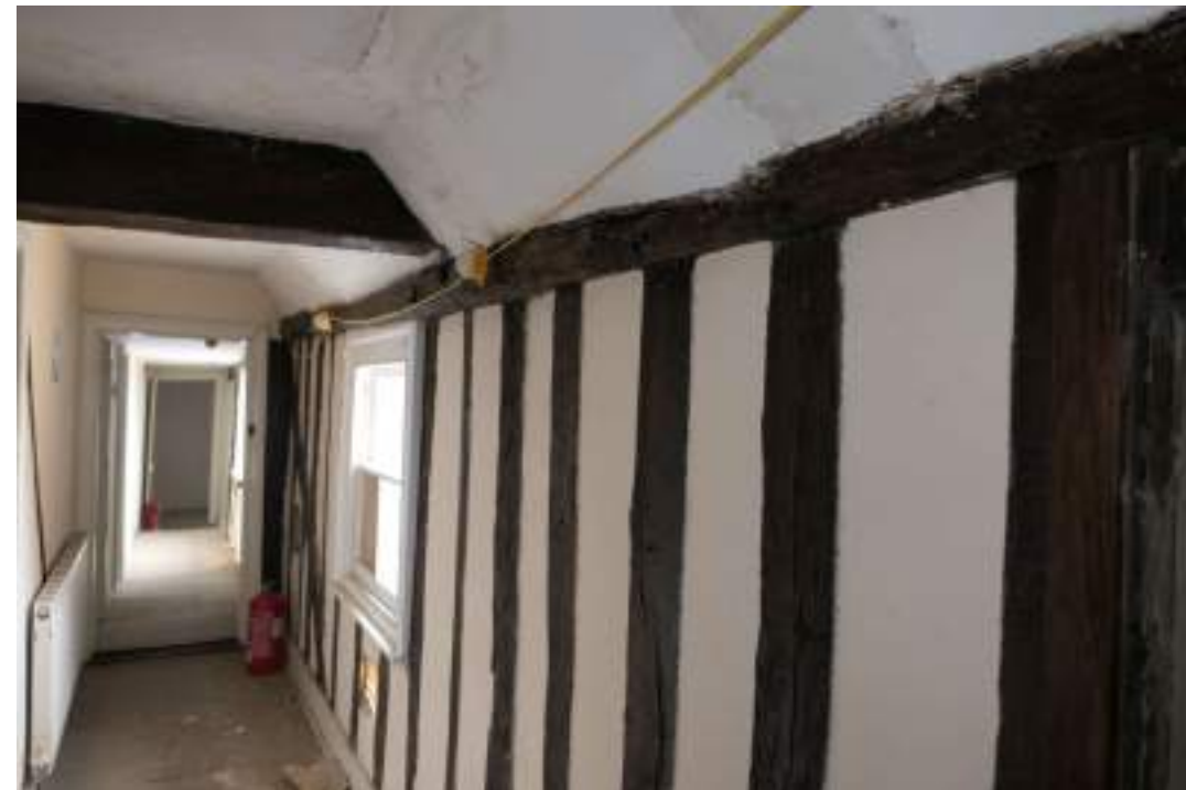
EEX62136_PhotoGraph_200 Detail of exposed timber-framing in south-eastern wall of corridor 4. Photograph taken facing east.
