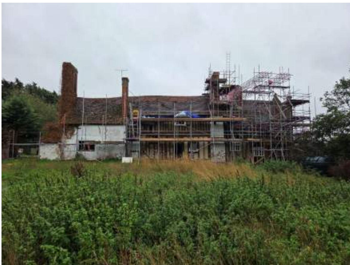
Photograph 15 North-western elevation (ranges 1, 2, 5 and 6). Photograph taken facing south-east.
