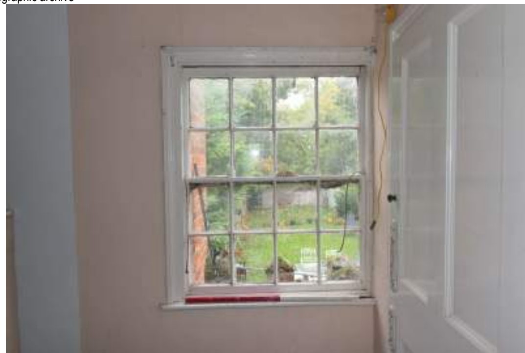
EEX62136_Photograph_214 Detail of window in north-eastern wall of bedroom 6. Photograph taken facing north-east.
