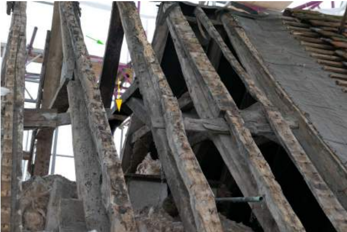
Photograph 20 Detail of roof construction above range 5. Green arrow highlighting blackened timbers and yellow arrow highlighting the void in the blackening, likely caused by a central purlin. Photograph taken facing south south-east.
