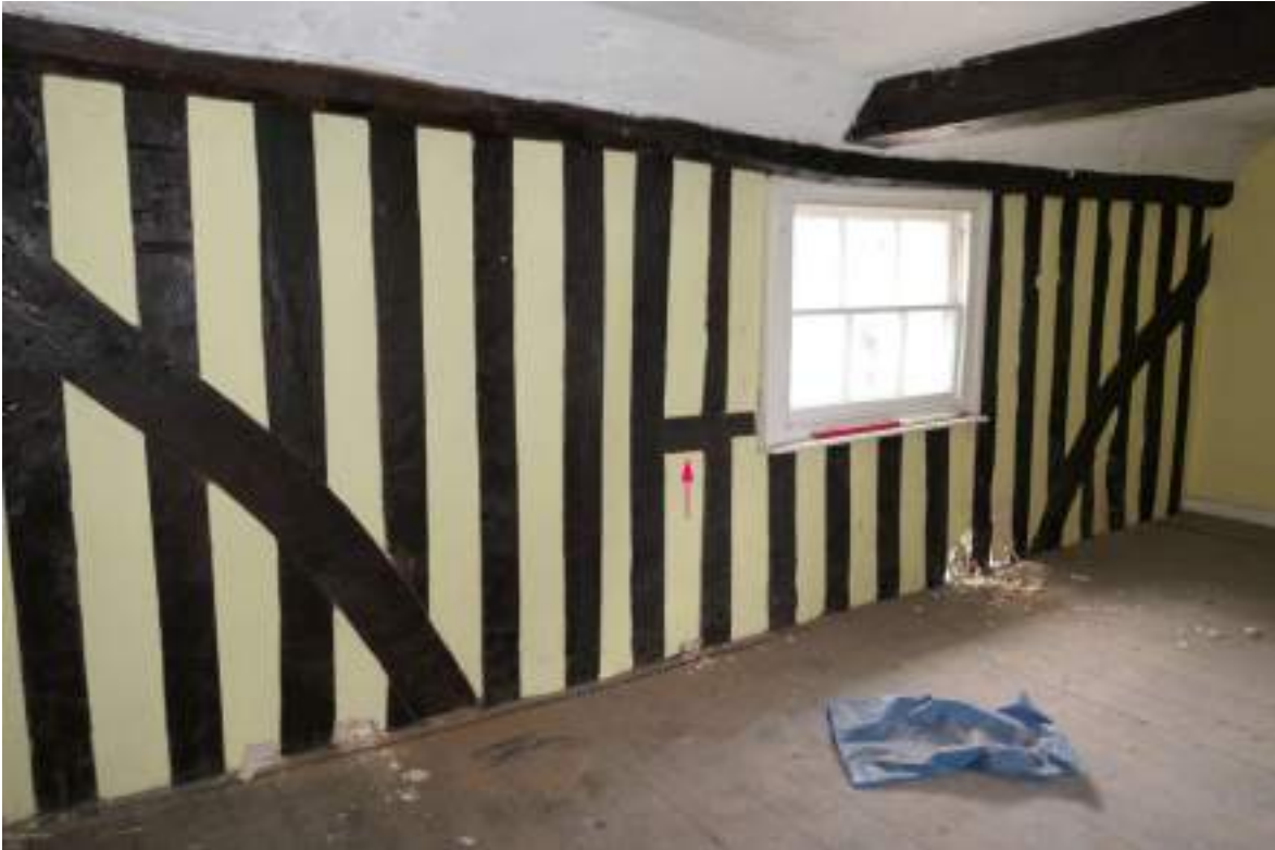
Photograph 44 Detail of exposed timber-framing in north-western wall of bedroom 4. Pink arrow highlighting a horizontal rail likely associated with an original window. Photograph taken facing north.
