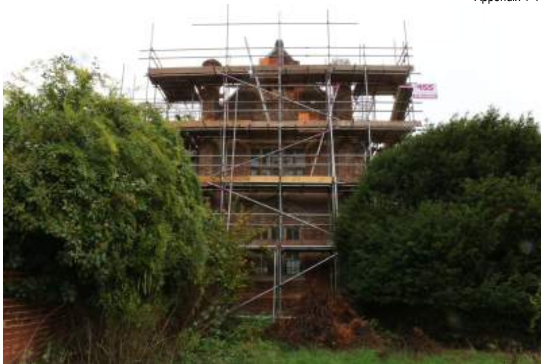
EEX62136_Photograph_073 South-western elevation. Photograph taken facing north-east.
