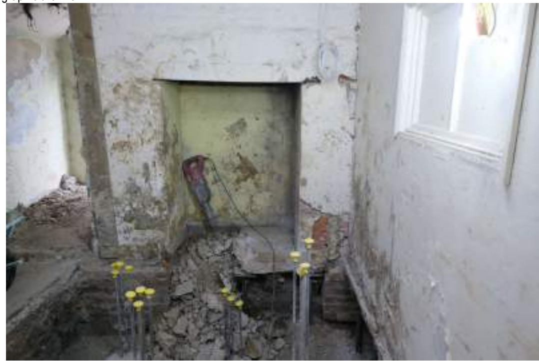
EEX62136_Photograph_258 Detail of fireplace in spare room 1 during reinforcement works. Photograph taken facing north-east.
