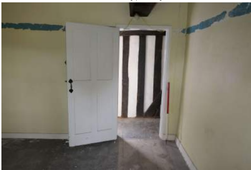
EEX62136_Photograph_223 Detail of door in south-eastern wall of bedroom 5. Photograph taken facing south-east.
