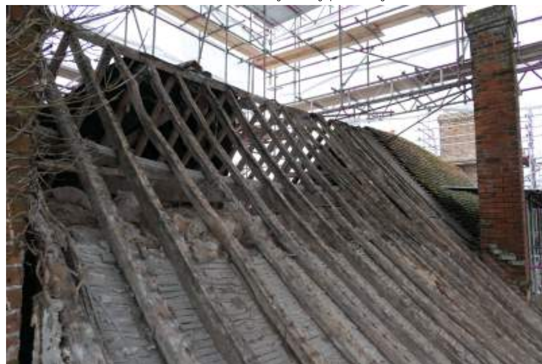
EEX62136_Photograph_060 Detail of roof structure above range 6. Photograph taken facing south.
