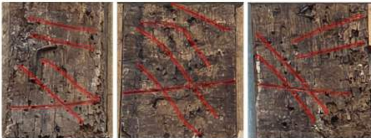
Photograph 9 Close up detail of carpenter's marks on range 5.
