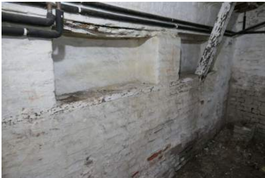
EEX62136_Photograph_247 Detail of alcoves in basement wall. Photograph taken facing west.
