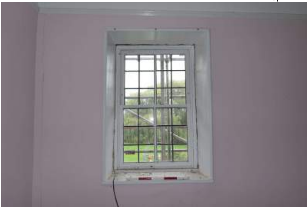
EEX62136_Photograph_181 Detail of window in south-eastern wall of bedroom 1. Photograph taken facing south-east.
