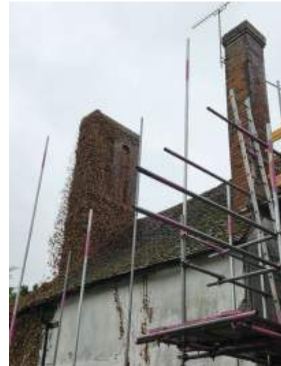
EEX62136_PhotoGraph_044 Detail of chimneys visible from the north-western elevation (range 6). Photograph taken facing east.
