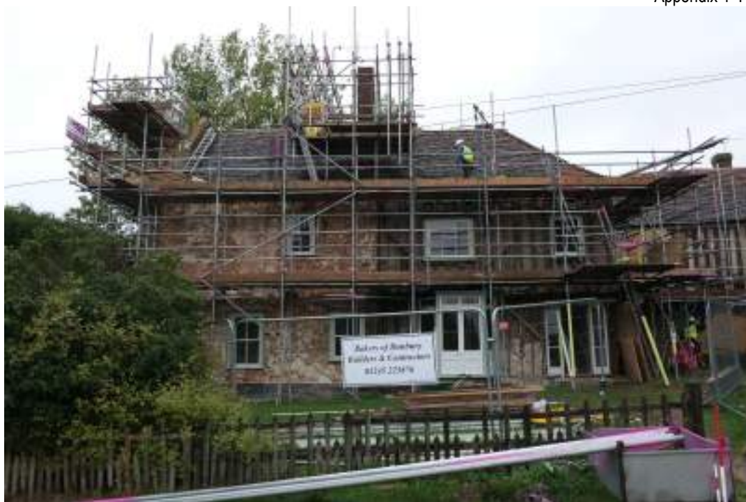
EEX62136_Photograph_045 South-eastern elevation (range 3 and 4). Photograph taken facing north-west.
