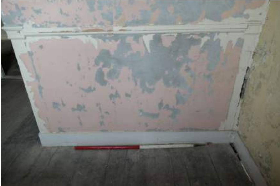
Photograph 39 Detail of stair balustrade incorporated into wall in bedroom 3. Photograph taken facing north-west.
