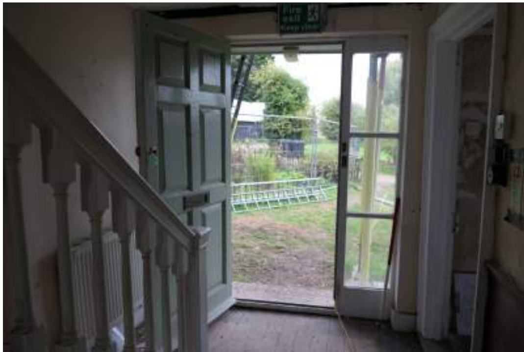
EEX62136_Photograph_127 Detail of door in south-eastern wall of entrance hall. Photograph taken facing south south-east.
