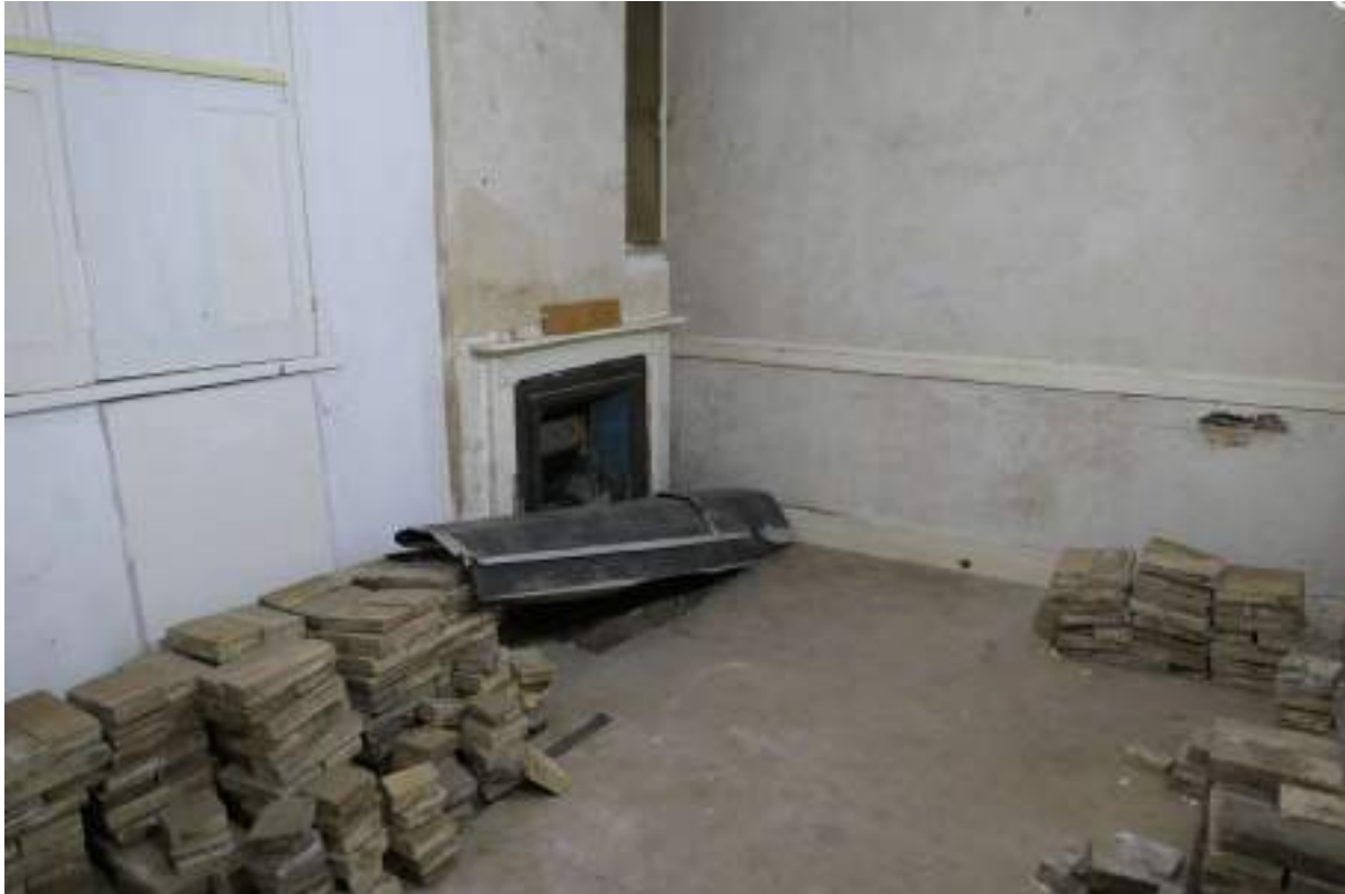
Photograph 35 Interior of spare room 2. Photograph taken facing north.
