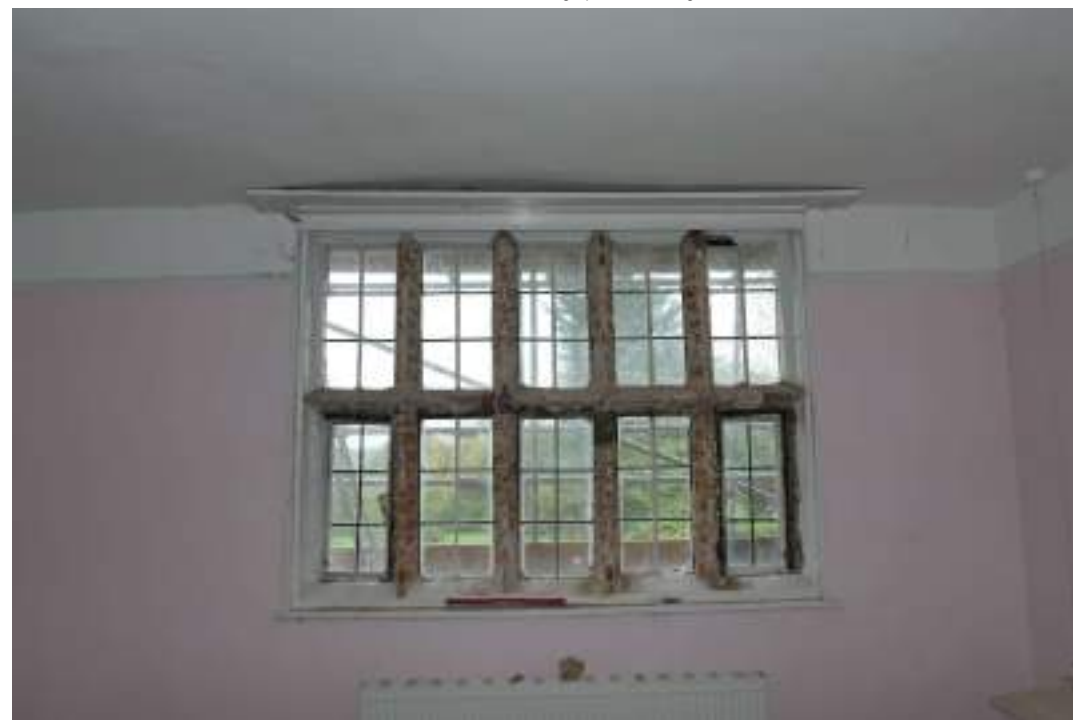
EEX62136_Photograph_176 Detail of window in the south-western wall of bedroom 1. Photograph taken facing south-west.
