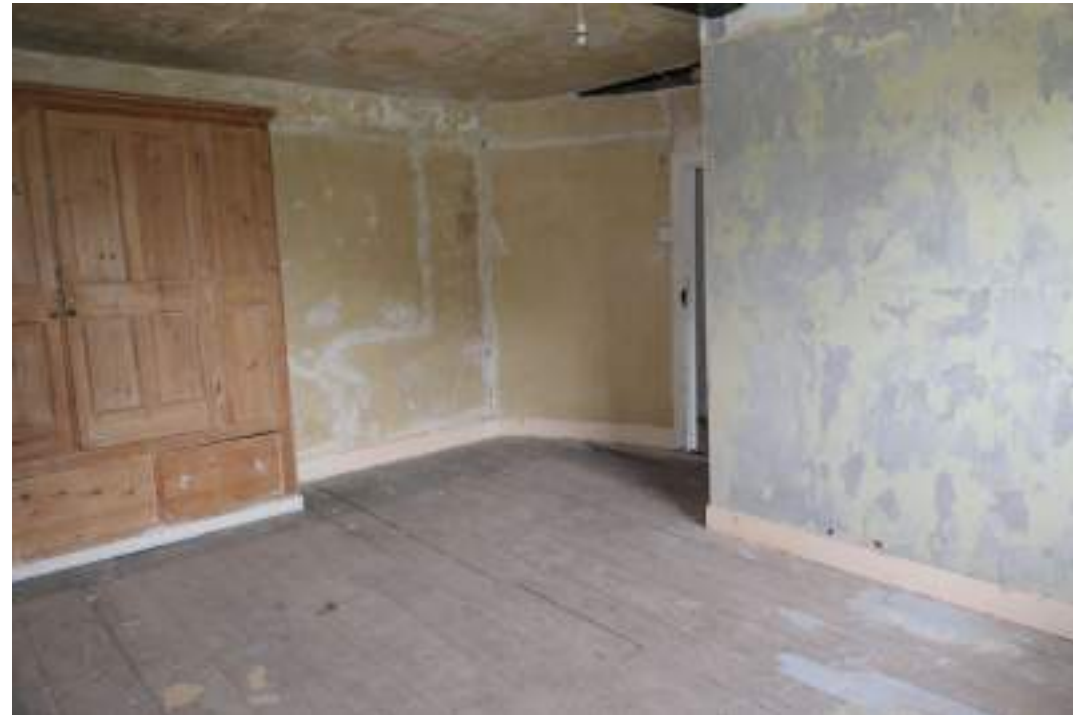
EEX62136_Photograph_184 Interior of bedroom 2. Photograph taken facing north.
