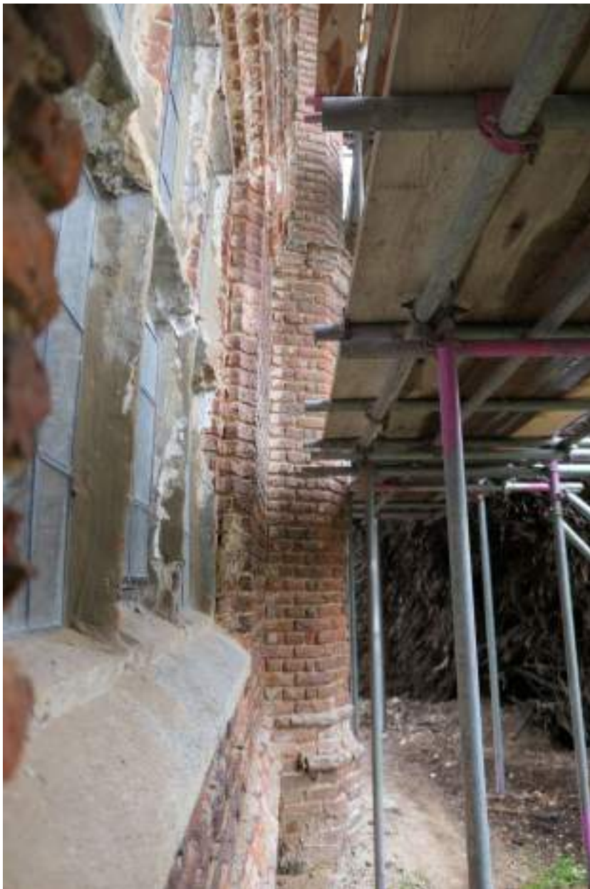
Photograph 12 Detail of octagonal corner buttress on south-western elevation (range 3). Photograph taken facing south-east.
