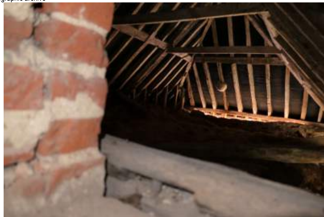
EEX62136_Photograph_058 Detail of roof construction above range 4. Photograph taken facing north.
