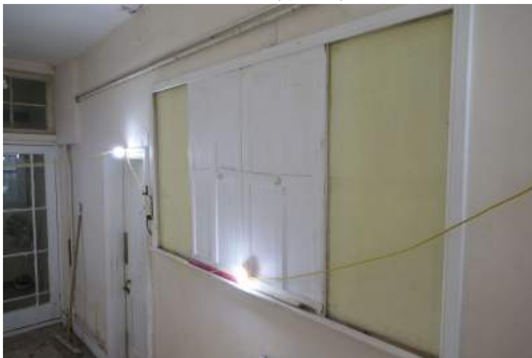
EEX62136_Photograph_123 Detail of window shutters in north-western wall of corridor 1. Photograph taken facing west.
