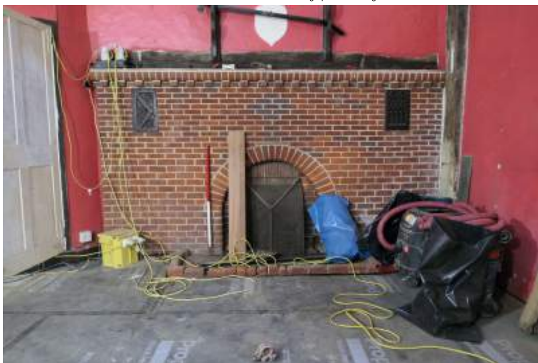
EEX62136_Photograph_103 Detail of fireplace in south-western wall of office. Photograph taken facing south-west.
