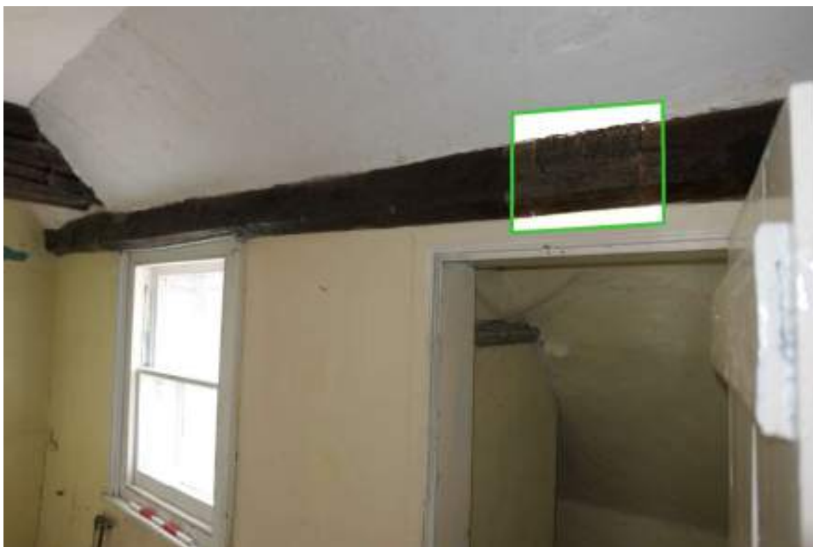
Photograph 48 Detail of exposed wall-plate in north-western wall of bedroom 5. Probable scarf-joint highlighted in green. Photograph taken facing west north-west.
