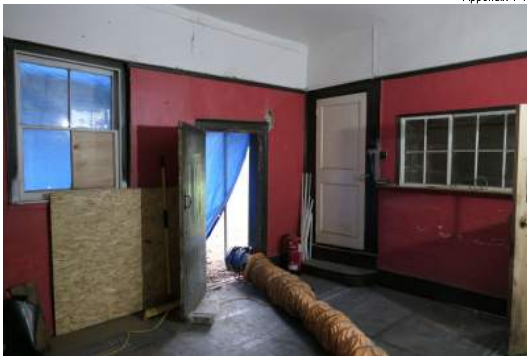
EEX62136_Photograph_093 Interior of office. Photograph taken facing north-east.
