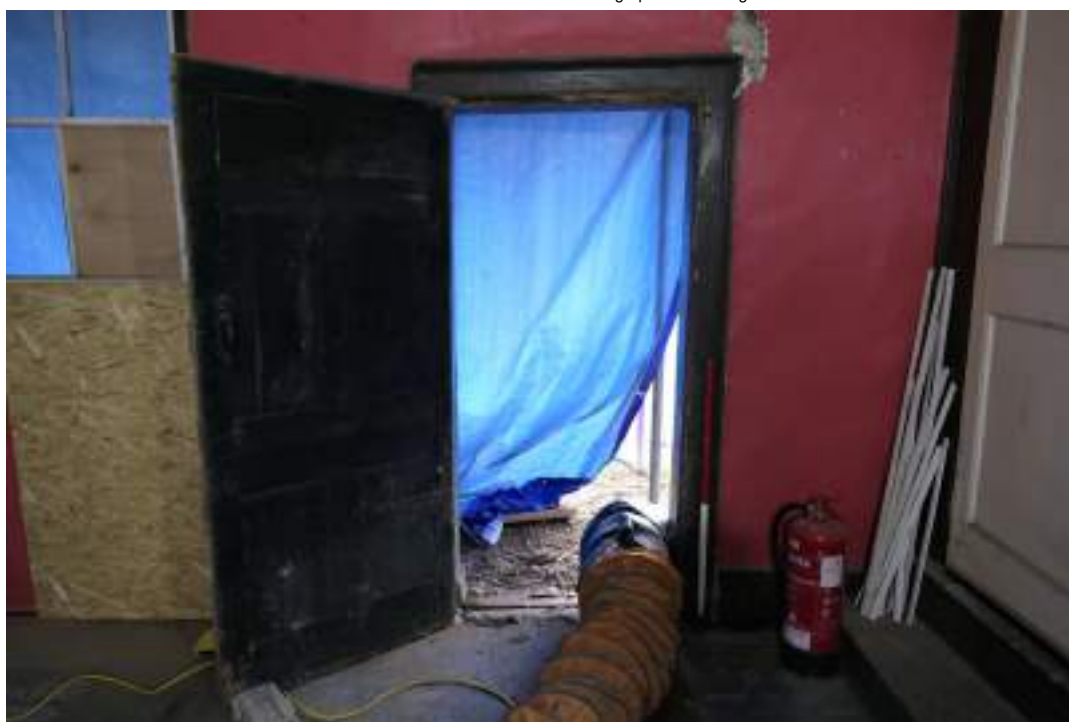
EEX62136_Photograph_099 Detail of door in north-western wall of office. Photograph taken facing north-west.
