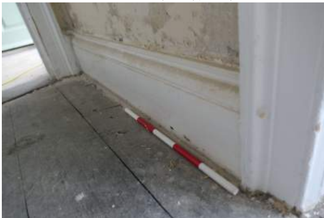
EEX62136_Photograph_139 Detail of skirting board in south-eastern wall of living room. Photograph taken facing east.
