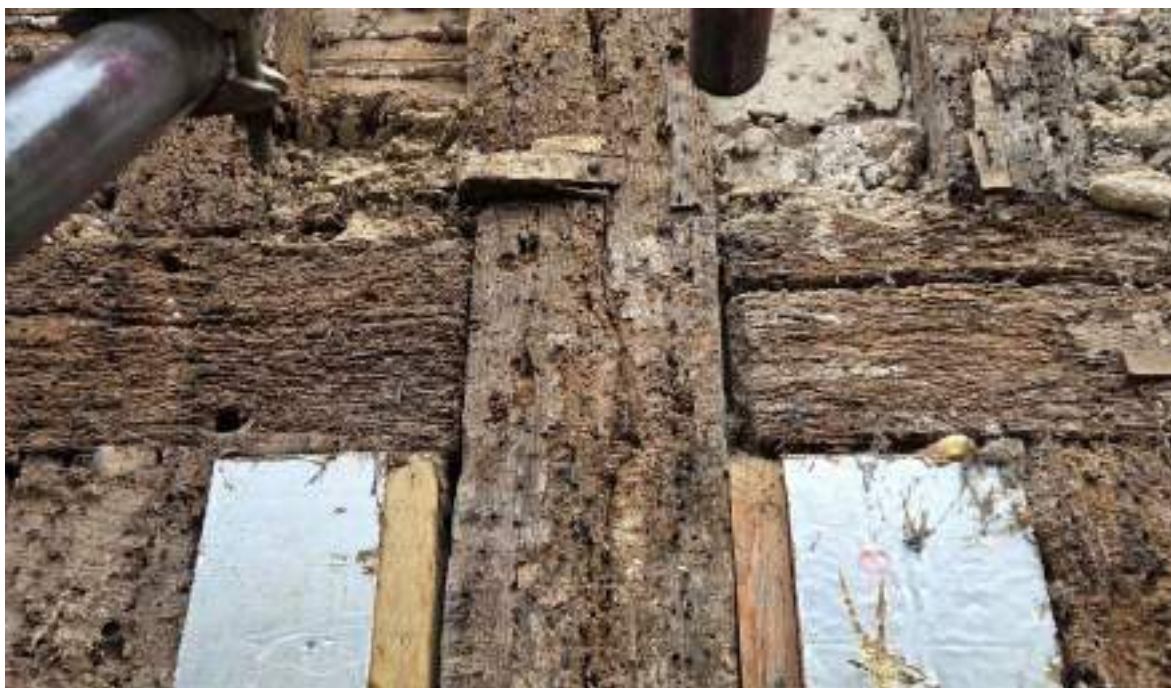
Photograph 14 Detail of intermediate post interrupting girding beam with an iron strap in south-western elevation (range 7). Photograph taken facing north-east.
