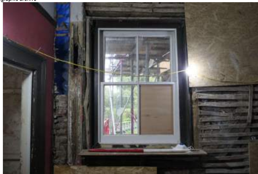
EEX62136_Photograph_098 Detail of window and exposed timber-framing in south-eastern wall of office. Photograph taken facing south-east.
