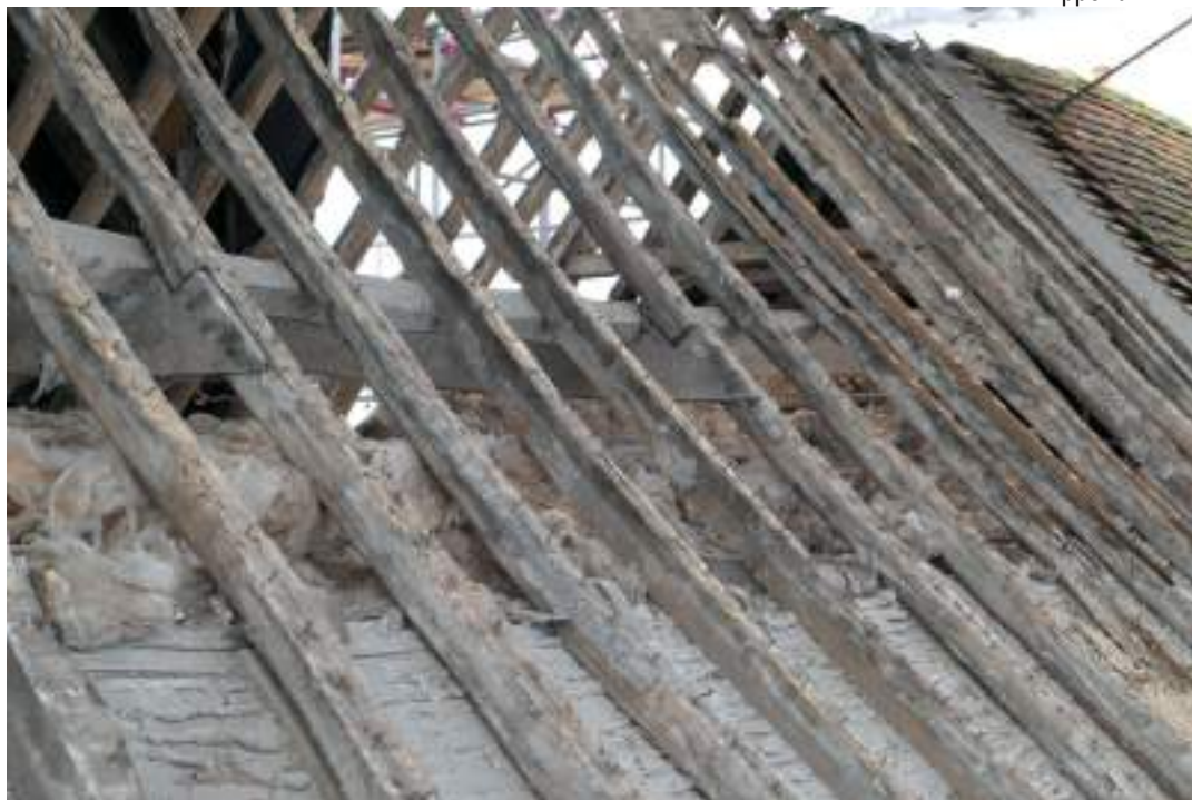
EEX62136_Photograph_061 Detail of lap-dovetail joints securing collars in roof of range 6. Photograph taken facing south.
