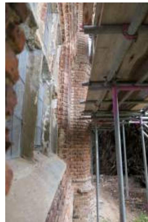
EEX62136_Photograph_018 Detail of octagonal corner buttress on south-western elevation (range 3). Photograph taken facing south-east.
