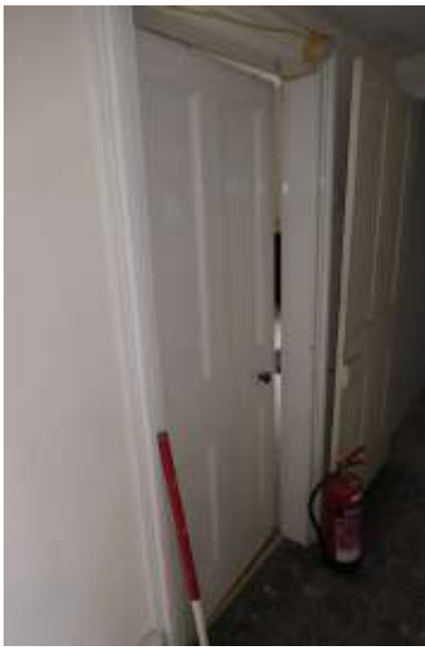
EEX62136_Photograph_209 Detail of doorway in north-western wall of corridor 4. Photograph taken facing north.
