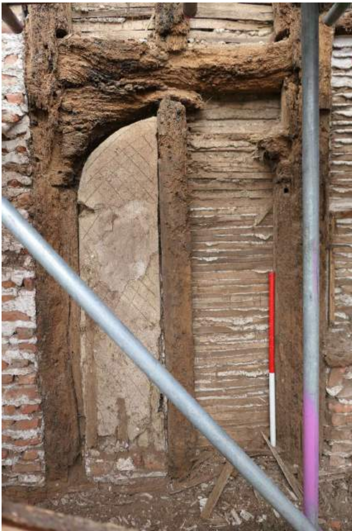
Photograph 7 Detail of doorway in south-eastern elevation (range 5). Photograph taken facing north-west.
