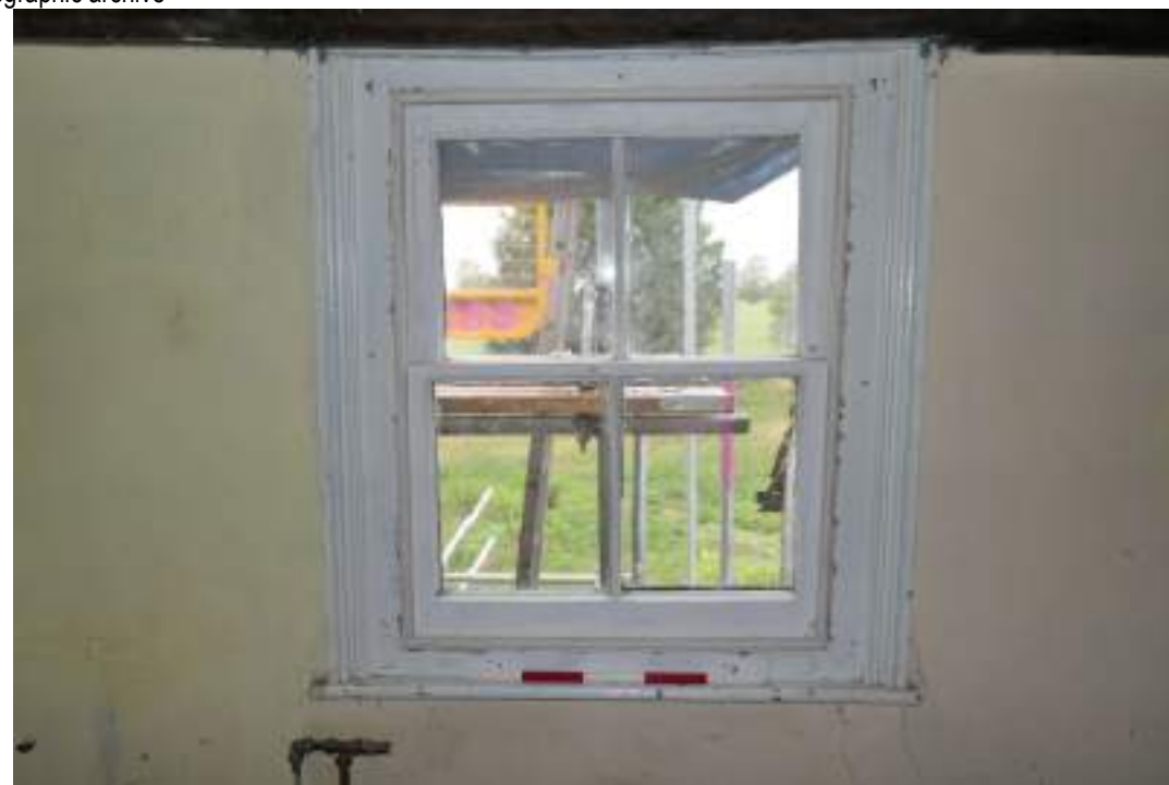
EEX62136_Photograph_222 Detail of window in north-western wall of bedroom 5. Photograph taken facing north-west.
