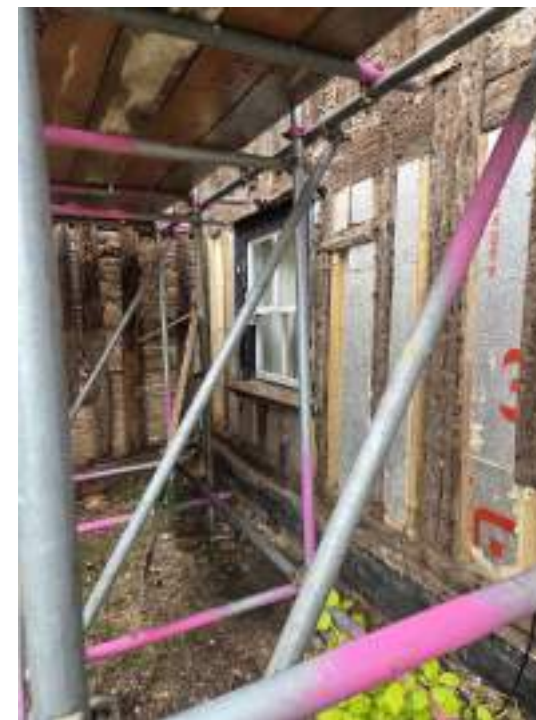
EEX62136_PhotoGraph_036 Detail of exposed timber-framing of south-western elevation (range 7). Photograph taken facing north.
