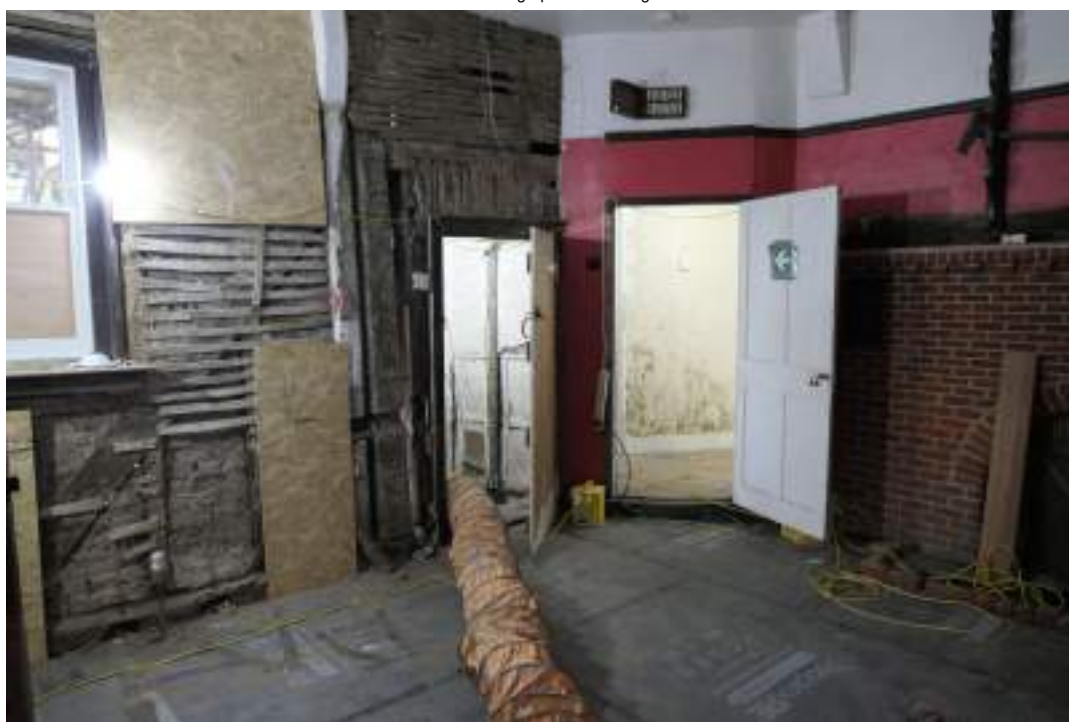
EEX62136_Photograph_095 Interior of office. Photograph taken facing north-east.
