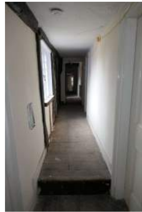
EEX62136_PhotoGraph_198 Interior of corridor 4. Photograph taken facing south-west.
