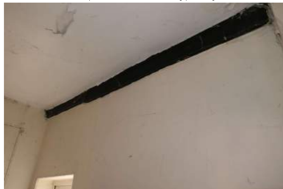
EEX62136_Photograph_168 Detail of exposed wall-plate in cupboard in corridor 3. Photograph taken facing west north-west.
