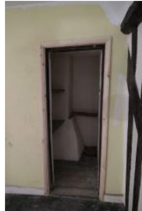
EEX62136_Photograph_256 Detail of hidden alcove in bedroom 4. Photograph taken facing south-west.
