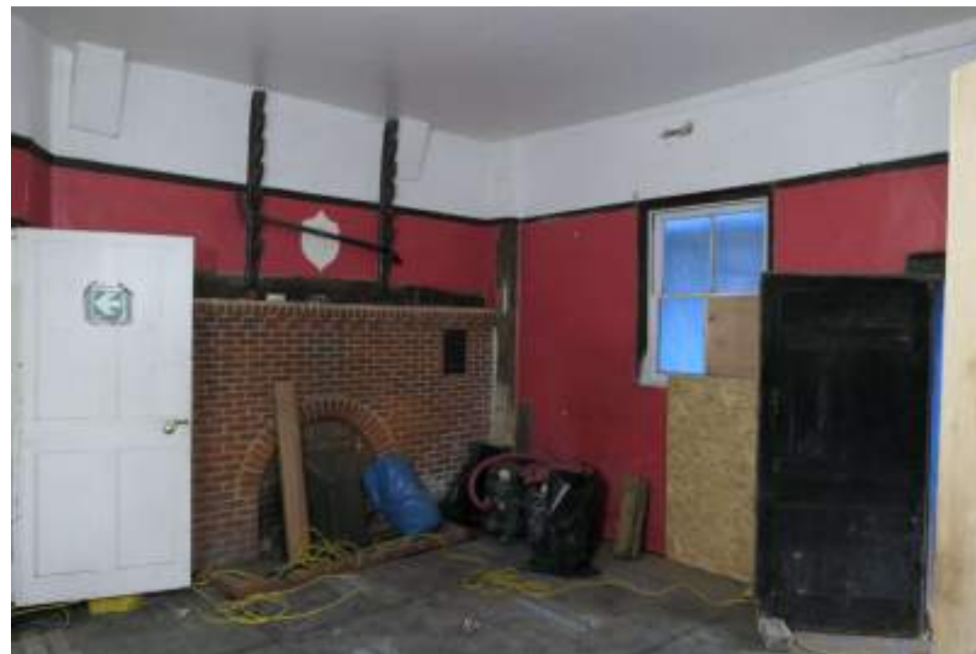
EEX62136_Photograph_092 Interior of office. Photograph taken facing north-west.
