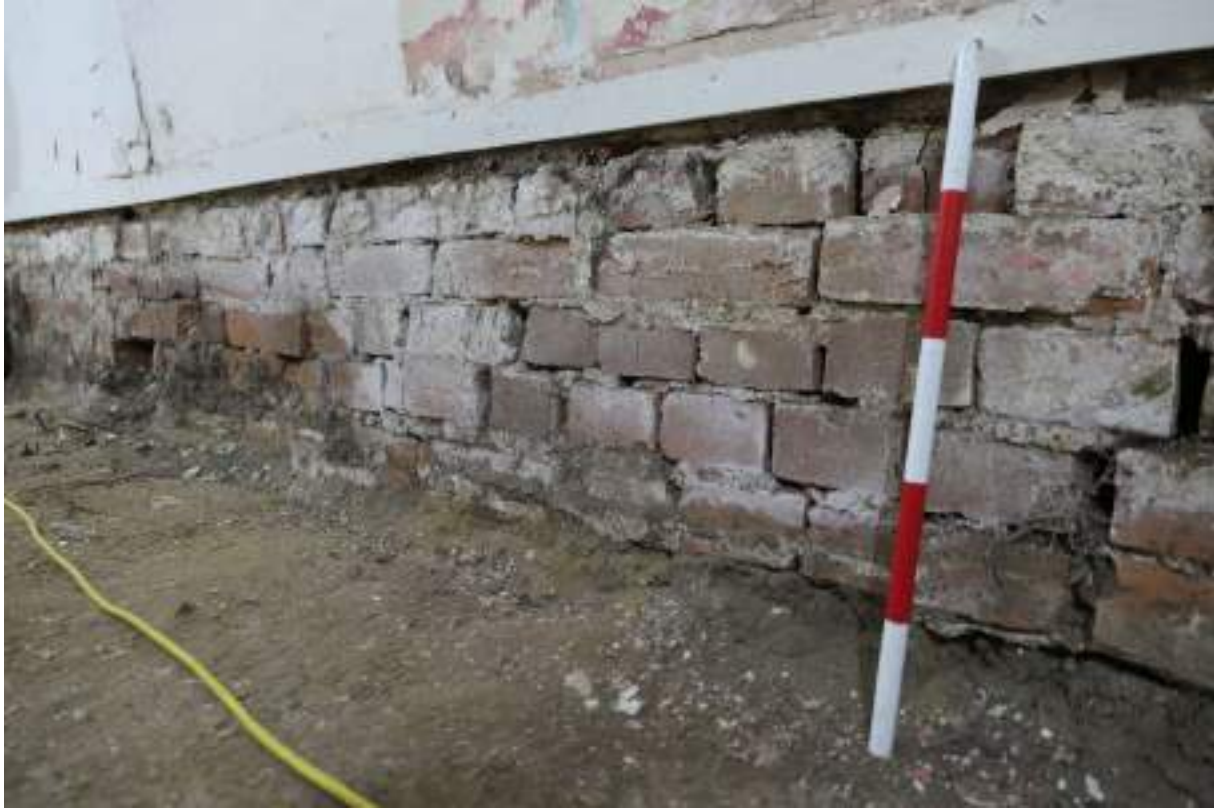
Photograph 34 Detail of brick plinth visible in south-eastern wall of corridor 2. Photograph taken facing east south-east.
