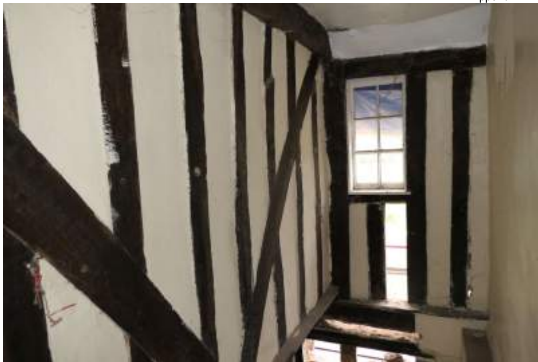
EEX62136_PhotoGraph_237 Interior of rear stairs. Photograph taken facing west north-west.
