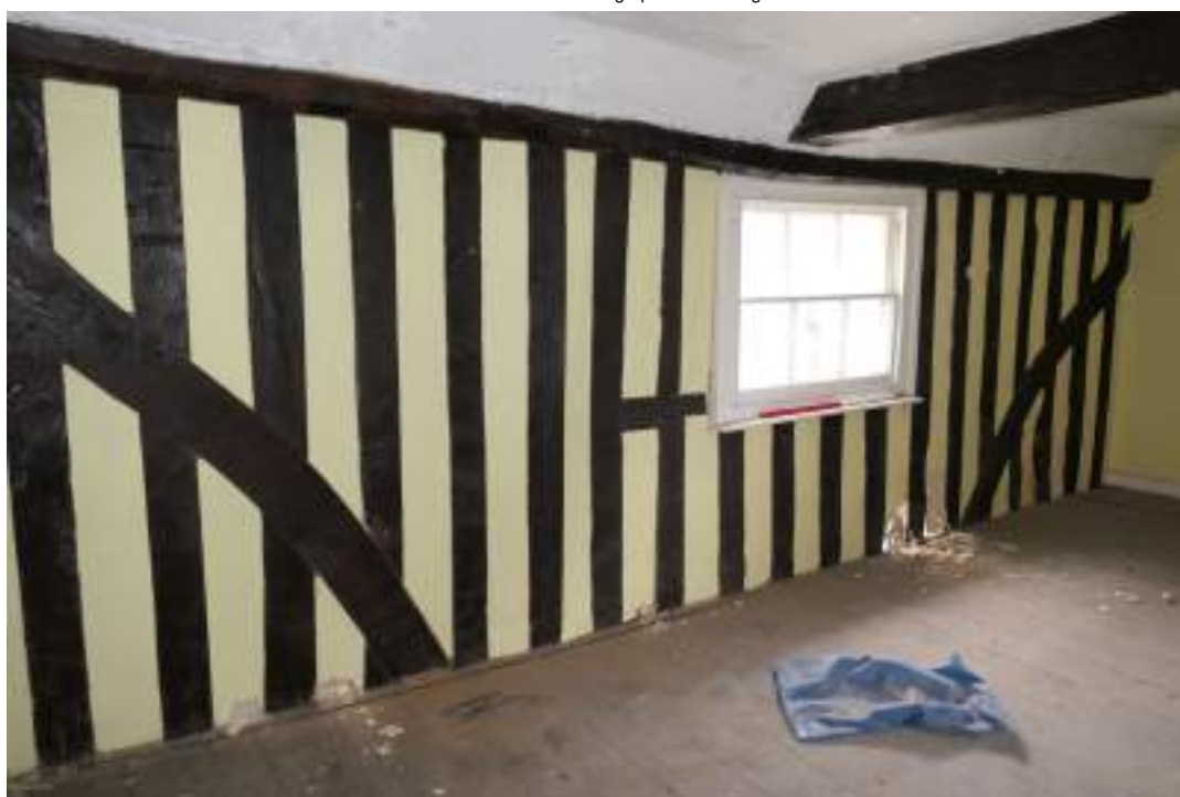
EEX62136_Photograph_231 Detail of exposed timber-framing in north-western wall of bedroom 4. Photograph taken facing north.
