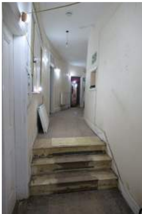
EEX62136_Photograph_111 Interior of corridor 1. Photograph taken facing north-east.
