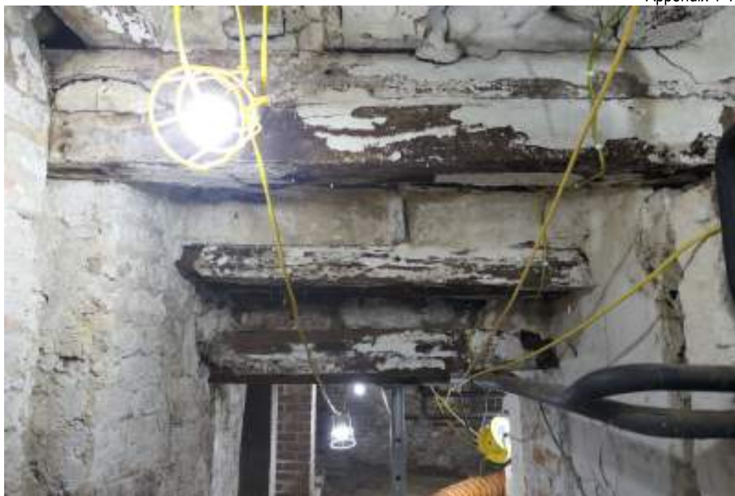
EEX62136_Photograph_057 Detail of roof timbers in basement. Photograph taken facing south-west.
