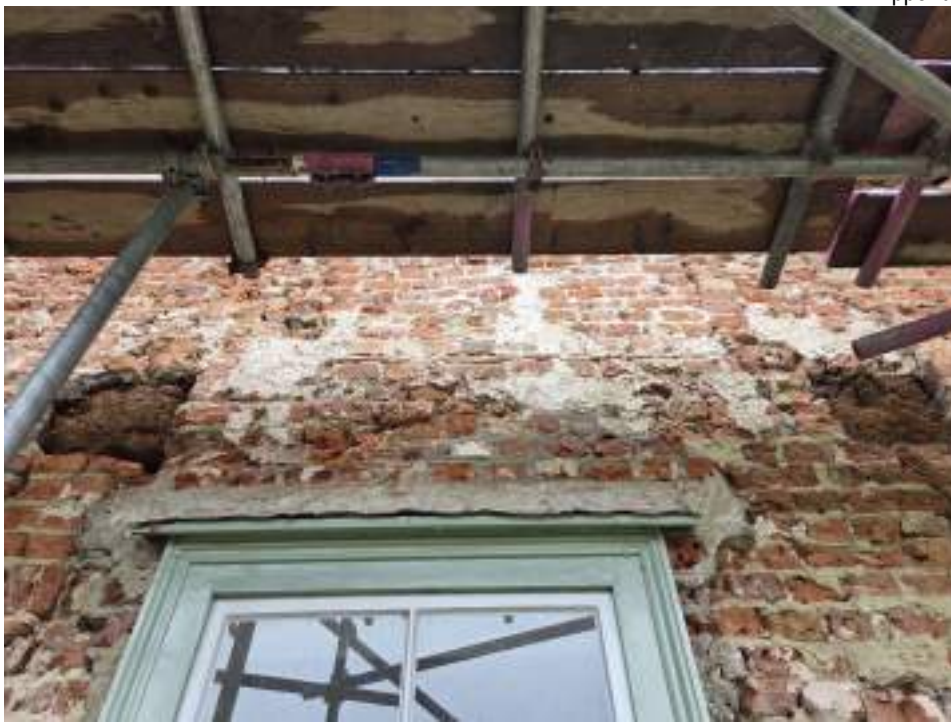
EEX62136_PhotoGraph_009 Detail of tiles in the brickwork of the south-eastern elevation (range 3). Photograph taken facing north-west.
