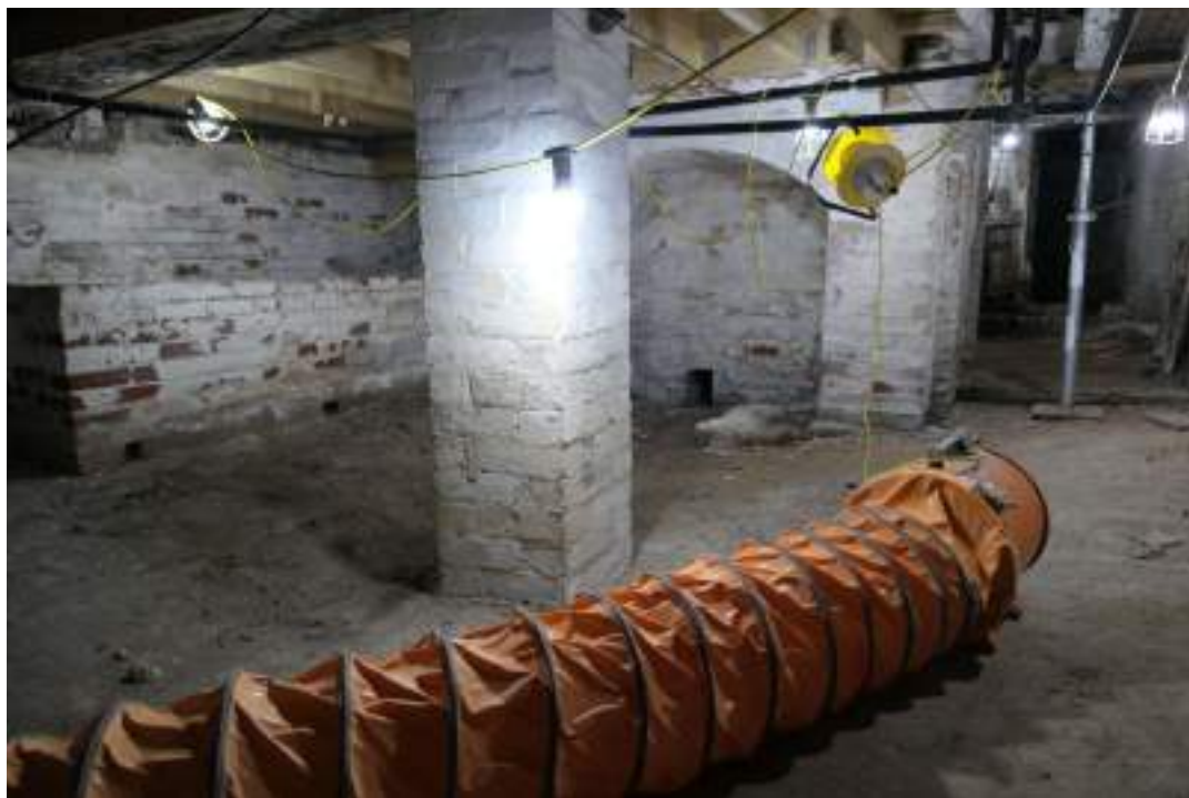
EEX62136_Photograph_251 Interior of basement. Photograph taken facing north.
