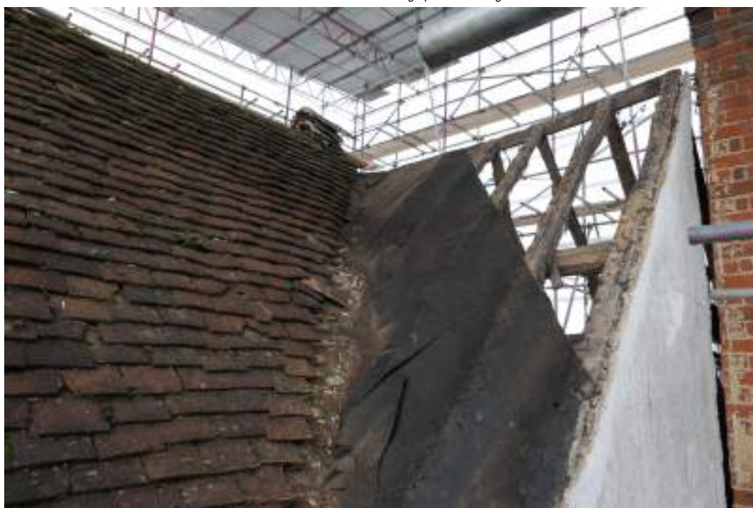
EEX62136_Photograph_059 Detail of roof above ranges 6 and 7. Photograph taken facing west.
