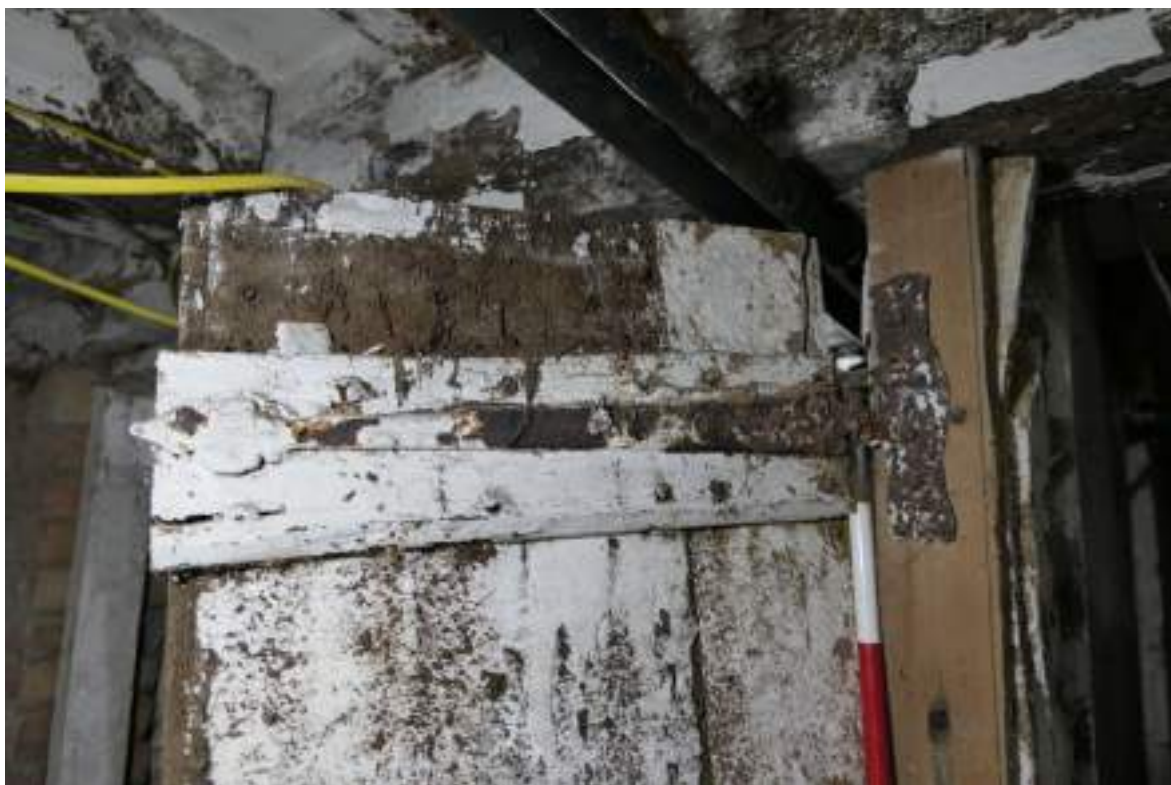
Photograph 23 Detail of strap hinge on door in basement. Photograph taken facing north.
