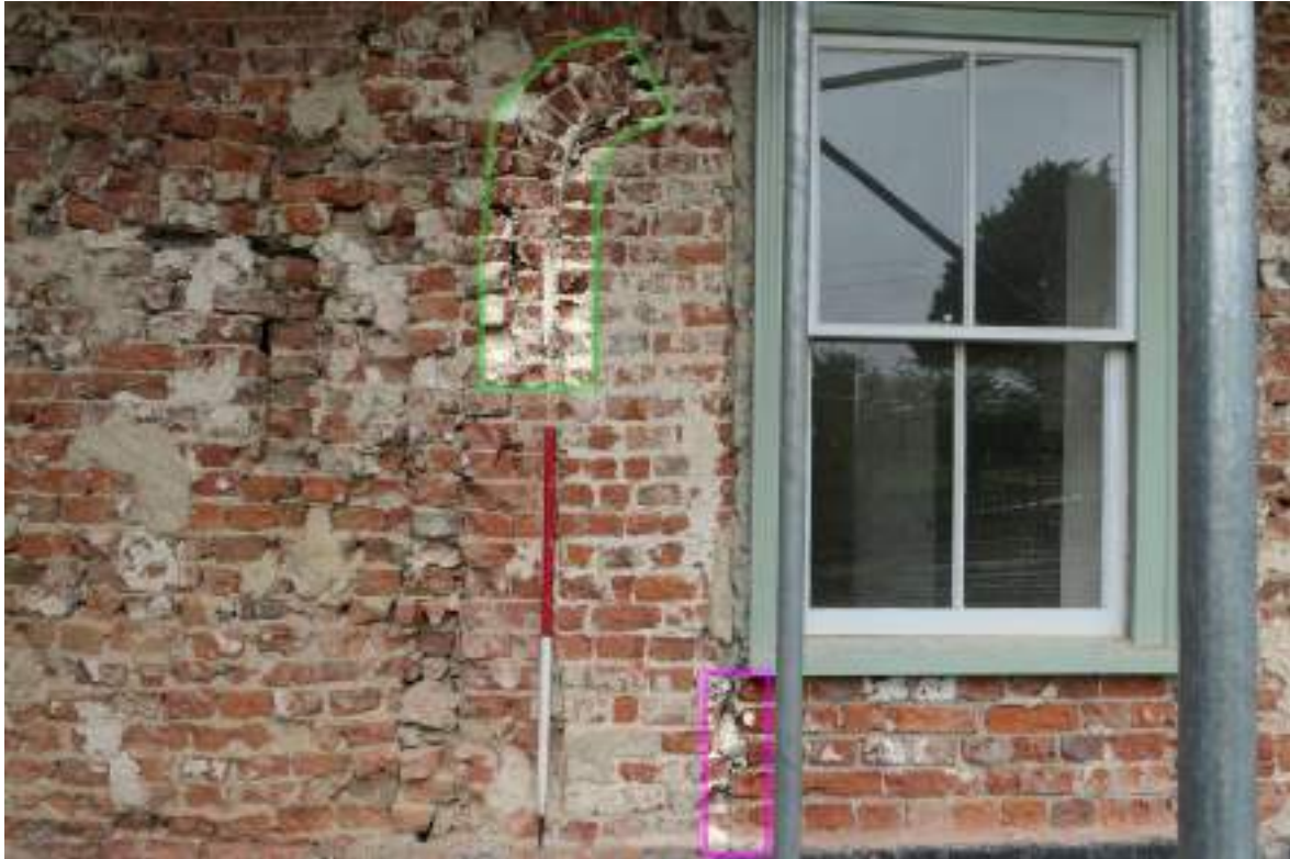
Photograph 4 Detail of blocked, partially surviving brick arch (green) and break in brickwork evidencing blocked doorway (pink) in south-eastern elevation (range 3). Photograph taken facing north-west.
