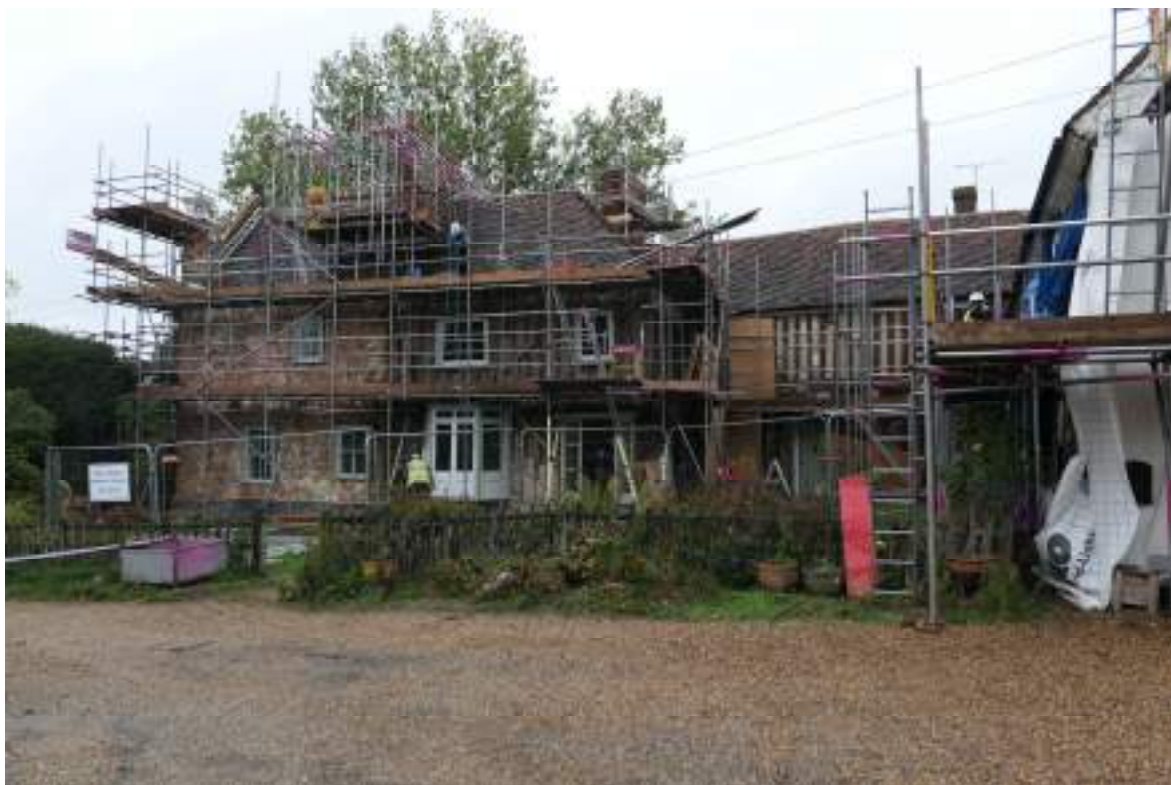
Photograph 1 South-eastern elevation (ranges 3, 4 and 5). Photograph taken facing west north-west.
