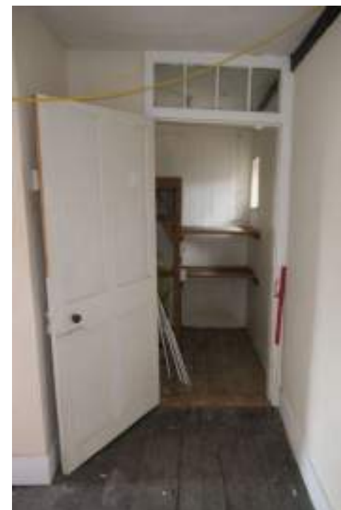
EEX62136_Photograph_166 Detail of door to cupboard in north-western wall of corridor 3. Photograph taken facing north-west.
