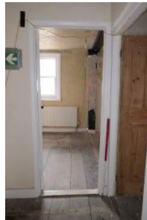
EEX62136_Photograph_160 Detail of door in south-eastern wall of corridor 3. Photograph taken facing south-east.
