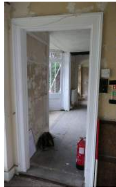
EEX62136_Photograph_126 Detail of door in south-western wall of entrance hall. Photograph taken facing south-west.
