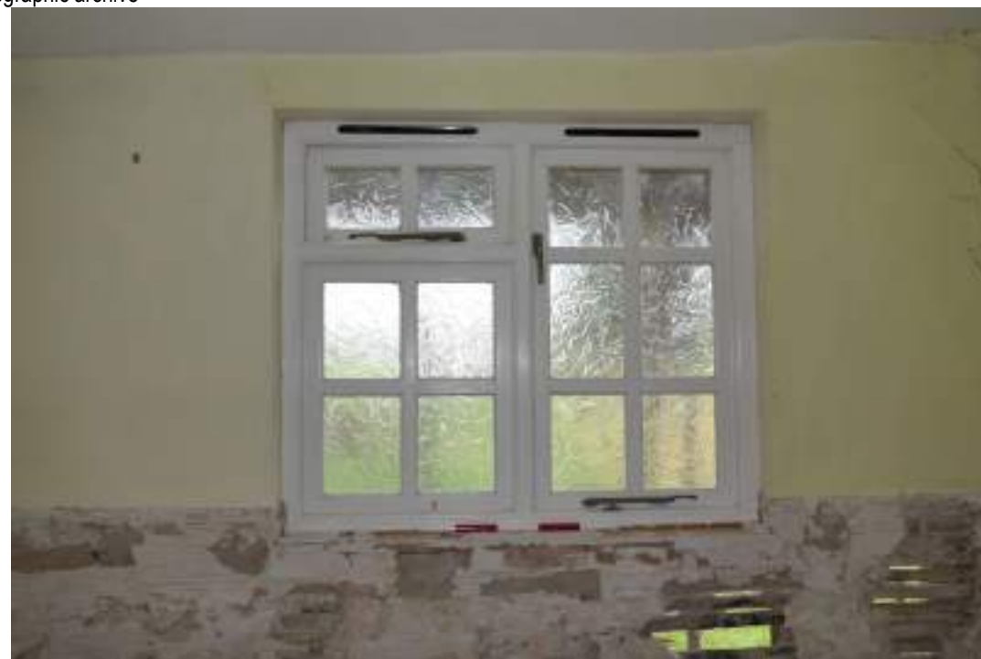
EEX62136_Photograph_142 Detail of window in north-western wall of bathroom. Photograph taken facing north-west.
