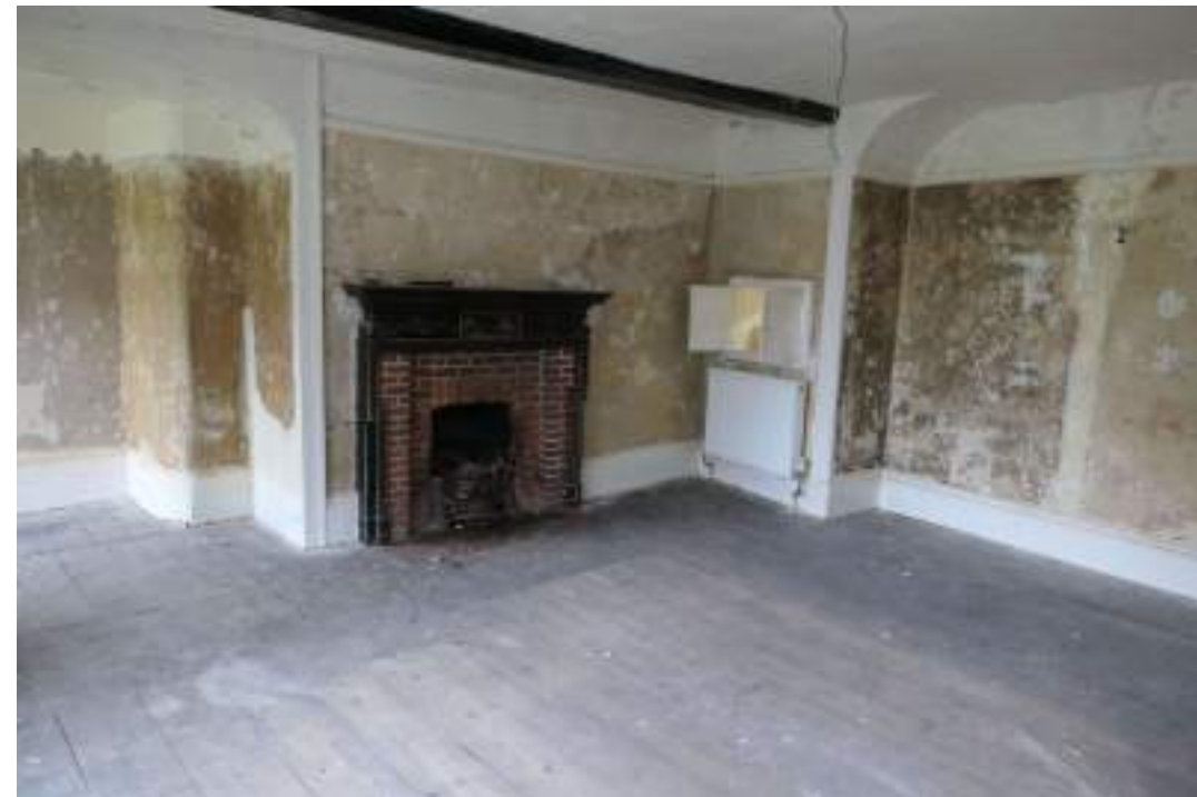
EEX62136_Photograph_128 Interior of living room. Photograph taken facing west.
