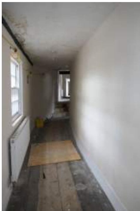
EEX62136_Photograph_159 Interior of corridor 3. Photograph taken facing south-east.
