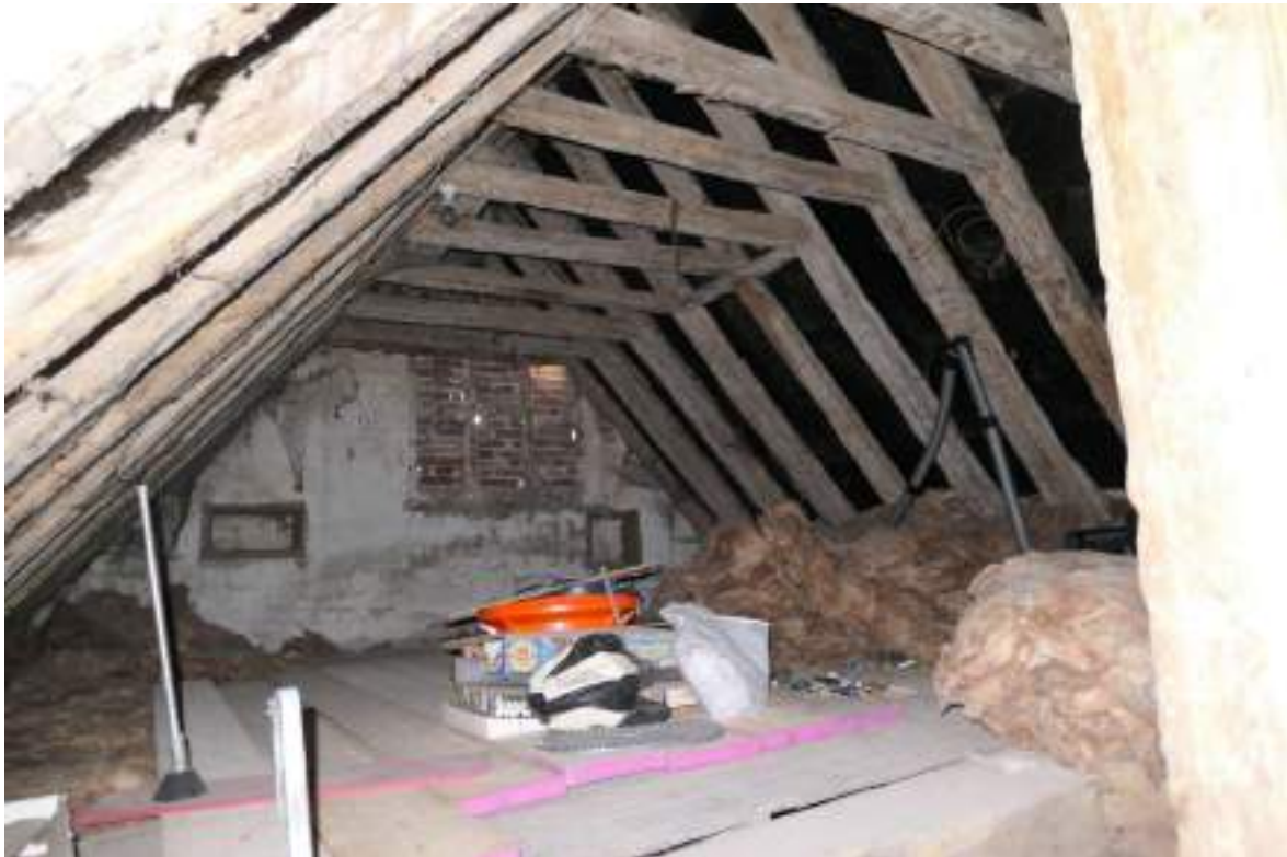
Photograph 18 Detail of roof construction above range 3. Photograph taken facing west.
