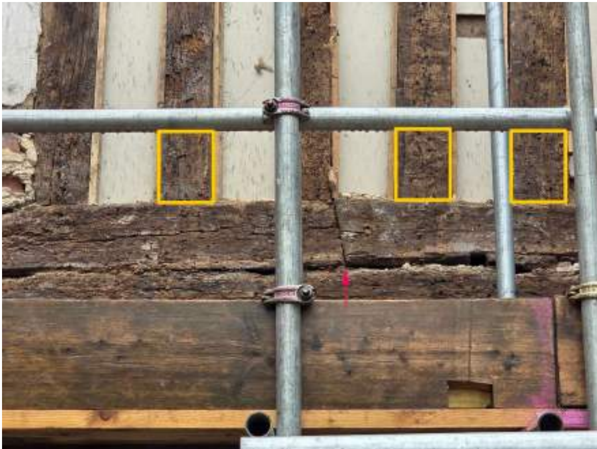
Photograph 8 Detail of scarf-joint in girding beam (pink arrow) and possible carpenter's marks (outlined in yellow, details shown in Photograph 9) on studs in south-eastern elevation (range 5). Note the double girding beam. Photograph taken facing north-west.
