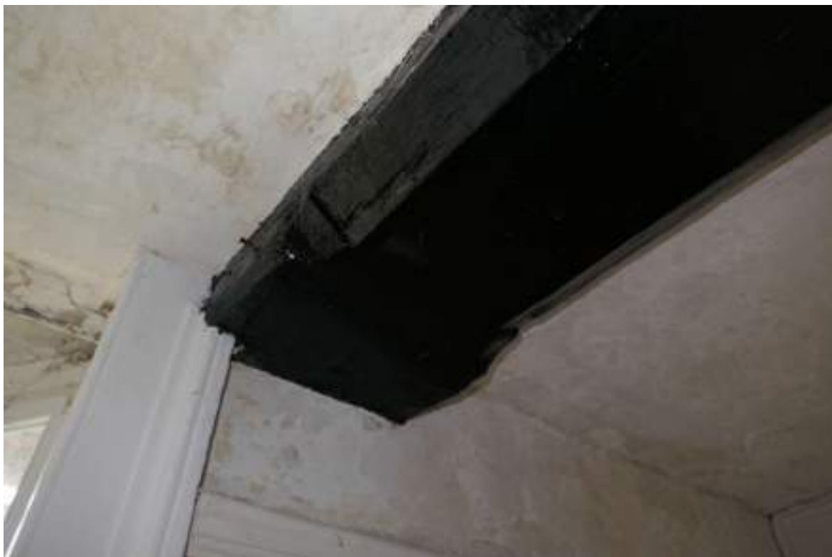
Photograph 27 Detail of curved stepped stop on chamfered binding beam in ceiling of living room. Photograph taken facing south.
