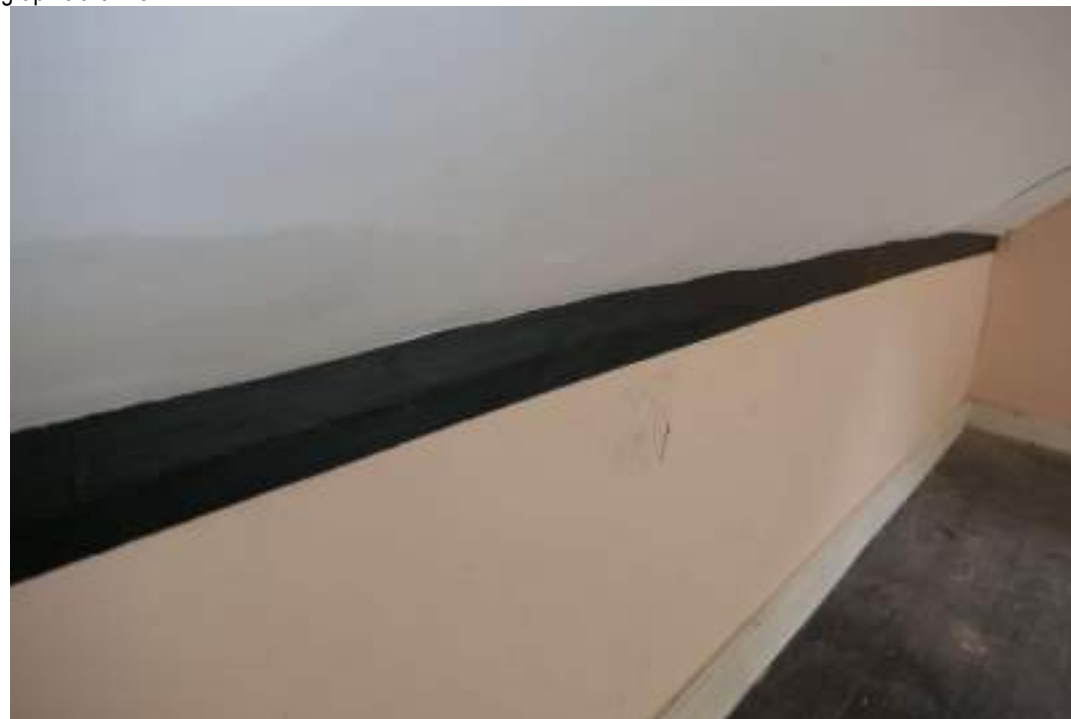
EEX62136_Photograph_218 Detail of exposed beam in north-western wall of bedroom 6. Photograph taken facing north.
