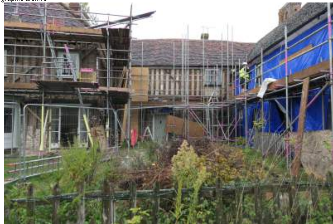
EEX62136_PhotoGraph_022 South-eastern elevation (range 5). Photograph taken facing north-west.
