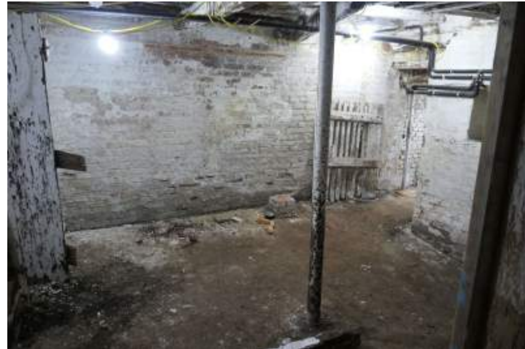
EEX62136_PhotoGraph_240 Interior of basement. Photograph taken facing south.
