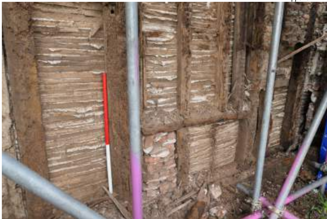
EEX62136_PhotoGraph_033 Detail of exposed timber-framing in south-eastern elevation (range 5). Photograph taken facing north.
