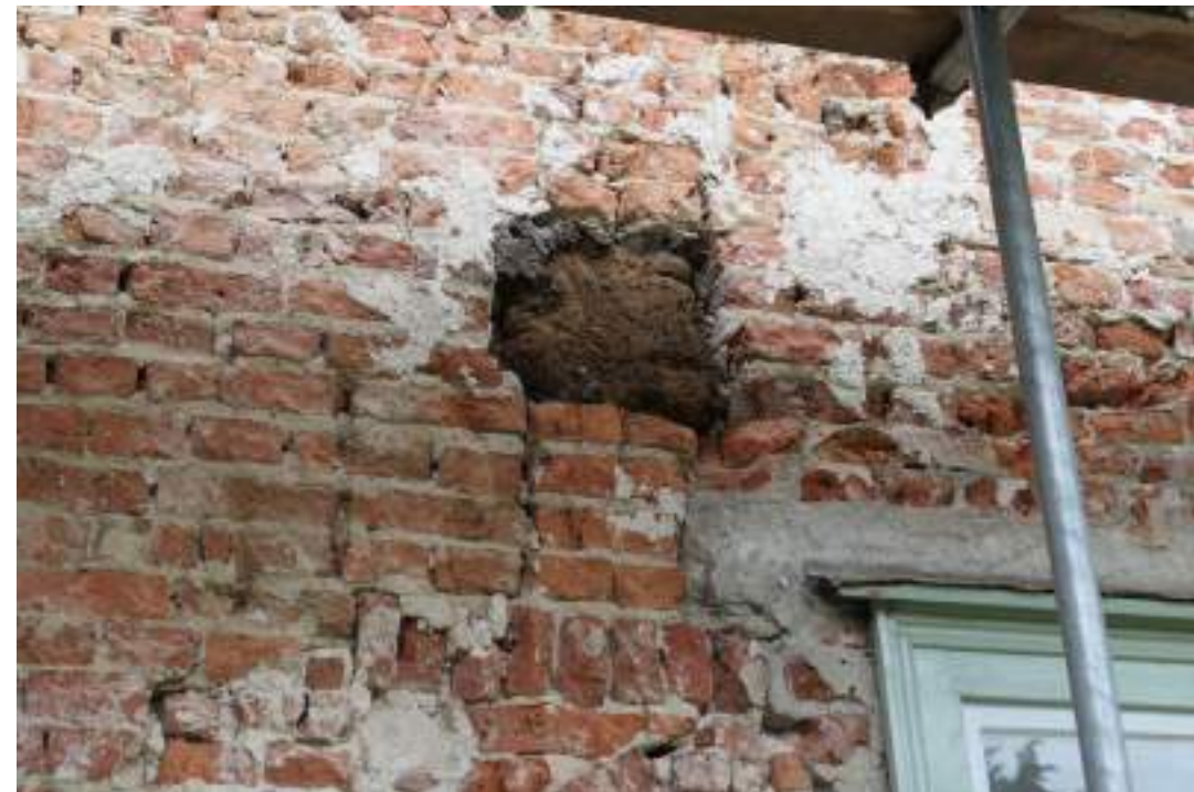
EEX62136_PhotoGraph_012 Detail of exposed binding beam visible in south-eastern elevation (range 3). Photograph taken facing north north-west.
