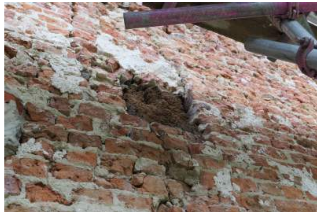
EEX62136_PhotoGraph_016 Detail of exposed binding beam in brickwork of south-eastern elevation (range 3). Photograph taken facing north.
