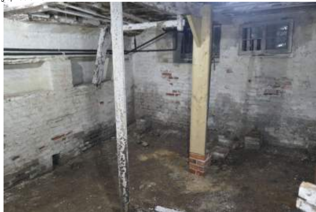
EEX62136_PhotoGraph_242 Interior of basement. Photograph taken facing west.
