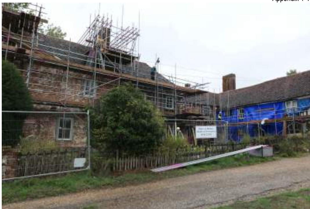
EEX62136_Photograph_053 South-eastern elevation (ranges 3, 4 and 5). Photograph taken facing north.
