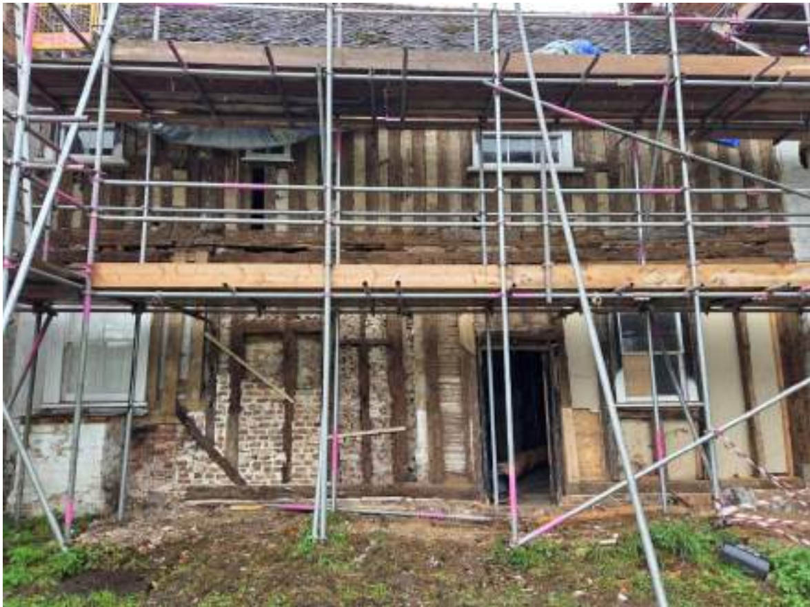
Photograph 16 Detail of exposed timber-framing of north-western elevation (range 5). Note the double girding beam. Photograph taken facing south-east.
