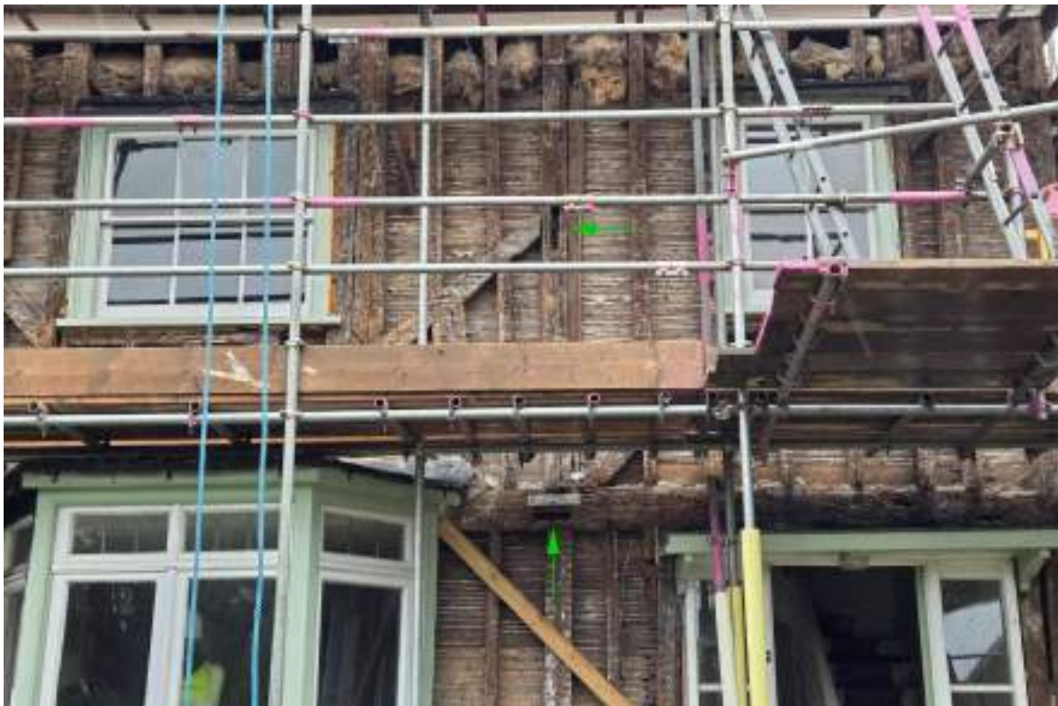
Photograph 5 Detail of exposed timber-framing, with reused timbers highlighted by green arrows, of south-eastern elevation (range 4). Photograph taken facing north-west.
