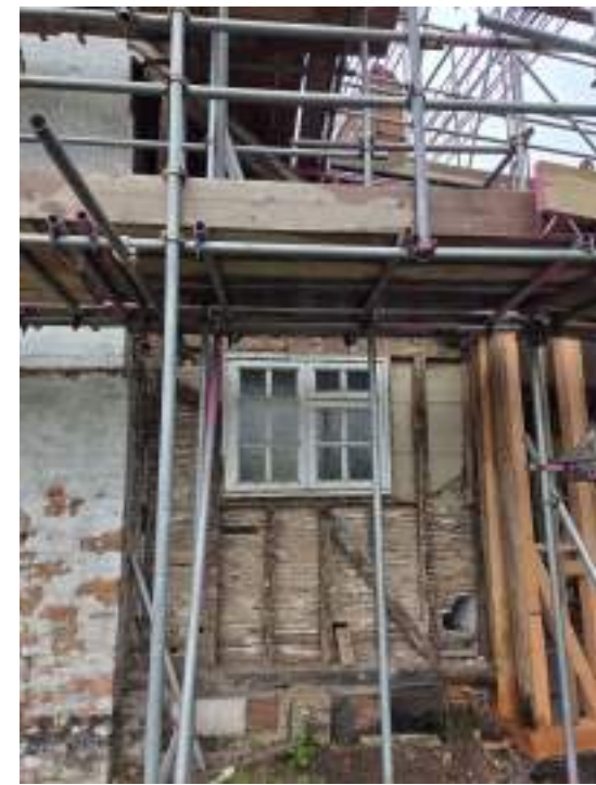
EEX62136_PhotoGraph_042 Detail of exposed timber-framing of north-western elevation (range 2). Photograph taken facing south-east.
