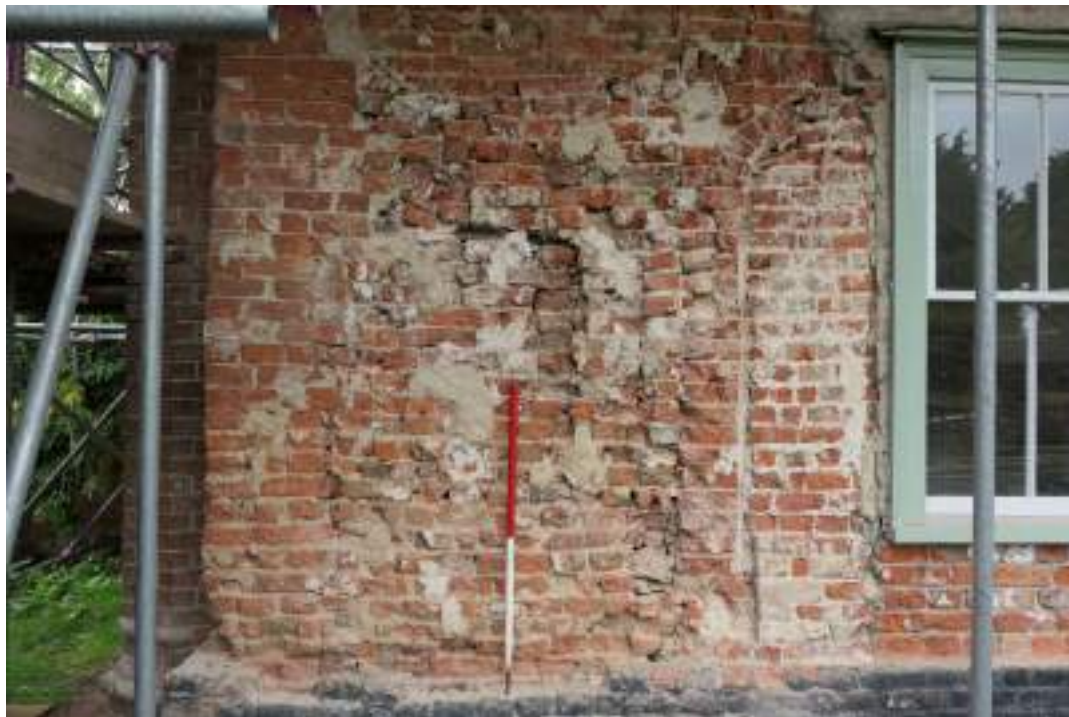
EEX62136_PhotoGraph_011 Detail of brickwork in south-eastern elevation (range 3). Photograph taken facing north-west.
