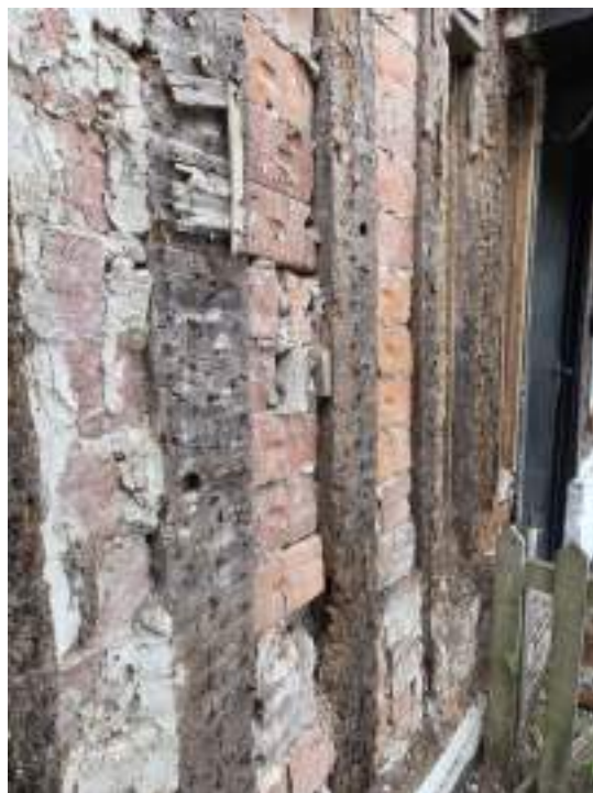
EEX62136_PhotoGraph_035 Detail of exposed timber-framing in south-western elevation (range 7). Photograph taken facing east.
