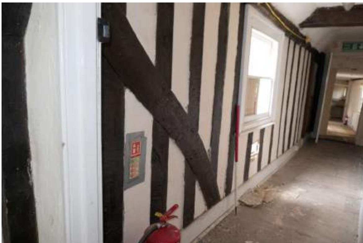
Photograph 41 Detail of exposed timber-framing in south-eastern wall of corridor 4. Photograph taken facing south.
