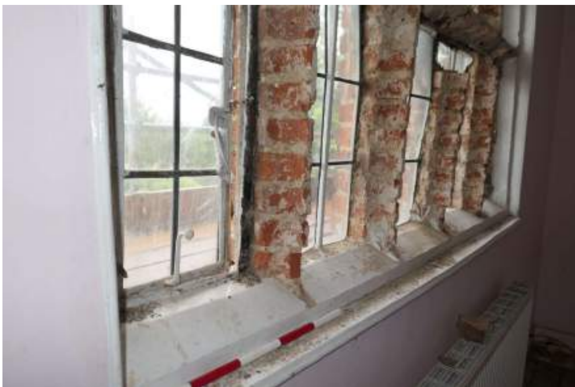
Photograph 37 Detail of brick mullions in window in south-western wall of bedroom 1. Photograph taken facing west.
