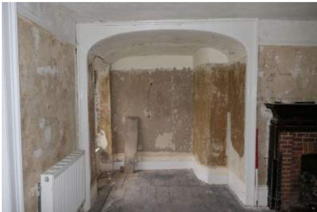
EEX62136_Photograph_135 Detail of arch in south-western wall of living room. Photograph taken facing south-west.
