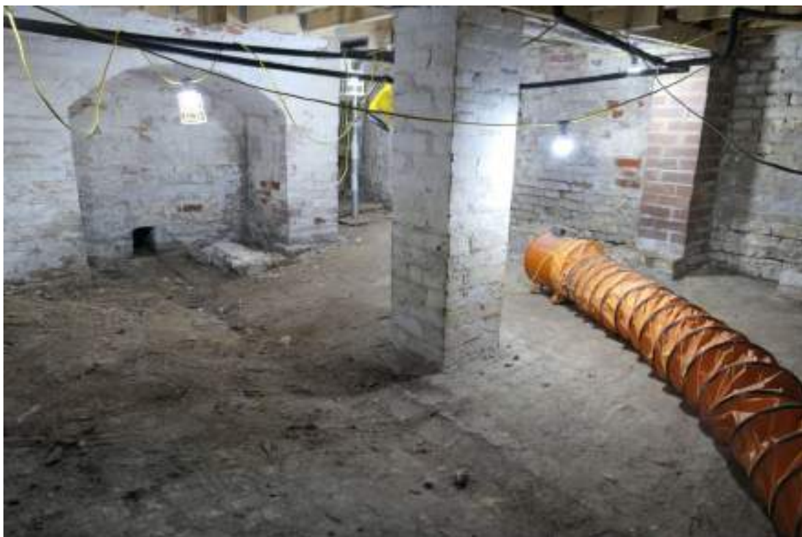
Photograph 22 Interior of basement. Photograph taken facing east.
