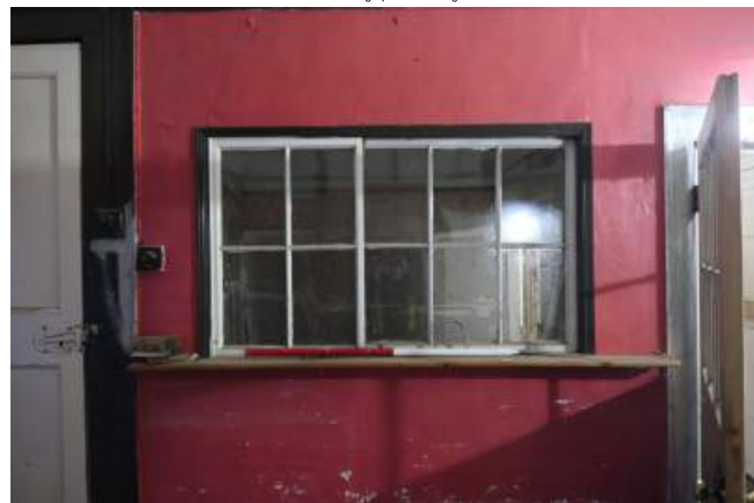
EEX62136_Photograph_096 Detail of interior window between store and office. Photograph taken facing north-east.
