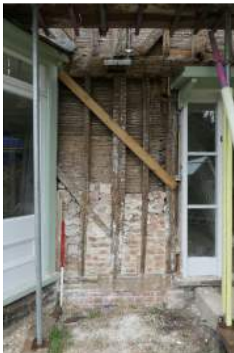
EEX62136_Photograph_047 Detail of timber-framing in south-eastern elevation (range 4). Photograph taken facing north-west.
