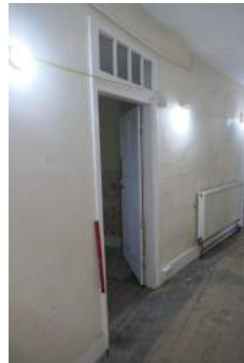
EEX62136_Photograph_122 Detail of doorway in north-western wall of corridor 1. Photograph taken facing north.
