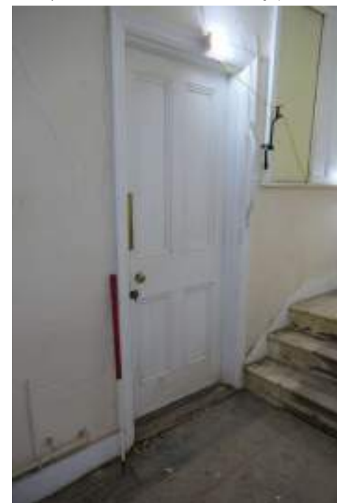
EEX62136_Photograph_124 Detail of door in north-western wall of corridor 1. Photograph taken facing north.
