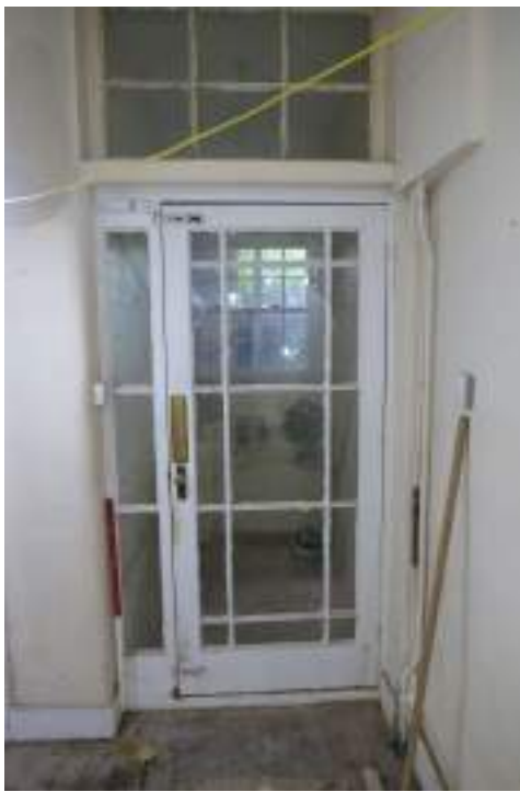
EEX62136_Photograph_125 Detail of door to pantry (inaccessible). Photograph taken facing south-west.
