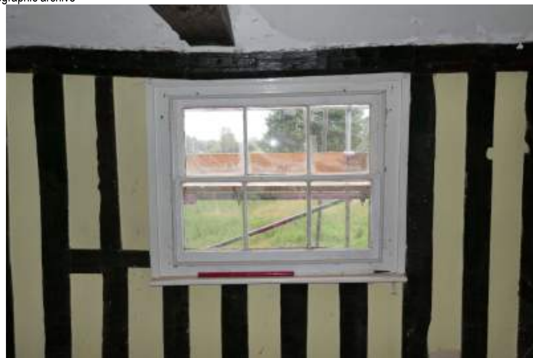
EEX62136_Photograph_230 Detail of window in north-western wall of bedroom 4. Photograph taken facing north-west.
