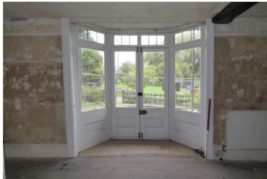
EEX62136_Photograph_136 Detail of canted bay window in south-eastern wall of living room. Photograph taken facing south-east.
