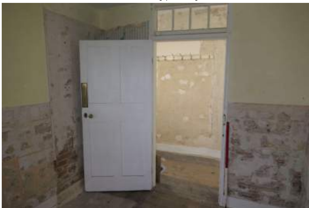
EEX62136_Photograph_143 Detail of door in south-eastern wall of bathroom. Photograph taken facing south-east.
