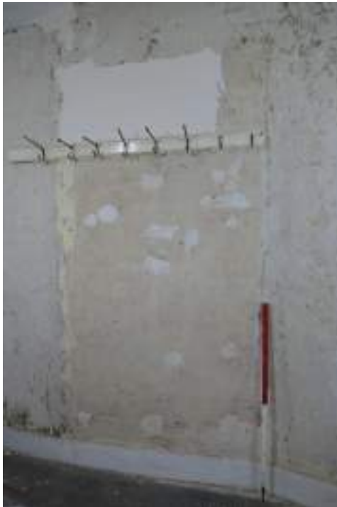
EEX62136_Photograph_119 Detail of blocked doorway in south-eastern wall of corridor 1. Photograph taken facing east south-east.
