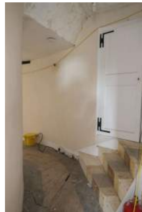
EEX62136_Photograph_158 Interior of corridor 3. Photograph taken facing north-west.
