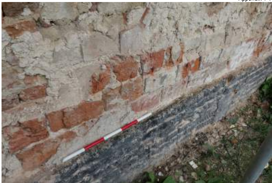
EEX62136_Photograph_017 Detail of bricks laid on-edge in brickwork and plinth of south-eastern elevation (range 3). Photograph taken facing north.
