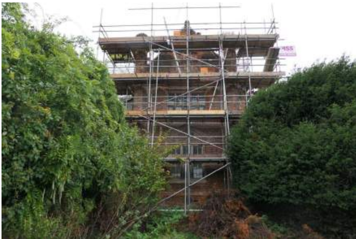
Photograph 10 South-western elevation (range 3). Photograph taken facing north-east.
