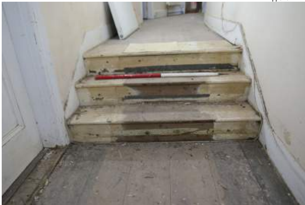
EEX62136_Photograph_121 Detail of stairs in corridor 1. Photograph taken facing north-east.
