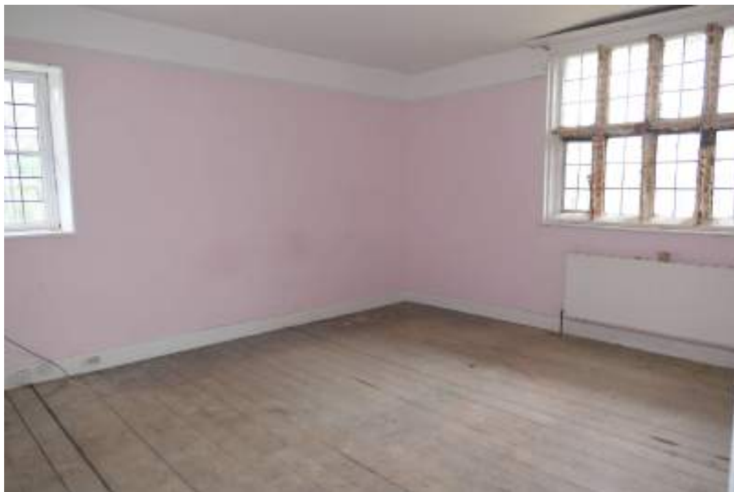
EEX62136_Photograph_171 Interior of bedroom 1. Photograph taken facing south.
