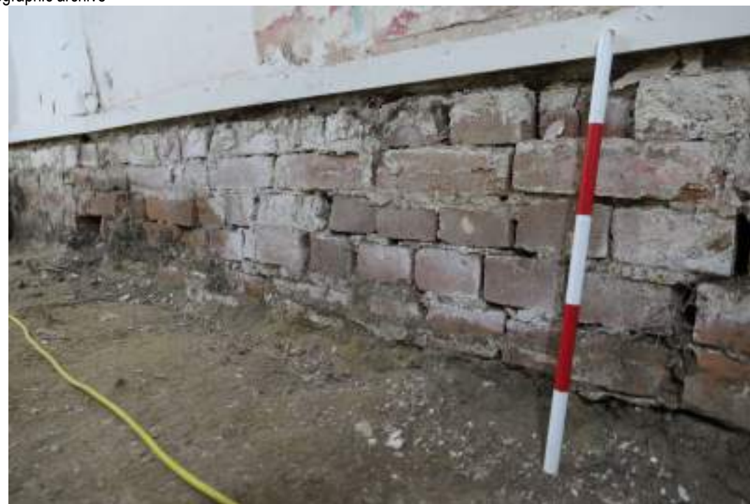
EEX62136_Photograph_074 Detail of brick plinth visible in south-eastern wall of corridor 2. Photograph taken facing east south-east.
