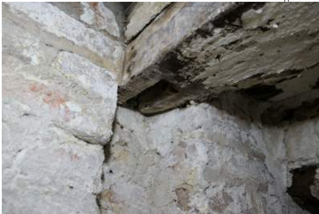
EEX62136_Photograph_249 Detail of empty mortice in ceiling beam in basement. Photograph taken facing south.
