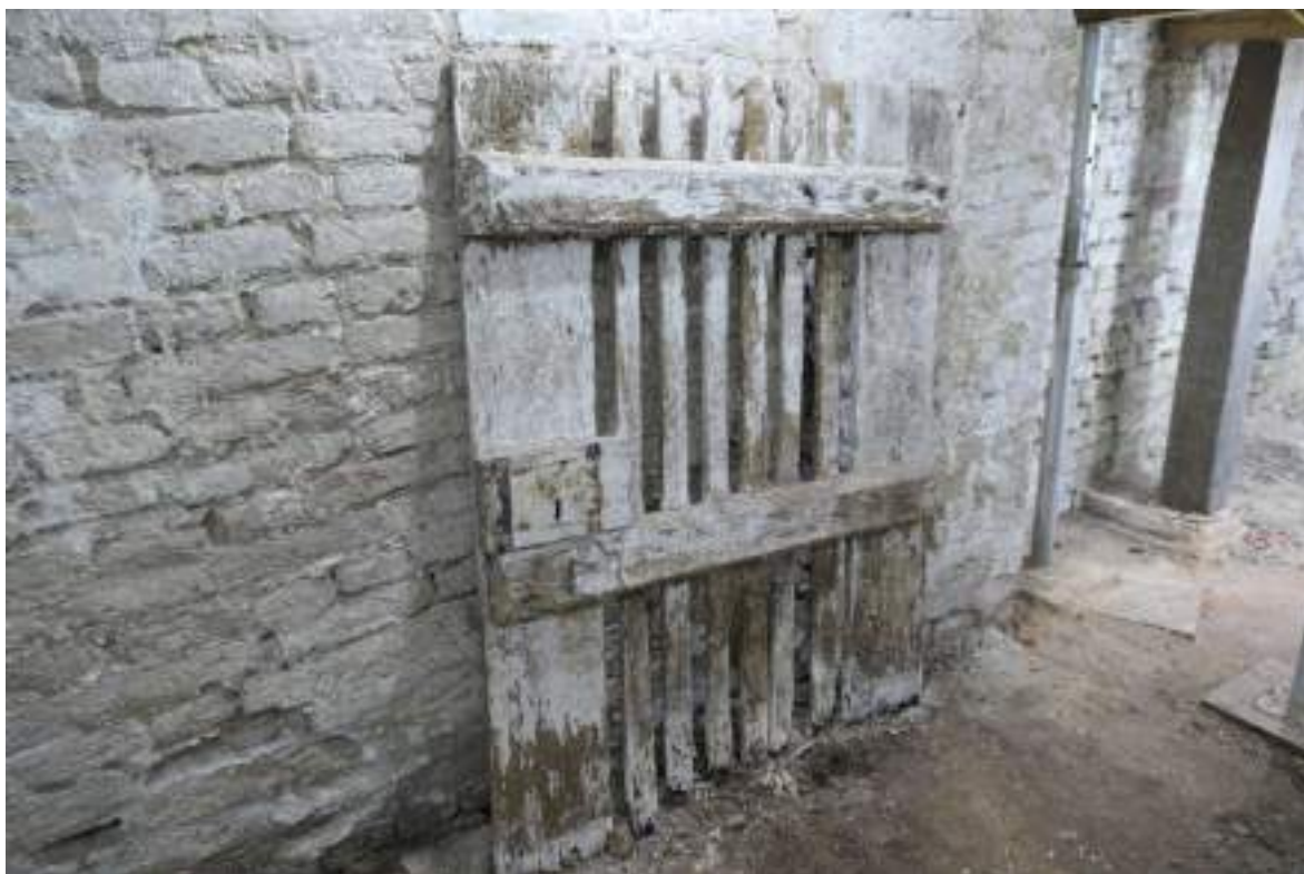
Photograph 24 Detail of door in basement. Photograph taken facing south-east.
