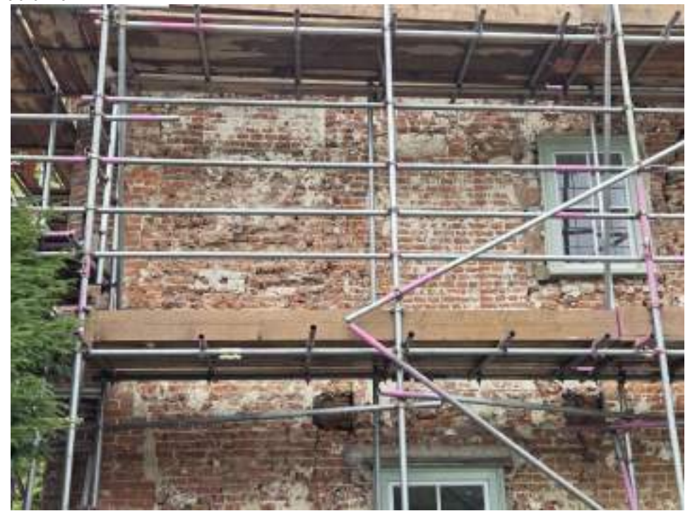
EEX62136_PhotoGraph_010 Detail of brickwork in south-eastern elevation (range 3). Photograph taken facing north-west.
