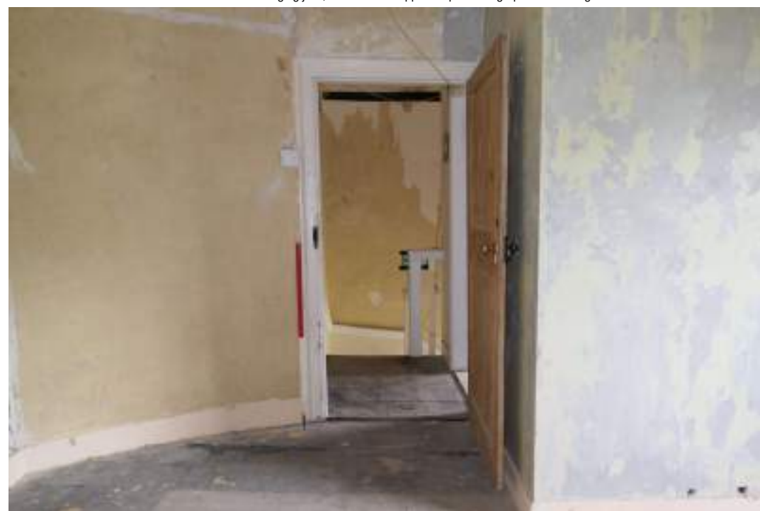
EEX62136_Photograph_188 Detail of door in north-eastern wall of bedroom 2. Photograph taken facing north-east.
