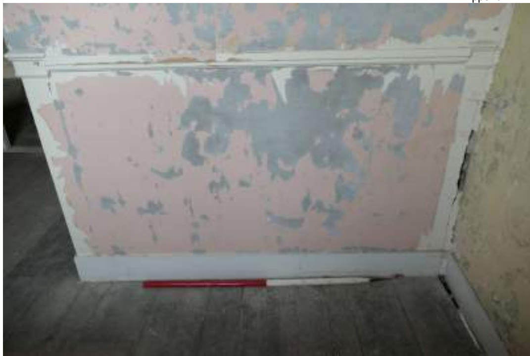
EEX62136_Photograph_193 Detail of stair baultrade incorporated in to wall in bedroom 3. Photograph taken facing north-west.
