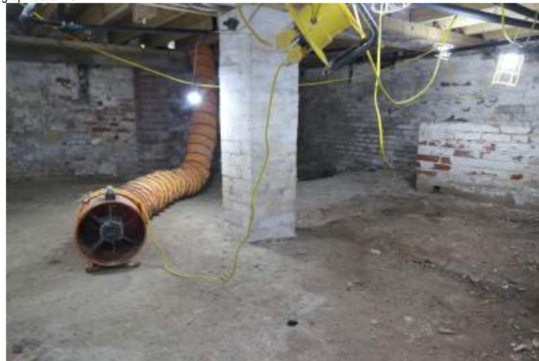
EEX62136_Photograph_250 Interior of basement. Photograph taken facing west.
