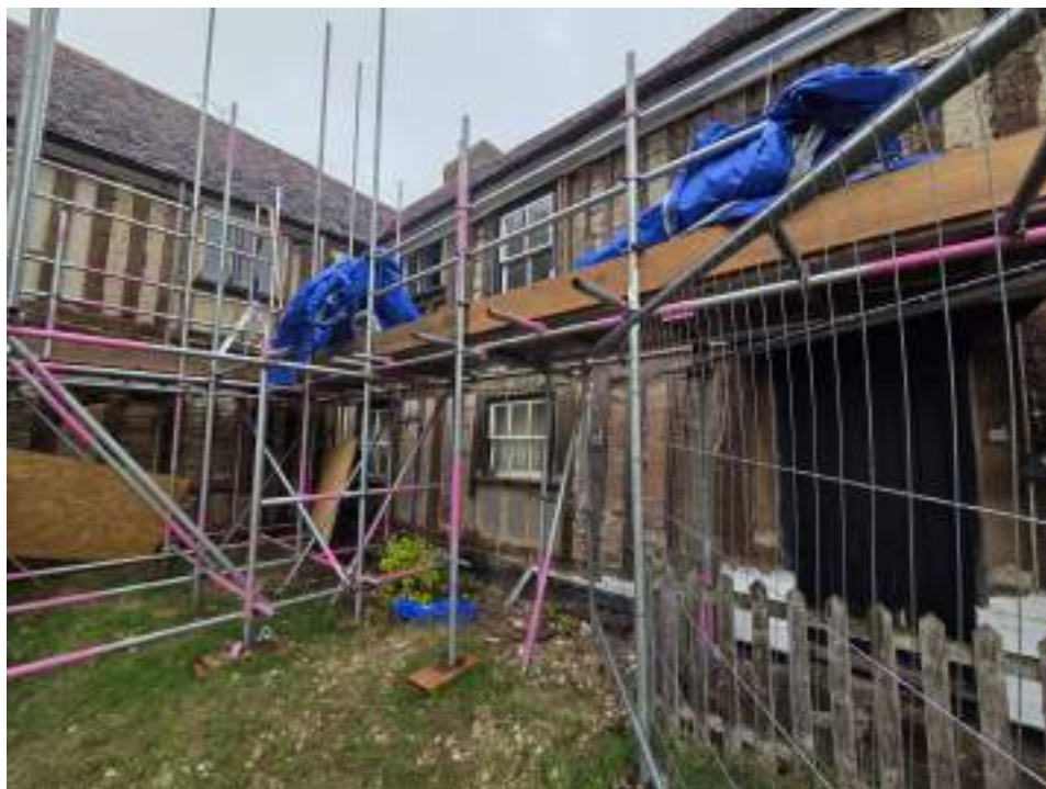
EEX62136_Photograph_019 South-eastern and south-western elevations (ranges 5 and 7). Photograph taken facing north.
