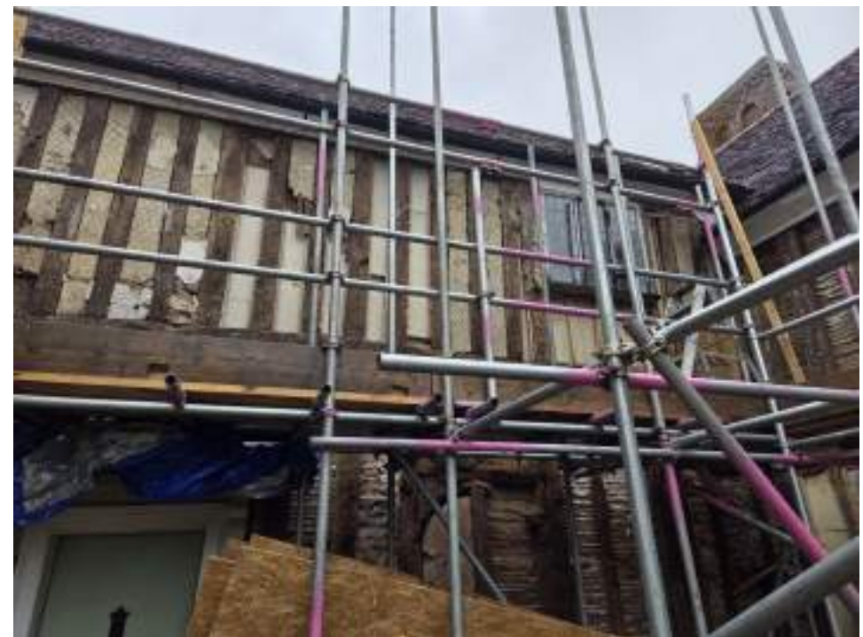
EEX62136_PhotoGraph_024 Detail of exposed timber-framing on upper register of south-eastern elevation (range 5). Photograph taken facing north north-west.
