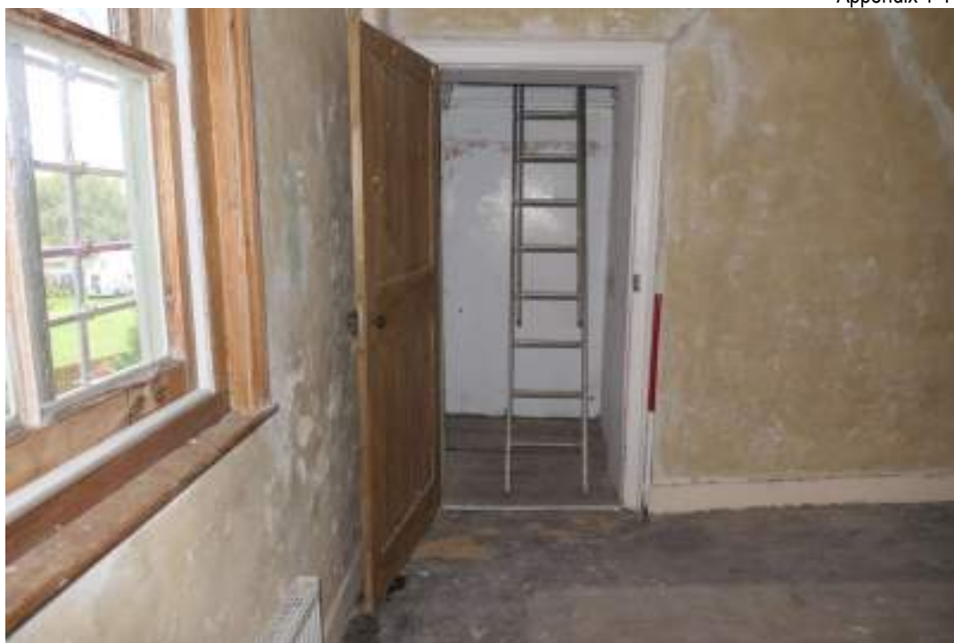
EEX62136_Photograph_189 Detail of door to loft access in bedroom 2. Photograph taken facing south-west.
