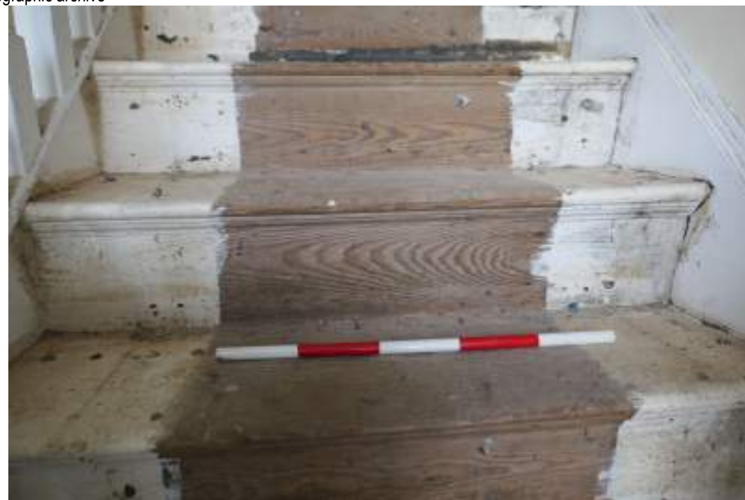
EEX62136_PhotoGraph_114 Detail of stairs in entrance hall. Photograph taken facing north-west.
