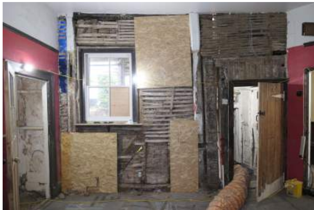
EEX62136_Photograph_107 Detail of exposed timber-framing in south-eastern wall of office. Photograph taken facing south-east.
