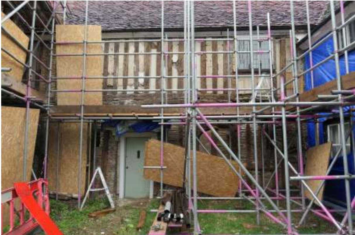
Photograph 6 South-eastern elevation (range 5). Photograph taken facing north-west.
