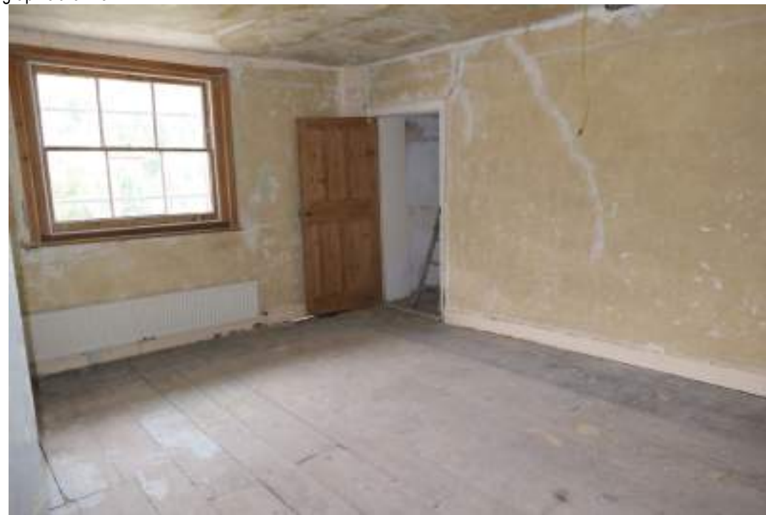
EEX62136_Photograph_182 Interior of bedroom 2. Photograph taken facing south.
