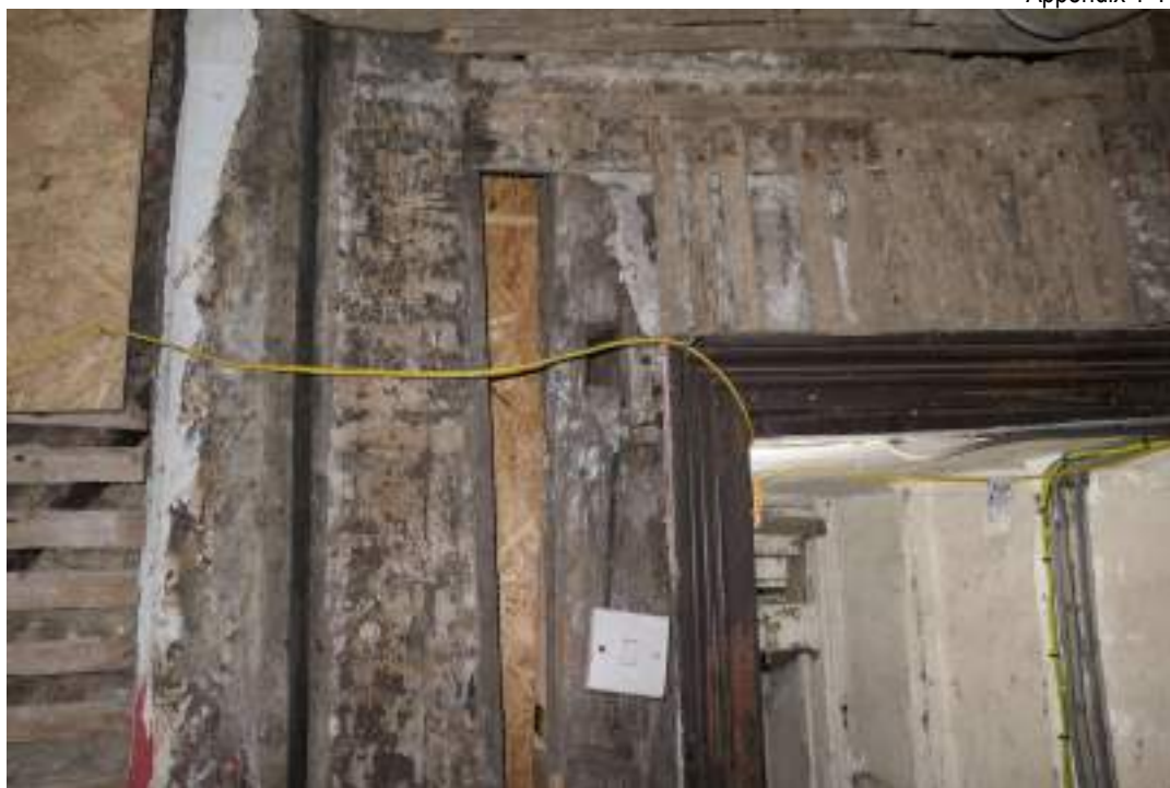
EEX62136_Photograph_109 Detail of empty mortice on post in south-eastern wall of office. Photograph taken facing south-east.
