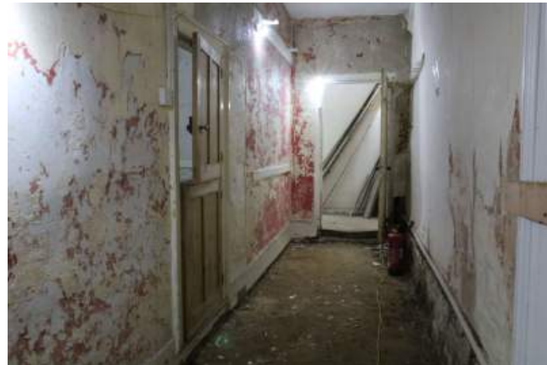
EEX62136_Photograph_072 Interior of corridor 2. Photograph taken facing north-east.
