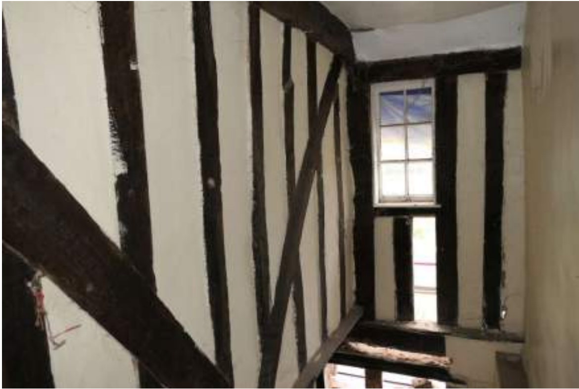
Photograph 46 Interior of rear stairs. Photograph taken facing west north-west.
