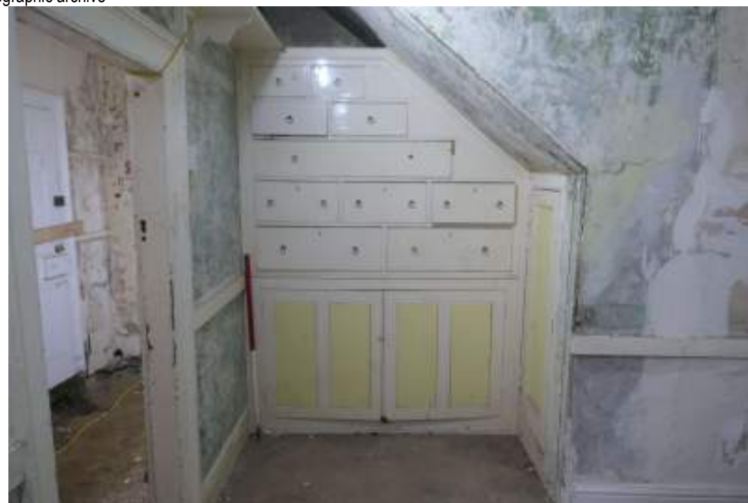
EEX62136_Photograph_082 Detail of in-built storage in spare room 2. Photograph taken facing south-west.
