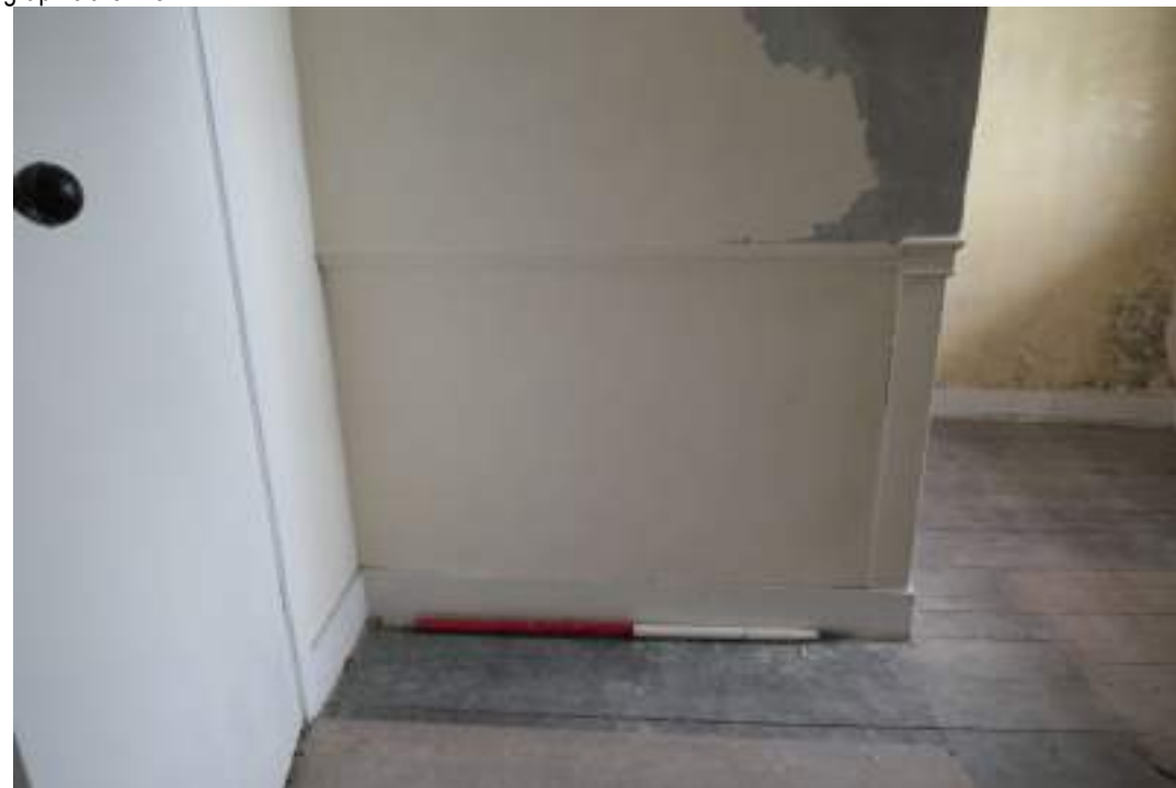
EEX62136_Photograph_194 Detail of stair balustrade incorporated in to wall in bedroom 3. Photograph taken facing north-east.
