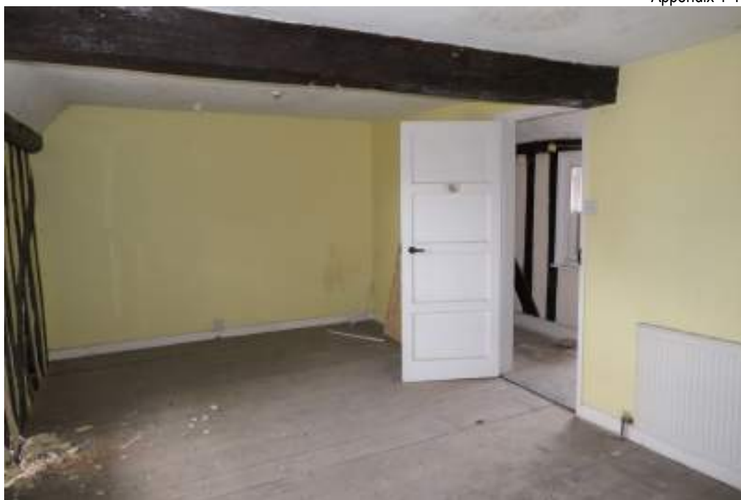
EEX62136_Photograph_229 Interior of bedroom 4. Photograph taken facing east.
