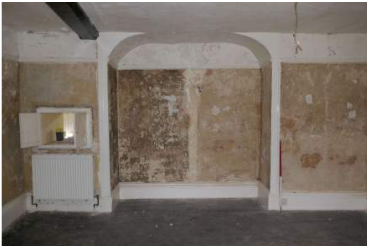
Photograph 28 Detail of arch in north-western wall in living room. Photograph taken facing north-west.
