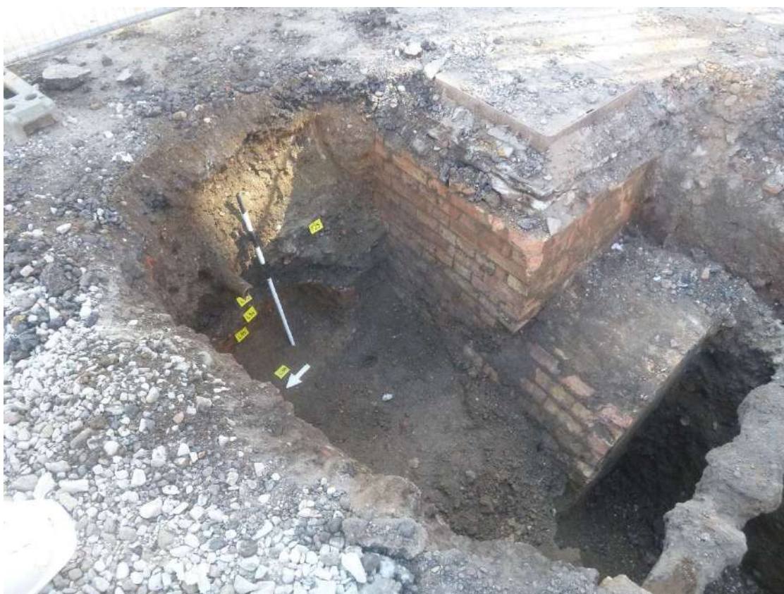
Photograph 24 Deep services associated with brick manhole/drain, looking south-east.
