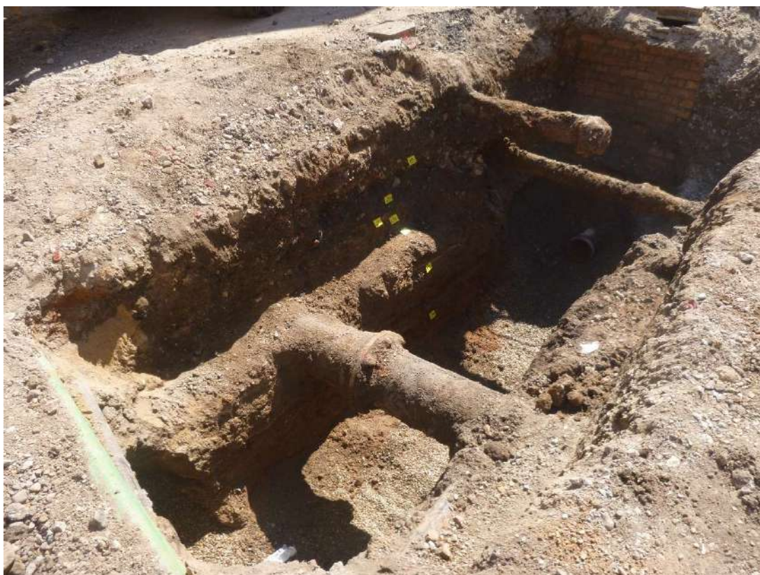
Photograph 25 Deep service trench to south of gully pit 6, looking south-south-east.
