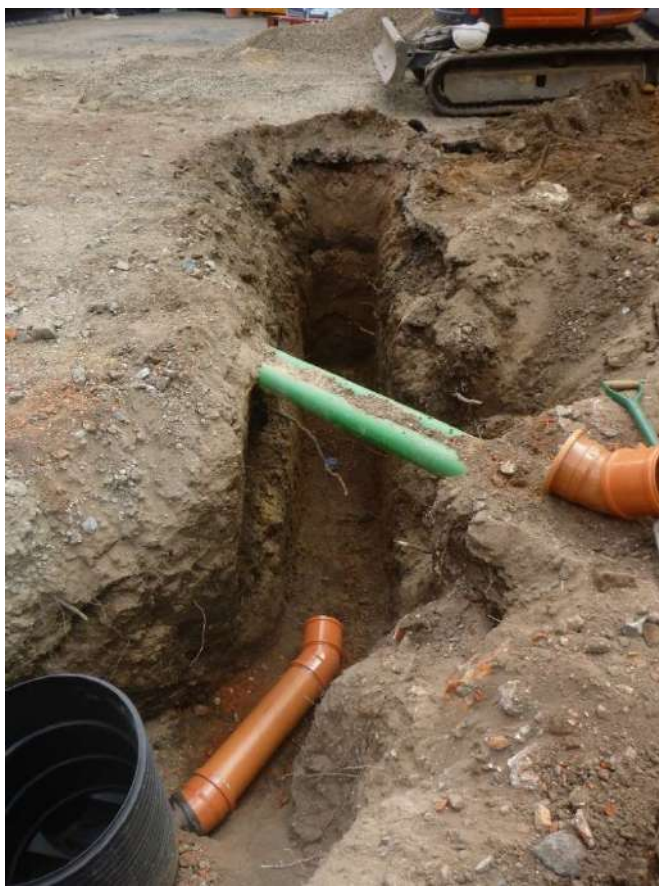
Photograph 10 Example of a deep service trench, looking south-east.
