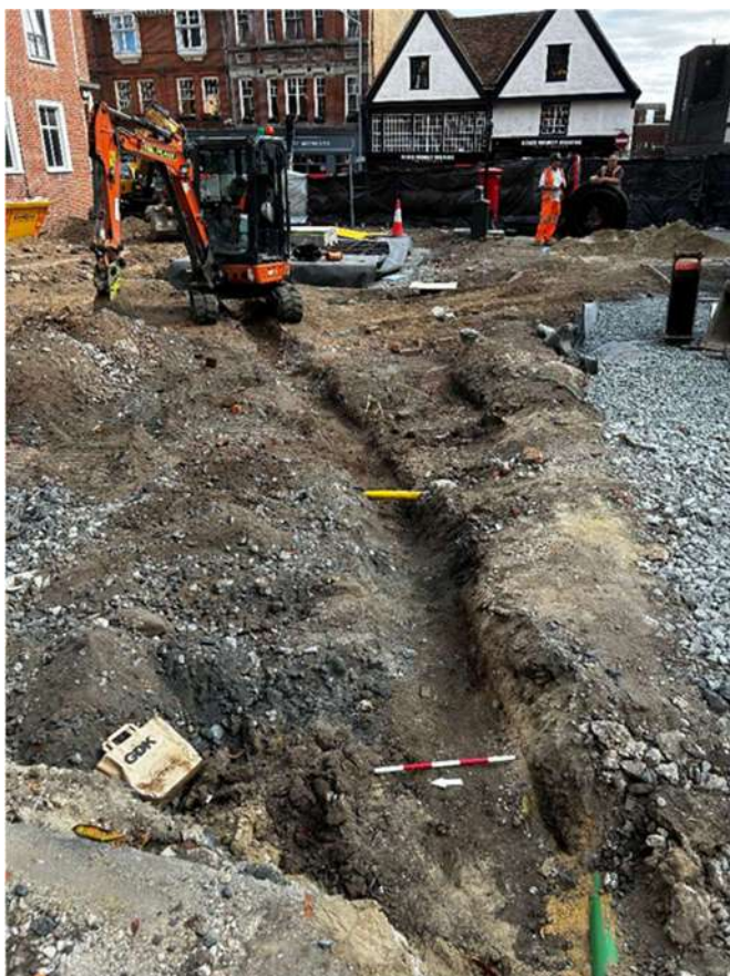
Photograph 11 Example of a shallow service trench, looking north-east.
