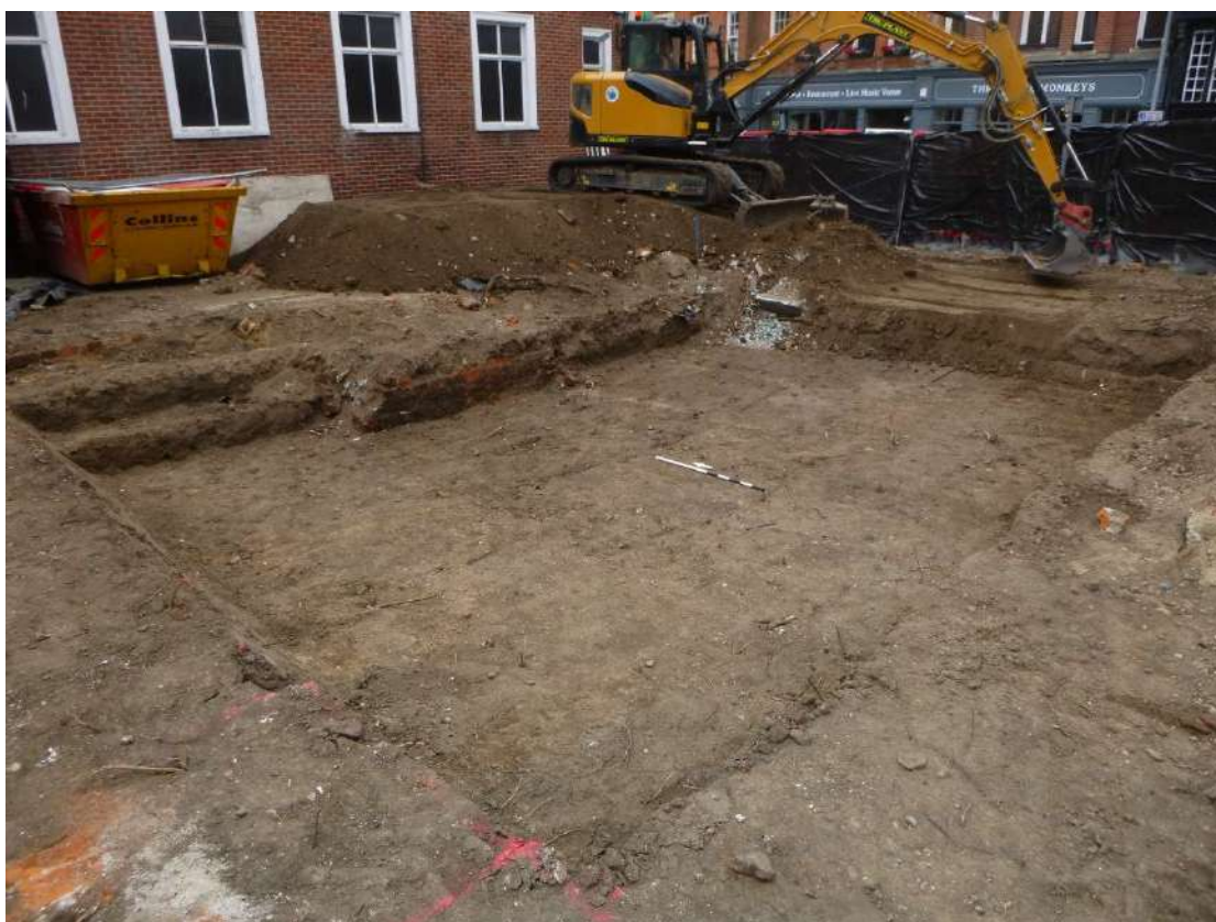
Photograph 8 Tree-pit 1, looking north-east.
