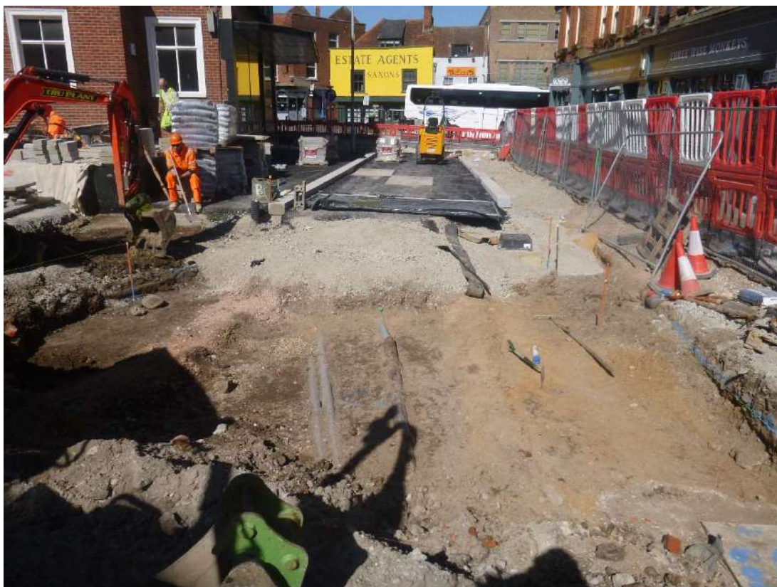
Photograph 22 Ground reduction on the corner of Culver Street East and St Nicholas Street, looking north.
