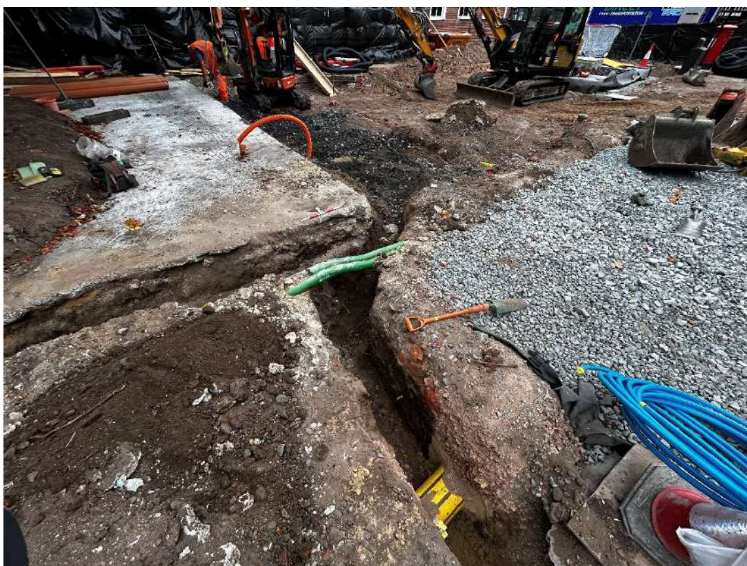
Photograph 9 Service trench, looking north-west.
