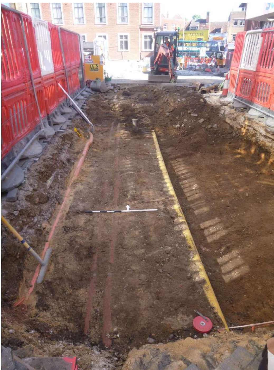
Photograph 27 Long Wyre Street reduction, looking north.
