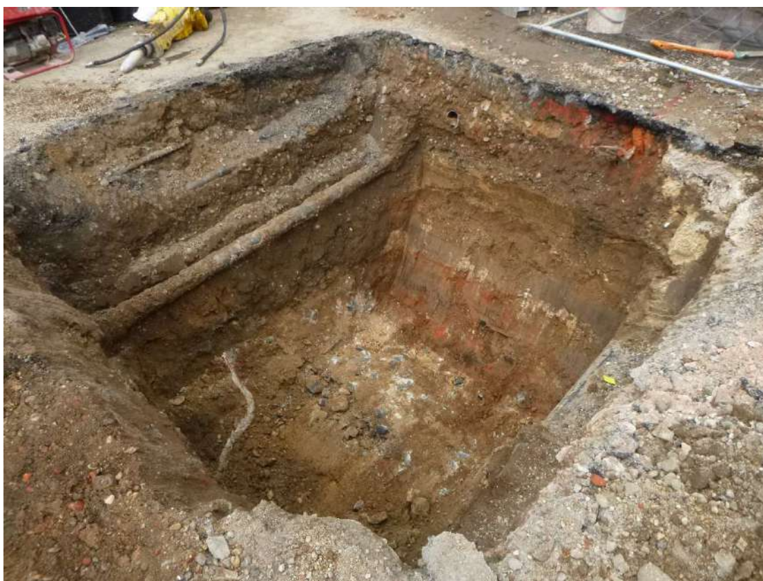
Photograph 14 Photograph showing the partial removal of wall foundation F47 in the base inspection chamber, looking west.
