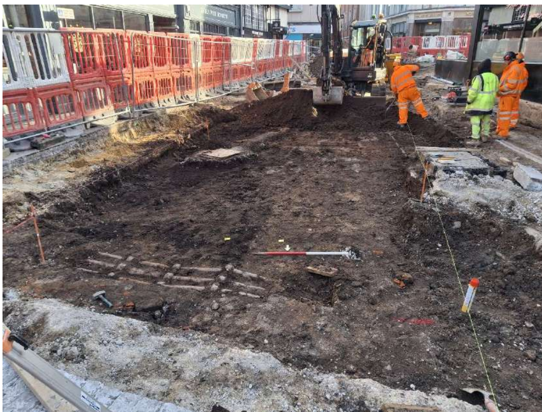
Photograph 20 St Nicholas Street ground reduction, at north end looking south.
