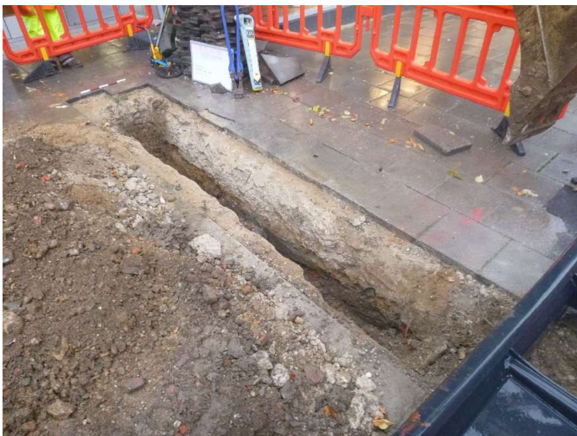
Photograph 1 Trial-hole 2, looking west.
