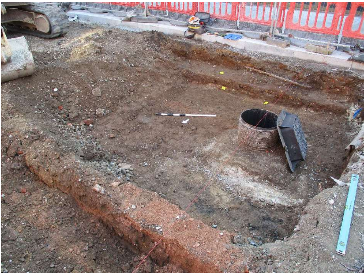
Photograph 21 Ground reduction along Culver Street East, looking south-south-east.
