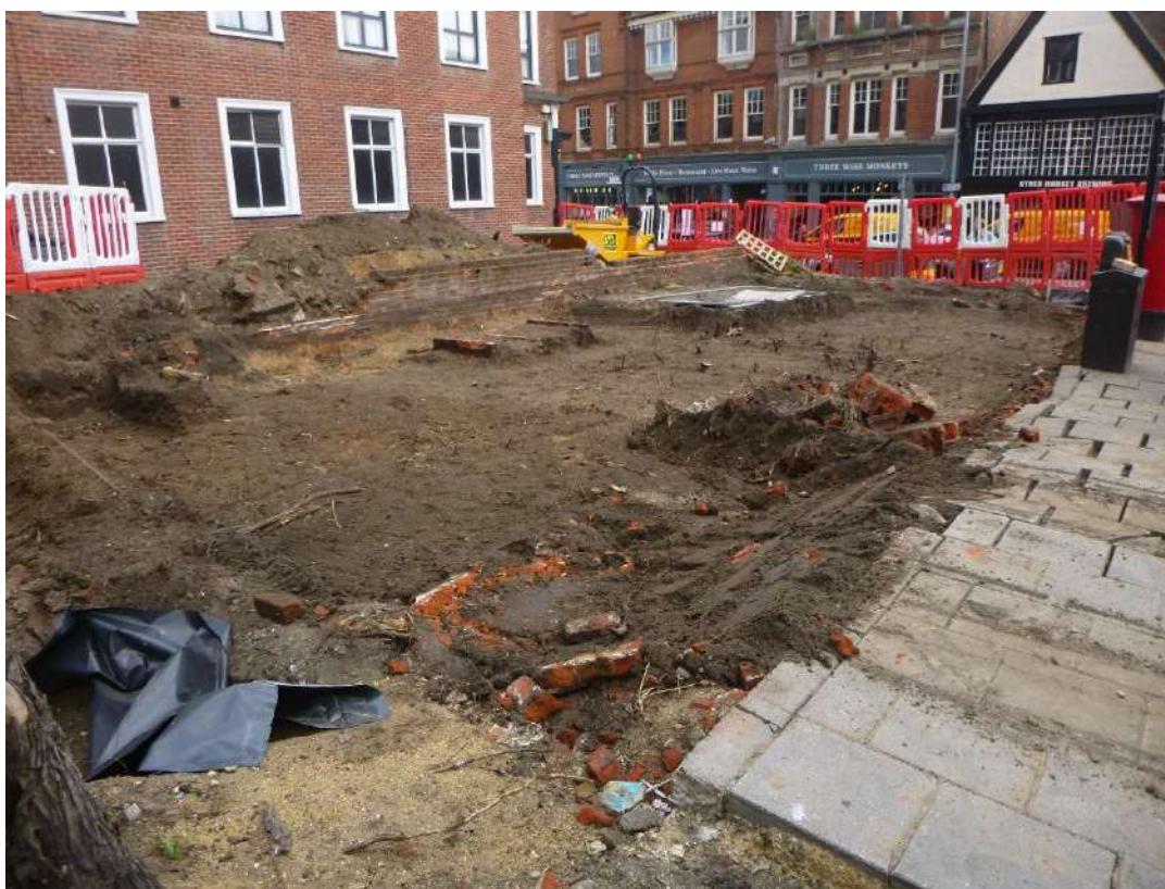
Photograph 3 Ground reduction area showing the remains of burial chambers F2 and F3 in foreground and F13/F14 in background, looking north-east.
