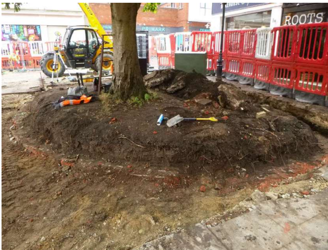
Photograph 4 Ground reduction around the tree, looking south.
