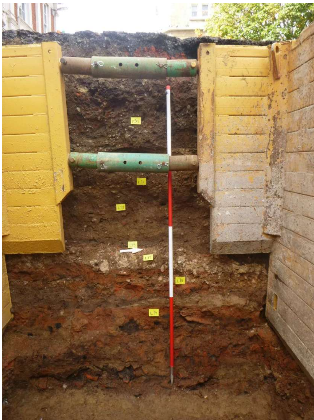
Photograph 15 Eastern section of the inspection chamber – F25, L11, L13, L15, L17, L18, L19 – looking west.
