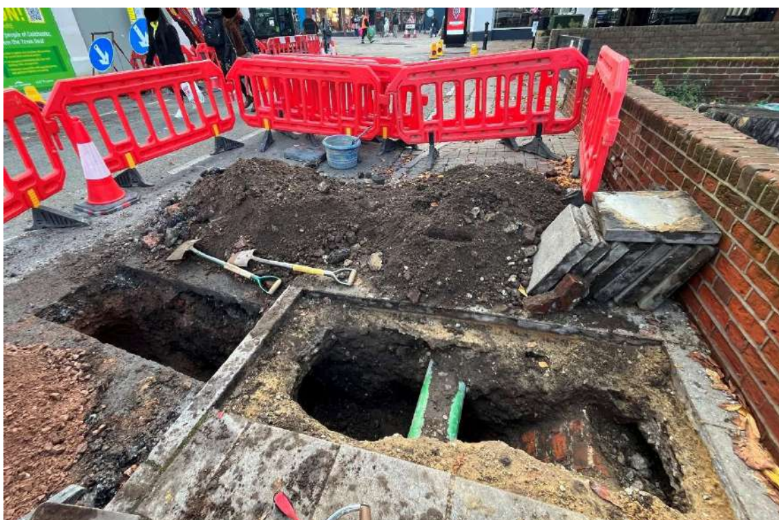
Photograph 2 Trial-hole 7 with the probable vaulted brick burial chamber visible to the bottom right, looking west.
