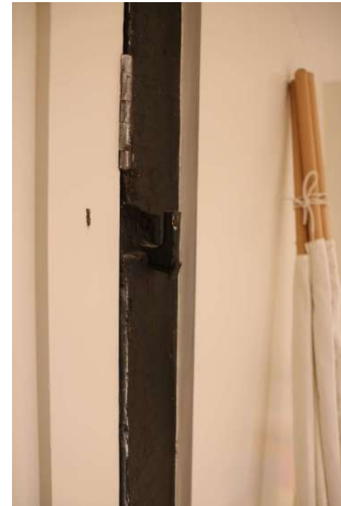
2025.12g_Photograph_164 Detail of pintle in door frame in south-eastern wall of bedroom 6. Photograph taken facing south.
