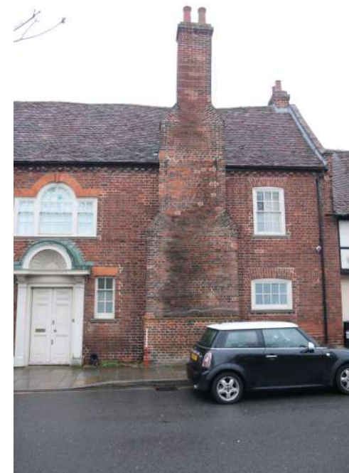
2025.12g_Photograph_256 Detail of south-eastern chimney breast on south-western elevation (range 1). Photograph taken facing north-east.
