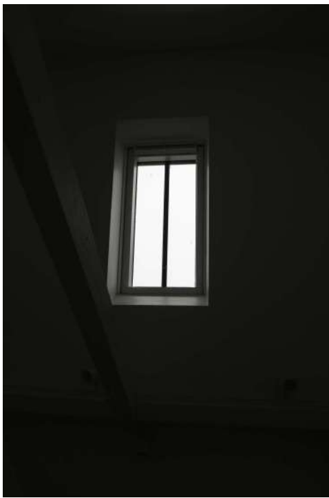
2025.12g_Photograph_185 Example of roof window in studio. Photograph taken facing south-east.
