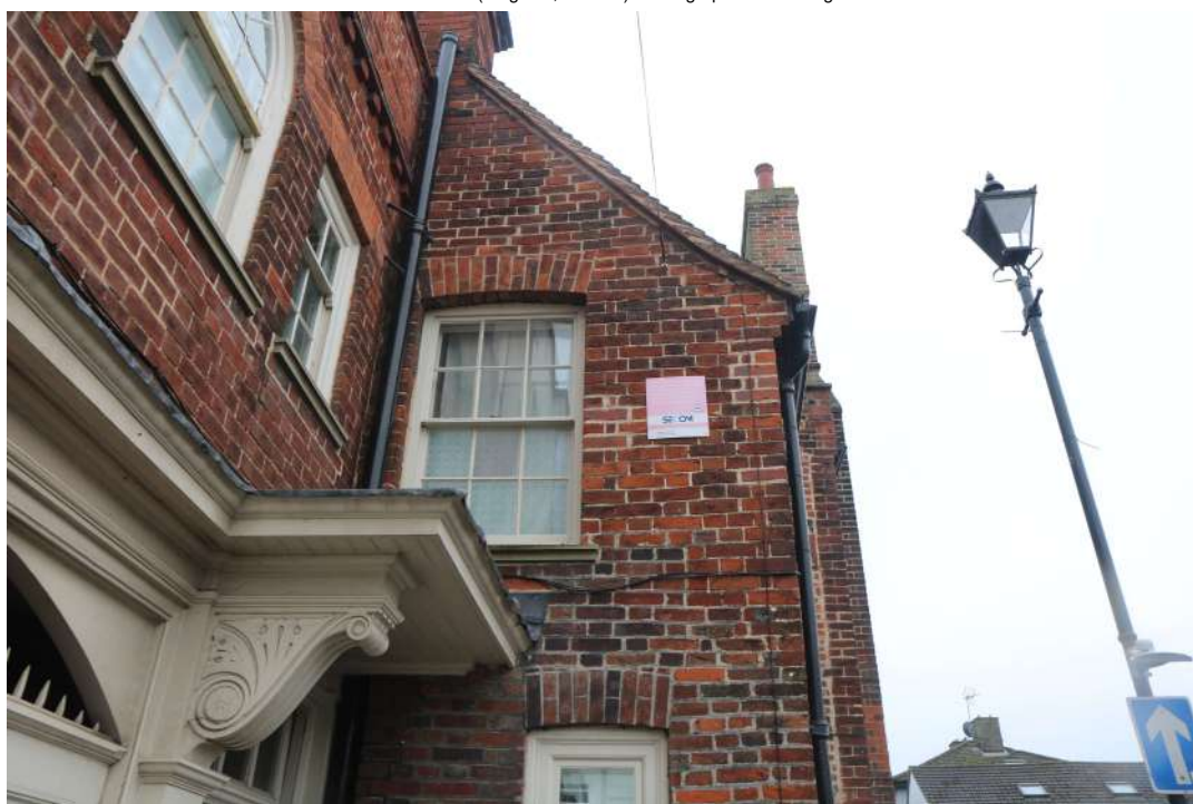
2025.12g_Photograph_239 Detail of window on north-western elevation, first floor (range 2). Photograph taken facing south-east.
