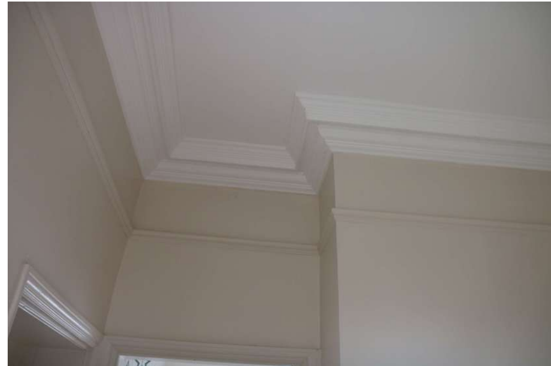
2025.12g_Photograph_092 Detail of picture rail and cornicing in landing 2. Photograph taken facing south-west.
