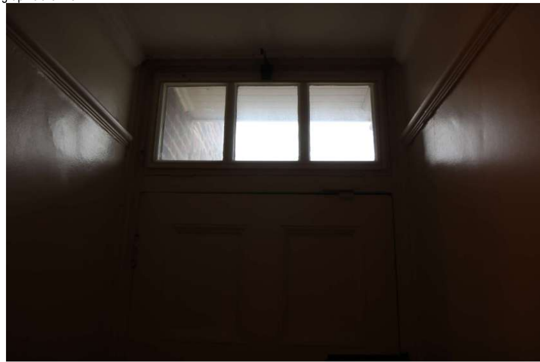
2025.12g_Photograph_054 Detail of fanlight in south-western wall of entrance hall 2. Photograph taken facing south-west.
