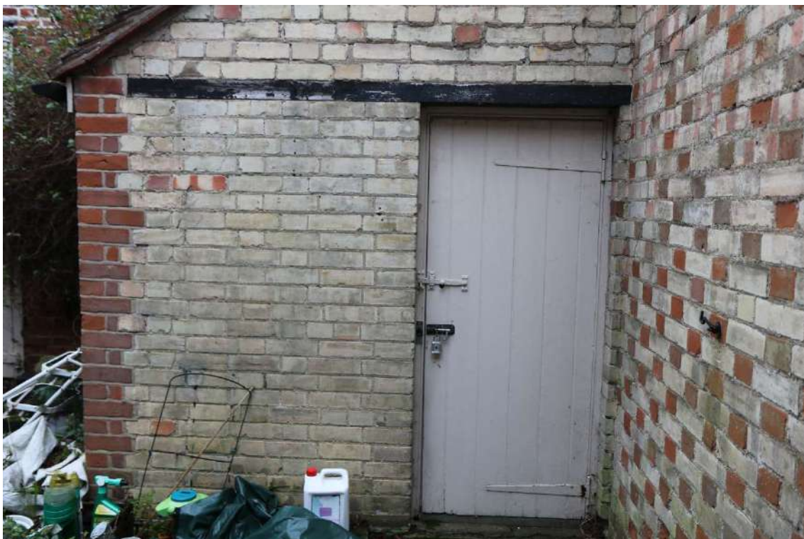
Photograph 45 South-western elevation of storage shed. Checkerboard brickwork visible to the right. Photograph taken facing north-east.
