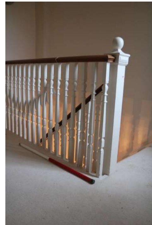
2025.12g_Photograph_120 Detail of balustrade and newel post of staircase 2. Photograph taken facing north.
