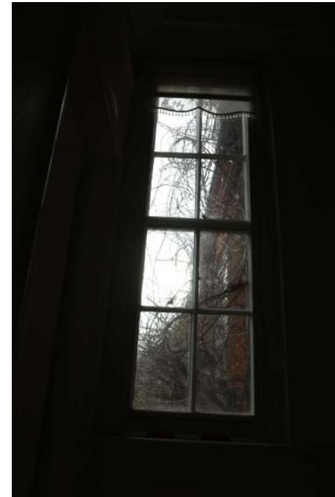
2025.12g_PhotoGraph_088 Detail of window in south-eastern wall of landing 2. Photograph taken facing south-east.
