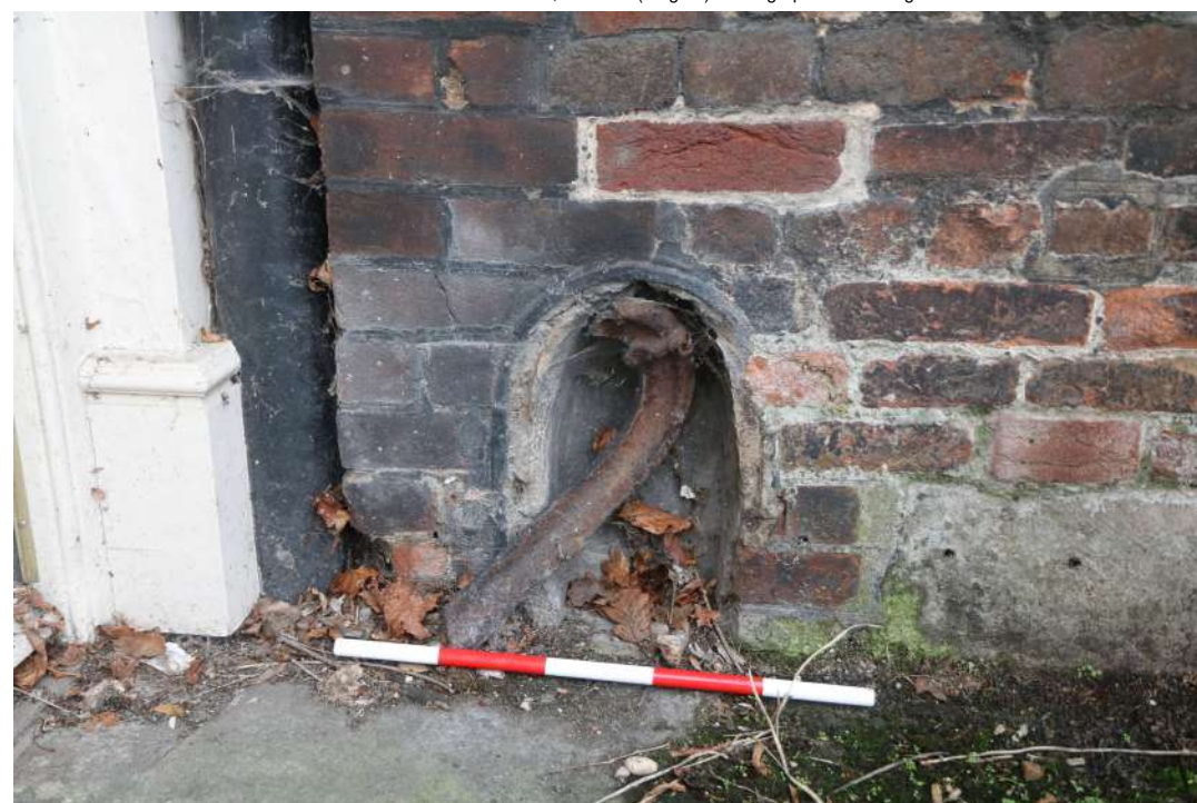
2025.12g_Photograph_240 Detail of boot scraper in north-western elevation (range 2). Photograph taken facing south-east.
