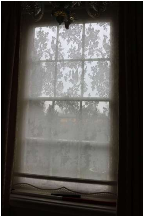
2025.12g_Photograph_139 Detail of window in north-eastern wall of landing 1. Photograph taken facing north north-east.
