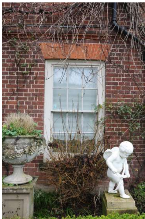
2025.12g_Photograph_207 Detail of window in south-eastern elevation, ground floor (range 3). Photograph taken facing north-west.
