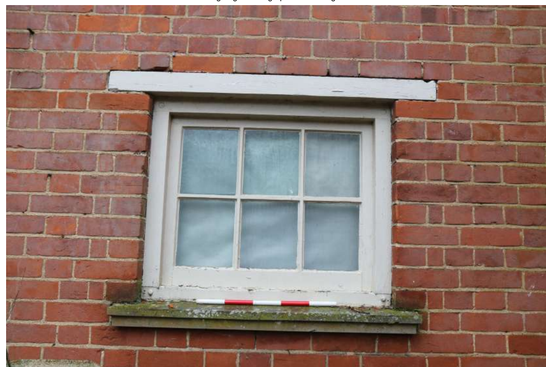
2025.12g_PhotoGraph_196 Detail of window in north-eastern elevation of studio (range 4). Photograph taken facing south-west.
