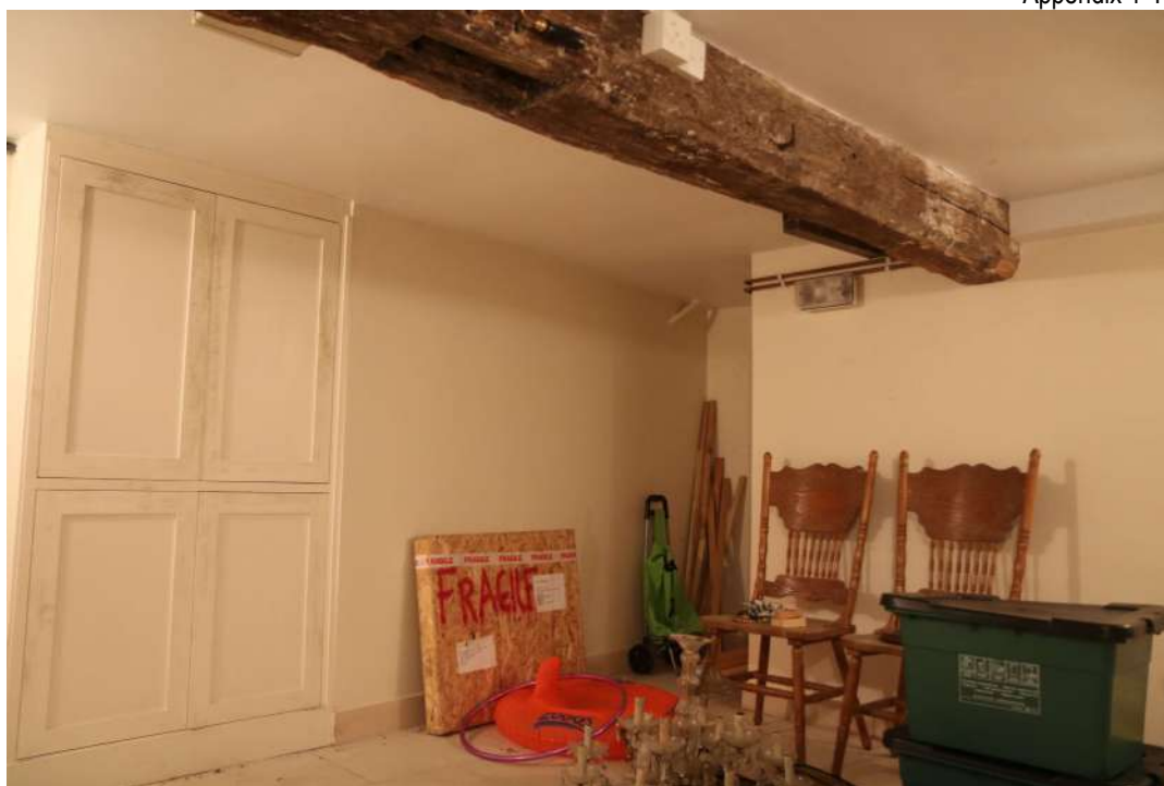
2025.12g_PhotoGraph_173 Interior of basement. Photograph taken facing south.
