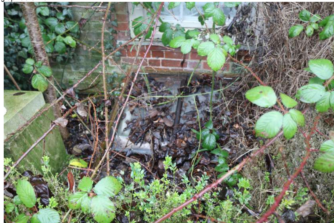
2025.12g_Photograph_226 Detail of basement window, north-eastern elevation (range 1). Photograph taken facing south south-west.
