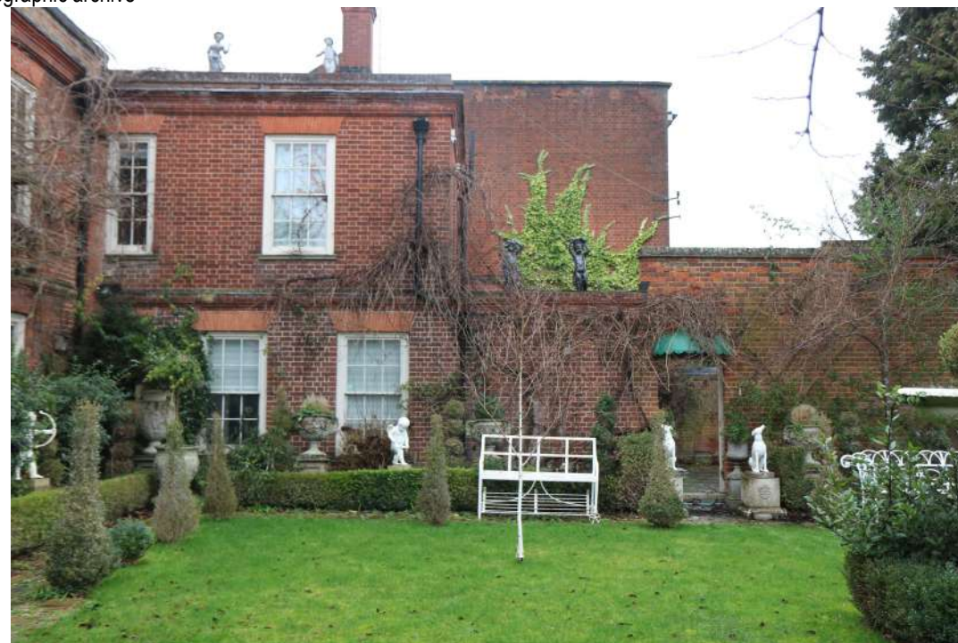
2025.12g_Photograph_206 South-eastern elevation (ranges 3 and 4). Photograph taken facing north-west.
