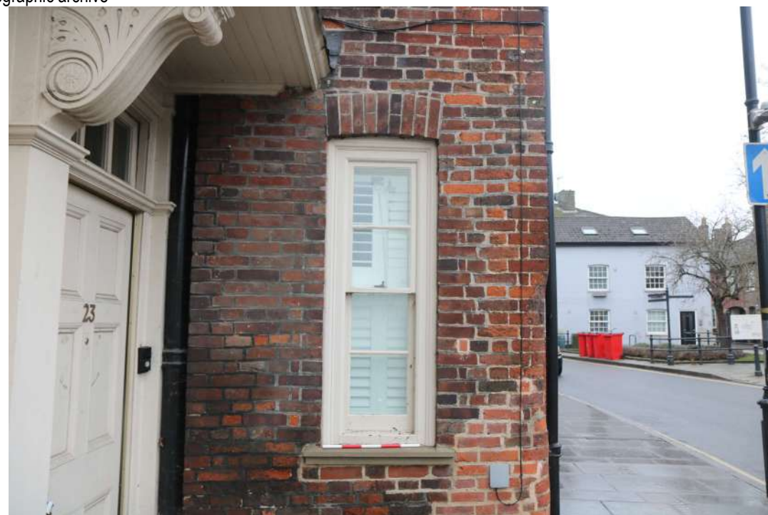
2025.12g_Photograph_238 Detail of window in north-western elevation, first floor (range 2). Photograph taken facing south-east.
