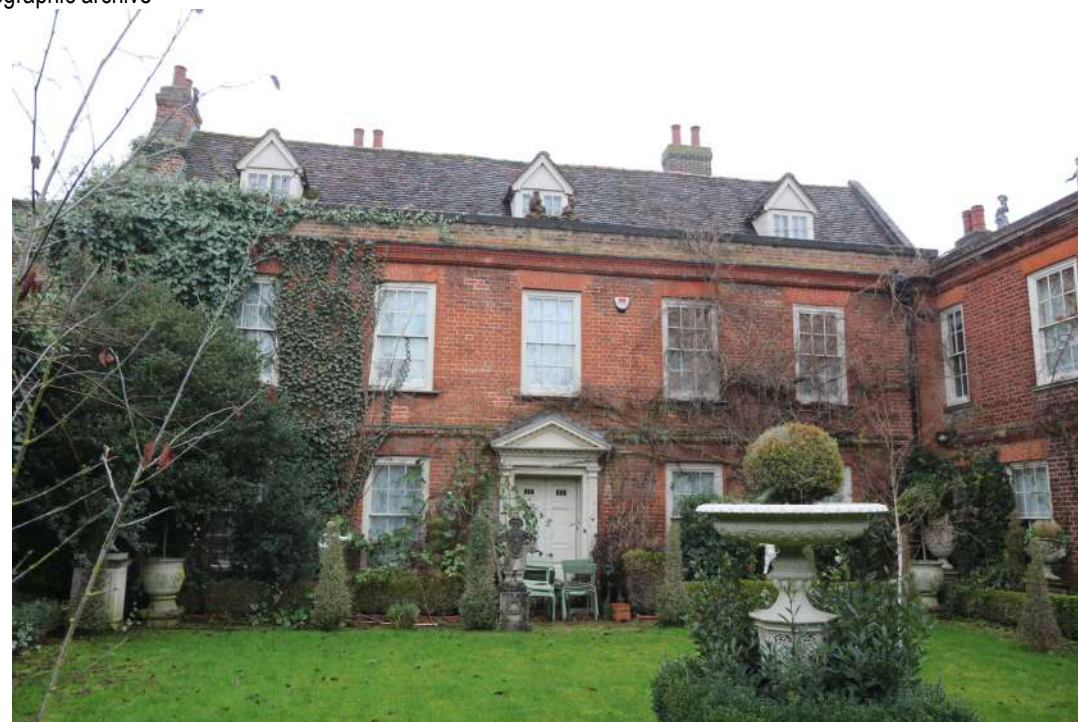
2025.12g_Photograph_214 North-eastern elevation (range 1). Photograph taken facing west south-west.
