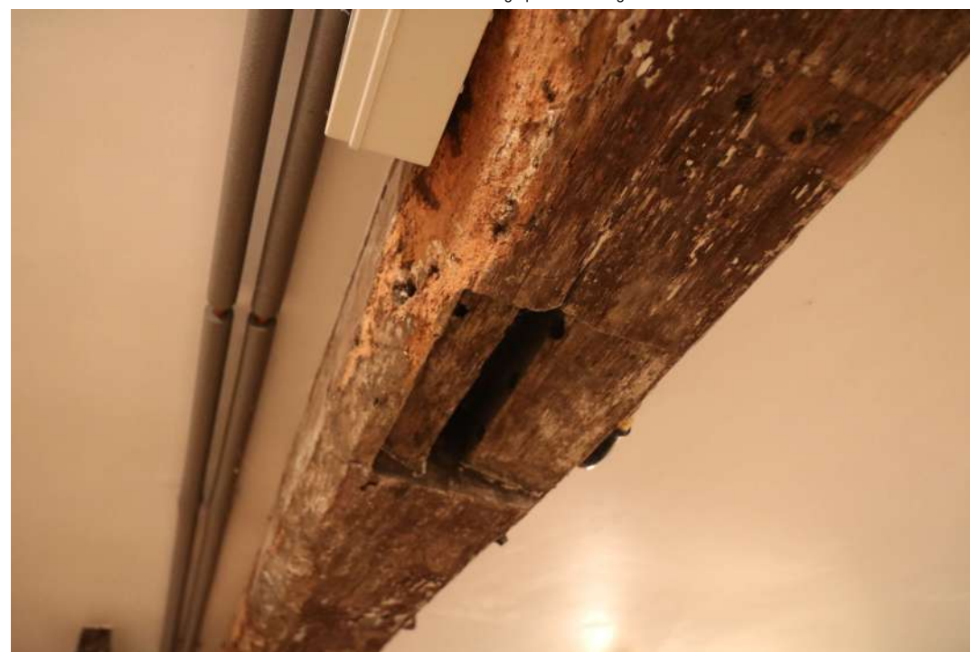
2025.12g_PhotoGraph_176 Detail of empty mortice on binding beam in basement ceiling. Photograph taken facing south-west.
