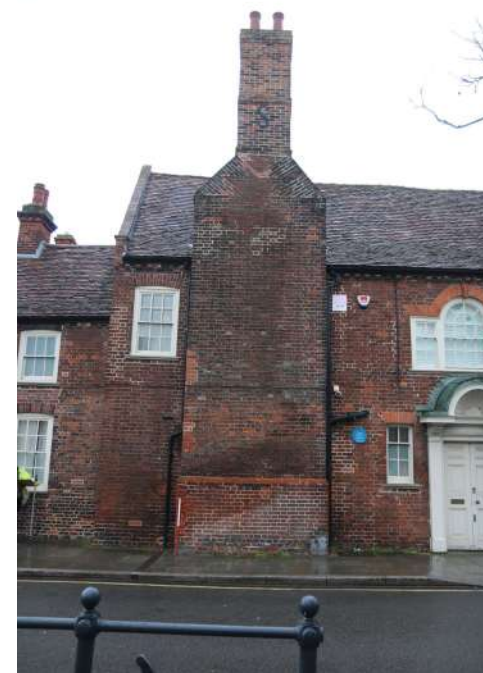
2025.12g_Photograph_252 Detail of north-western chimney breast on south-western elevation (range 1). Photograph taken facing north-east.
