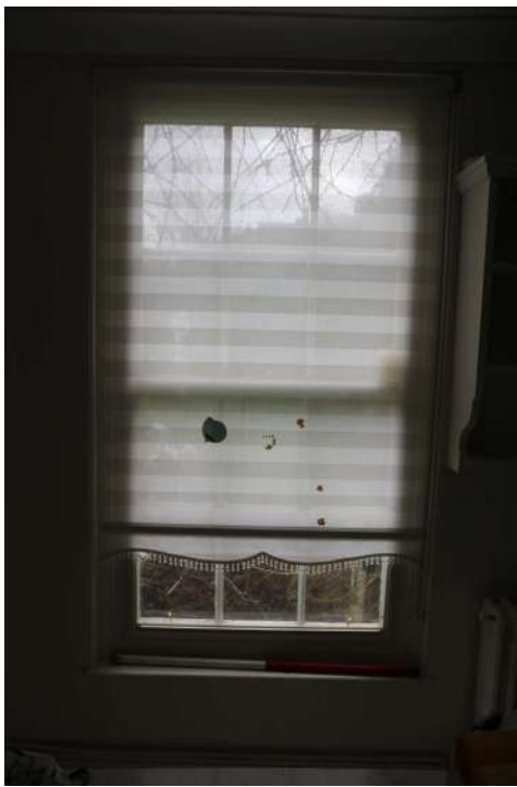
2025.12g_Photograph_073 Detail of window in south-eastern wall of kitchen. Photograph taken facing south-east.
