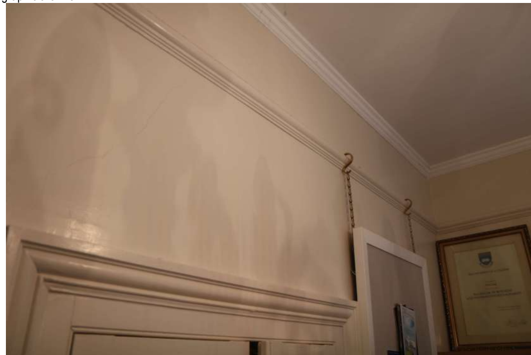
2025.12g_Photograph_066 Detail of picture rail in study. Photograph taken facing south.
