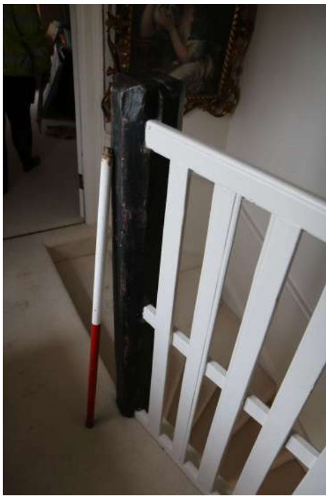
2025.12g_Photograph_157 Detail of hand-carved newel post in staircase 1 (second floor). Photograph taken facing south.
