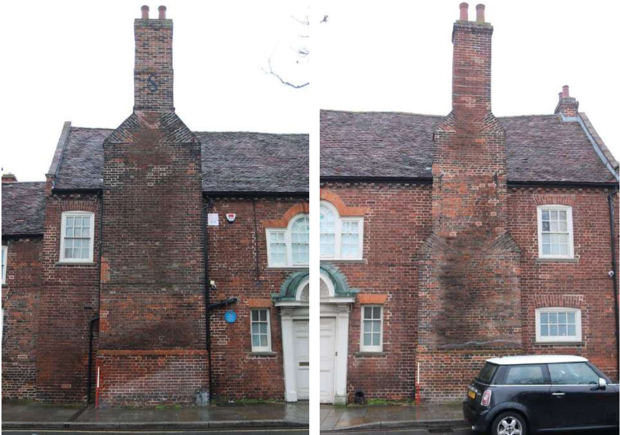
Photographs 6 & 7 Detail of chimney breasts on south-western elevation of range 1. Photograph taken facing north-east.
