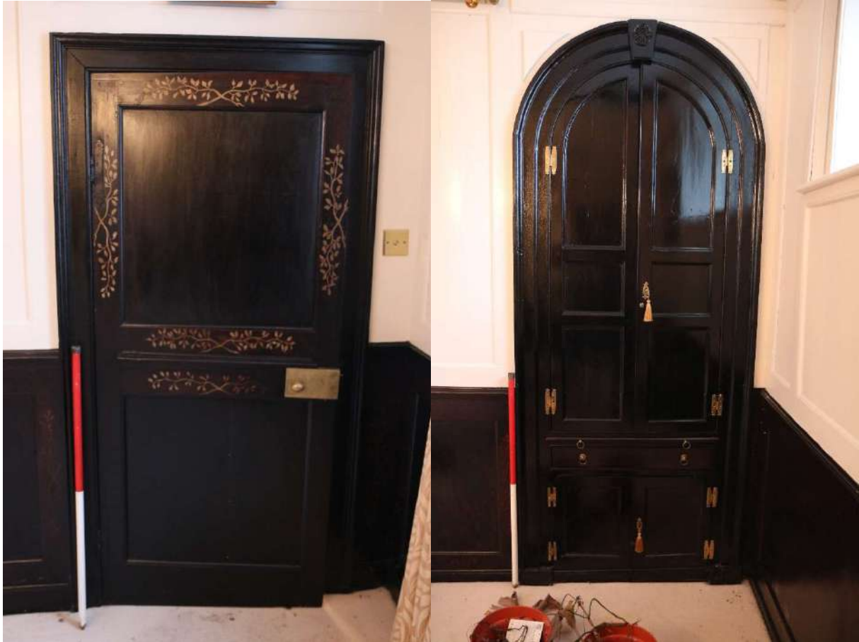
Photograph 17 Detail of door in north-western wall of drawing room. Photograph taken facing north-west.
