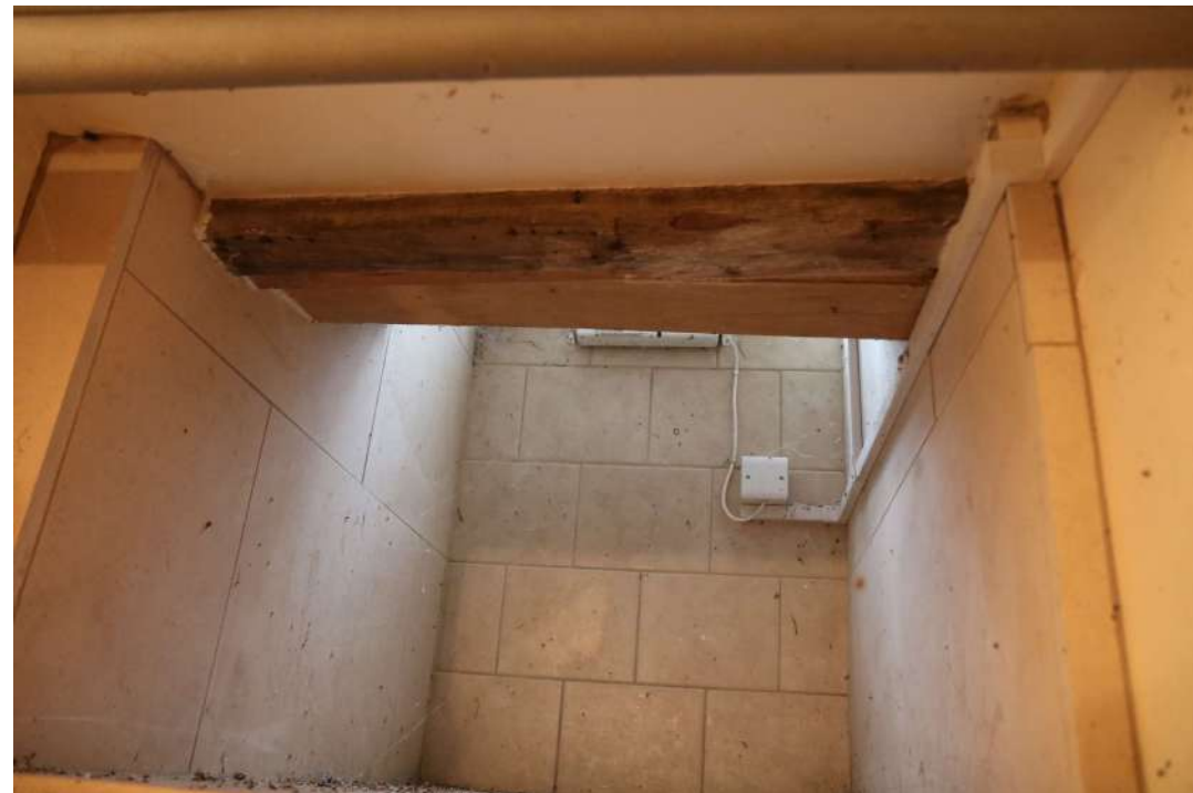
2025.12g_PhotoGraph_180 Detail of opening in north-eastern wall of cellar. Photograph taken facing north-east.
