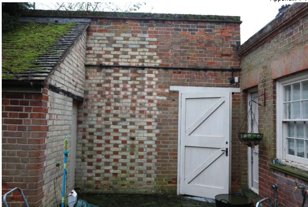
2025.12g_Photograph_205 North-western elevation of the courtyard (range 4). Photograph taken facing south-east.
