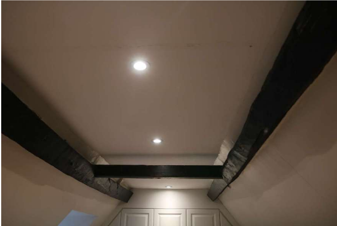
Photograph 40 Detail of exposed purlins in ceiling of bedroom 7. Photograph taken facing south-east.
