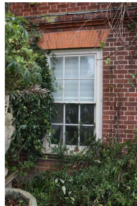
2025.12g_Photograph_208 Detail of window in south-eastern elevation, ground floor (range 3). Photograph taken facing west north-west.
