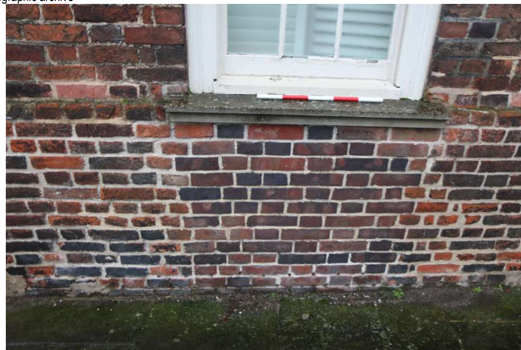
2025.12g_Photograph_250 Detail of change in brickwork in south-western elevation (range 2). Photograph taken facing north-east.
