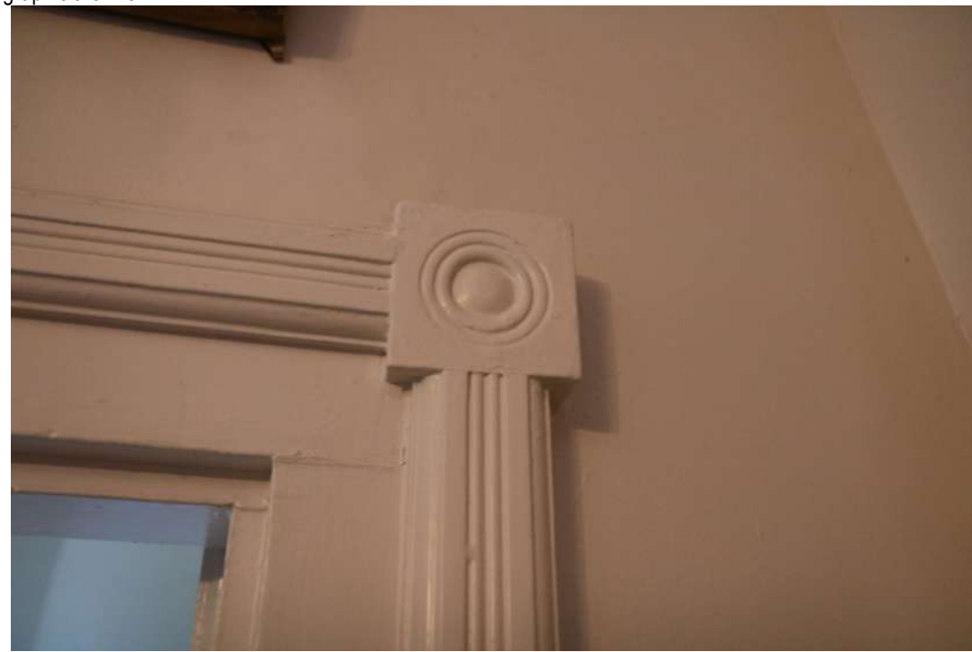
2025.12g_Photograph_126 Detail of decorative doorframe in north-western wall of bedroom 4. Photograph taken facing north-west.
