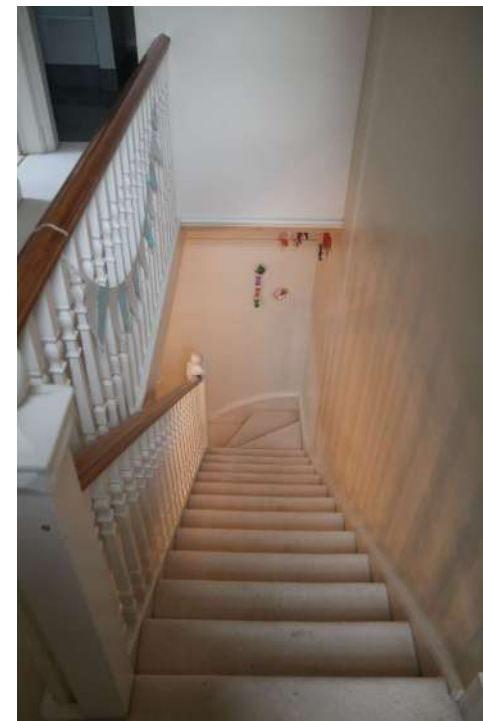
2025.12g_Photograph_082 Detail of staircase 2. Photograph taken facing north-west.
