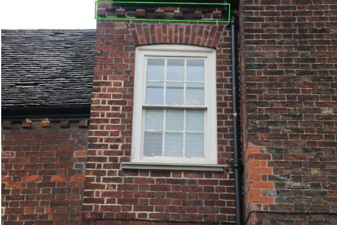
Photograph 8 Detail of window in south-western elevation of range 1, first floor. Dentilled brickwork highlighted in green. Photograph taken facing north-east.
