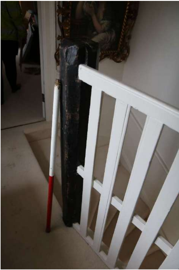
Photograph 39 Detail of hand-carved newel post in staircase 1 (second floor). Photograph taken facing south.
