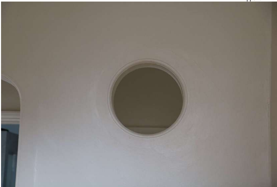
2025.12g_PhotoGraph_085 Detail of circular opening in landing 2 wall. Photograph taken facing north-west.
