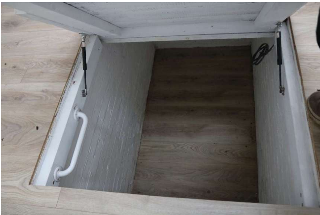
Photograph 47 Pit in floor of studio. Photograph taken facing south-west.
