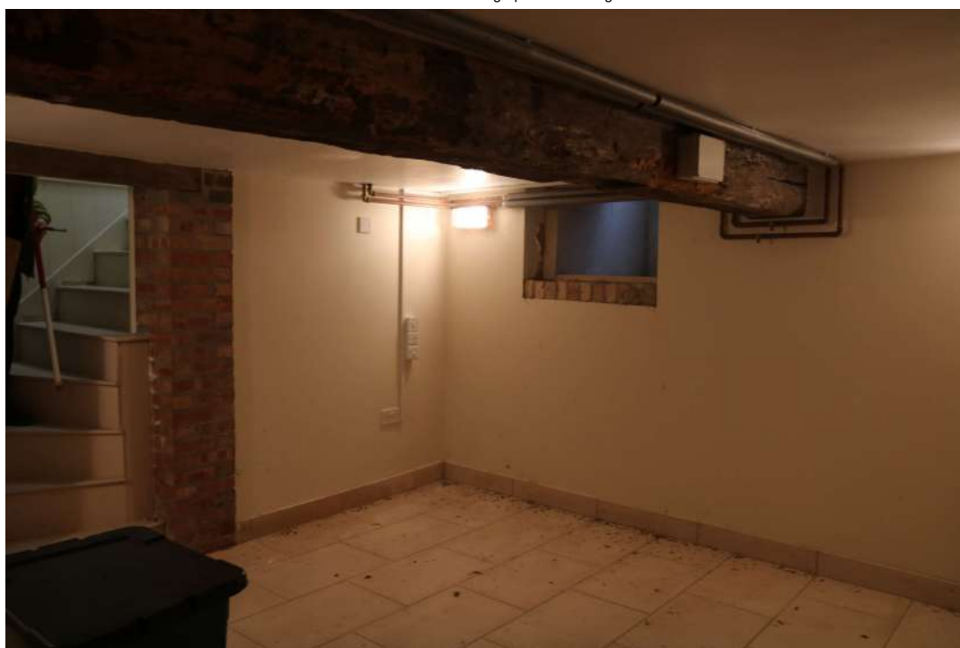
2025.12g_PhotoGraph_175 Interior of basement. Photograph taken facing north.
