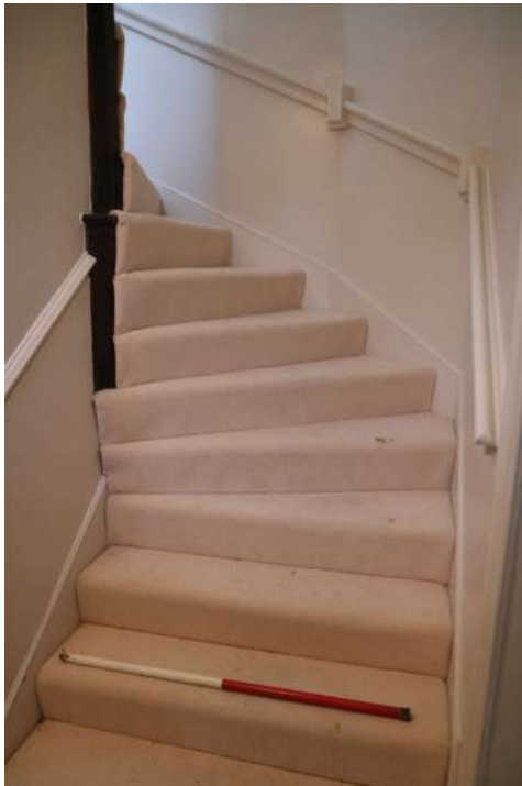
2025.12g_Photograph_031 Detail of staircase 1. Photograph taken facing south-west.
