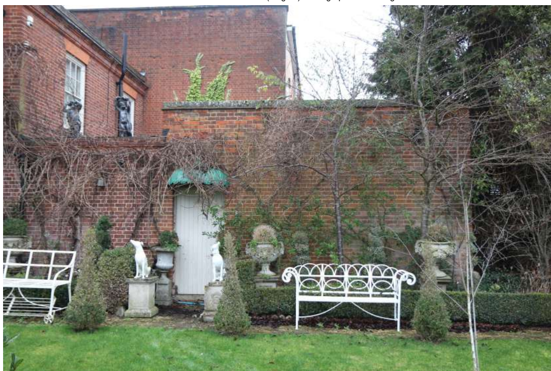
2025.12g_Photograph_199 South-eastern elevation (range 4). Photograph taken facing north-west.
