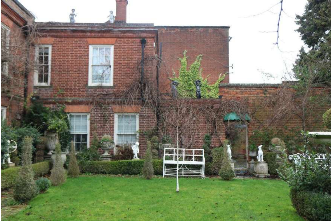
Photograph 4 South-eastern elevation of ranges 3 and 4. Photograph taken facing north-west.
