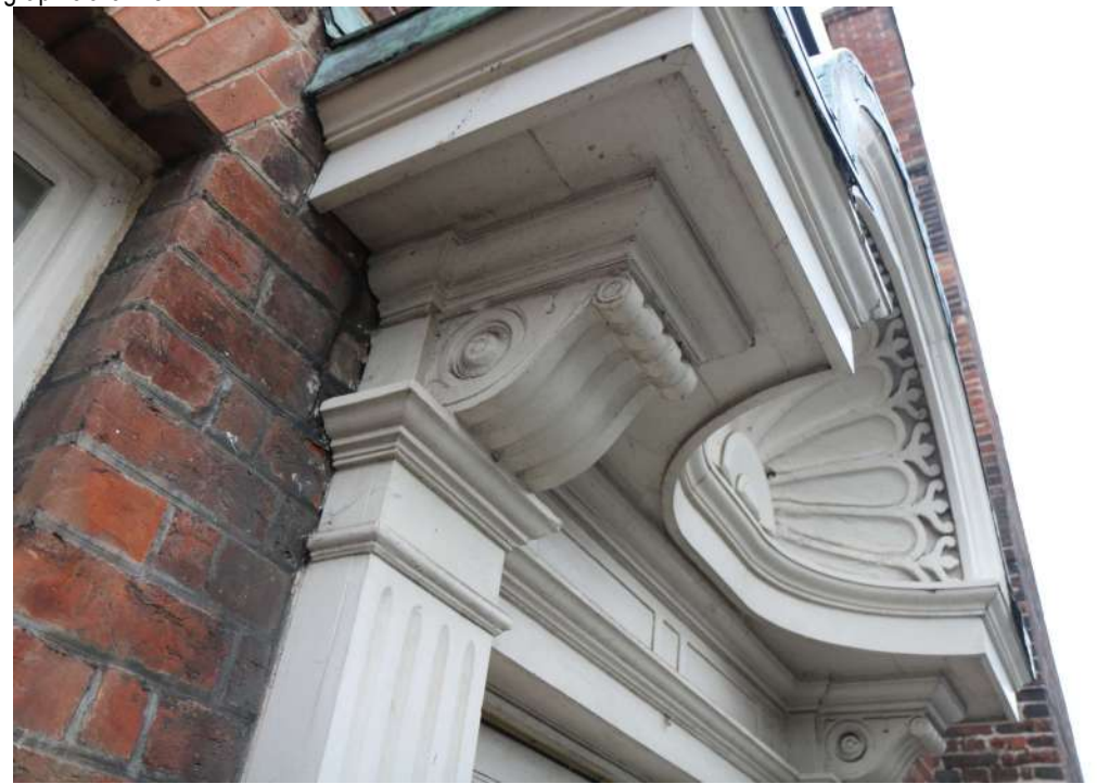
2025.12g_Photograph_254 Decorative detail in door surround, south-western elevation (range 1). Photograph taken facing east.
