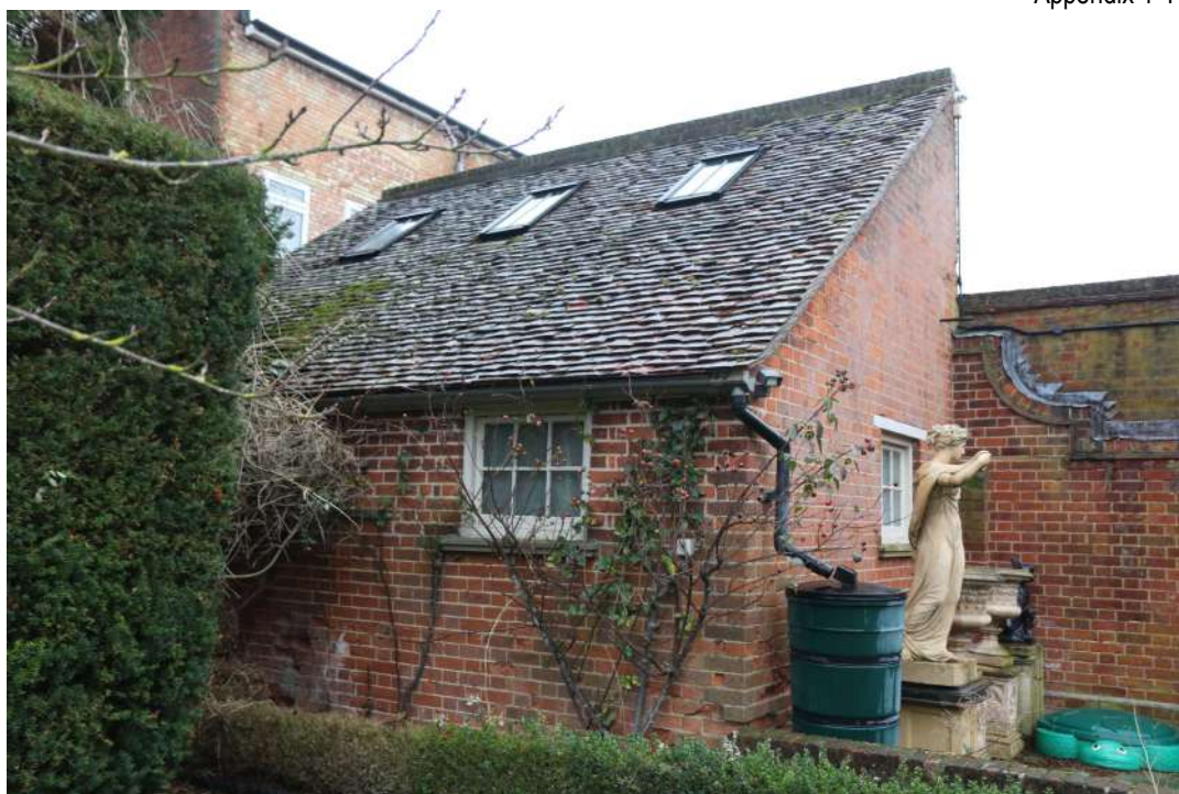
2025.12g_Photograph_197 South-eastern elevation of studio (range 4). Photograph taken facing west.
