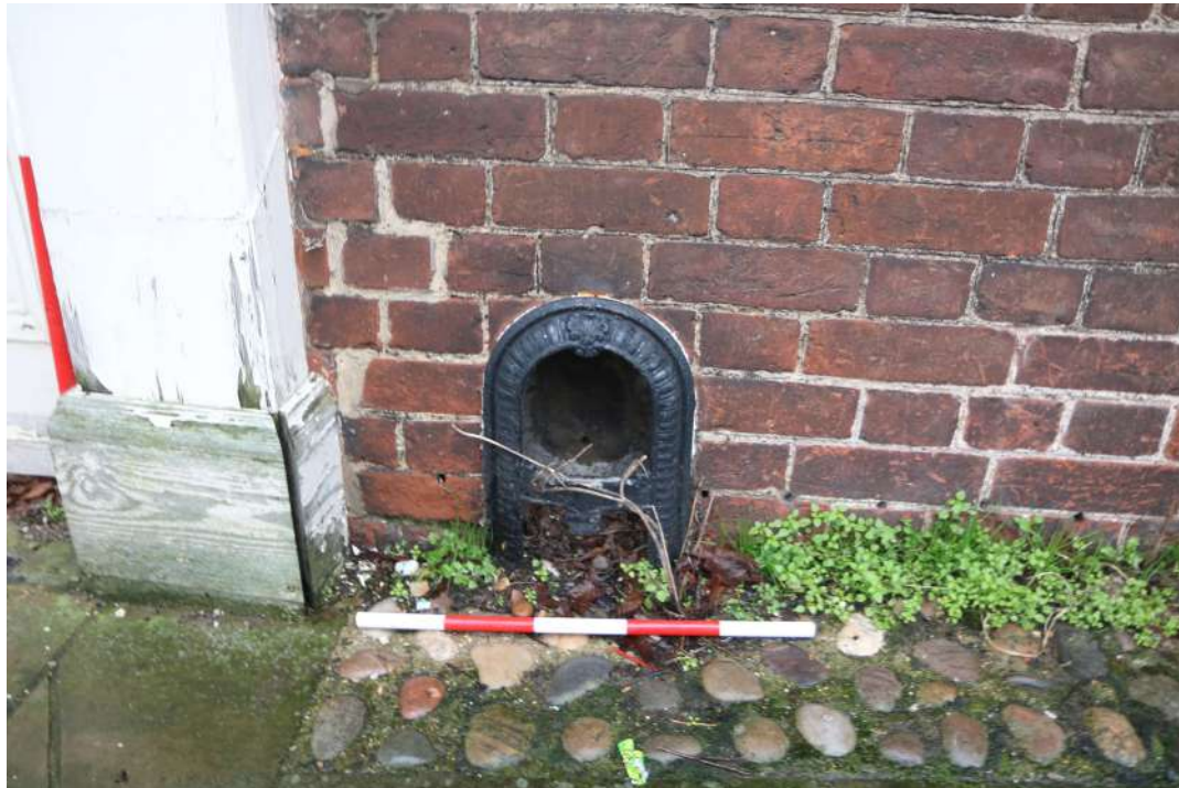
2025.12g_Photograph_255 Detail of boot scraper in south-western elevation (range 1). Photograph taken facing north-east.
