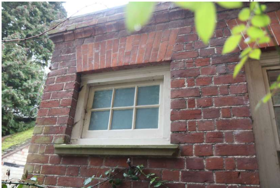
2025.12g_Photograph_233 Detail of window on north-western elevation (range 3). Photograph taken facing south.
