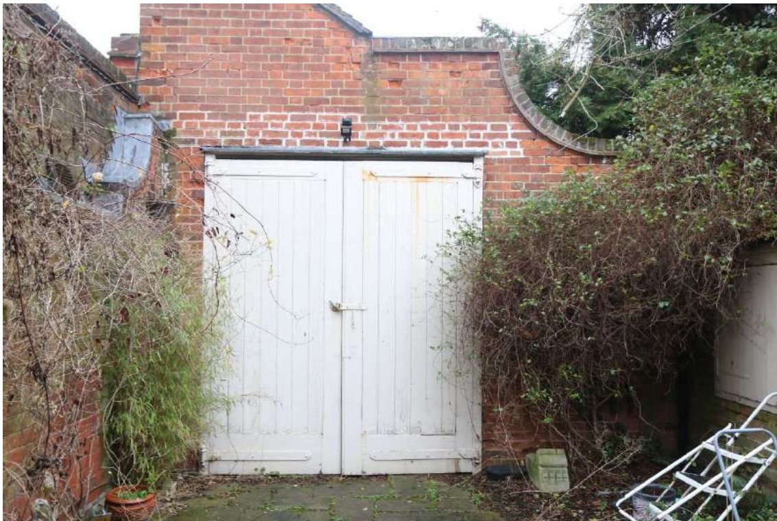
Photograph 43 South-western elevation of studio. Photograph taken facing north-east.
