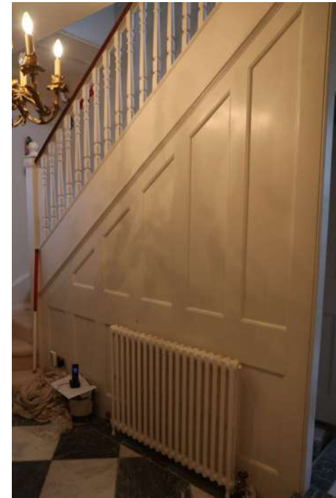
2025.12g_Photograph_056 Detail staircase 2. Photograph taken facing north.
