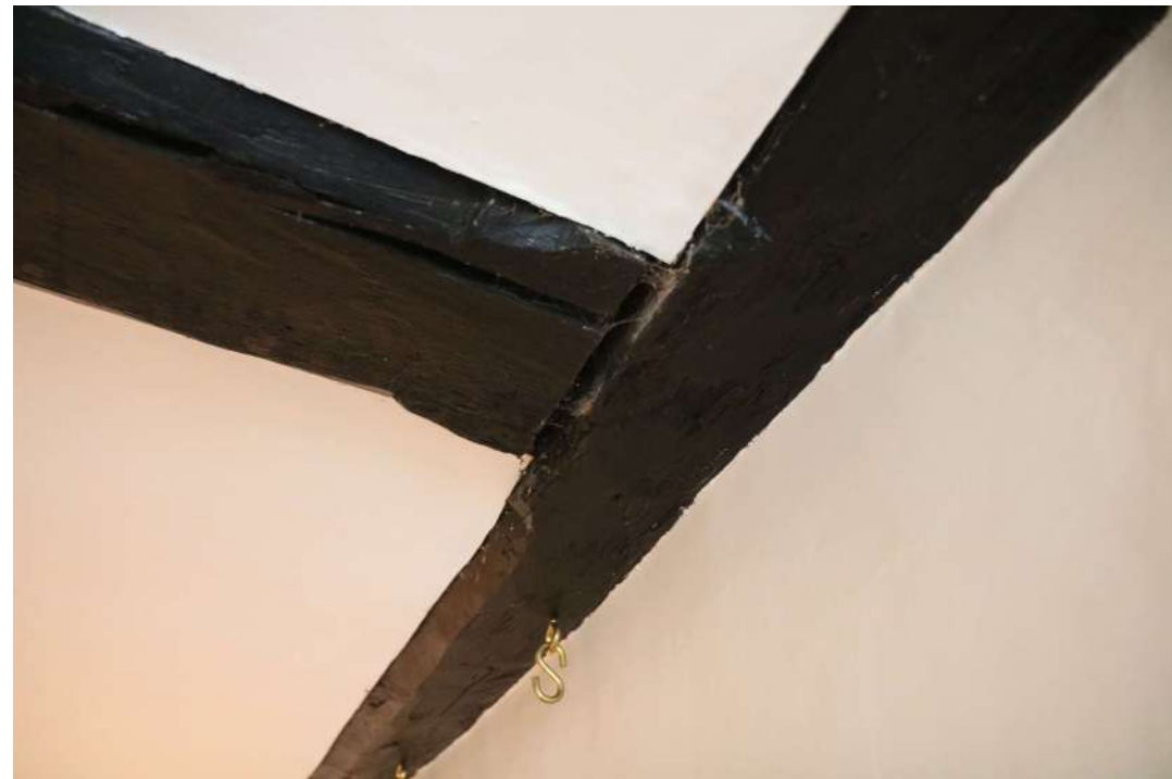
2025.12g_PhotoGraph_028 Detail of carved stops in ceiling of entrance hall 1. Photograph taken facing north.
