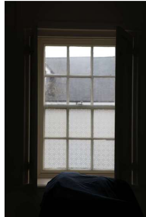
2025.12g_Photograph_148 Detail of window in south-western wall of bedroom 5. Photograph taken facing south-west.
