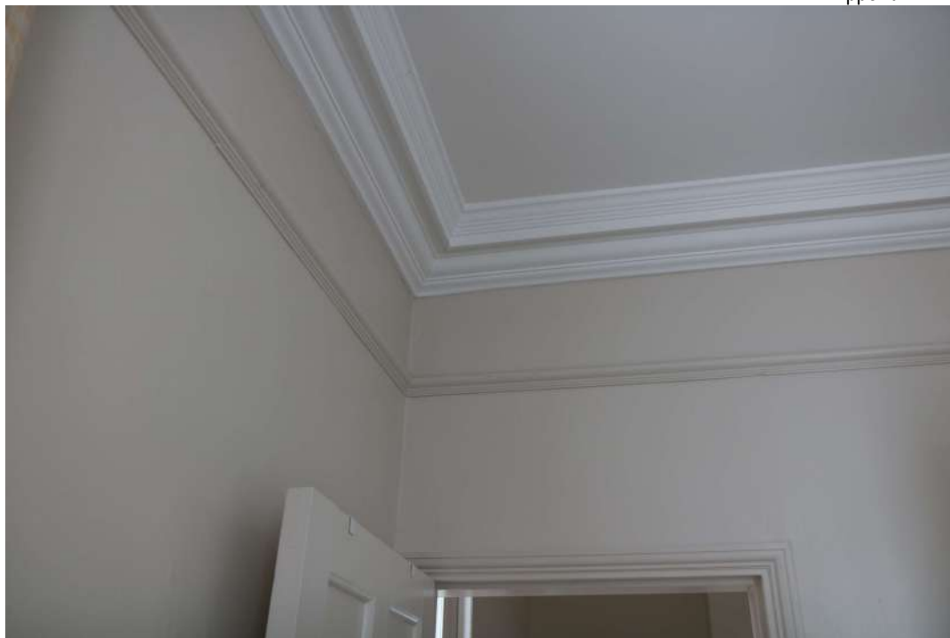
2025.12g_Photograph_109 Detail of picture rail and cornicing in bedroom 2. Photograph taken facing south south-west.
