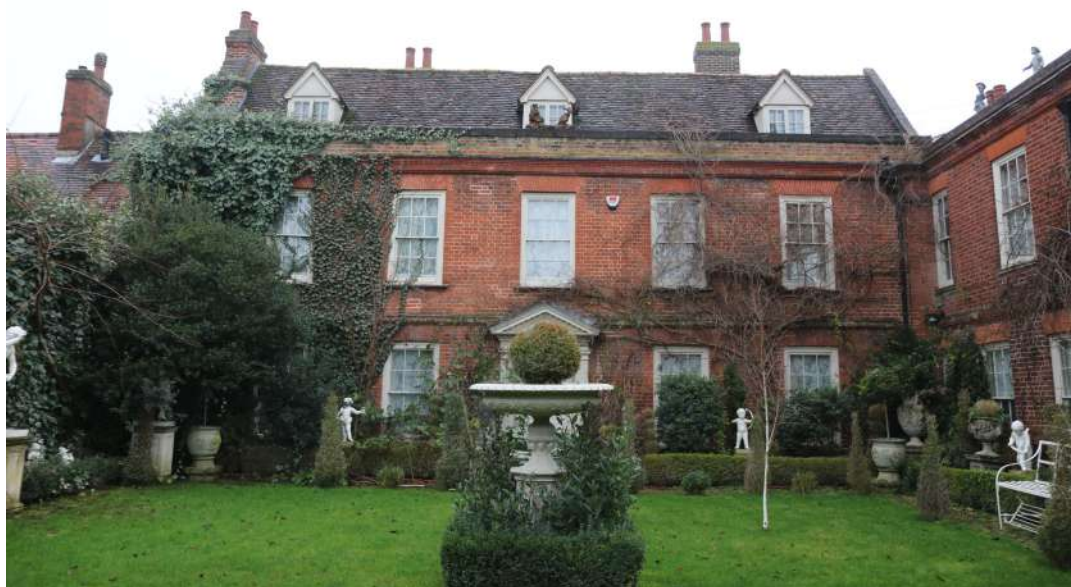
2025.12g_Photograph_213 North-eastern elevation (range 1). Photograph taken facing south-west.
