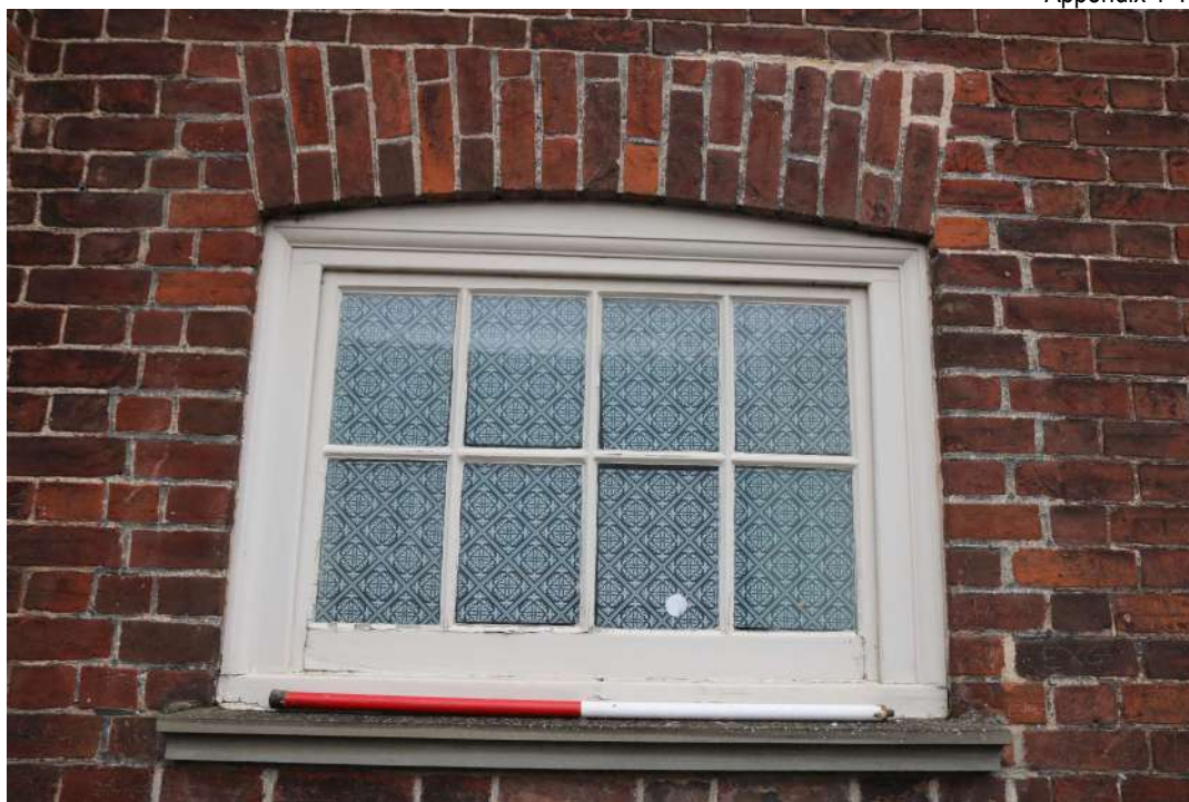
2025.12g_PhotoGraph_257 Detail of window in south-western elevation, ground floor (range 1). Photograph taken facing north-east.
