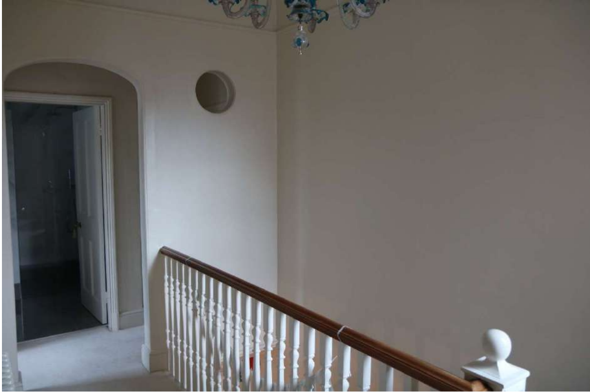
Photograph 38 Interior of landing 2. Photograph taken facing north.
