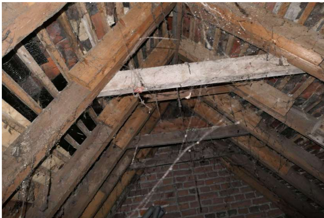
2025.12g_PhotoGraph_259 Detail of roof construction of range 2. Photograph taken facing north-west.
