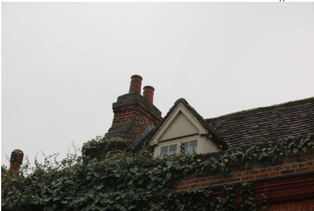
2025.12g_Photograph_225 Detail of south-western chimney. Photograph taken facing south.
