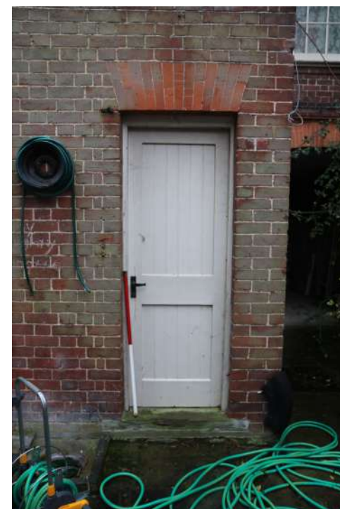
2025.12g_Photograph_230 Detail of door on north-eastern elevation (range 3). Photograph taken facing south-west.
