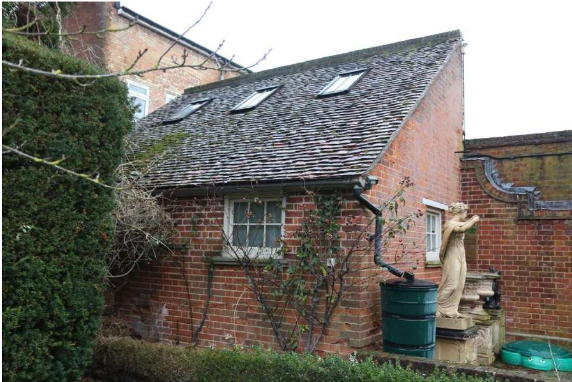
Photograph 44 South-eastern elevation of studio. Photograph taken facing west.
