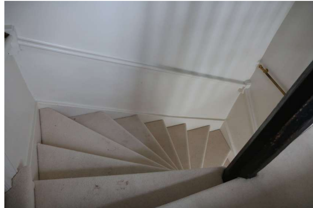
2025.12g_Photograph_156 Detail of staircase 1. Photograph taken facing south-west.
