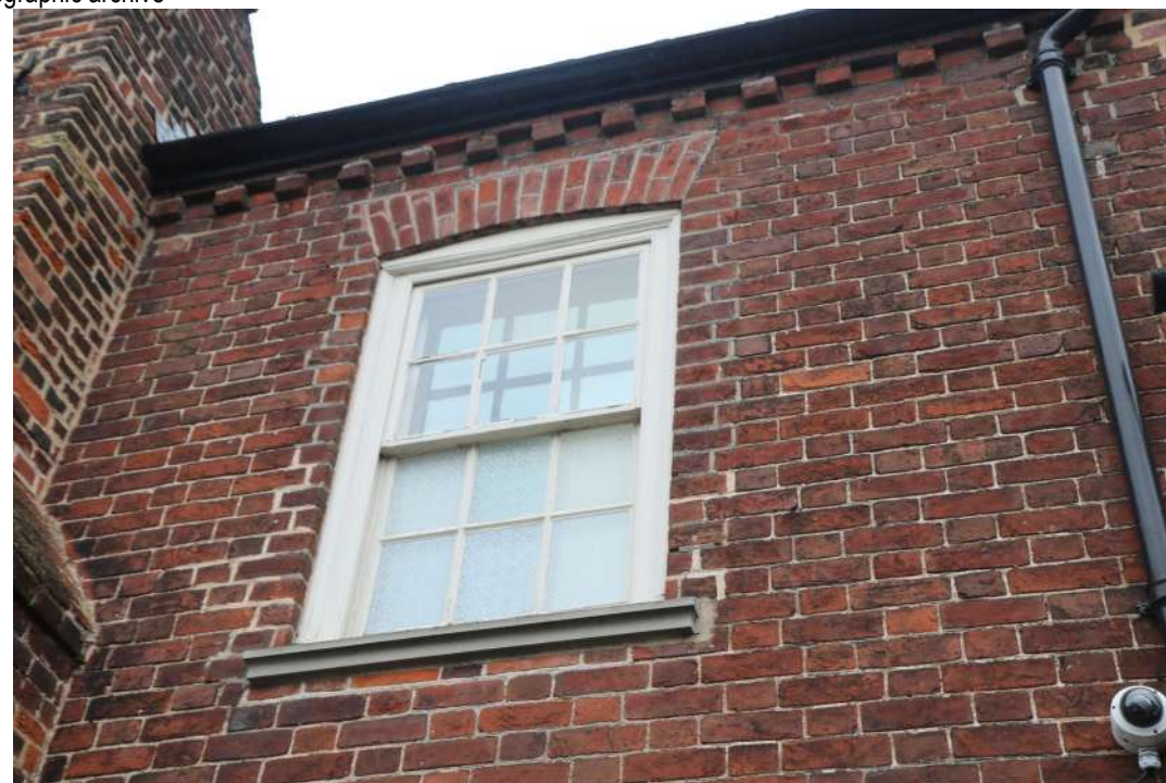
2025.12g_PhotoGraph_258 Detail of window in north-western elevation, first floor (range 1). Photograph taken facing north north-east.
