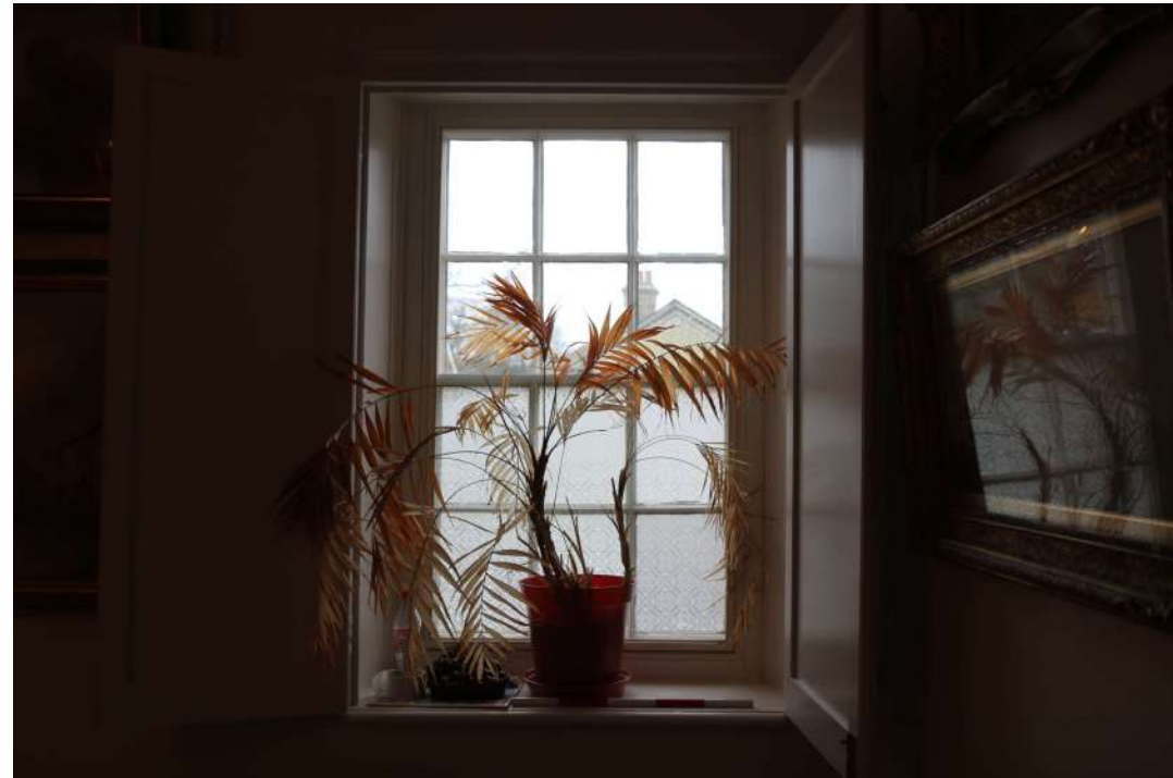
2025.12g_Photograph_128 Detail of window in south-western wall of bedroom 4. Photograph taken facing south-west.
