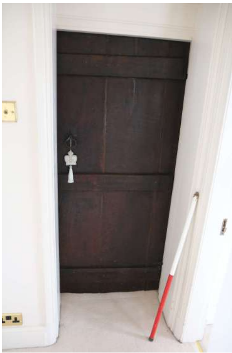
2025.12g_Photograph_089 Detail of door in south-eastern wall of landing 2. Photograph taken facing south-west.
