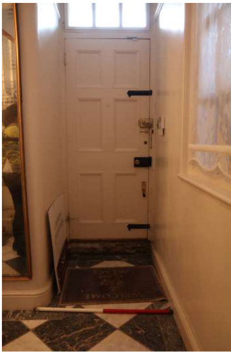
2025.12g_Photograph_053 Detail of door in south-western wall of entrance hall 2. Photograph taken facing south-west.
