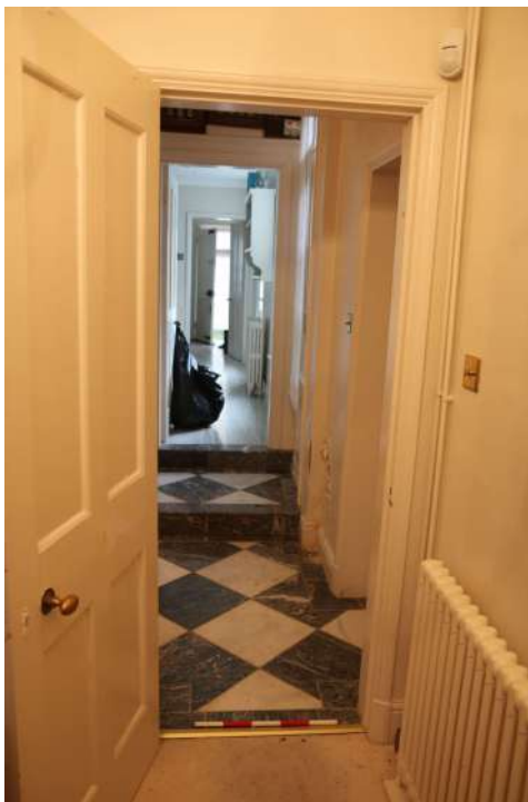
2025.12g_Photograph_065 Detail of door in north-eastern wall of study. Photograph taken facing north-east.
