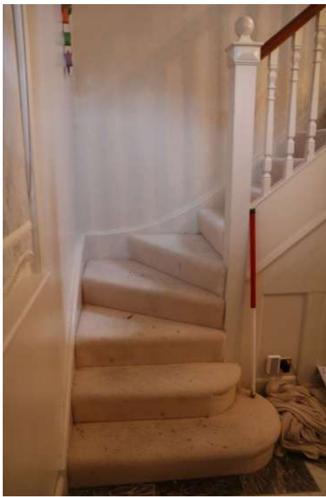
2025.12g_Photograph_057 Detail of staircase 2. Photograph taken facing north-east.
