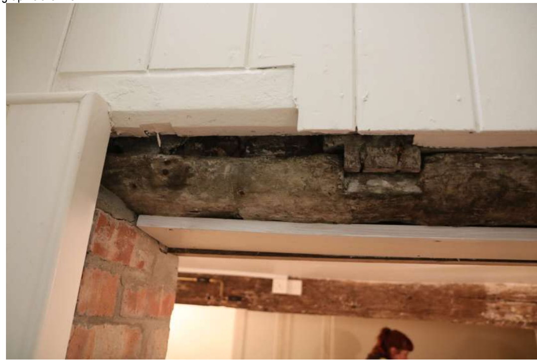
2025.12g_PhotoGraph_178 Detail of exposed timber in basement ceiling. Photograph taken facing south-east.
