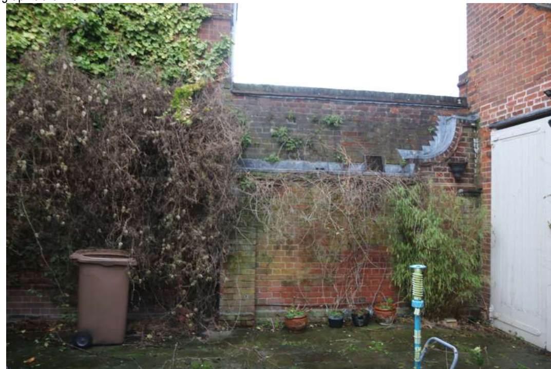
2025.12g_Photograph_234 South-eastern elevation (range 4). Photograph taken facing north-west.
