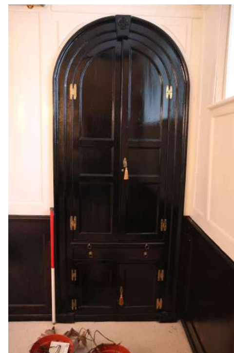
2025.12g_Photograph_010 Detail of built-in cupboard in south-eastern wall of drawing room. Photograph taken facing south-east.
