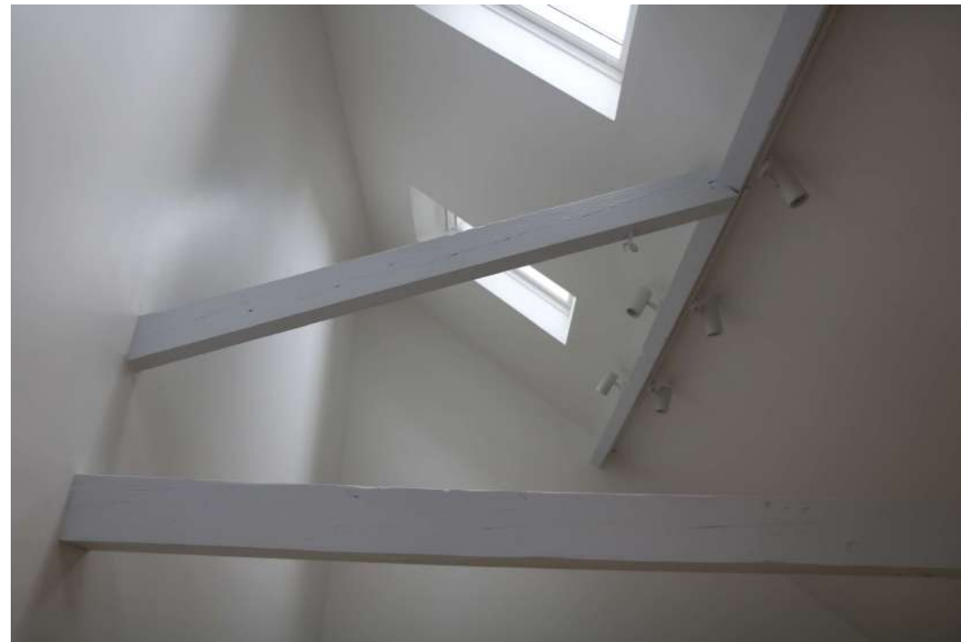
2025.12g_Photograph_184 Detail of exposed roof timbers in studio. Photograph taken facing north-east.
