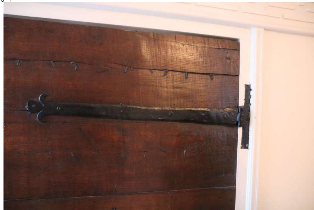
2025.12g_PhotoGraph_134 Detail of strap hinge on door in south-eastern wall of bedroom 4. Photograph taken facing south-east.
