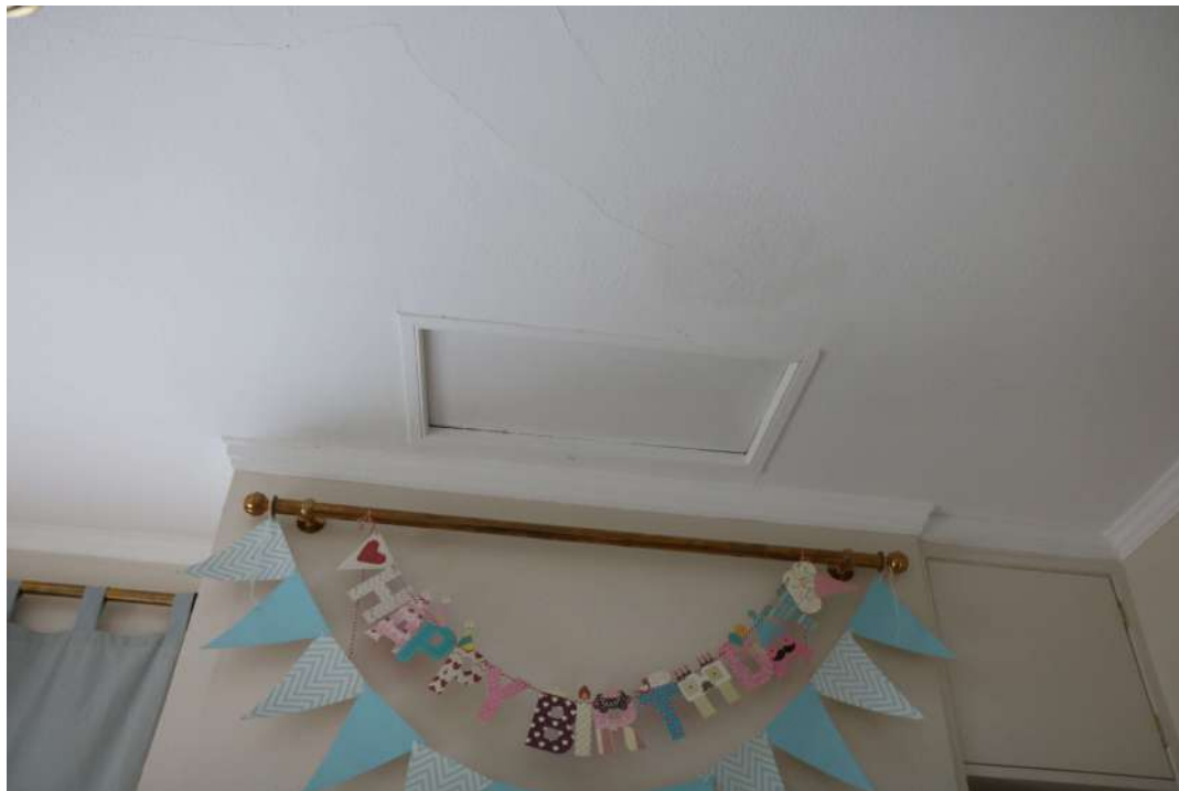
2025.12g_Photograph_119 Detail of opening in ceiling of bedroom 3. Photograph taken facing north-west.
