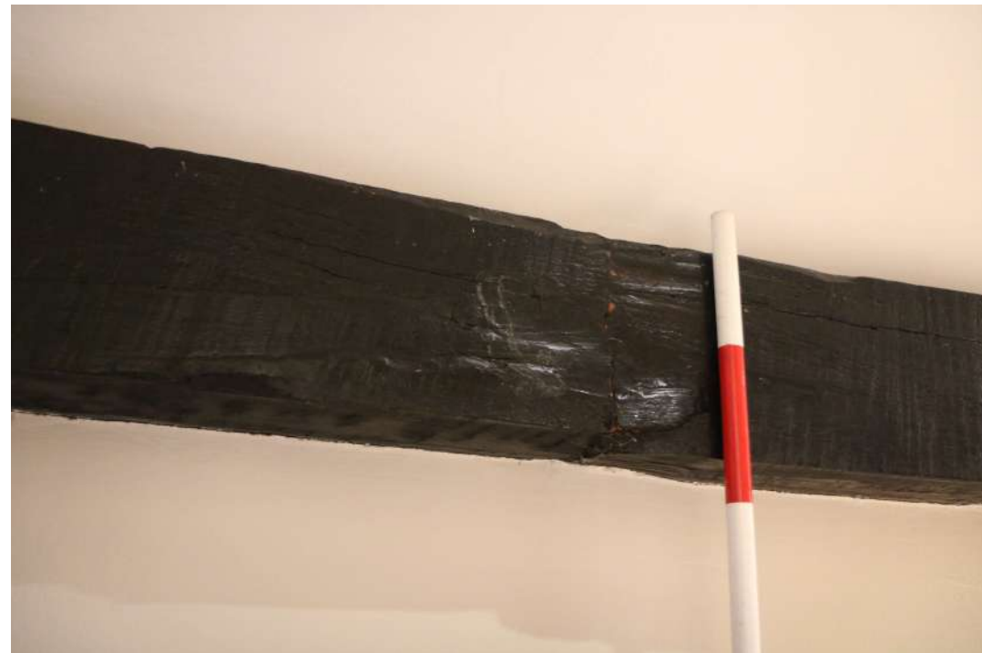
2025.12g_PhotoGraph_168 Detail of possible scarf-joint in south-western purlin in bedroom 7. Photograph taken facing west.
