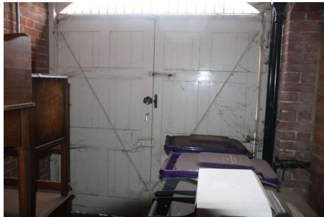
2025.12g_Photograph_192 Detail of doors in south-western wall of courtyard passage. Photograph taken facing south-west.
