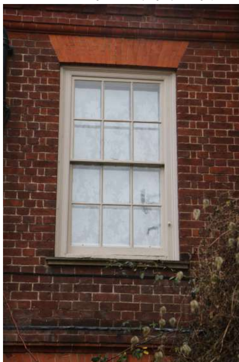
2025.12g_Photograph_231 Detail of window on north-eastern elevation, first floor (range 3). Photograph taken facing south-west.
