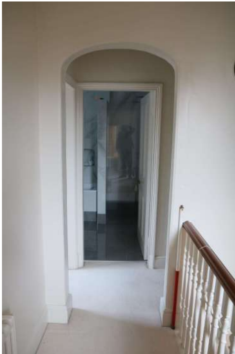
2025.12g_Photograph_091 Detail of arched opening in landing 2. Photograph taken facing north-west.
