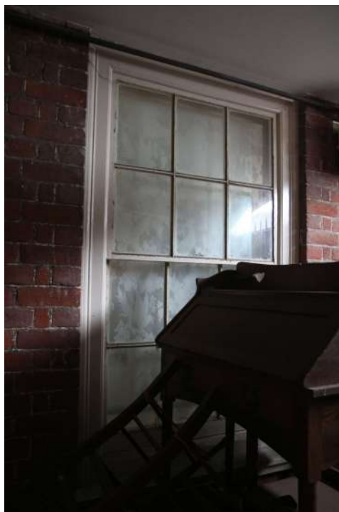
2025.12g_Photograph_191 Detail of window in south-eastern wall of courtyard passage. Photograph taken facing south.
