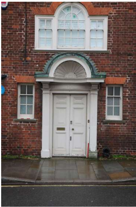
2025.12g_Photograph_253 Detail of door and windows in south-western elevation (range 1). Photograph taken facing north-east.
