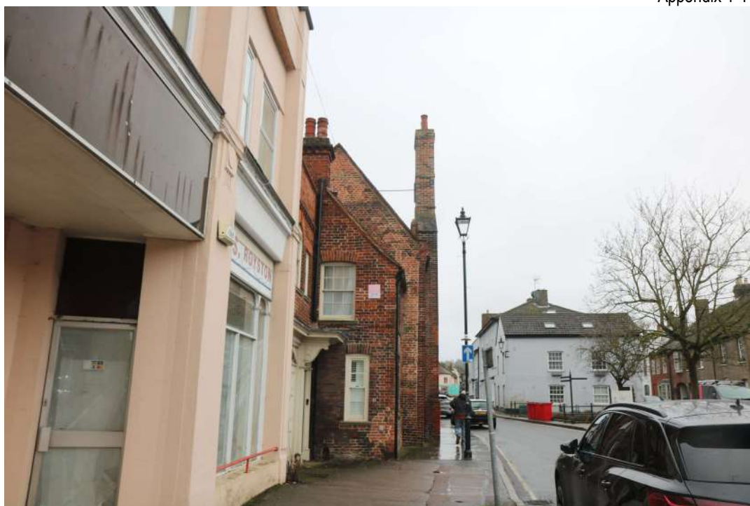
2025.12g_Photograph_237 North-western elevation (ranges 1, 2 and 3). Photograph taken facing south-east.
