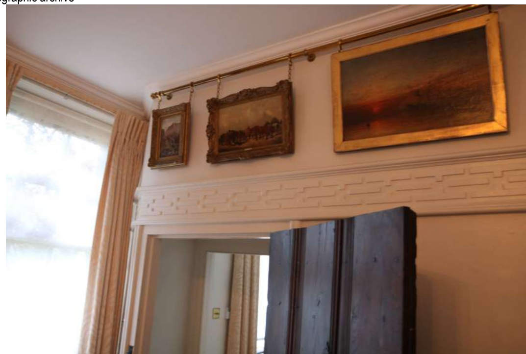
2025.12g_Photograph_130 Detail of decorative frieze on south-eastern wall of bedroom 4. Photograph taken facing south south-east.
