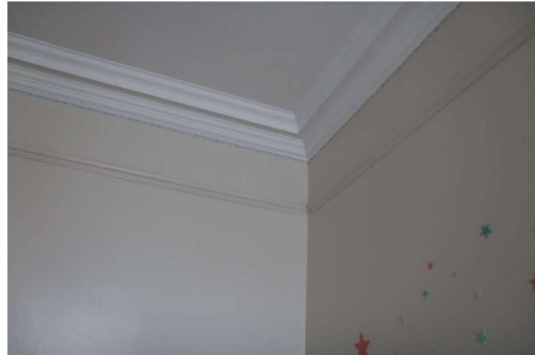
2025.12g_Photograph_100 Detail of picture rail and cornicing in bedroom 1. Photograph taken facing west.
