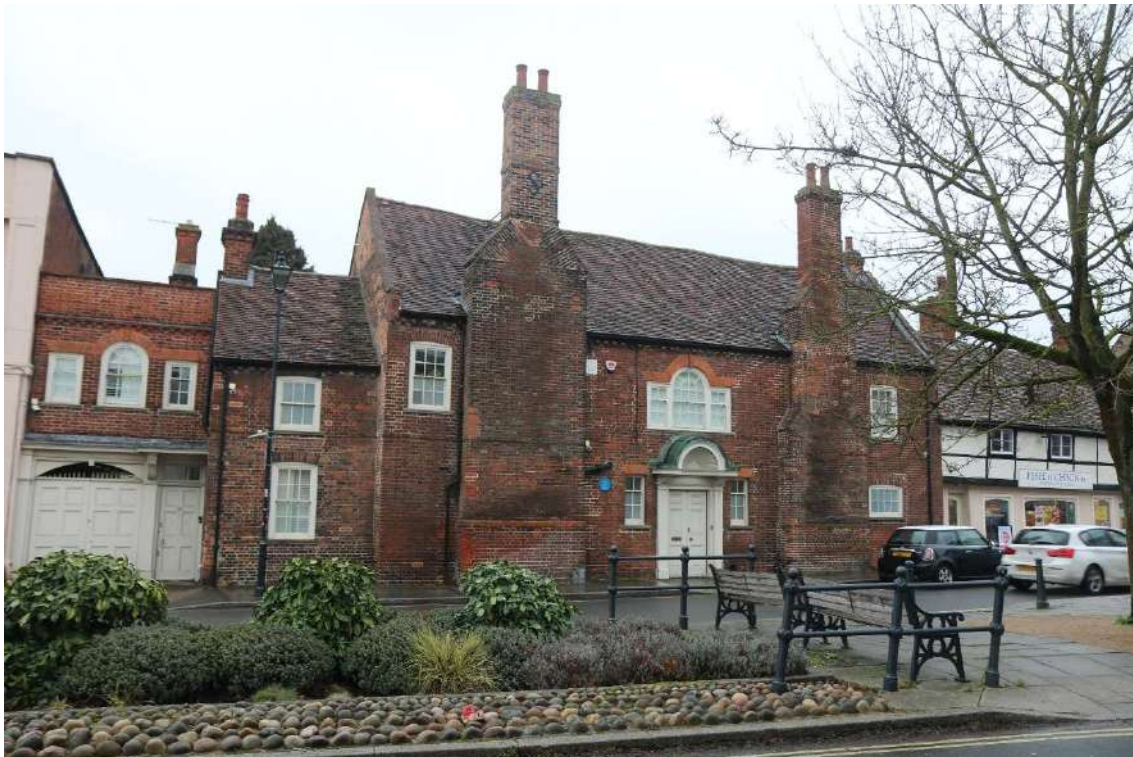
Photograph 5 South-western elevation. Photograph taken facing east.
