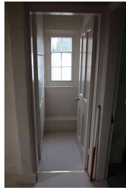
2025.12g_Photograph_094 Detail of door in south-western wall of landing 2. Photograph taken facing south-west.
