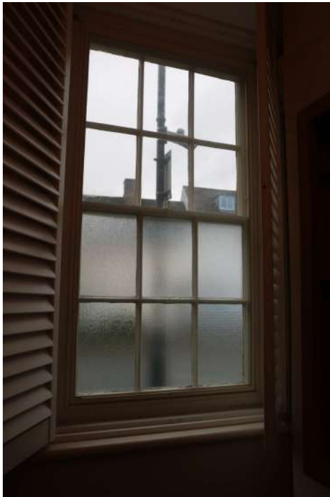
2025.12g_Photograph_063 Detail of window in south-western wall of study. Photograph taken facing west south-west.
