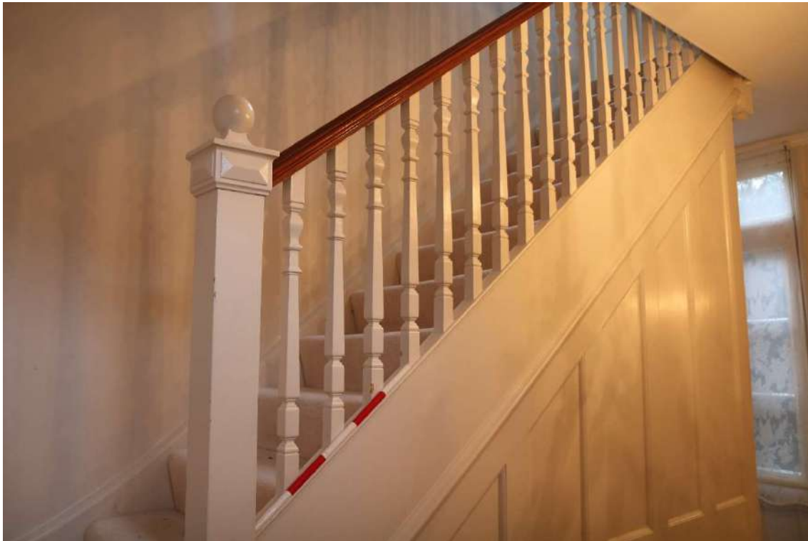
Photograph 24 Detail of newel post, handrail and balusters of staircase 2. Photograph taken facing east.
