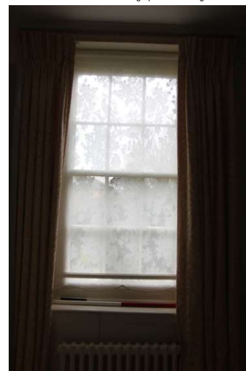
2025.12g_Photograph_144 Detail of window in north-eastern wall of bedroom 5. Photograph taken facing north-east.
