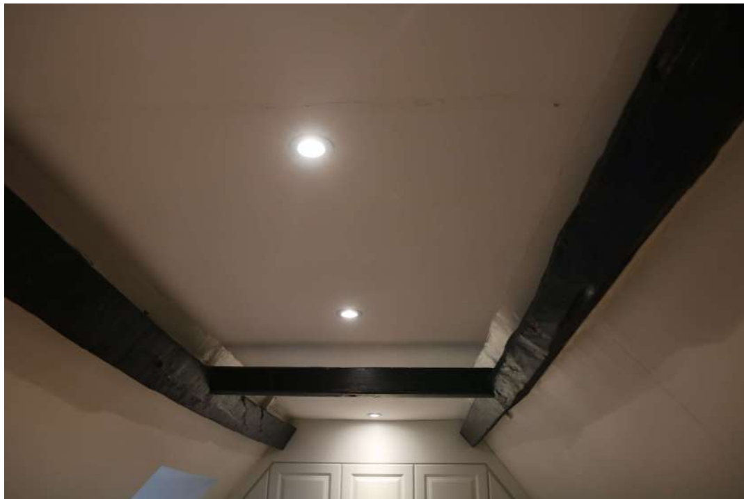
2025.12g_PhotoGraph_167 Detail of exposed purlins in ceiling of bedroom 7. Photograph taken facing south-east.
