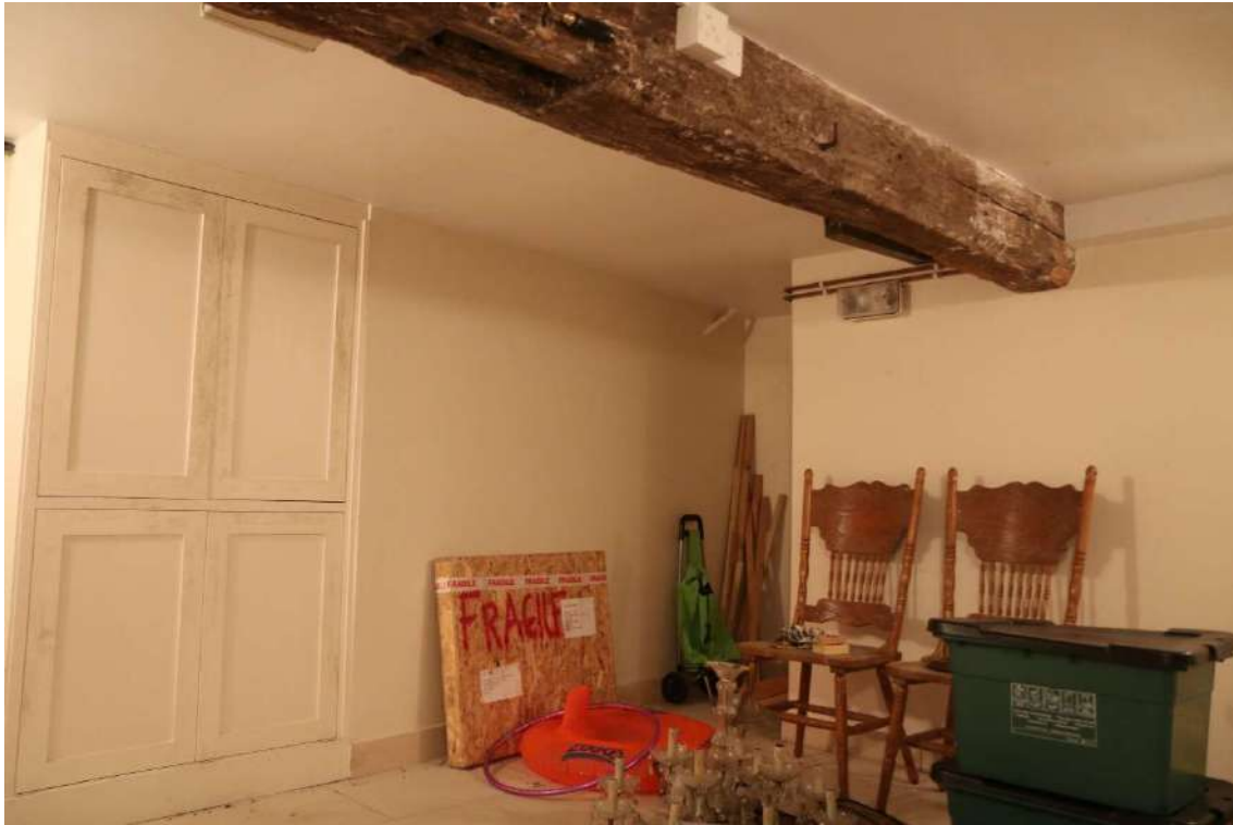
Photograph 13 Interior of basement. Photograph taken facing south.
