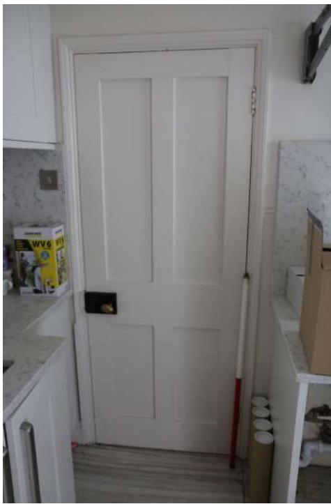
2025.12g_Photograph_077 Detail of door in south-western wall of utility room. Photograph taken facing south-west.
