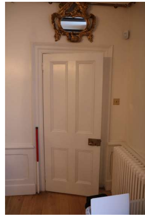
2025.12g_Photograph_046 Detail of door in north-western wall of dining room. Photograph taken facing north-west.
