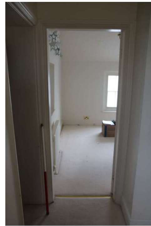
2025.12g_Photograph_090 Detail of door in south-western wall of landing 2. Photograph taken facing south-west.
