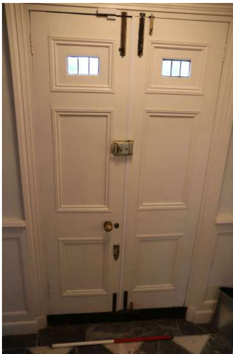
2025.12g_Photograph_029 Detail of doors in north-eastern wall of entrance hall 1. Photograph taken facing north-east.
