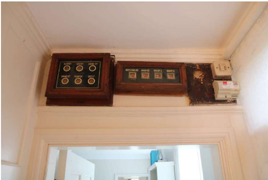
Photograph 25 Detail of butler's bell boxes on north-eastern wall of entrance hall 2. Photograph taken facing north-east.
