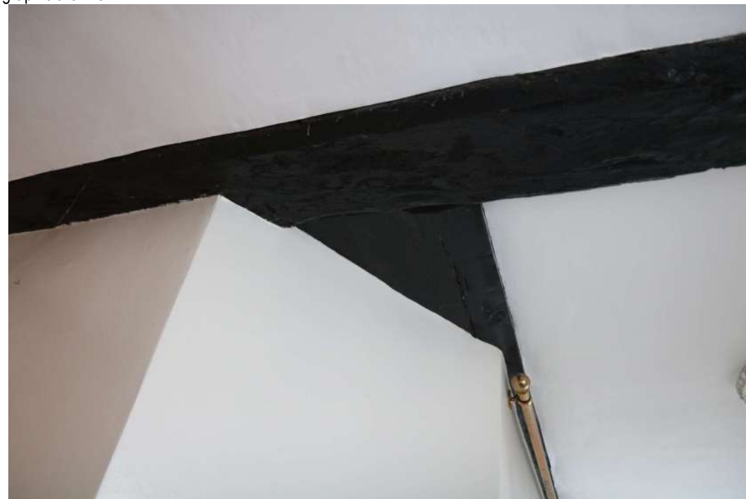
2025.12g_PhotoGraph_026 Detail of exposed timbers in ceiling of entrance hall 1. Photograph taken facing east.
