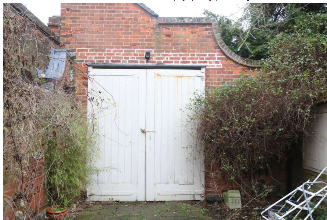
2025.12g_Photograph_200 South-western elevation of studio (range 4). Photograph taken facing north-east.
