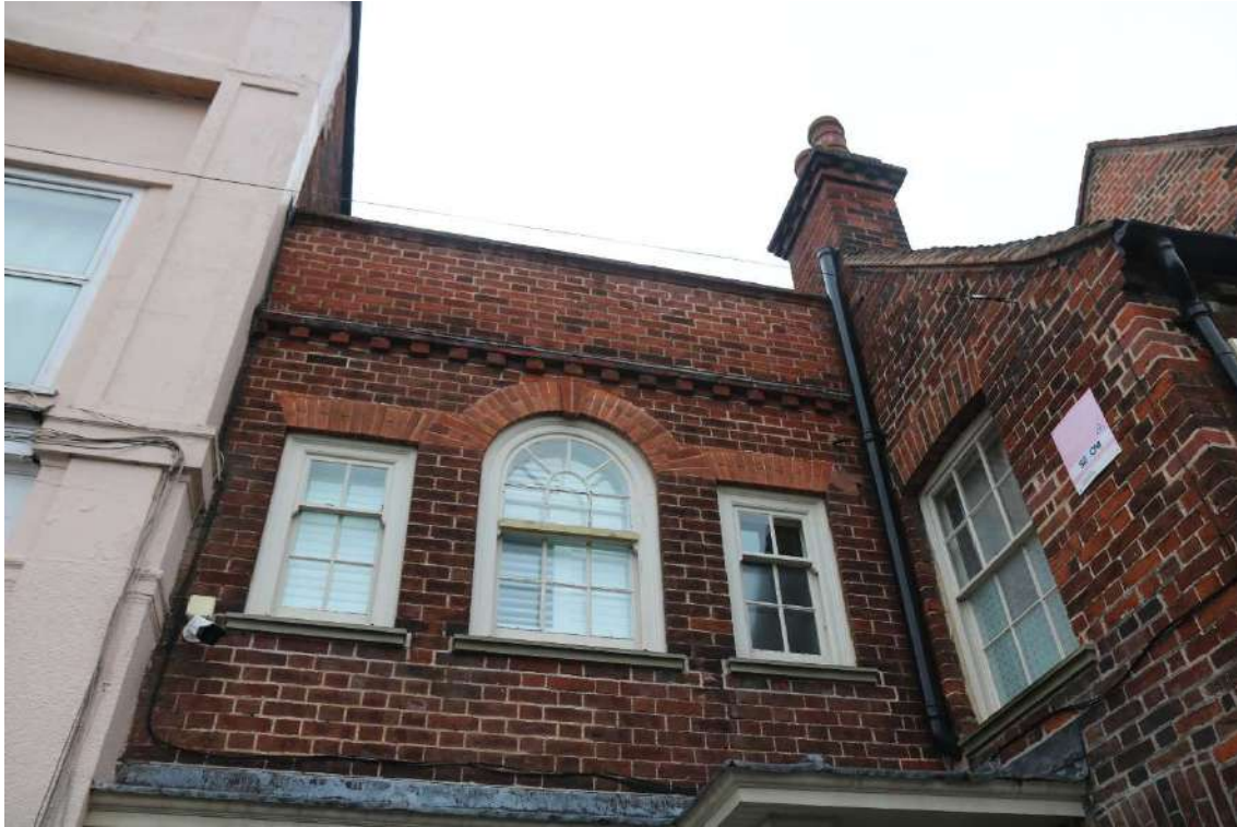
Photograph 9 Detail of windows and parapet of south-western elevation, first floor of range 3. Photograph taken facing east north-east.
