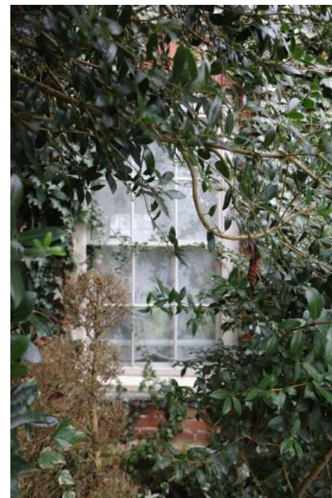
2025.12g_Photograph_216 Detail of window in north-eastern elevation, ground floor (range 1). Photograph taken facing north-west.
