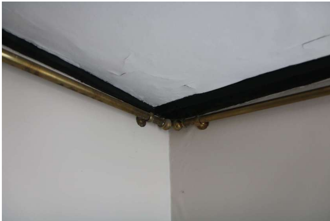
2025.12g_PhotoGraph_027 Detail of exposed timber in ceiling of entrance hall 1. Photograph taken facing east.
