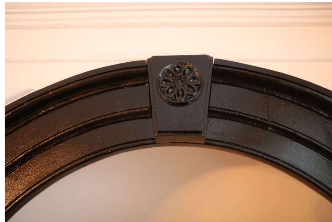
2025.12g_Photograph_012 Detail of decorative carving on arch of built-in cupboard in south-eastern wall of drawing room. Photograph taken facing south-east.
