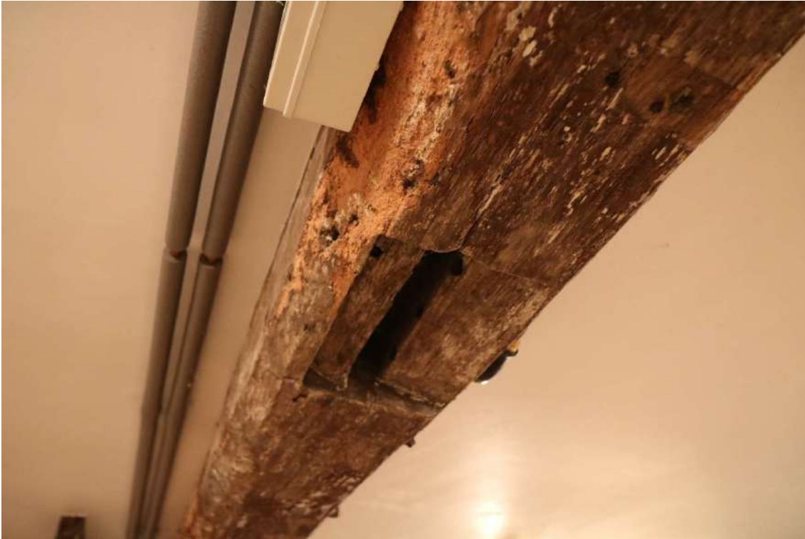
Photograph 14 Detail of empty mortice on binding beam in basement ceiling. Photograph taken facing south-west.
