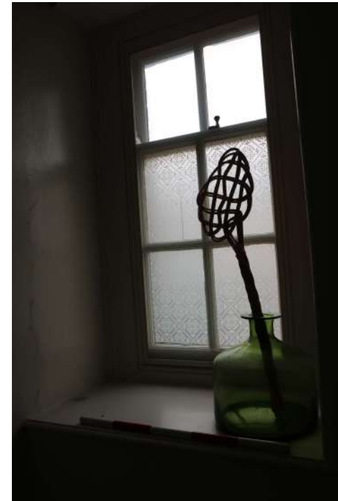
2025.12g_Photograph_024 Detail of window in south-western wall of entrance hall 1. Photograph taken facing south south-west.
