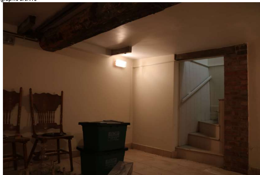
2025.12g_PhotoGraph_174 Interior of basement. Photograph taken facing west.
