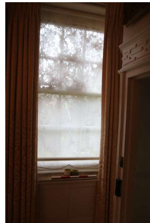
2025.12g_Photograph_132 Detail of window in north-eastern wall of bedroom 4. Photograph taken facing north-east.
