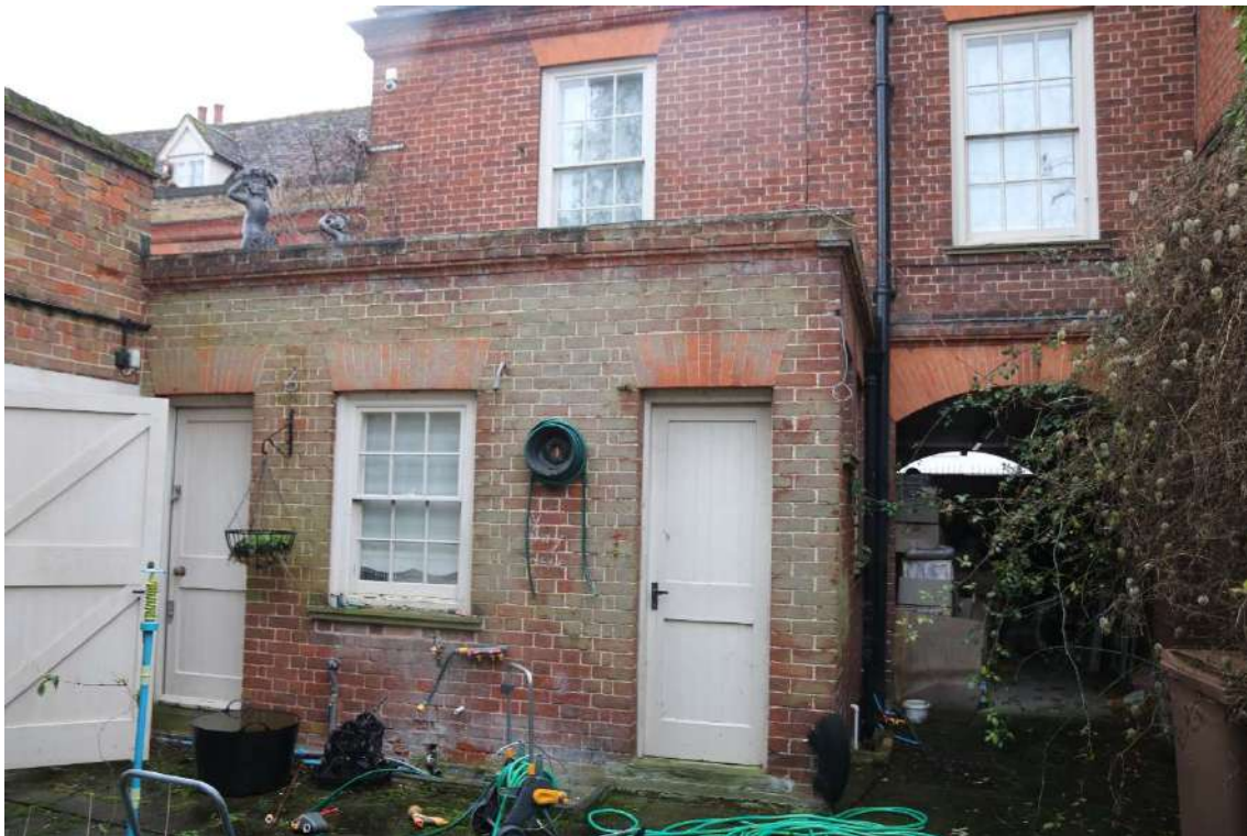
Photograph 3 North-eastern elevation of range 3. Photograph taken facing south south-west.
