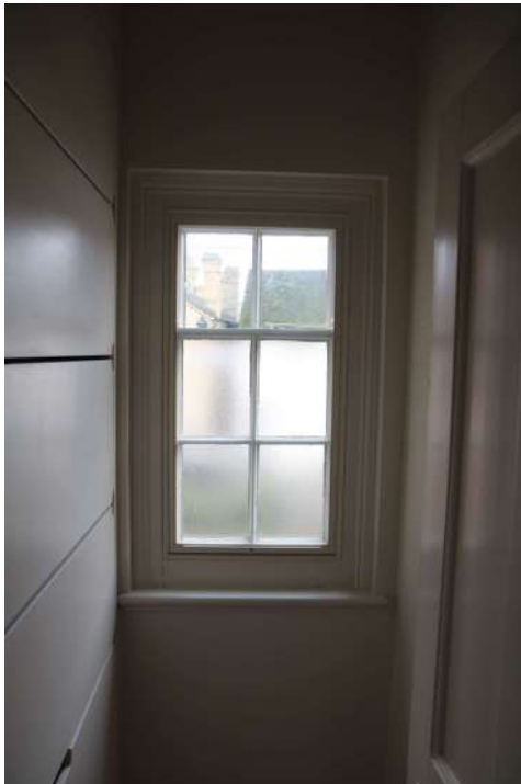
2025.12g_Photograph_095 Detail of window in south-western wall of store. Photograph taken facing south-west.
