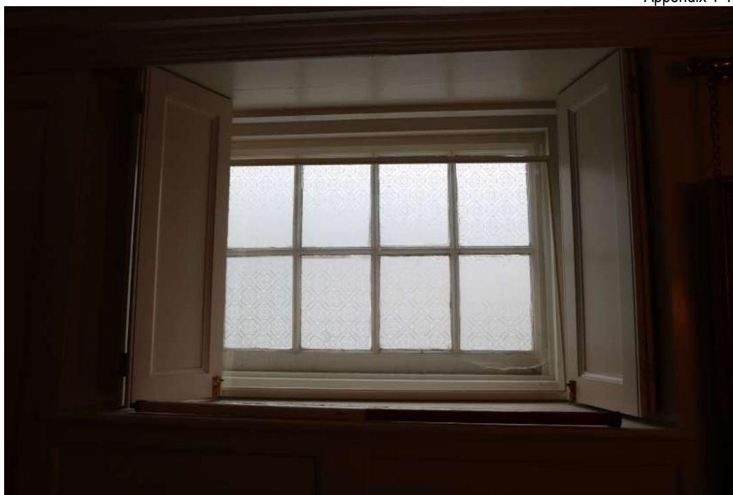
2025.12g_Photograph_009 Detail of window in south-western wall of drawing room. Photograph taken facing south-west.
