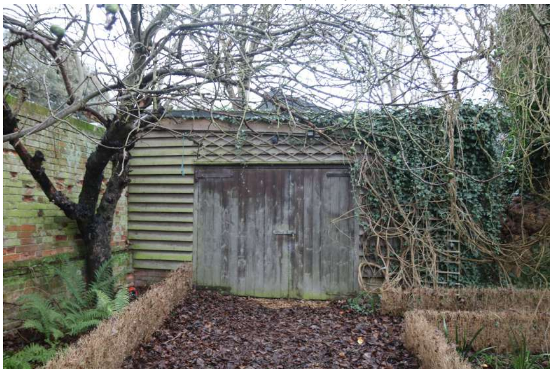
2025.12g_Photograph_235 North-western elevation of garage. Photograph taken facing south-east.
