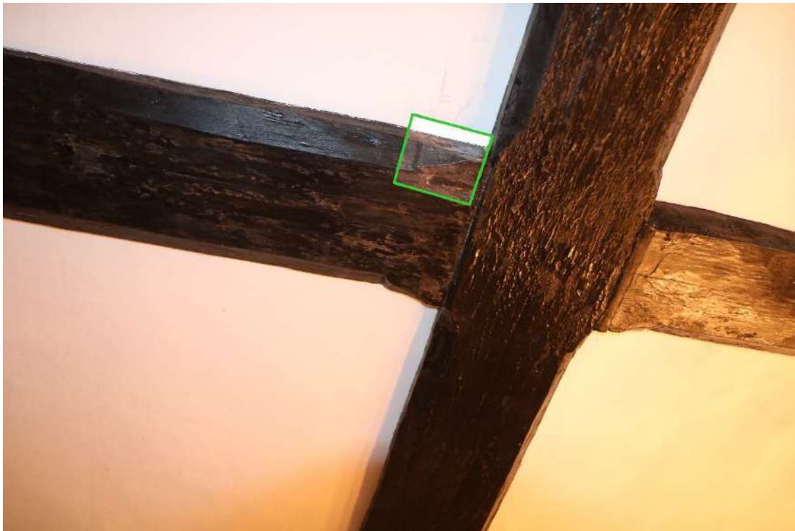
Photograph 16 Detail of carved stops in binding beam and bridging joists in ceiling of drawing room. Example of a lamb's tongue stop highlighted in green. Photograph taken facing west.
