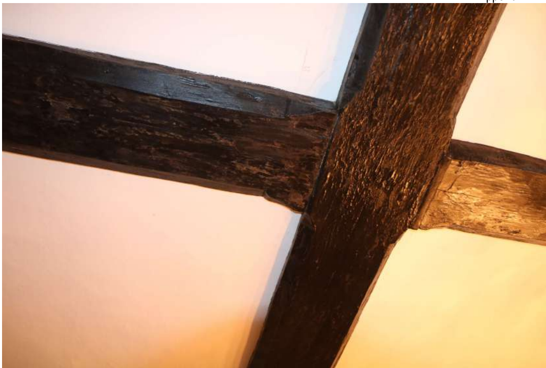
2025.12g_Photograph_005 Detail of carved stops in binding beam and bridging joists in ceiling of drawing room. Photograph taken facing west.
