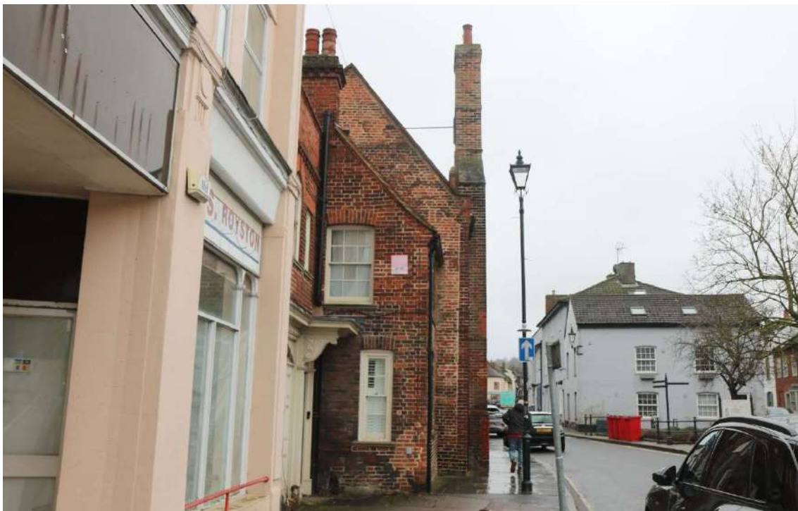
Photograph 10 North-western elevation. Photograph taken facing south-east.
