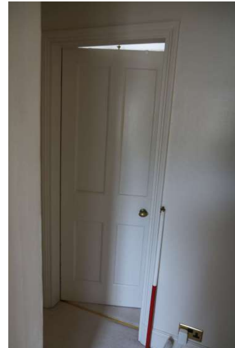
2025.12g_Photograph_096 Detail of door in north-eastern wall of landing 2. Photograph taken facing north north-east.
