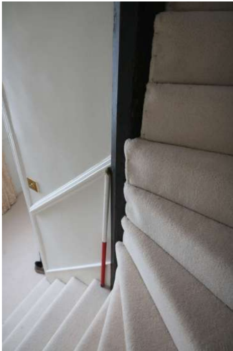
2025.12g_Photograph_155 Detail of hand-carved post in staircase 1. Photograph taken facing south.
