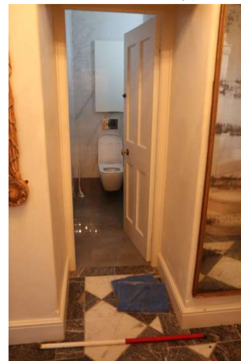
2025.12g_Photograph_052 Detail of door in south-western wall of entrance hall 2. Photograph taken facing south-west.
