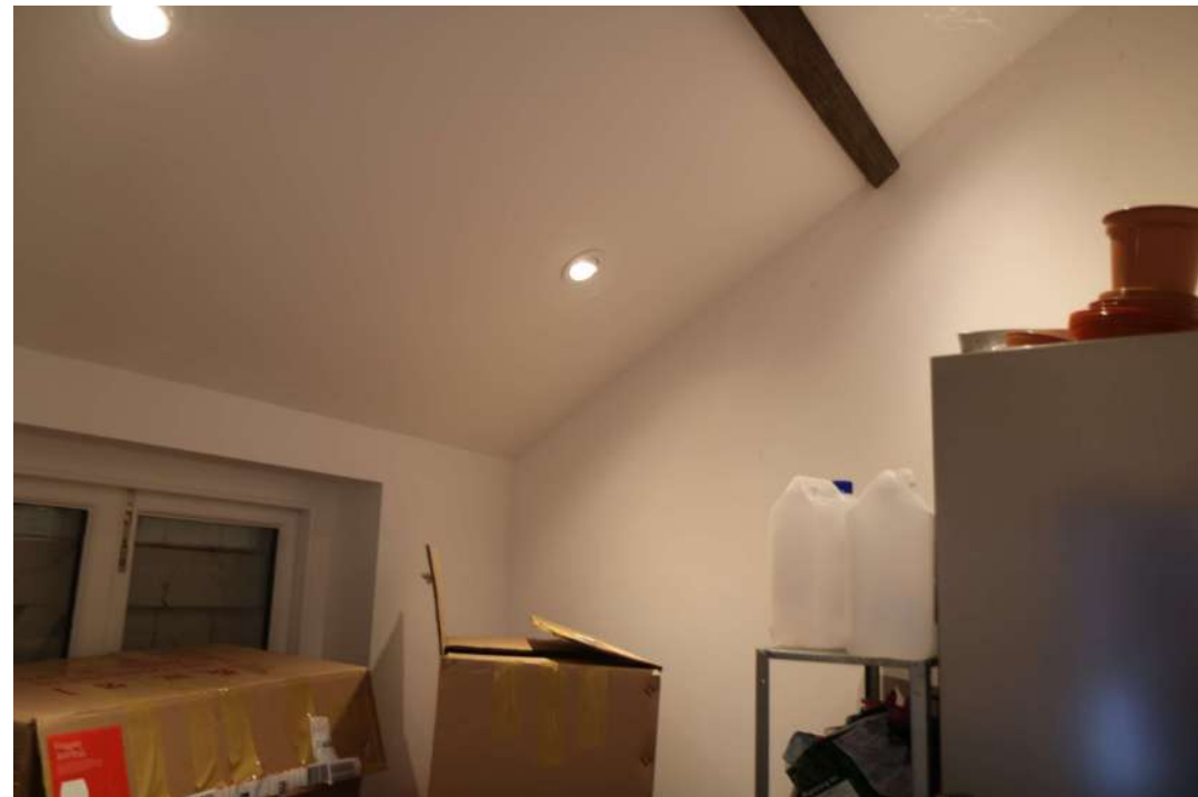
2025.12g_Photograph_188 Interior of storage shed. Photograph Taken facing north.
