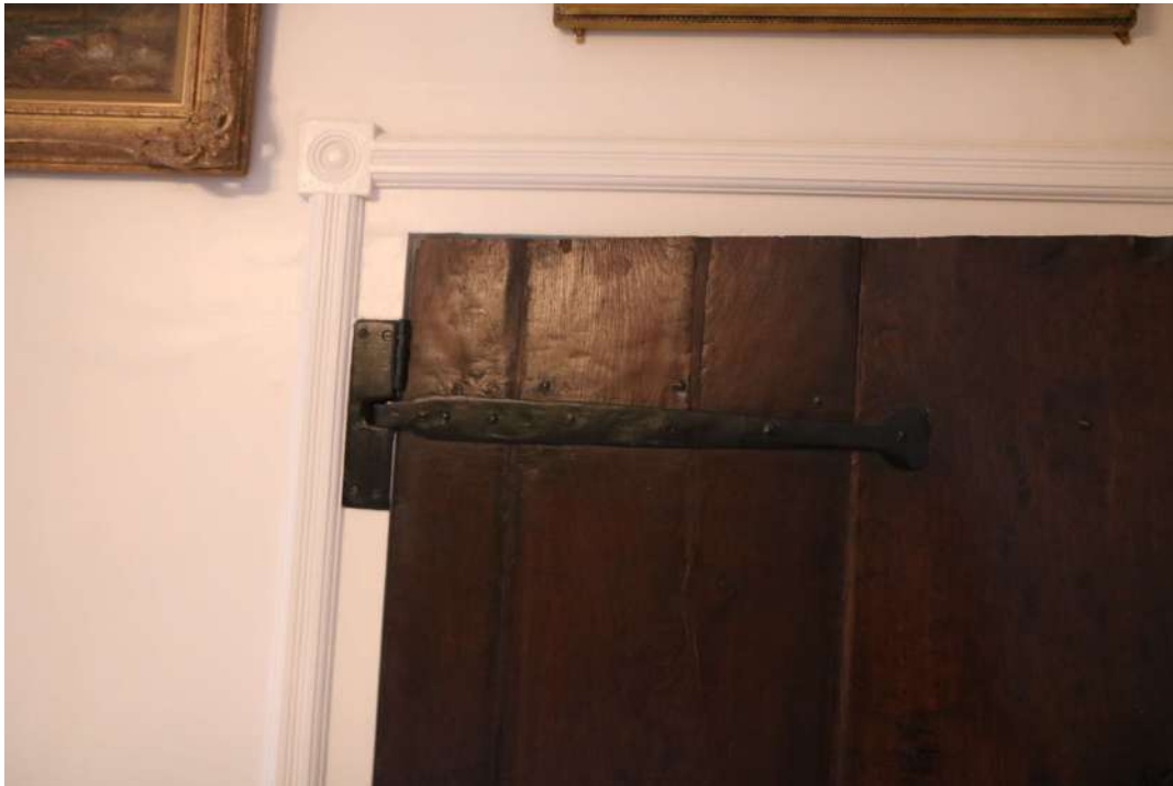
2025.12g_Photograph_127 Detail of strap hinge on door in north-western wall of bedroom 4. Photograph taken facing north-west.
