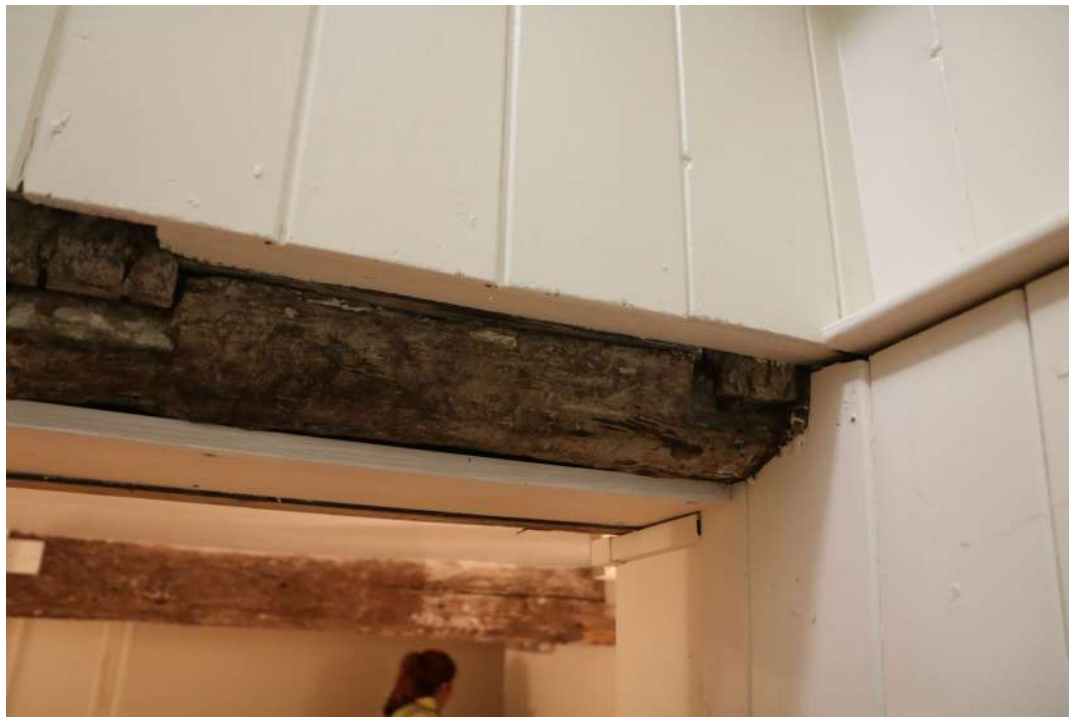
2025.12g_PhotoGraph_179 Detail of exposed timber in basement ceiling. Photograph taken facing south.
