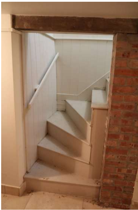
2025.12g_PhotoGraph_177 Detail of basement stairs. Photograph taken facing north-west.
