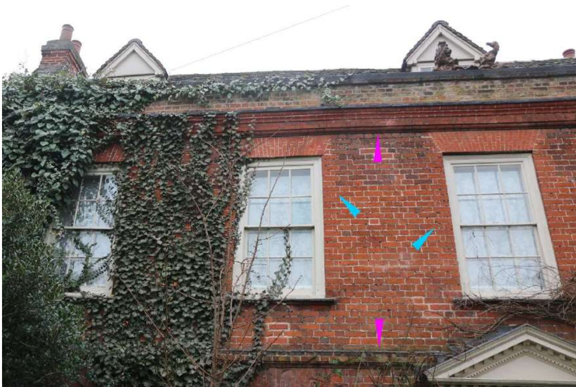
Photograph 2 Detail of windows in north-eastern elevation, first floor. Blue arrows highlight the queen closers and pink arrows highlighting the decorative brickwork. Photograph taken facing south-west.
