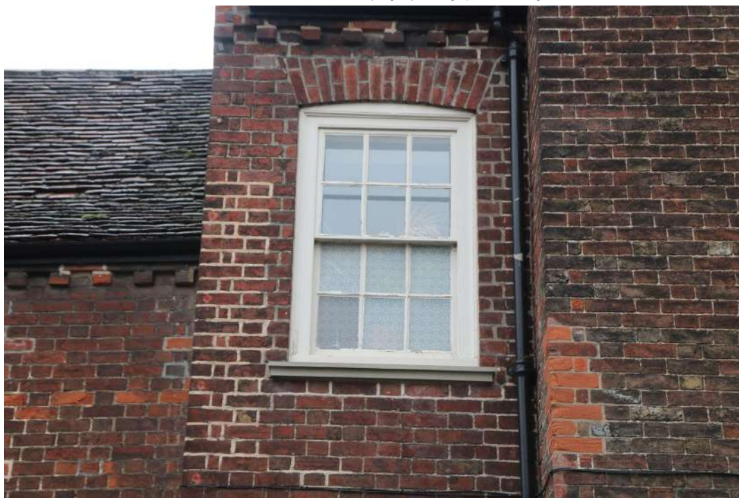
2025.12g_Photograph_251 Detail of window in south-western elevation, first floor (range 2). Photograph taken facing north-east.
