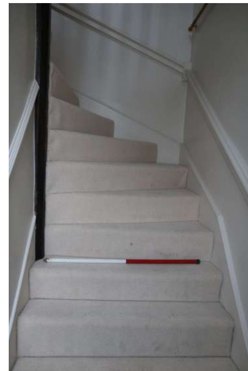
2025.12g_Photograph_154 Detail of staircase 1. Photograph taken facing south-west.
