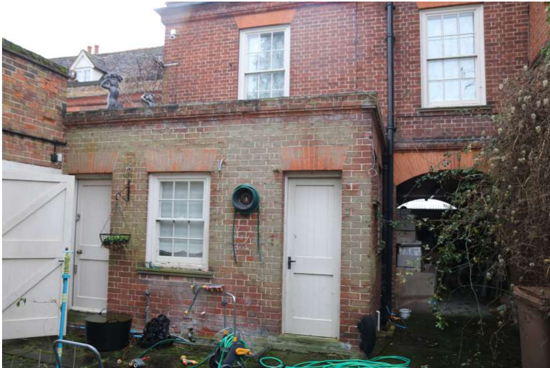
2025.12g_Photograph_227 North-eastern elevation (range 3). Photograph taken facing south south-west.
