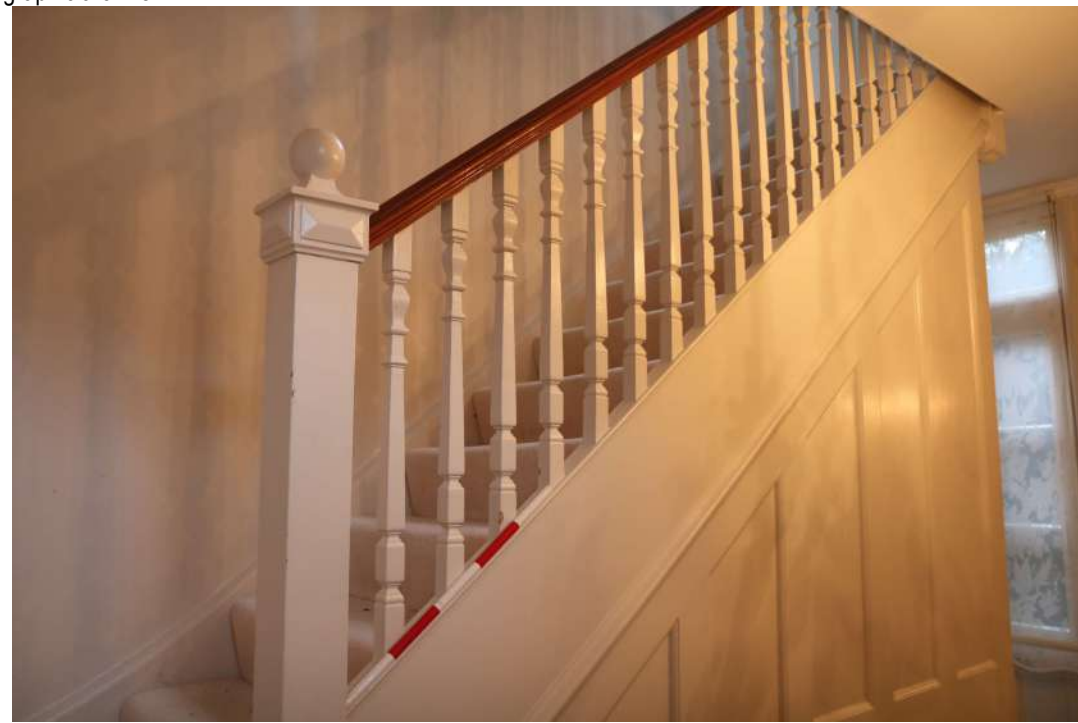
2025.12g_Photograph_058 Detail of newel post, handrail and balusters of staircase 2. Photograph taken facing east.
