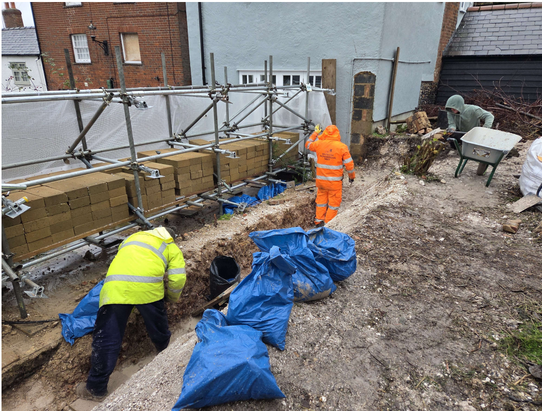
Photograph 1 The trench during excavation, looking north-east.
