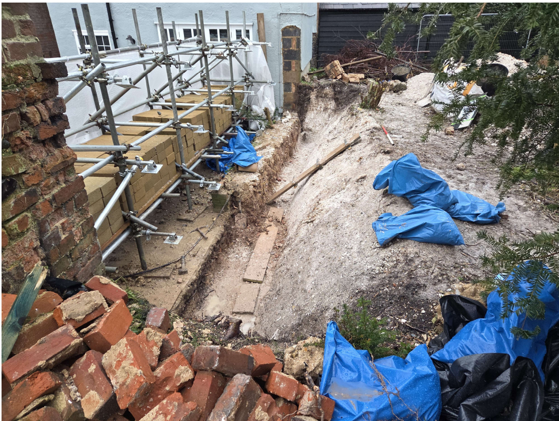
Photograph 2 The fully excavated trench, looking east.
