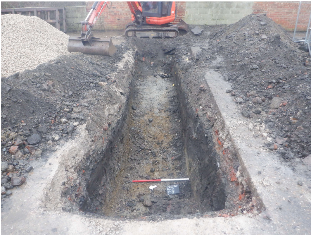
Photograph 1 Trench 1, looking east-north-east.
