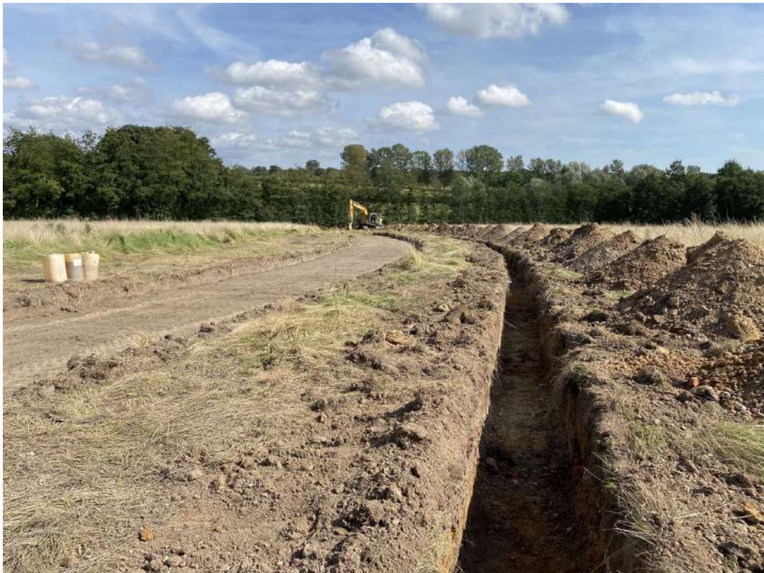
Photograph 5 Service trench – view east.
