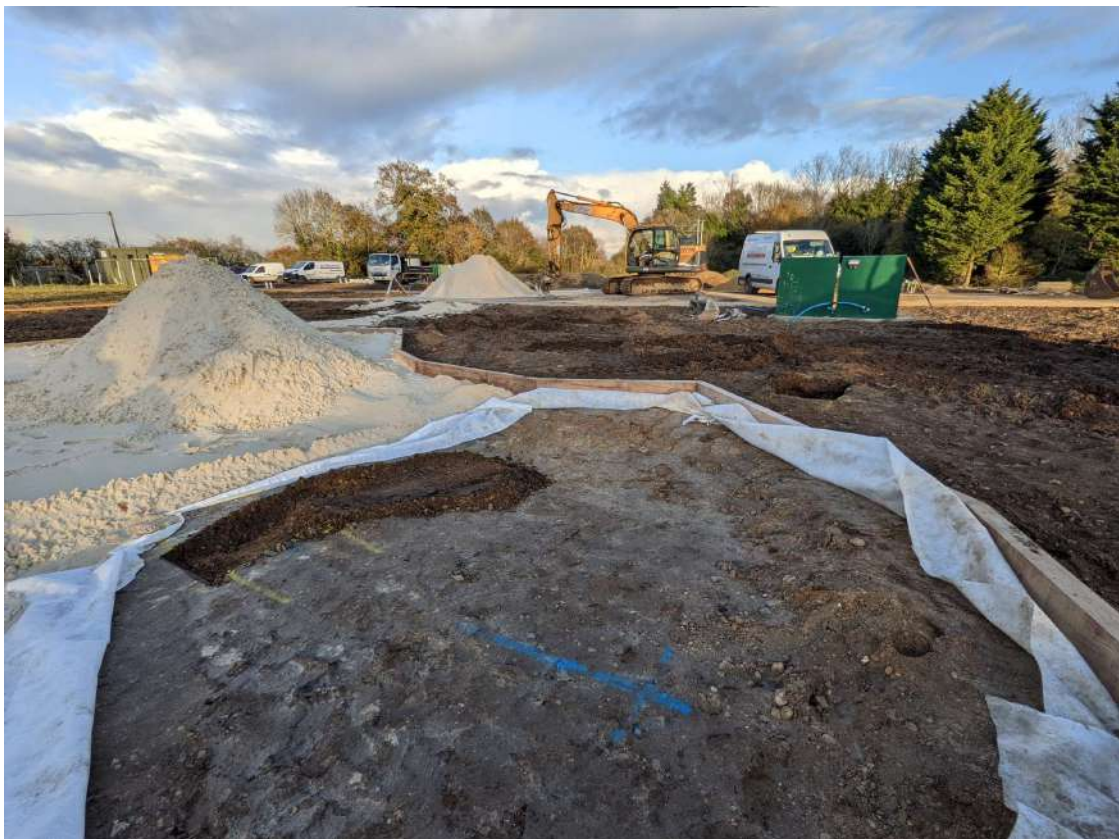
Photograph 11 Sand pit area – view north-east.
