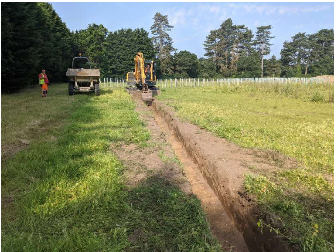
Photograph 6 Service trench working shot – view west.
