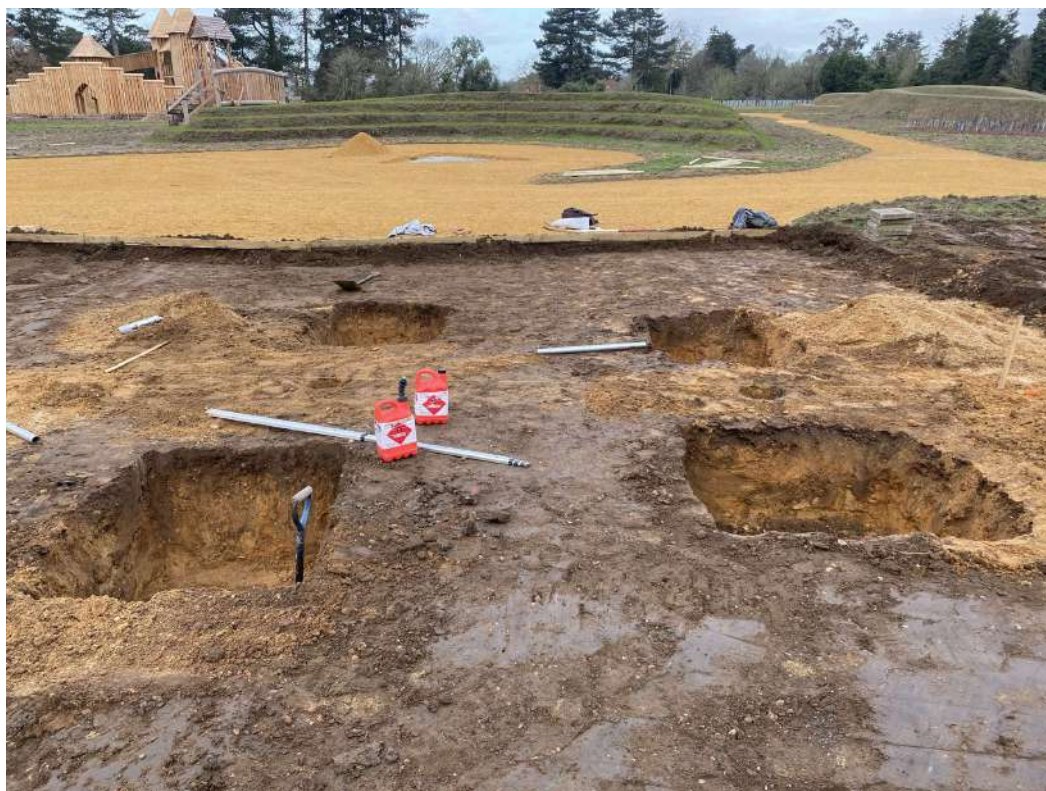
Photograph 13 Galleon foundation pads – view west.
