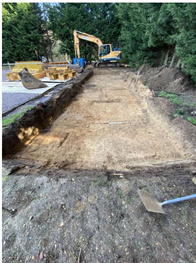
Photograph 12 Tank trench – view north-east.
