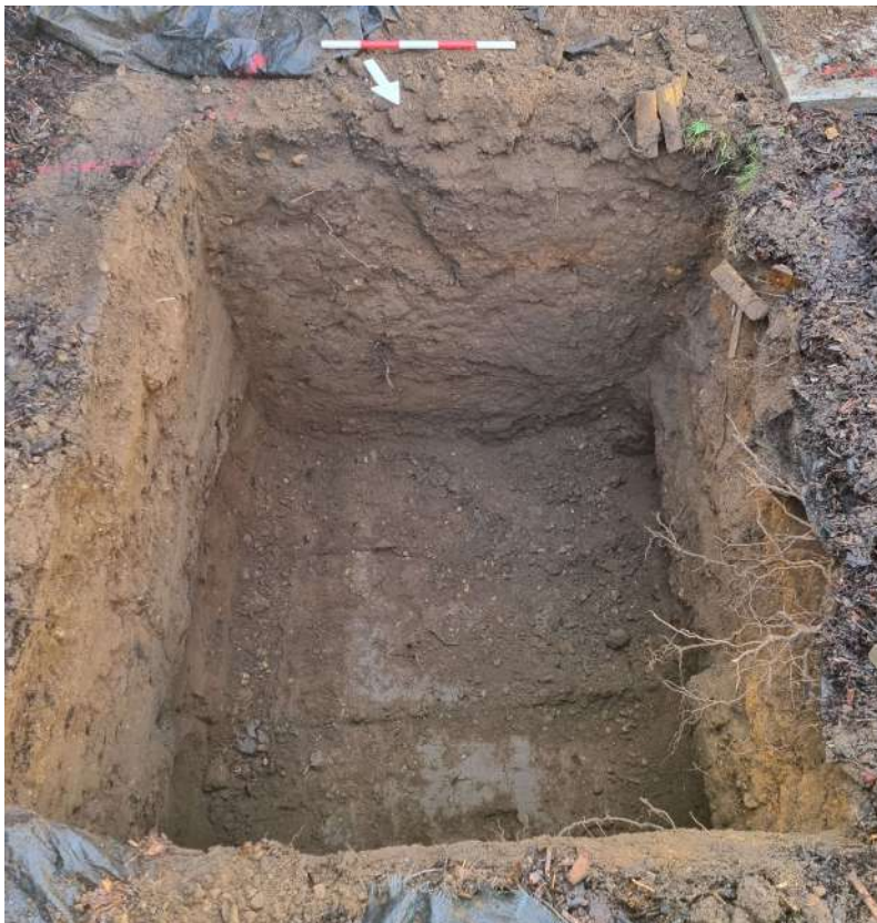
Photograph 6 The soakaway, looking south.
