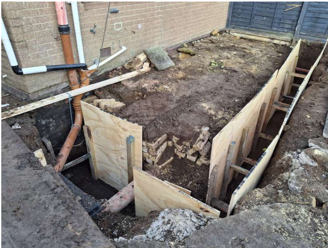
Photograph 2 The foundation trenches, looking north-west.
