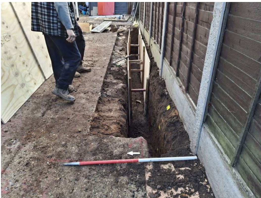
Photograph 4 The far southern foundation trench (with F1 in base), looking east.
