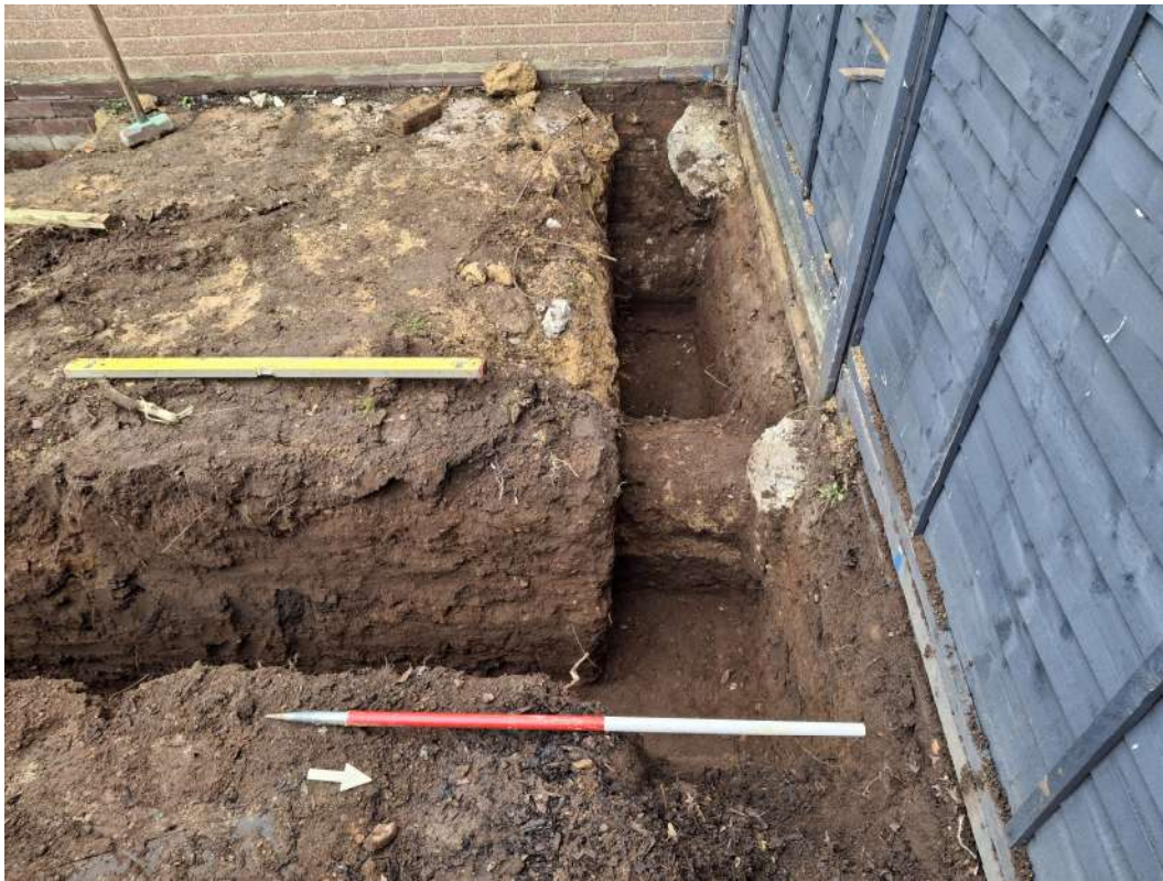
Photograph 1 The far northern foundation trench, looking west.
