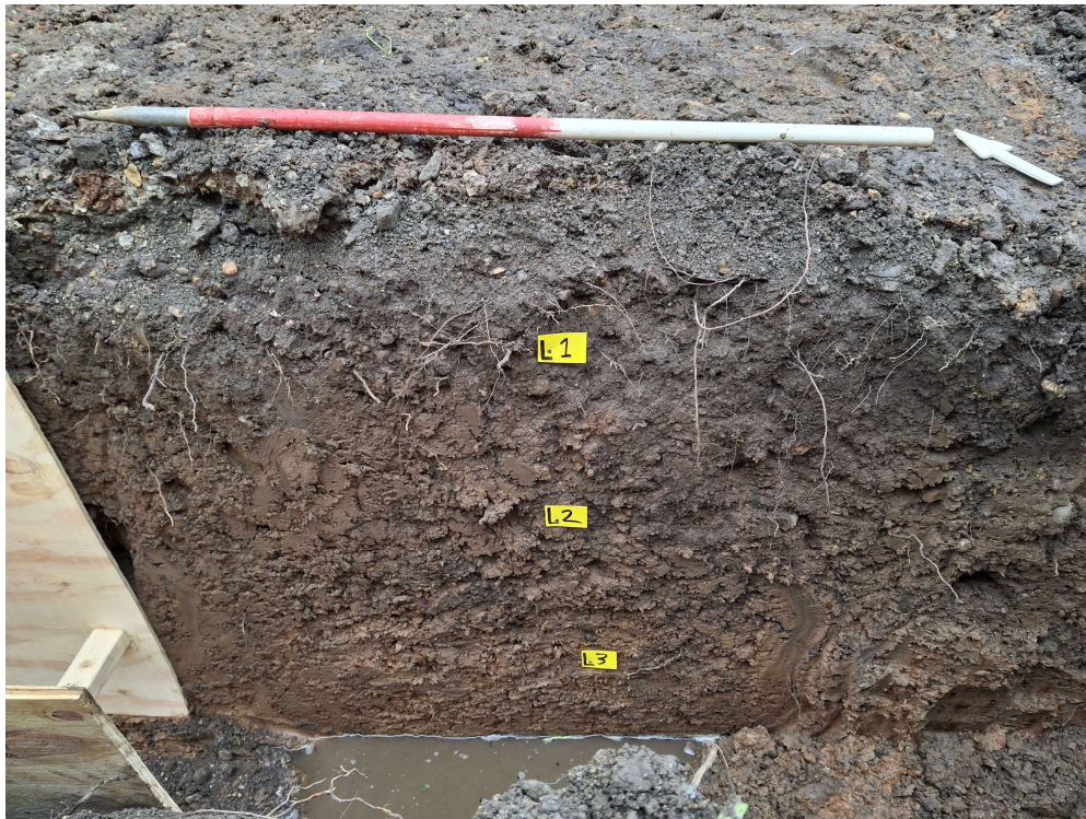
Photograph 4 Representative section of foundation trench, looking north-east.
