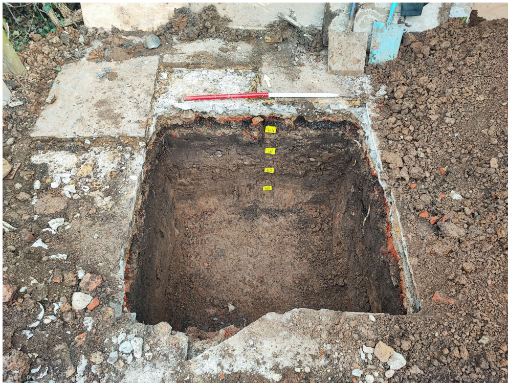
Photograph 5 Representative section of soakaway, looking north.
