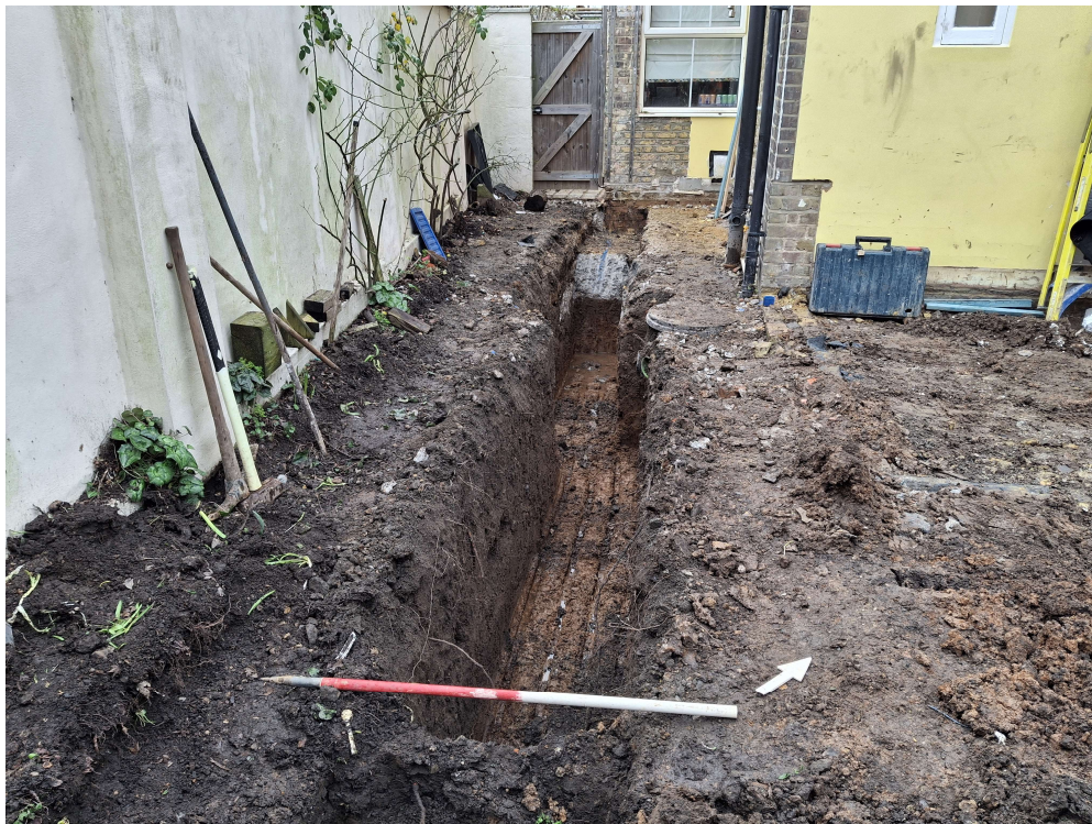
Photograph 1 Foundation trench, looking north-west.
