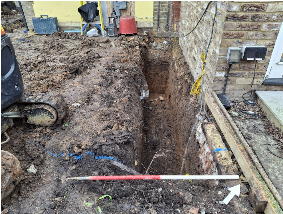
Photograph 2 Foundation trench, looking north-west.
