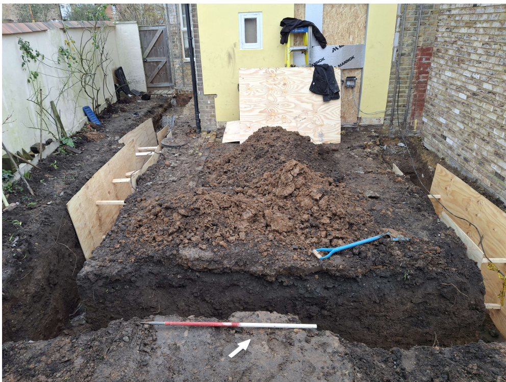
Photograph 3 Foundation trench, looking north-west.
