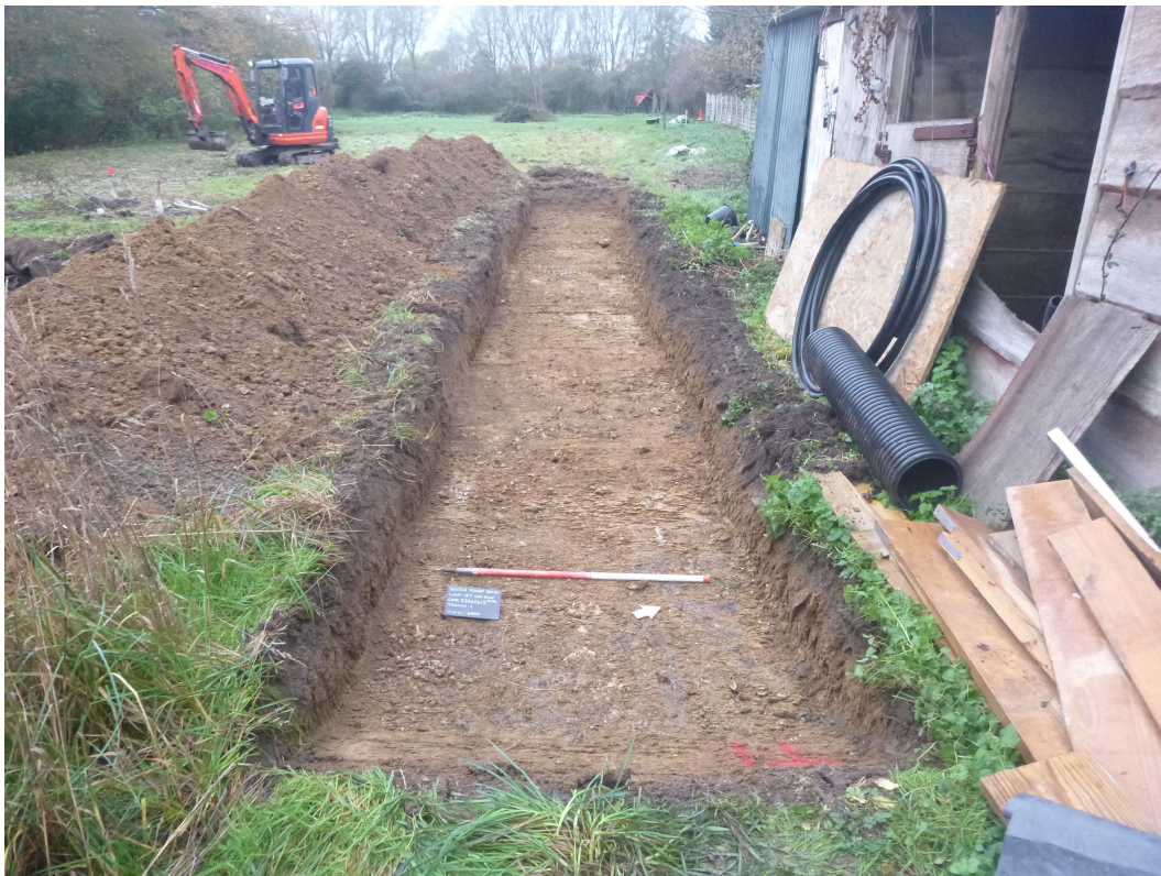
Photograph 1 Trench 1, looking west north-west.
