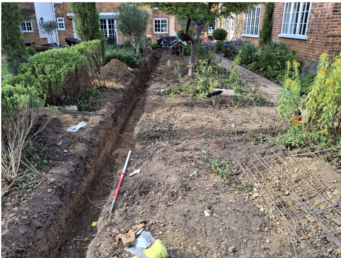
Photograph 1 The garden wall foundation trench, looking north-west.
