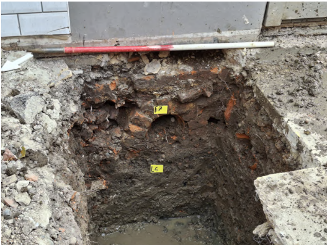
Photograph 9 Representative section of extension foundation trench including culvert F7 and backfill L6, looking south-east.
