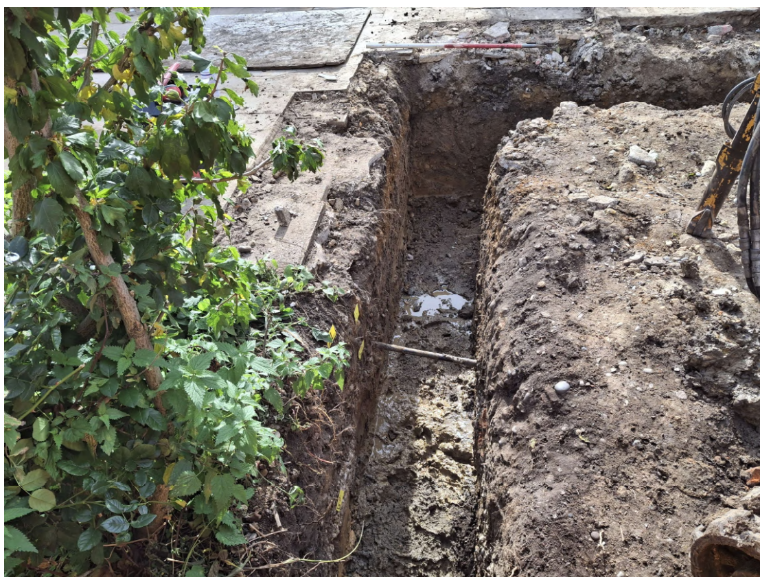
Photograph 6 The extension foundation trench, looking south-west.
