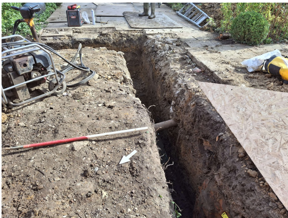
Photograph 5 The extension foundation trench, looking south-east.
