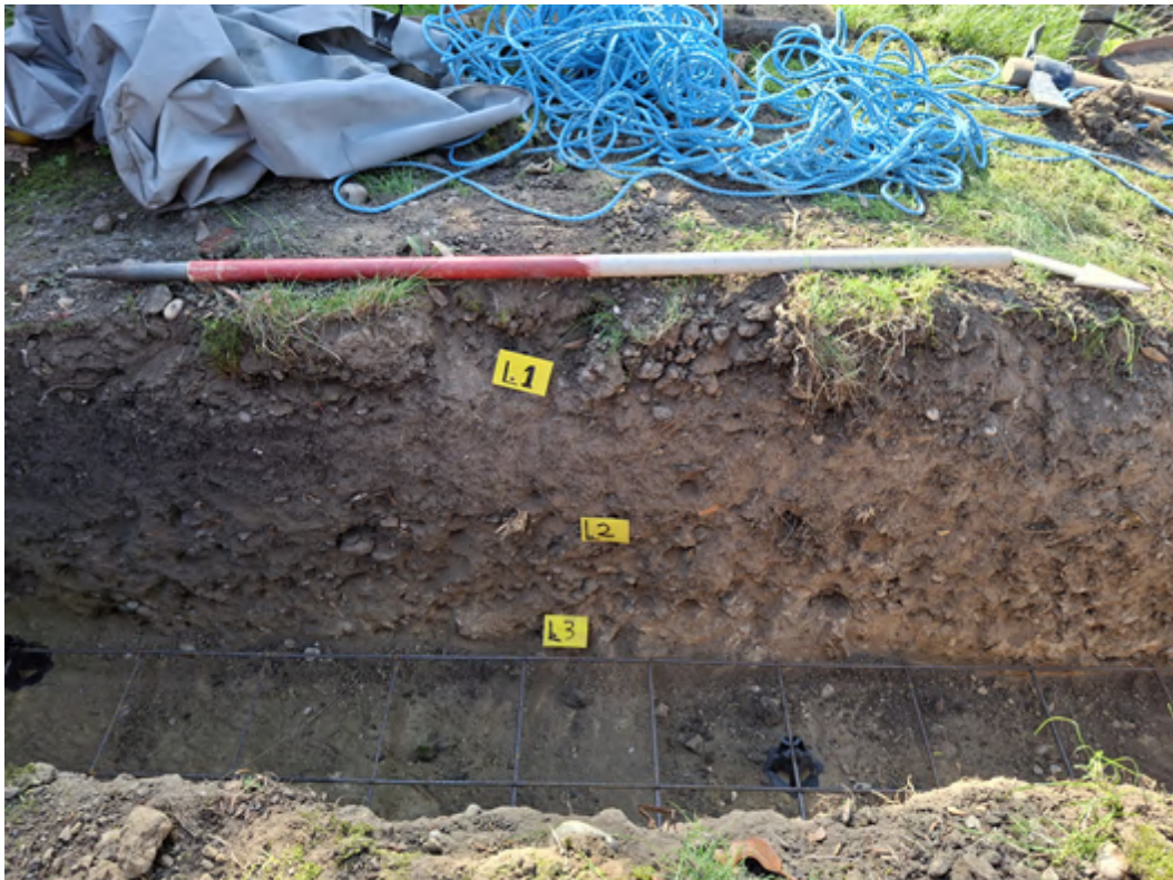
Photograph 4 Representative section of the garden wall foundation trench, looking south-west.
