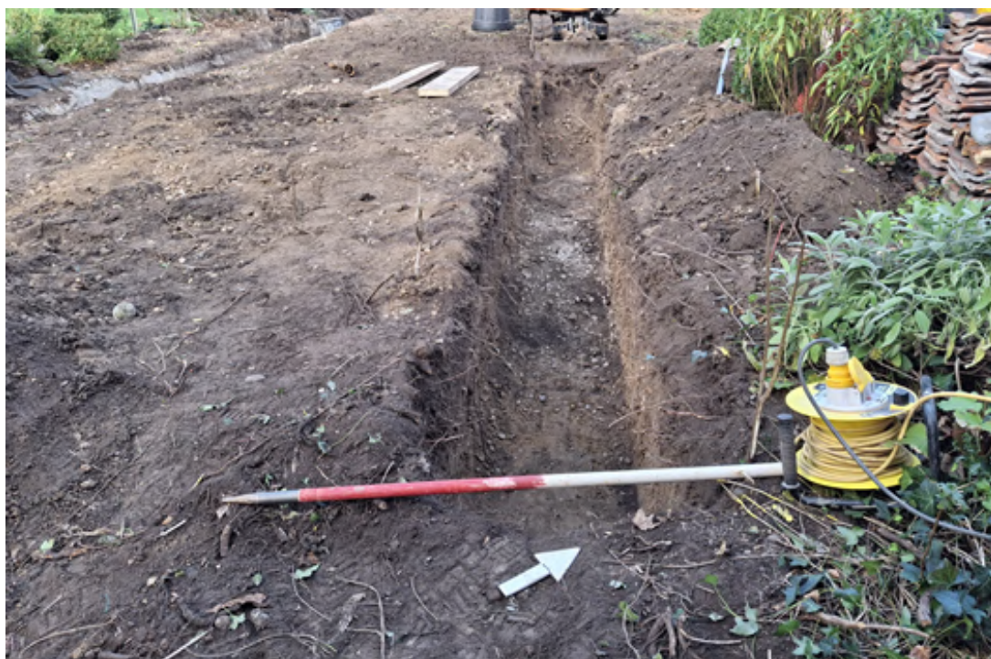
Photograph 11 The soakaway, looking south-east.
