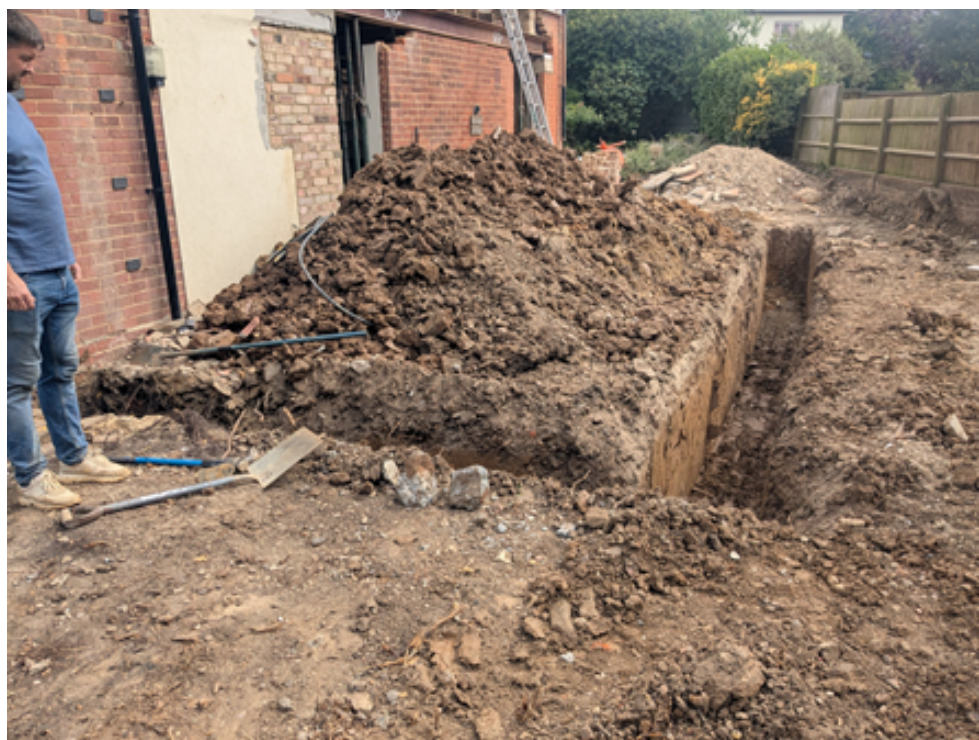
Photograph 1 Foundation trench, view south-east.
