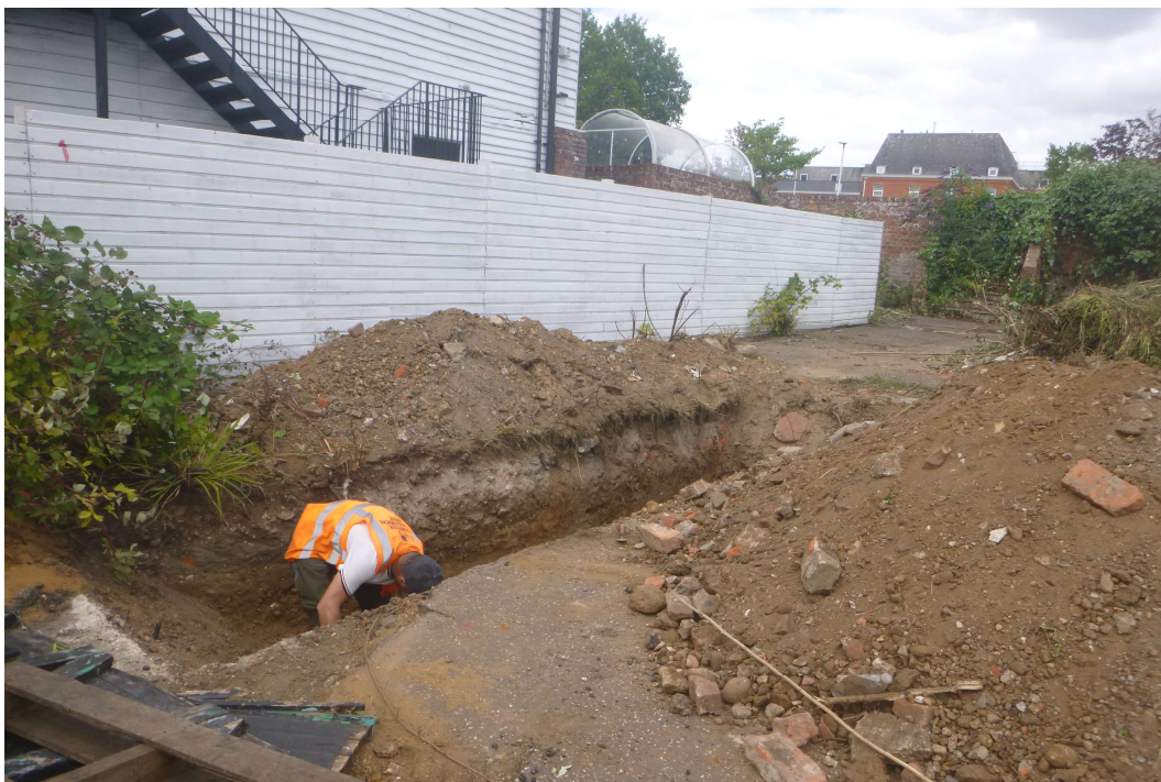
Photograph 1 Trench 1 overview, looking north-west.
