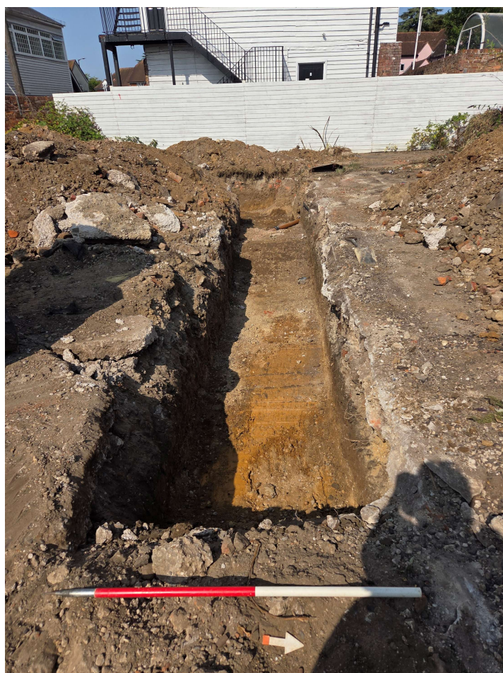
Photograph 3 Trench 2 overview, looking west.
