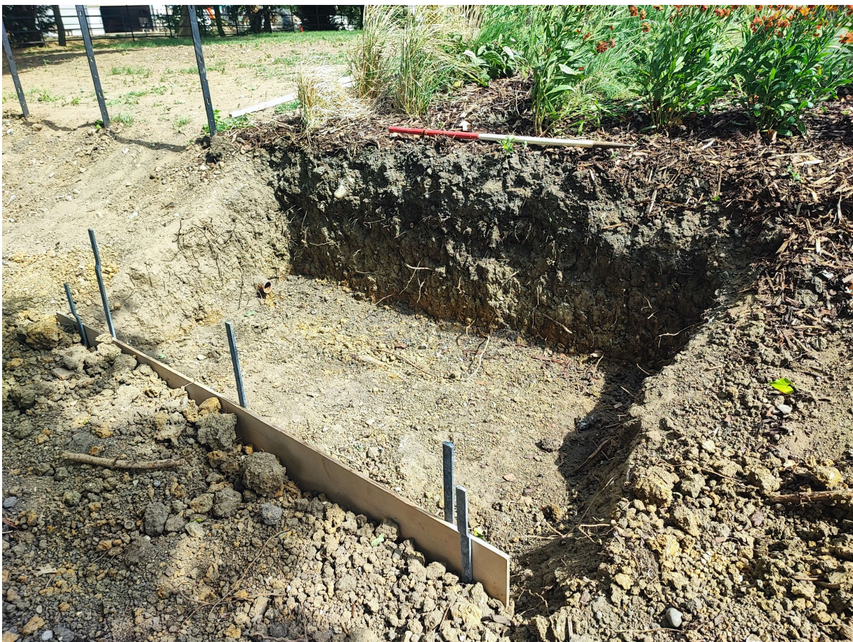
Photograph 1 Pad I, view north.
