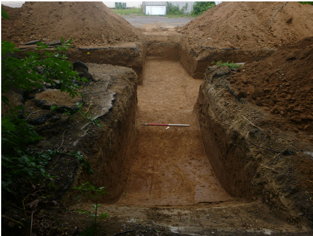
Photograph 2 The trench, view north-west.
