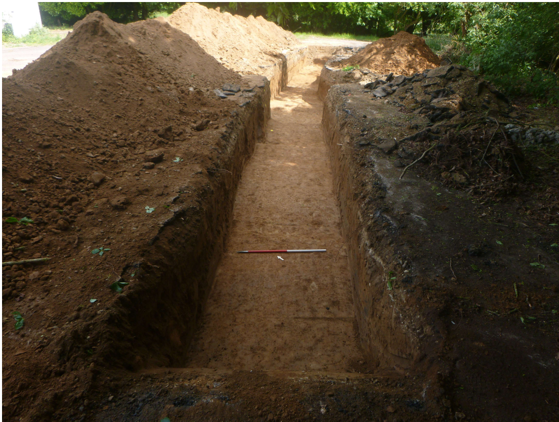
Photograph 1 The trench, view north-east.
