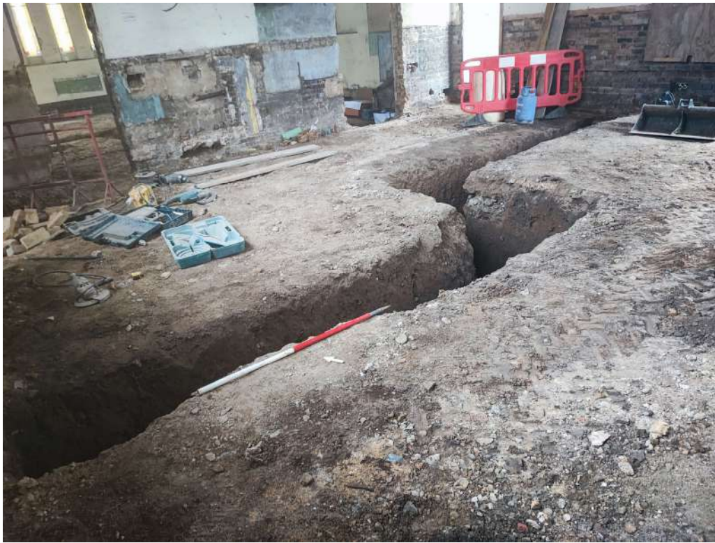
Photograph 3 Trench in plot 2, facing north-east.
