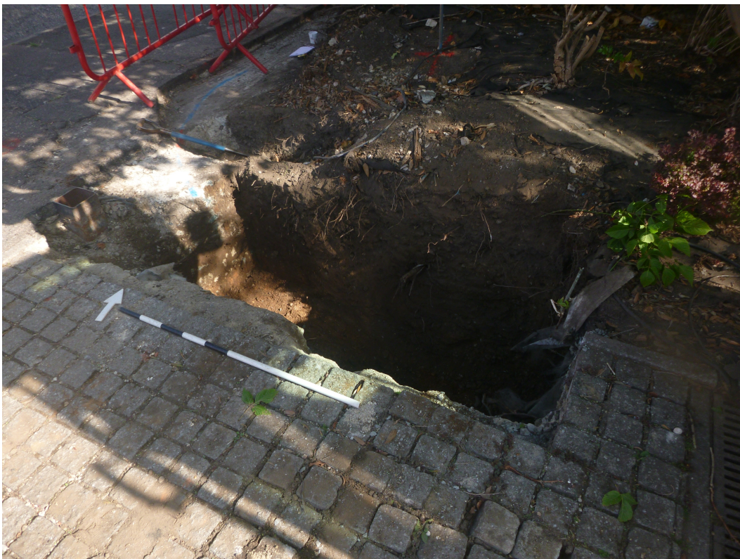
Photograph 3 Foundation trench, looking north.
