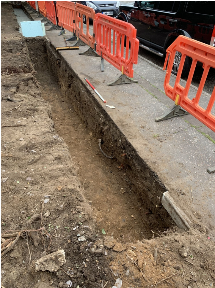
Photograph 5 Foundation trench, looking south-west.
