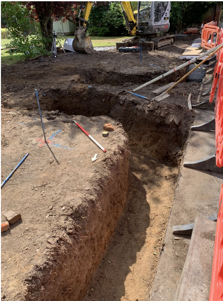
Photograph 6 Foundation pad and trench, looking south.
